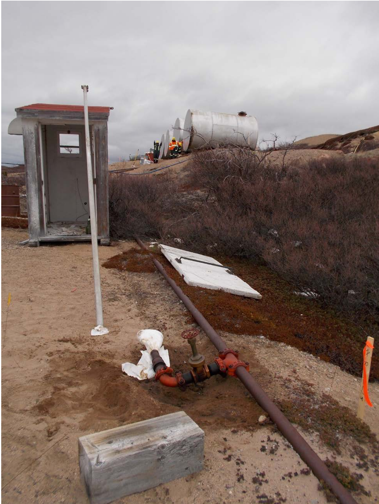
Photo 1: Looking northeast over APEC 1, stained soil beneath the pipeline. APEC 7, small cabin, is visible in the back left, and APEC 9 (Tank 1), APEC 10 (Tank 2), APEC 11 (Tank 3) and APEC 12 (Tank 4) can be seen on the hill in the background.
