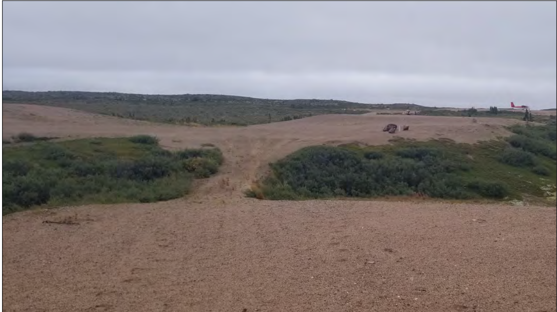
Photo 5: Erosion on Access Road to Weather Station, Viewpoint 118
