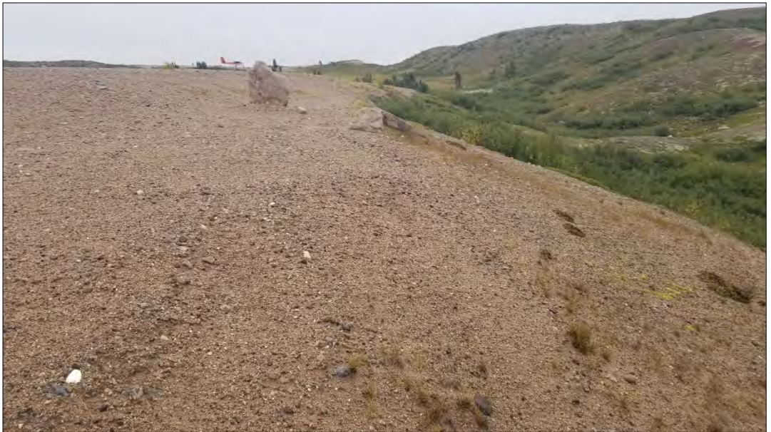
Photo 4: Southeast Corner, Absence of Erosion Channel, Viewpoint 76
