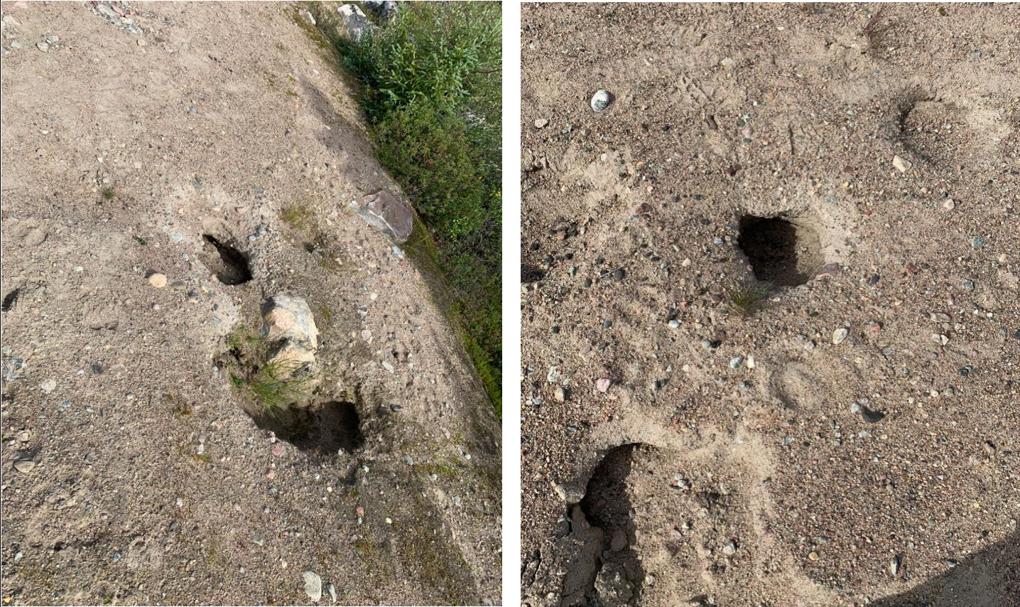
Photograph 1: Settlement Holes in Road between Airstrip and NHWL
