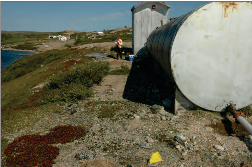
Photo E-6: APEC 4b - Tank 5 - Delineation of tanks; staining can be seen at the valve
