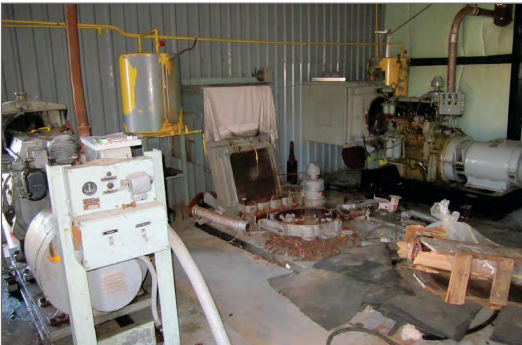
Photo H-26: APEC 15 - Building 2 - Total lead, leachable lead and PCBs painted generators, total lead, leachable lead and PCBs painted plastic over fiberglass insulation, ceiling and concrete floor miscellaneous fluids in generators and lead acid batteries
