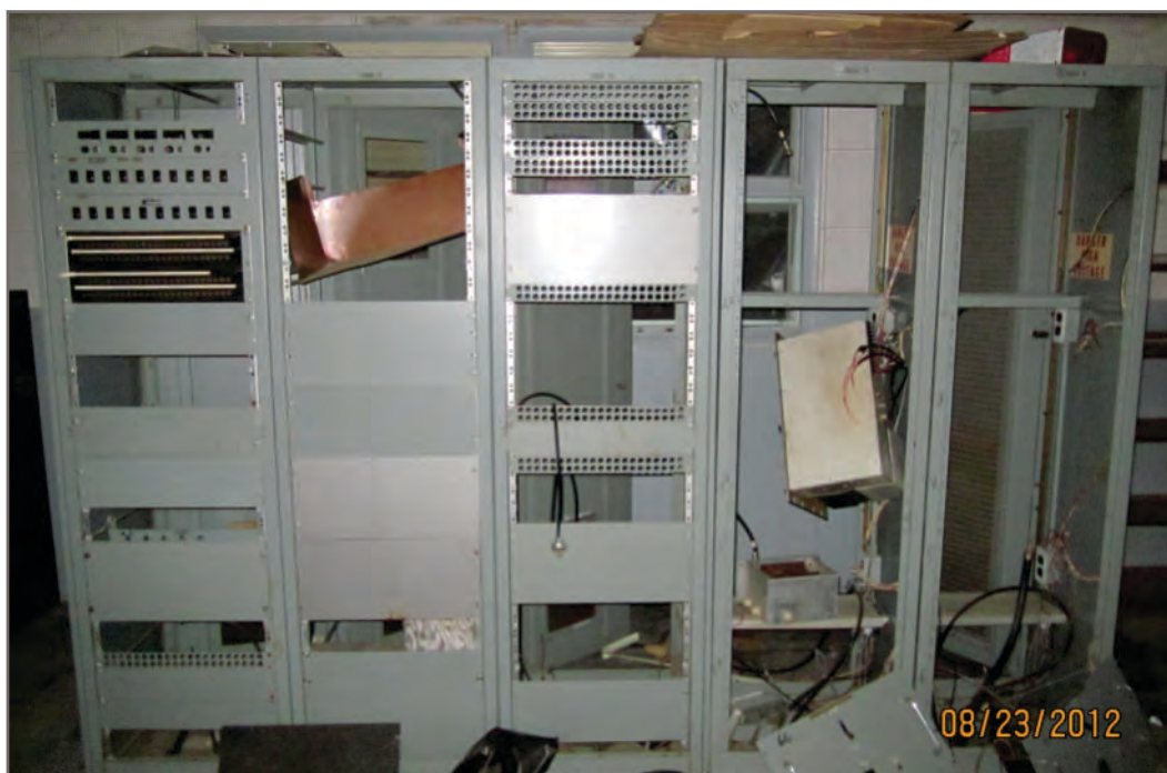
Photo H-22: APEC 14 - Building 1 - Main floor electrical box. Asbestos walls and ceiling, PCBs, mercury and lead solder in electrical parts.
