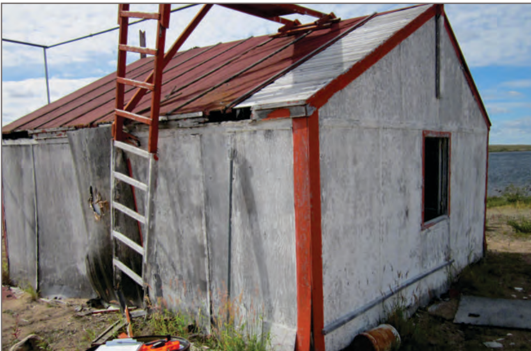
Photo H-28: APEC 16 - Building 3 - Asbestos black felt, attic insulation, window caulking and total lead and leachable lead painted wood
