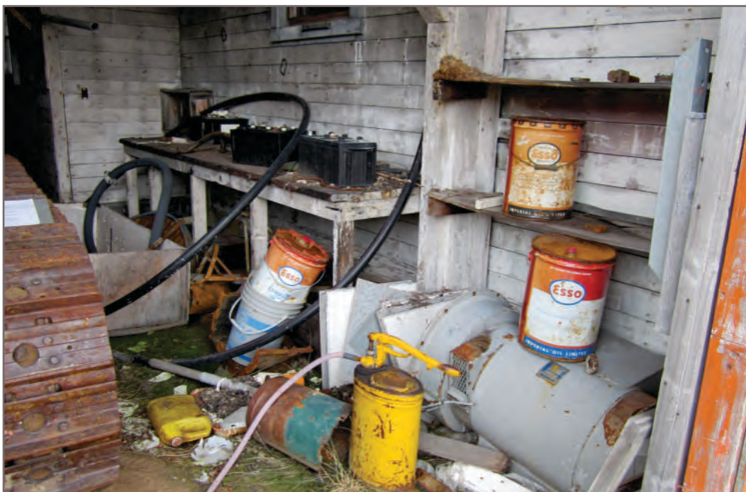
Photo H-35: APEC 18 - Building 5 - Total lead and leachable lead painted wood and equipment, lead acid batteries and miscellaneous containers of oil/lubricants
