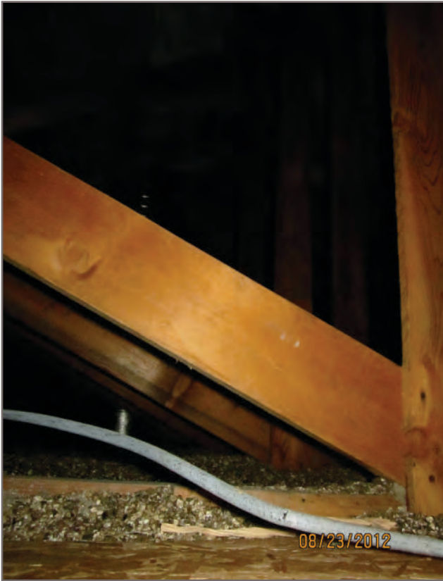
Photo H-23: APEC 14 - Building 1 - Asbestos attic insulation
