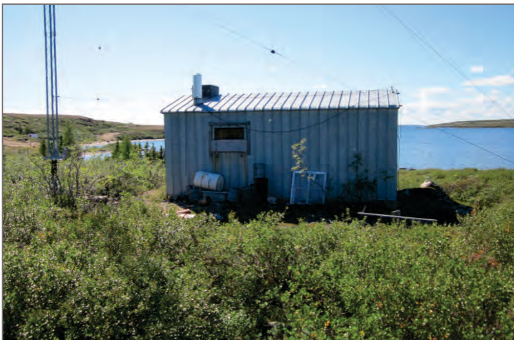
Photo H-46: APEC 22 - Building 9 - Metal exterior and total lead and leachable lead painted metal tower and drums, and drum content (organic)
