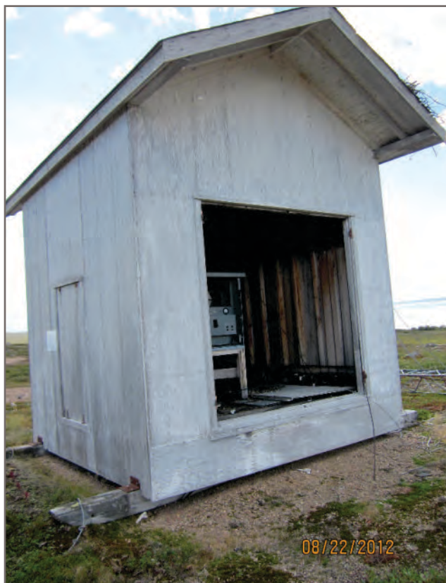
Photo H-61: APEC N/A - Building 10 - Antenna Tuning Unit Shelter, Total lead and leachable lead painted wood and asbestos panel
