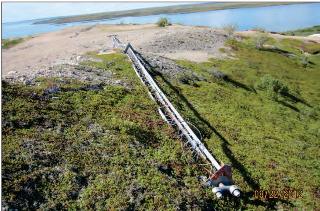
Photo H-64: APEC N/A - Scattered debris throughout and adjacent to the site - Two total lead and leachable lead painted metal towers west of the main building cluster, on the top of the hill
