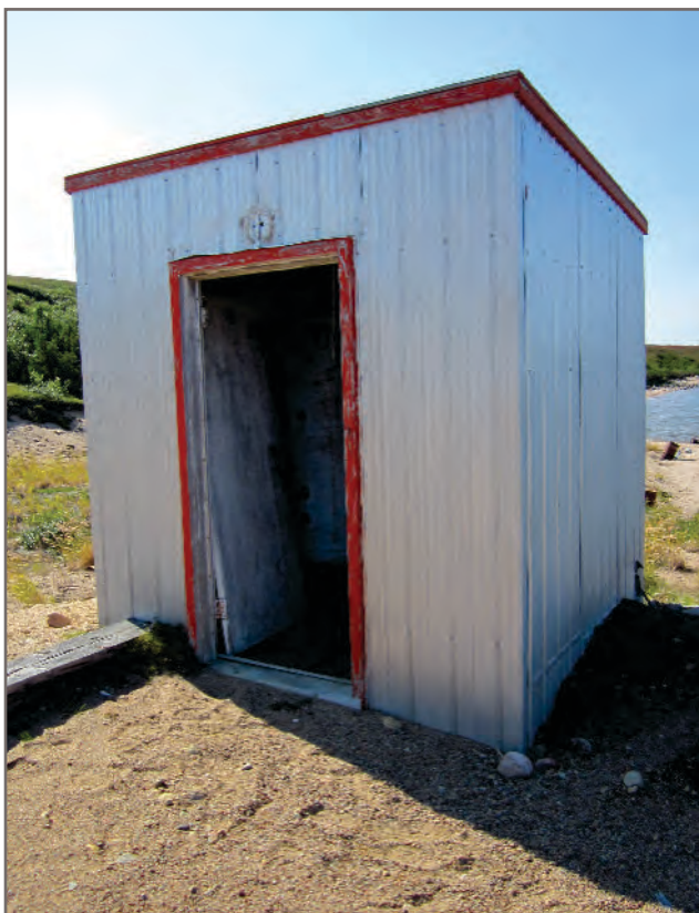
Photo H-58: APEC 29 - Pumphouse - Asbestos black felt, total lead and leachable lead painted equipment and wood
