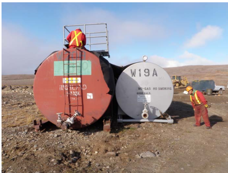
Photo 6 (P9080025) Sample 10-36449 Fox-3: Wastewater Tank (grey) that contains Barrel Rinse water and wastewater from Barrel Processing Area # 1.
