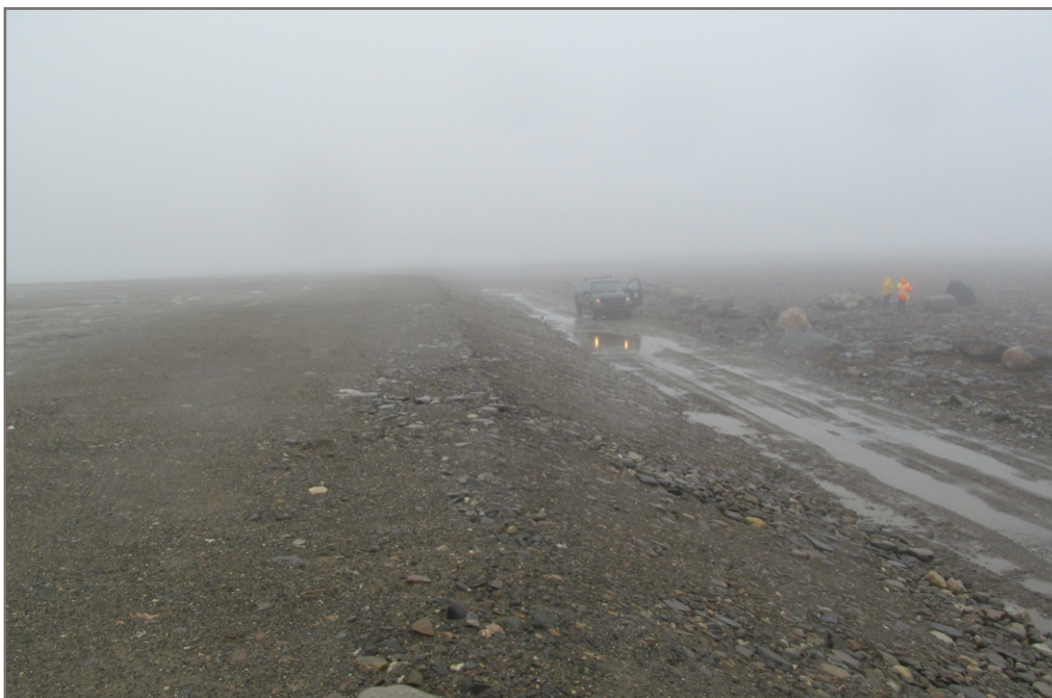
PHOTO 13 IMG 0070: Non-Hazardous Waste Landfill - Minor water ponding along north side of landfill.
