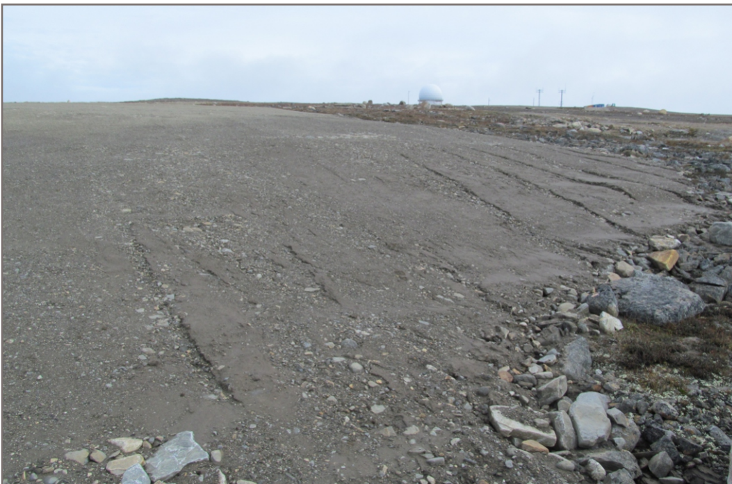
PHOTO 12 IMG 0141: Station West Landfill - Minor erosion noted along south sideslope of Lobe F.
