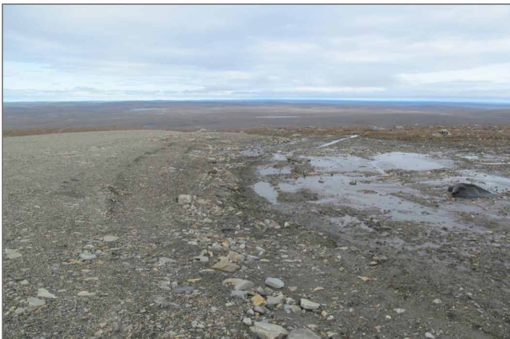
PHOTO 10 IMG 0125: Station West Landfill - Area of ponded water noted along north side of Lobe E2.
