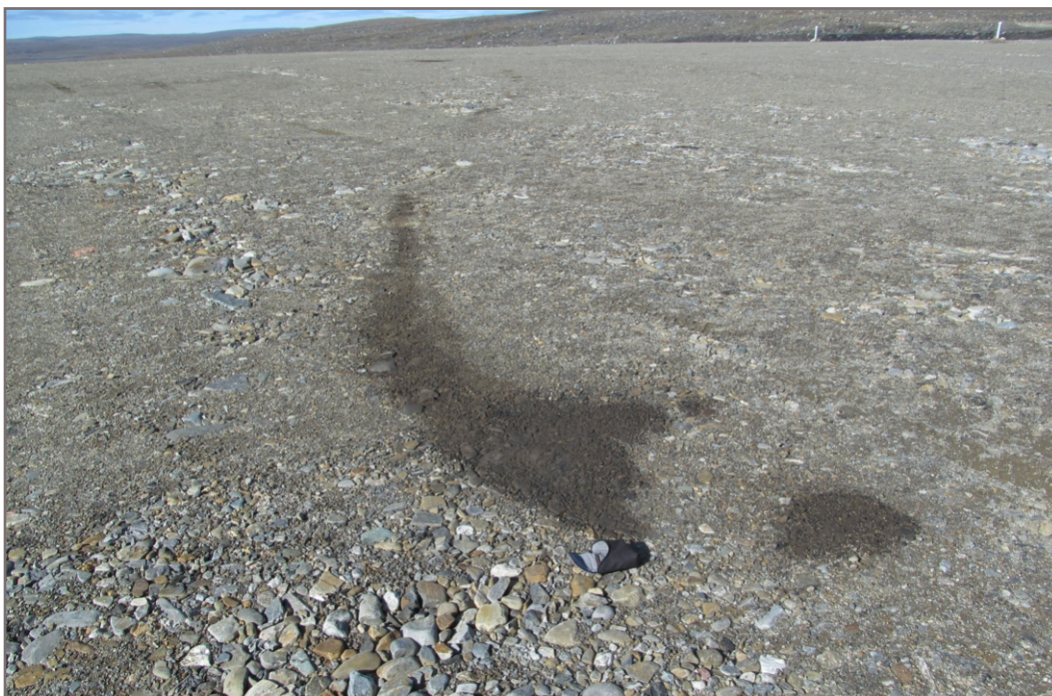
PHOTO 22 IMG 0195: Tier II Disposal Facility - Hydrocarbon staining on the surface of the facility at various locations as shown on Figure FOX-3.5.
