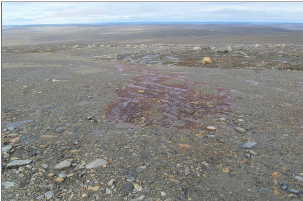
PHOTO 8 IMG 0115: Station West Landfill - Iron staining along northwest portion of Lobe A.
