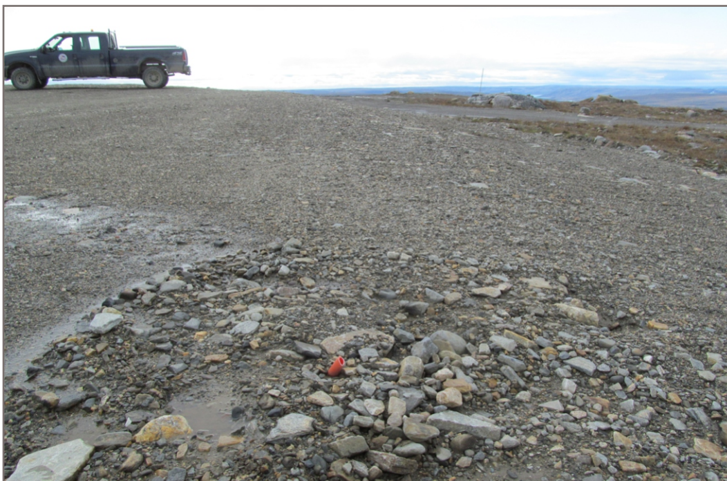
PHOTO 6 IMG 0123: Station West Landfill - Plastic Pipe protruding from the landfill at south end of Lobe A.
