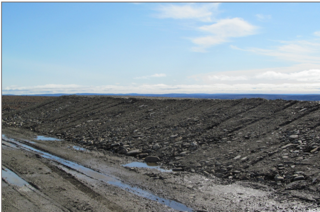
PHOTO 14 IMG 0183: Non-Hazardous Waste Landfill - Minor erosion along northeast sideslope of landfill.
