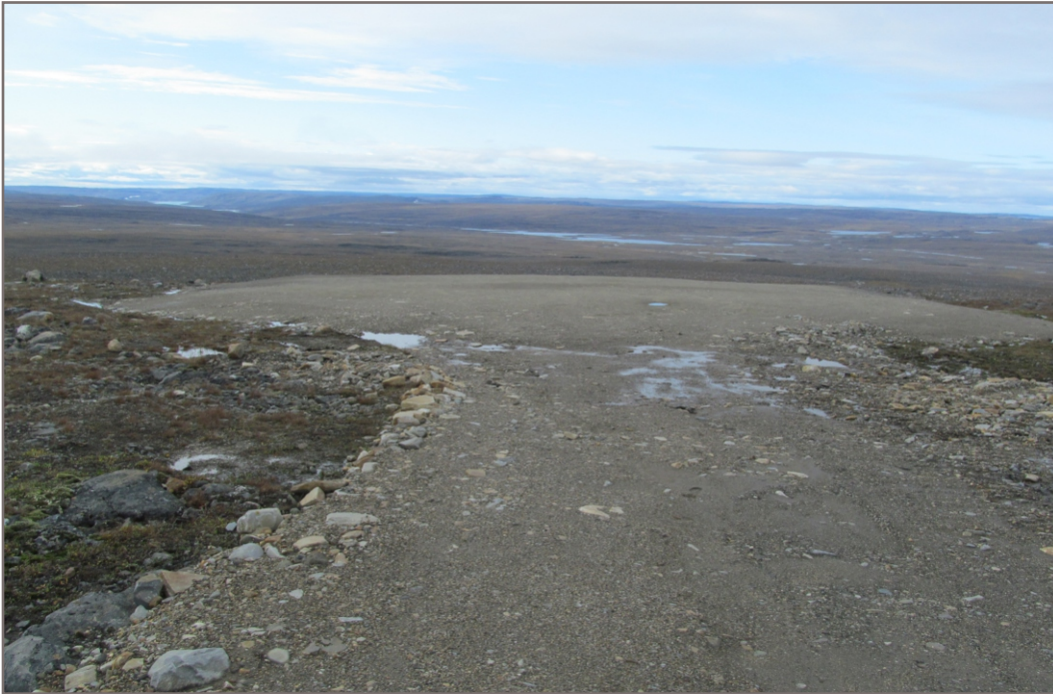
PHOTO 11 IMG 0132: Station West Landfill - Small isolated depression of ponded water noted at north end of Lobe F.
