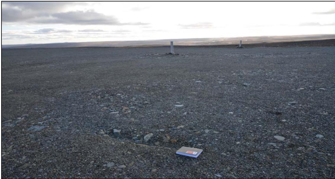
Figure 13: Photo – 2013-F3-TII-44 - Feature B - View SW - of minor linear depression on the northern landfill surface. New observation.
