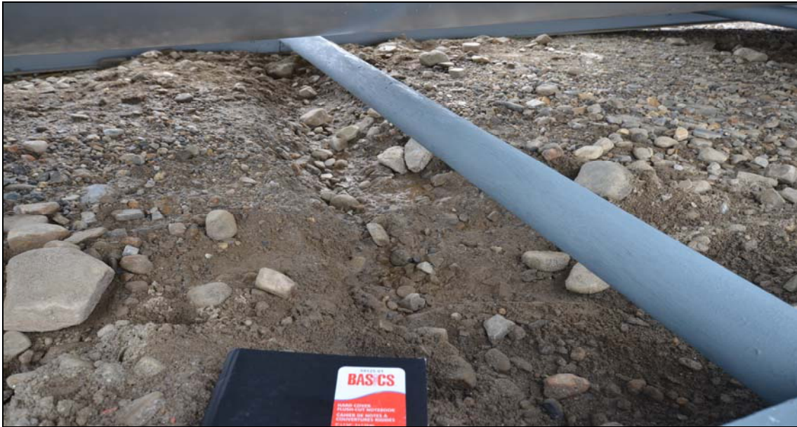
Figure 1: Photo - 2013-F3-SW-20 - Feature F - Close-up of linear depression under cross beam of fuel tankbase located on Lobe A - (new observation).
