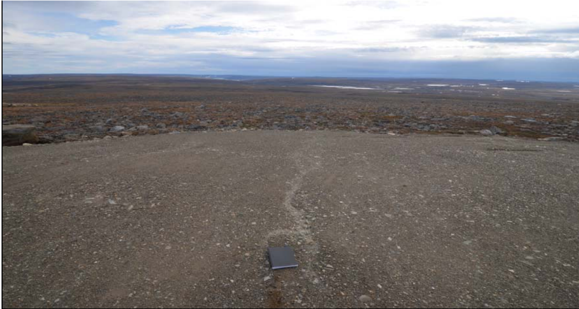
Figure 3: Photo - Feature M - view S of erosion channel extending from the landfill surface to the southwestern toe of the lobe, taken from the top of the channel on Lobe F - (new observation).
