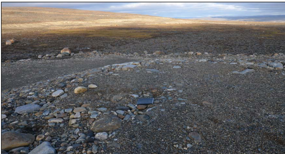
Figure 12: Photo – 2013-F3-TII-42 - Feature A - View SW - of minor depression on the landfill surface at the northeast corner. New observation.
