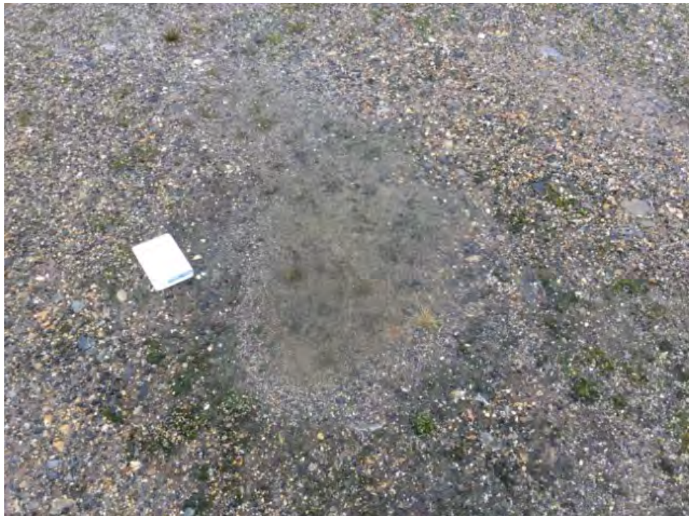
Photo 98: Station West Landfill, Lobe F – Feature K, shallow depression with ponded water (ATT222_Photo1.jpg)
