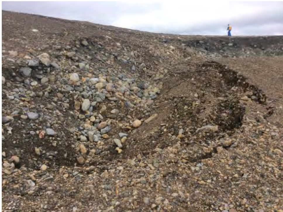
Photo E2: Thermokarst – Edge of thaw settlement – Feature A (ATT31_Photo1.jpg)
