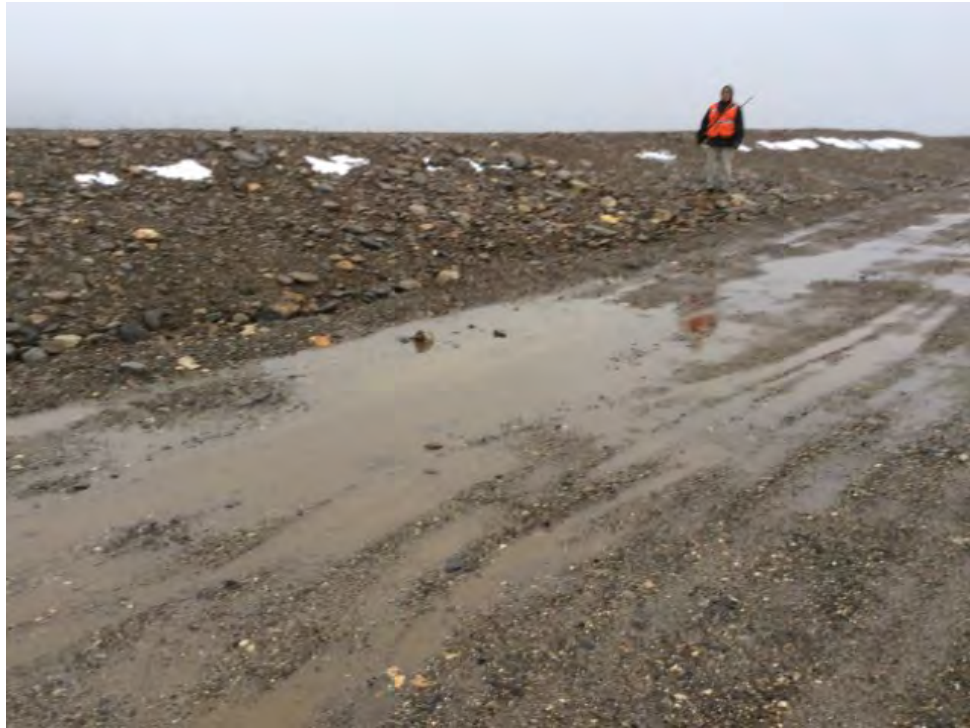
Photo 59: Non-Haz Waste Landfill – Feature F, ponded water along north toe, facing west (ATT172_Photo2.jpg)
