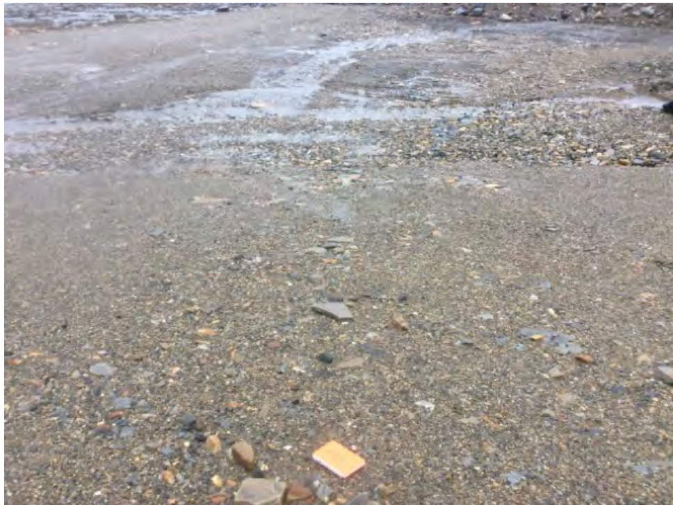
Photo 10: West Landfill – Feature H, minor self-armouring erosion channel on north slope, looking north (ATT18_Photo1.jpg)
