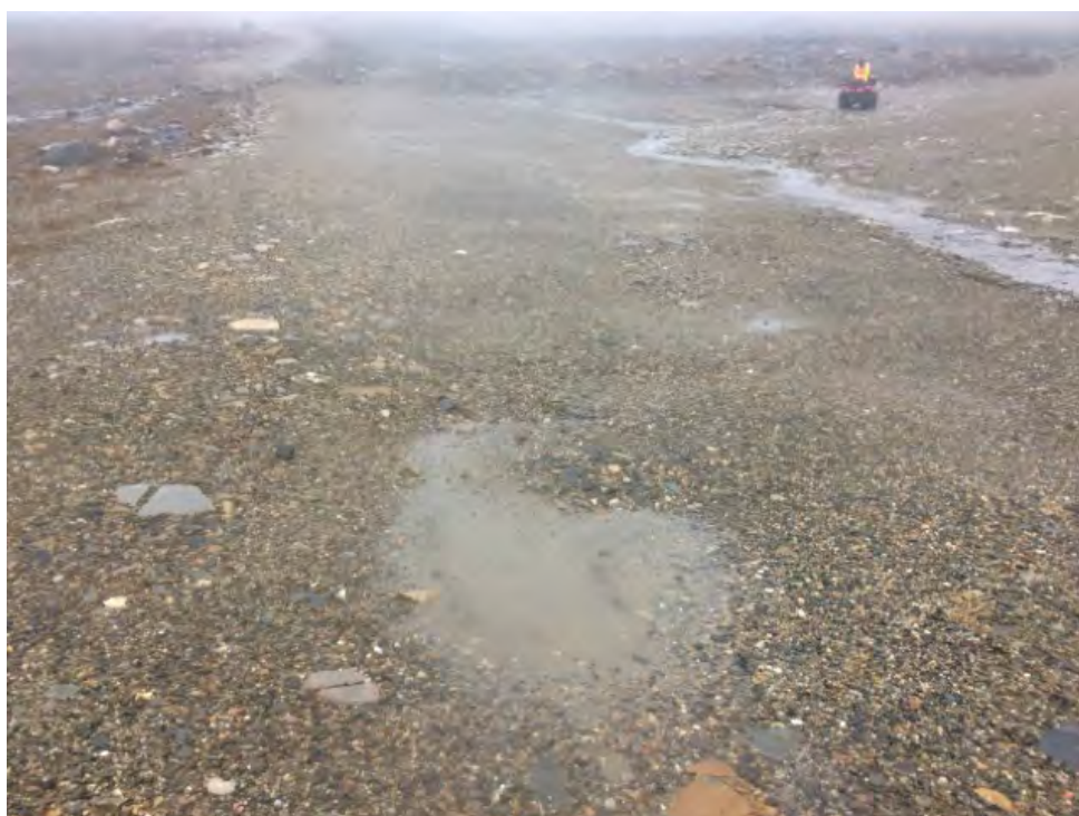
Photo 18: West Landfill – Feature D, ponded water and drainage channel along access road (ATT29_Photo1.jpg)
