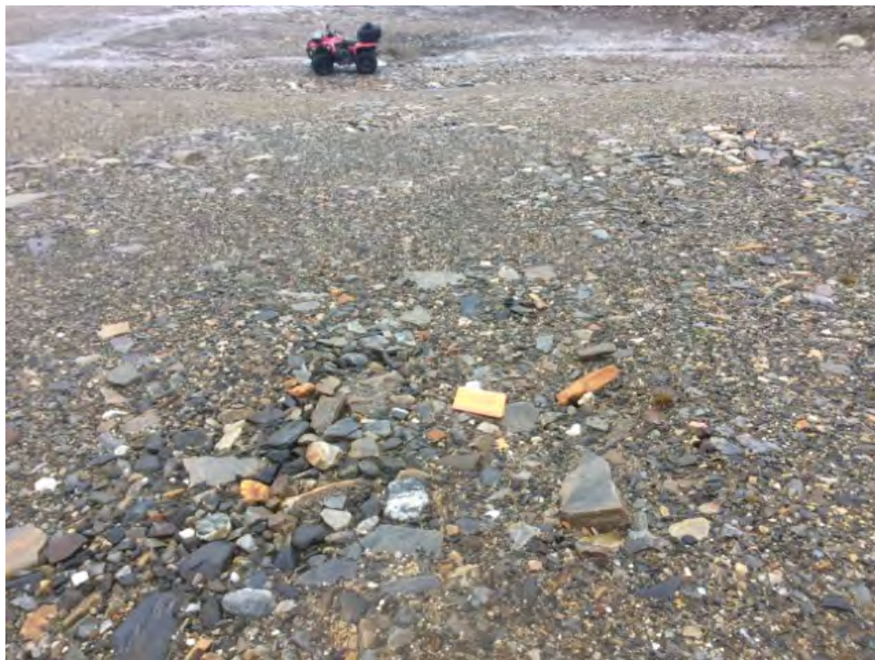
Photo 11: West Landfill – Feature A, minor settlement and rough area on the cover surface (ATT19_Photo1.jpg)
