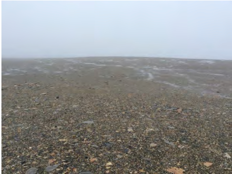
Photo 81: Station West Landfill, Lobe A – Cover surface facing northwest, shallow depressions with ponded water (previous Feature E) and shallow runoff channels (previous Feature U) in background (ATT193_Photo1.jpg)
