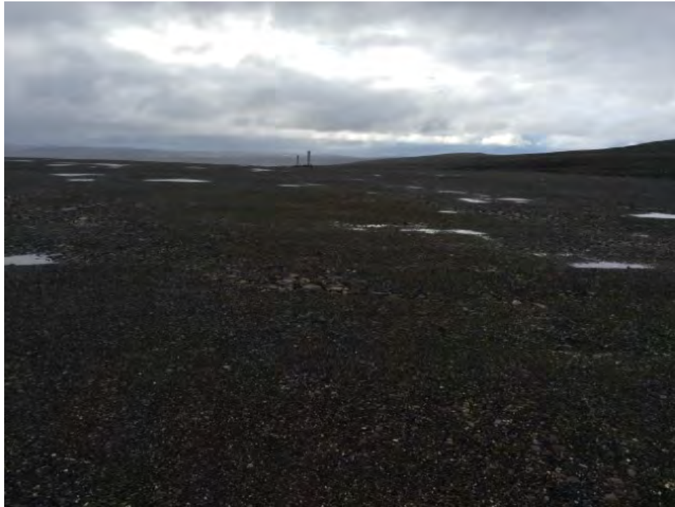
Photo 27: Tier II Disposal Facility – Ponded water on cover surface, previously reported Features A and B (settlement) and Feature H, facing west (ATT123_Photo1.jpg)
