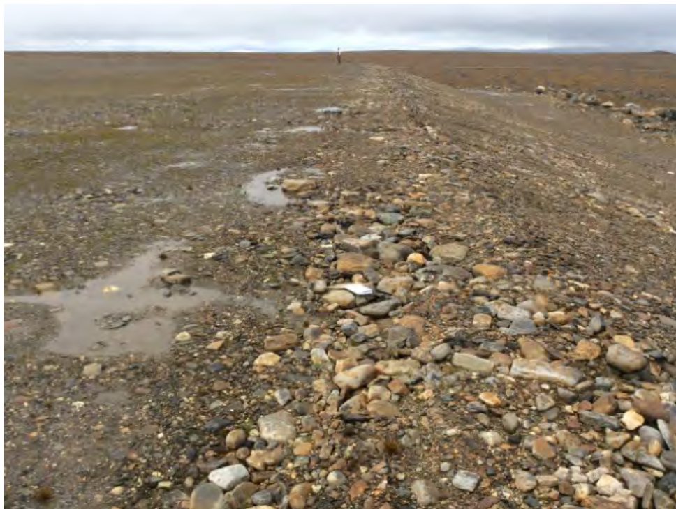
Photo 47: Non-Haz Waste Landfill – South crest edge, facing east, previous reported crack (Feature D) appears to be coarser fill on slope near crest edge (ATT152_Photo1.jpg)
