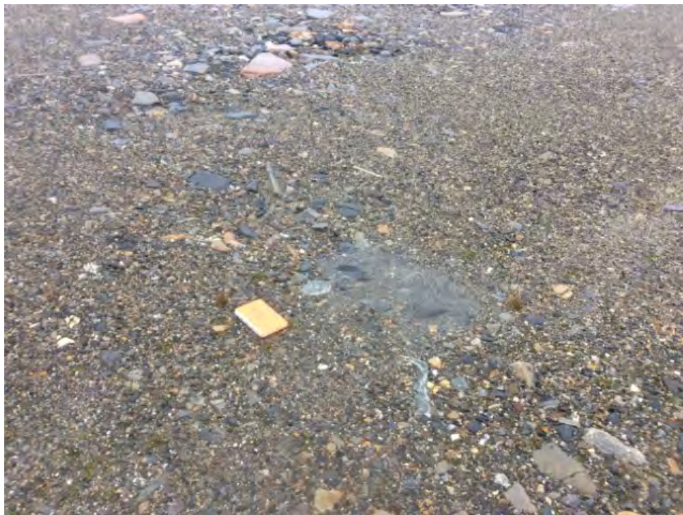
Photo 13: West Landfill – Feature B, ponded water, previously reported as settlement, 1 x 1 m (ATT22_Photo1.jpg)
