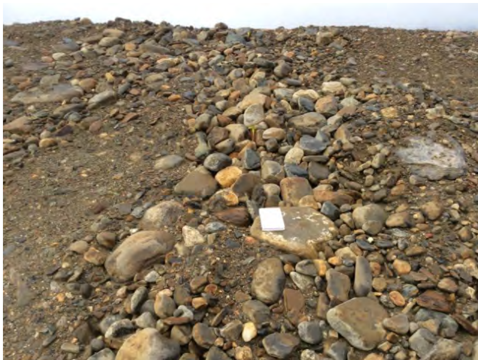
Photo 45: Non-Haz Waste Landfill – Feature I, self-armouring erosion on west slope (ATT150_Photo1.jpg)
