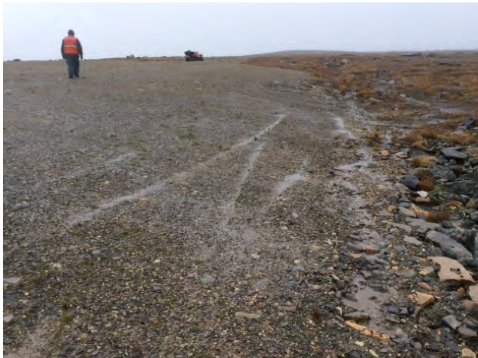
Photo 106: Station West Landfill, Lobe F – East slope, facing north, water running along toe (Feature AB) (ATT231_Photo1.jpg)
