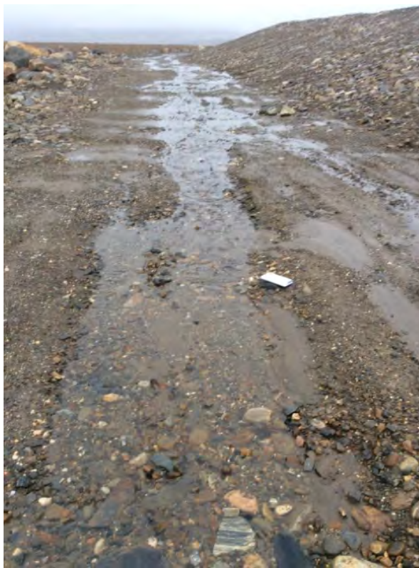
Photo 53: Non-Haz Waste Landfill – Feature K, water running along east toe (ATT160_Photo1.jpg)
