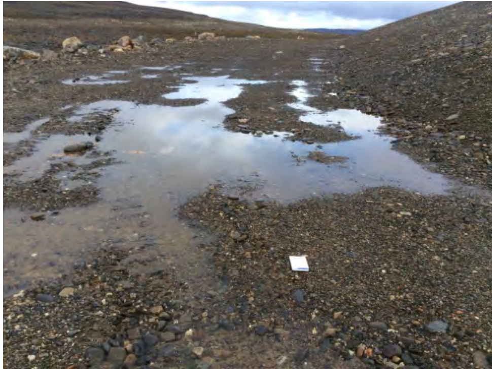
Photo 31: Tier II Disposal Facility – Feature J, ponded water at northwest toe (ATT128_Photo1.jpg)
