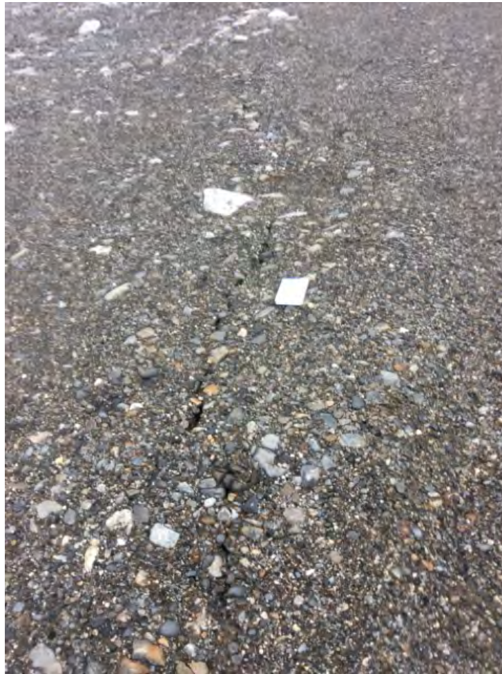
Photo E18: Thermokarst – Feature E - small crack on slope down to filled settlement area (ATT47_Photo1.jpg)
