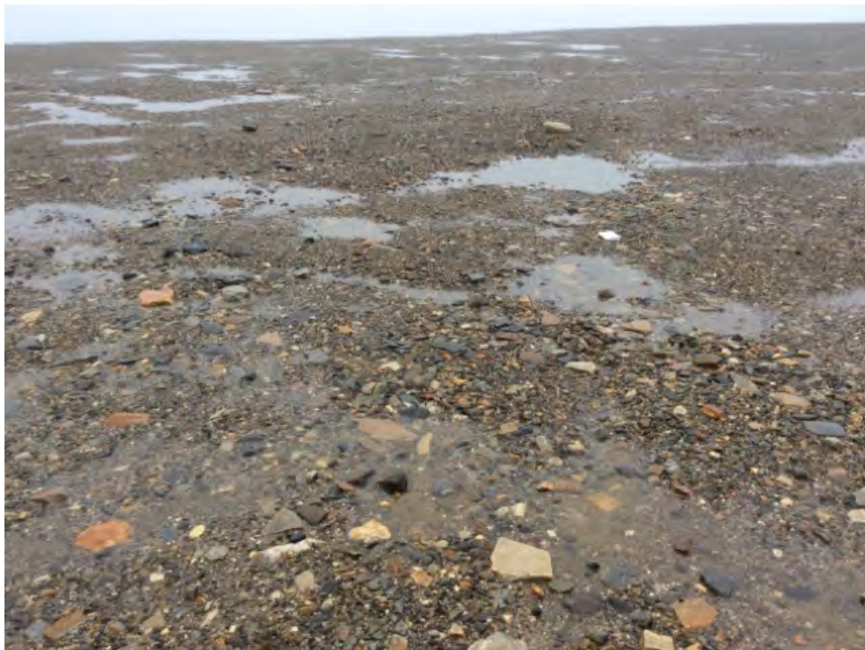
Photo 80: Station West Landfill, Lobe A – Shallow depressions with ponded water (previous Feature W) (ATT192_Photo1.jpg)
