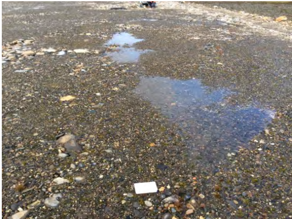
Photo 24: Tier II Disposal Facility – Feature I, ponded water on crest surface in southeast corner (ATT118_Photo1.jpg)
