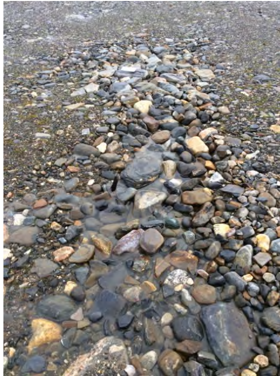
Photo 39: Tier II Disposal Facility – Feature M, cobbles and boulders on cover surface with ponded water (ATT141_Photo1.jpg)
