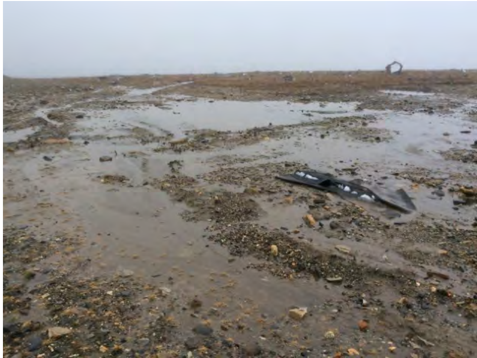
Photo 91: Station West Landfill, Lobe E2 – North toe, geotextile (previous Feature I) surrounded by ponded water (Feature AA) (ATT206_Photo1.jpg)
