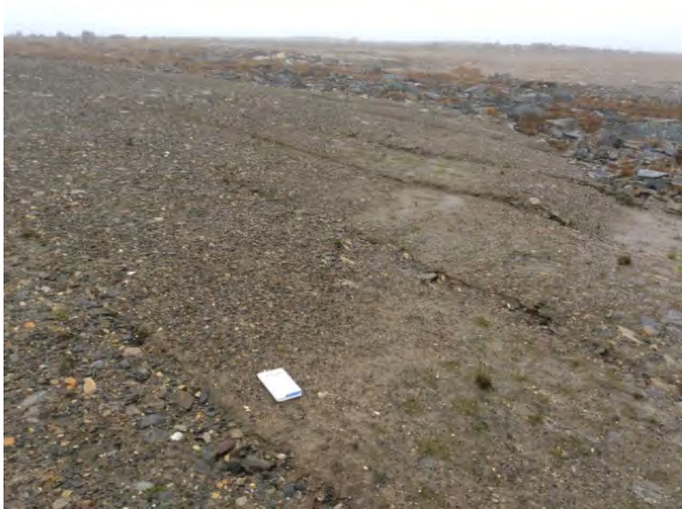
Photo 103: Station West Landfill, Lobe F – Feature P, minor self-armouring erosion from linear equipment tracks (ATT228_Photo1.jpg)
