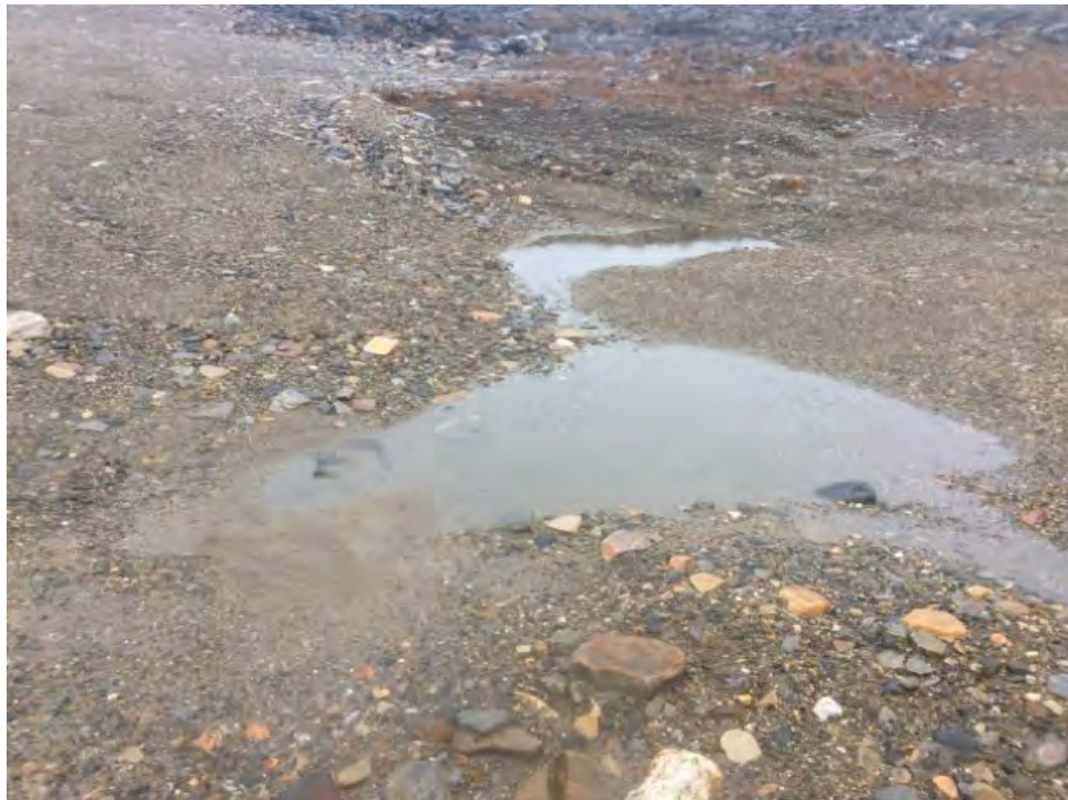
Photo 4: West Landfill – Feature G, ponded water at south toe (ATT10_Photo1.jpg)
