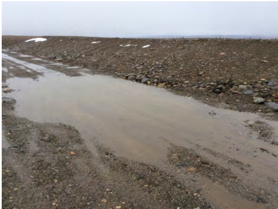
Photo 58: Non-Haz Waste Landfill – Feature F, ponded water along north toe, facing east (ATT171_Photo1.jpg)
