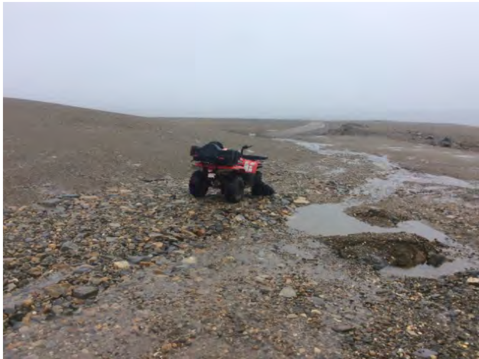
Photo 8: West Landfill – Feature D, ponded water at north toe, looking west (ATT14_Photo1.jpg)
