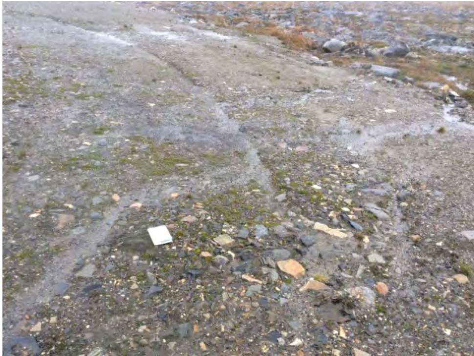
Photo 101: Station West Landfill, Lobe F – Feature M, minor self-armouring erosion on southwest slope (ATT226_Photo1.jpg)
