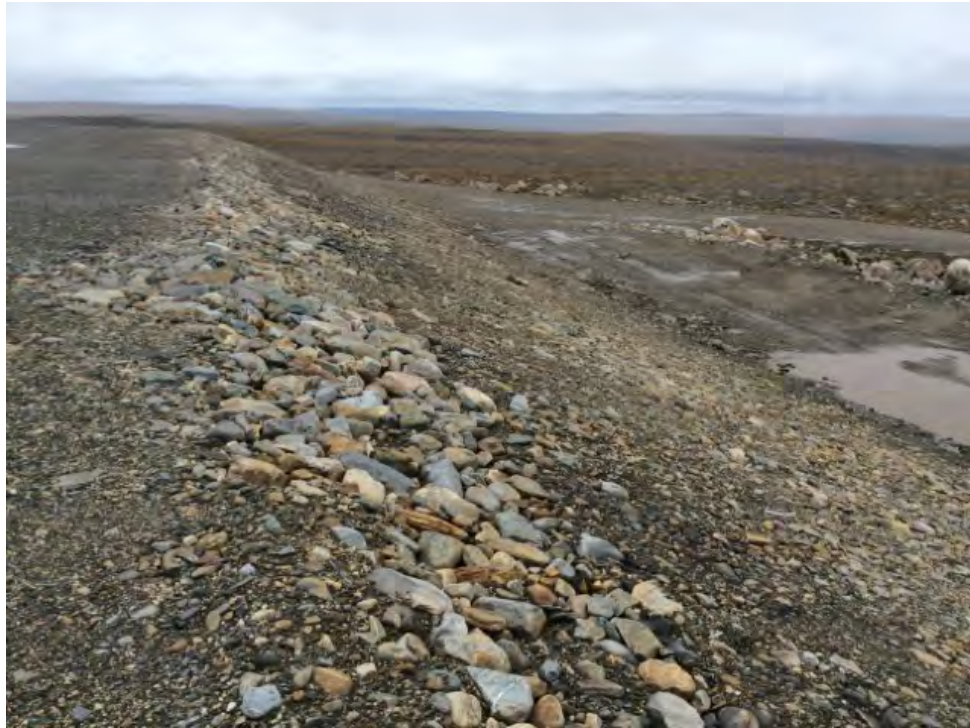
Photo 33: Tier II Disposal Facility – West crest edge, facing south, ponded water at toe (Feature K) (ATT135_Photo1.jpg)
