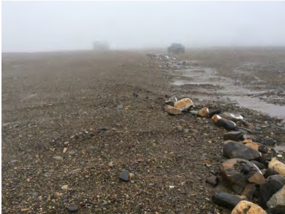
Photo 79: Station West Landfill, Lobe A – Southeast crest edge, facing northeast, ponded/running water along toe (new Feature X) (ATT191_Photo1.jpg)
