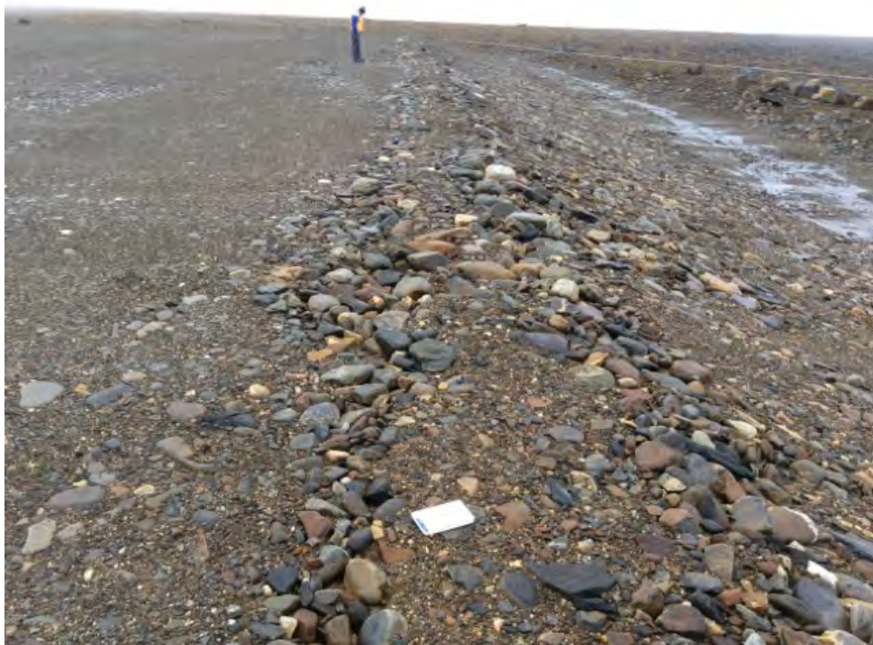
Photo 52: Non-Haz Waste Landfill – East crest edge, facing north, coarse boulders at crest edge where fines have washed out (ATT159_Photo1.jpg)
