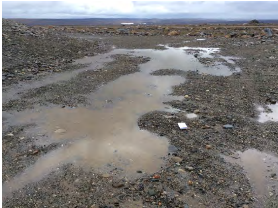
Photo 30: Tier II Disposal Facility – Feature J, ponded water at northwest toe (ATT127_Photo1.jpg)
