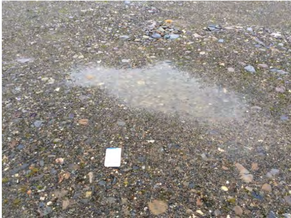
Photo 63: Non-Haz Waste Landfill – Feature M, shallow depression with ponded water (ATT167_Photo1.jpg)
