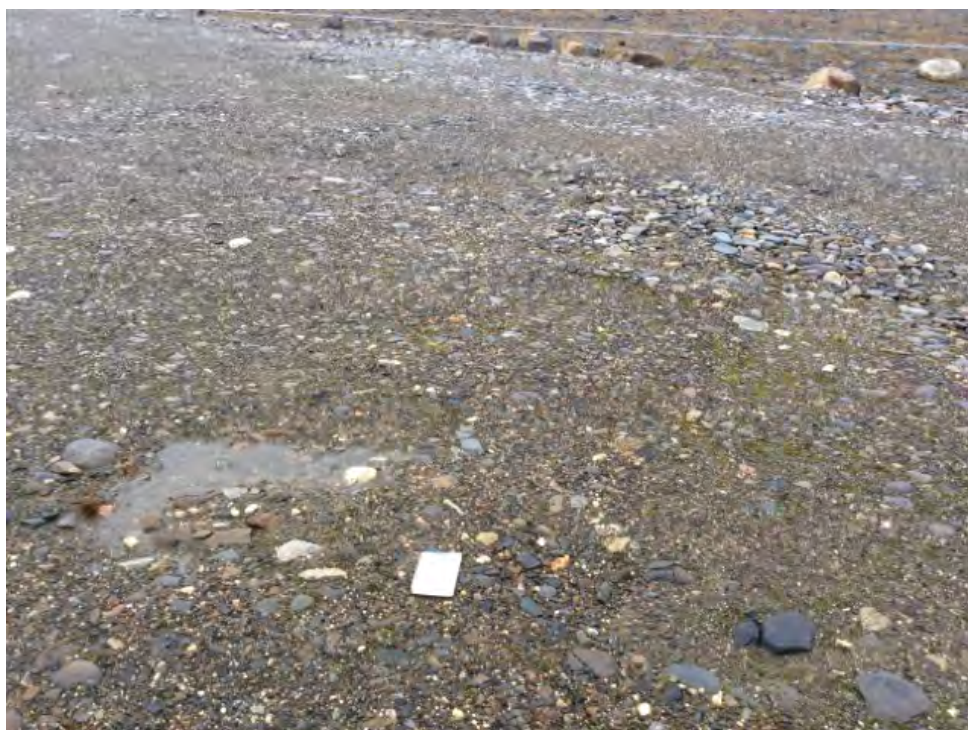
Photo 62: Non-Haz Waste Landfill – previously observed Features A and B, small depressions with ponded water (ATT166_Photo1.jpg)
