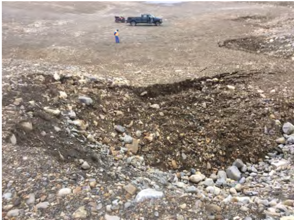
Photo E5: Thermokarst – Feature A - thaw settlement perimeter (ATT34_Photo1.jpg)
