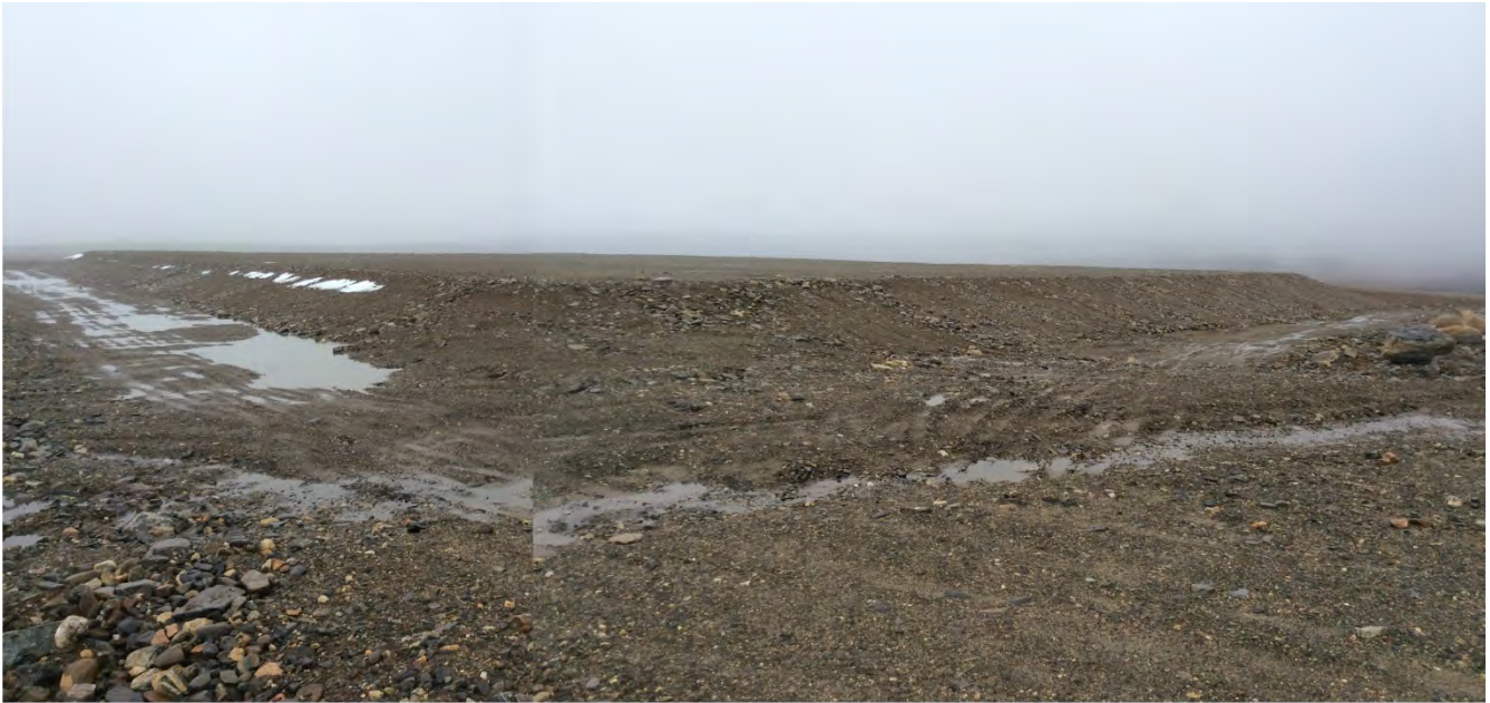
Photo 65: Non-Haz Waste Landfill – North and west slopes, ponded water along north toe (Feature F), ponded water along west toe (Feature H) (ATT174_Photo1.jpg) (ATT175_Photo2.jpg)
