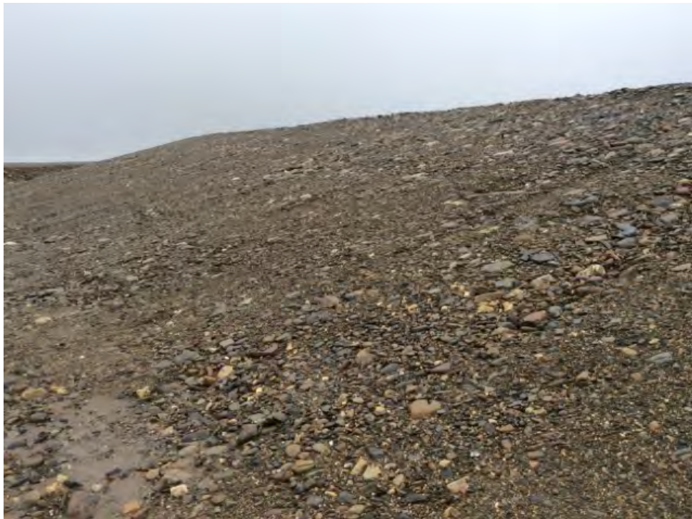
Photo 50: Non-Haz Waste Landfill – South slope facing northwest, some self-armouring erosion leaving cobbles and boulders (ATT155_Photo1.jpg)
