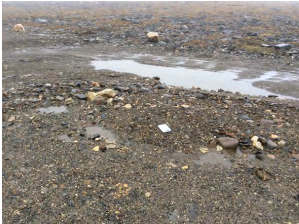
Photo 60: Non-Haz Waste Landfill – Small depressions with ponded water on northwest crest corner (Feature L), ponded water at the toe (Feature F) (ATT173_Photo1.jpg)
