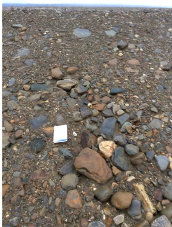
Photo 56: Non-Haz Waste Landfill – Feature C, previously noted erosion on north slope is self-armouring (ATT164_Photo1.jpg)
