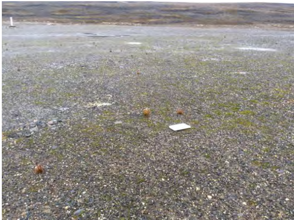
Photo 38: Tier II Disposal Facility – very sparse vegetation on cover surface (Feature L), depression with ponded water in background (Feature H) (ATT140_Photo1.jpg)
