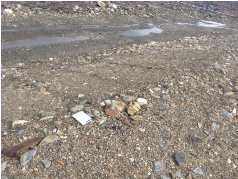
Photo 21: FOX-3 – Non Hazardous Waste Landfill – North slope – Feature C – self-armouring erosion [Acceptable], facing northeast (ATT35_Photo35.jpg)
