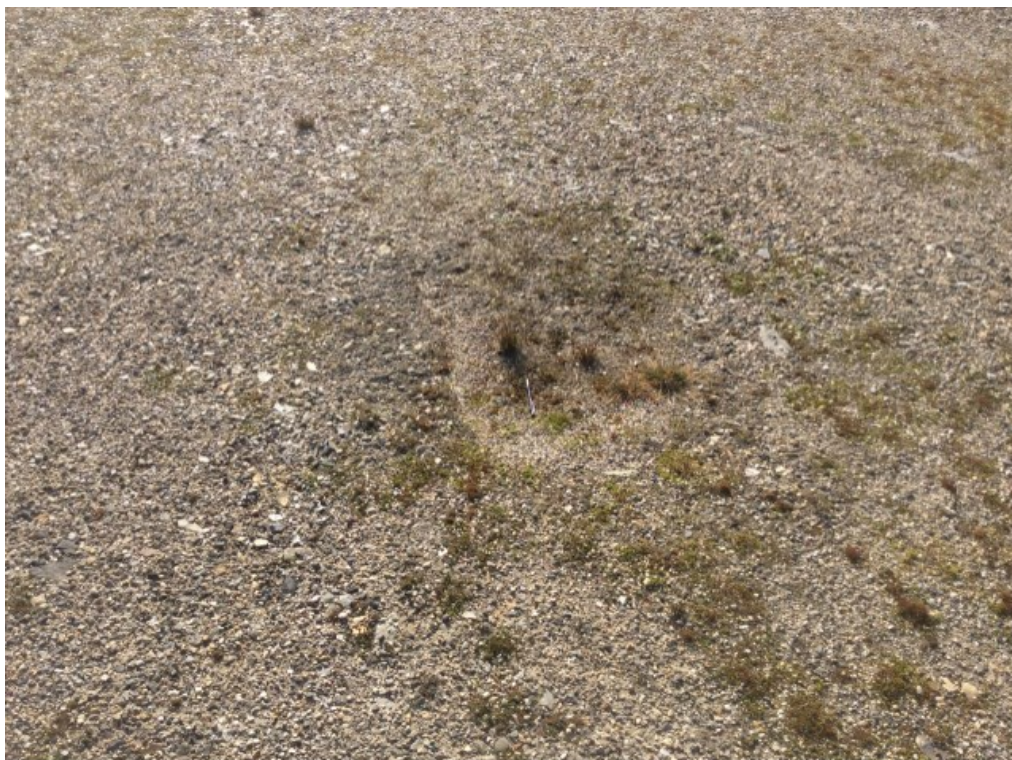
Photo 84: FOX-3 – Station West Landfill – Lobe F, north crest surface – Feature K – shallow depression [Acceptable], facing southwest (ATT30_Photo30.jpg)
