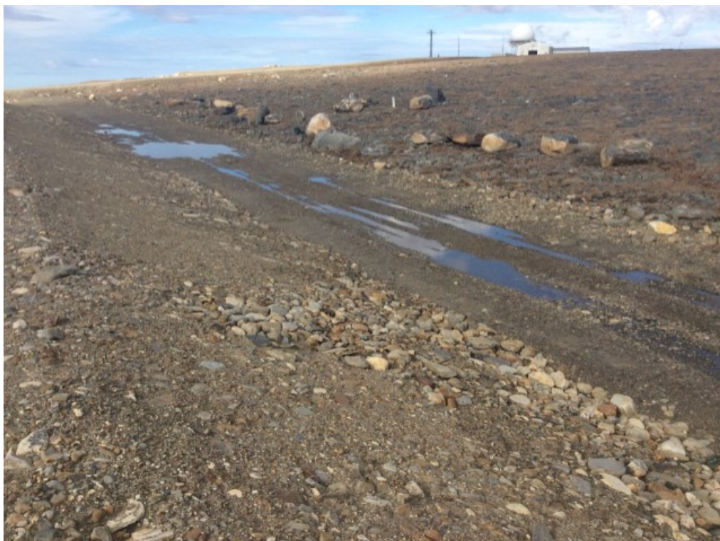
Photo 20: FOX-3 – Non Hazardous Waste Landfill – North toe – Feature F – Ponded water along toe [Acceptable], facing west (ATT34_Photo34.jpg)
