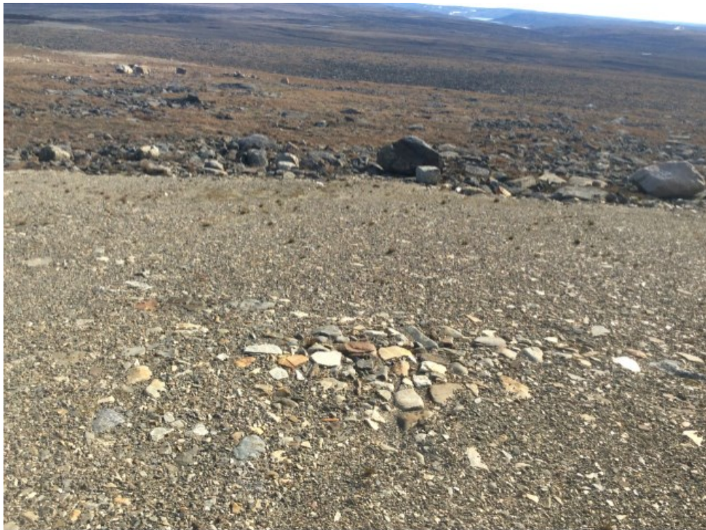
Photo 83: FOX-3 – Station West Landfill – Lobe F, southeast slope – Feature P – Minor self-armouring erosion [Acceptable], facing southeast (ATT26_Photo26.jpg)
