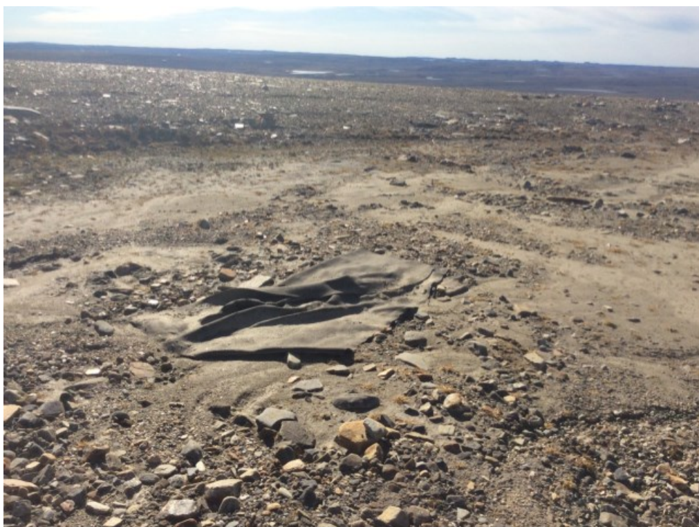
Photo 79: FOX-3 – Station West Landfill – Lobe E2, northeast toe – Feature I – Geotextile [Acceptable], facing west (ATT20_Photo20.jpg)
