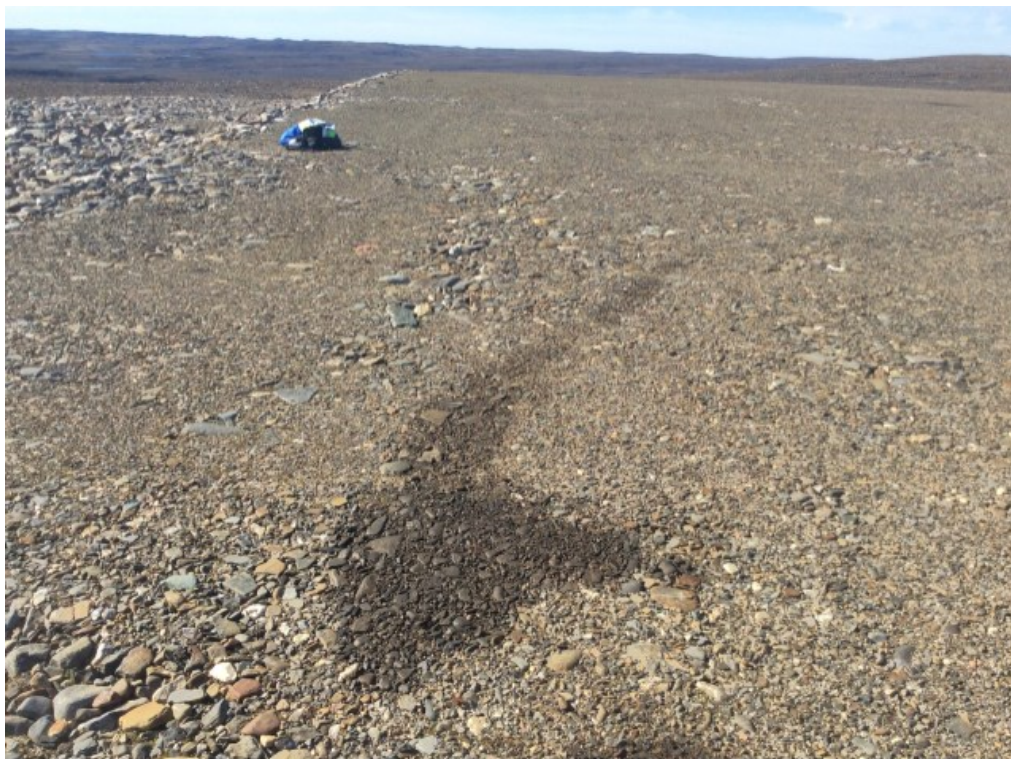
Photo 151: FOX-3 – Tier II Disposal Facility – Cover surface, Feature D – Staining, facing west (ATT6_Photo6.jpg)
