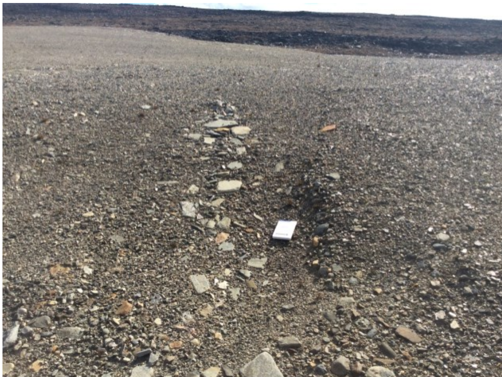
Photo 181: FOX-3 – West Landfill – West slope – Feature E – Minor settlement [Acceptable], facing northeast (ATT56_Photo56.jpg)
