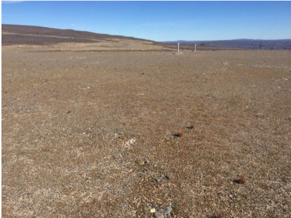
Photo 147: FOX-3 – Tier II Disposal Facility – Central cover surface – Feature L – Some very sparse vegetation [Acceptable], facing east (ATT8_Photo8.jpg)
