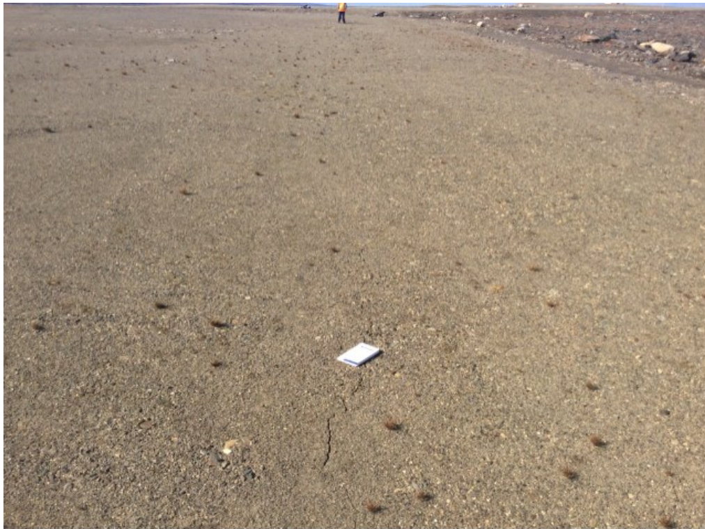
Photo 27: FOX-3 – Non Hazardous Waste Landfill – North crest – Feature O – Minor tension crack along the north crest, facing west (1 point) (ATT45_Photo45.jpg)
