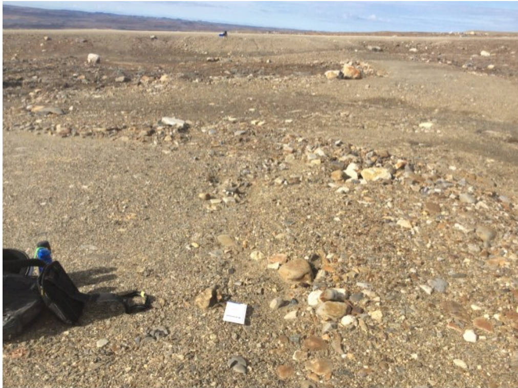
Photo 17: FOX-3 – Non Hazardous Waste Landfill – Northwest crest corner – Feature L – Small depressions [Acceptable], facing northwest (ATT33_Photo33.jpg)
