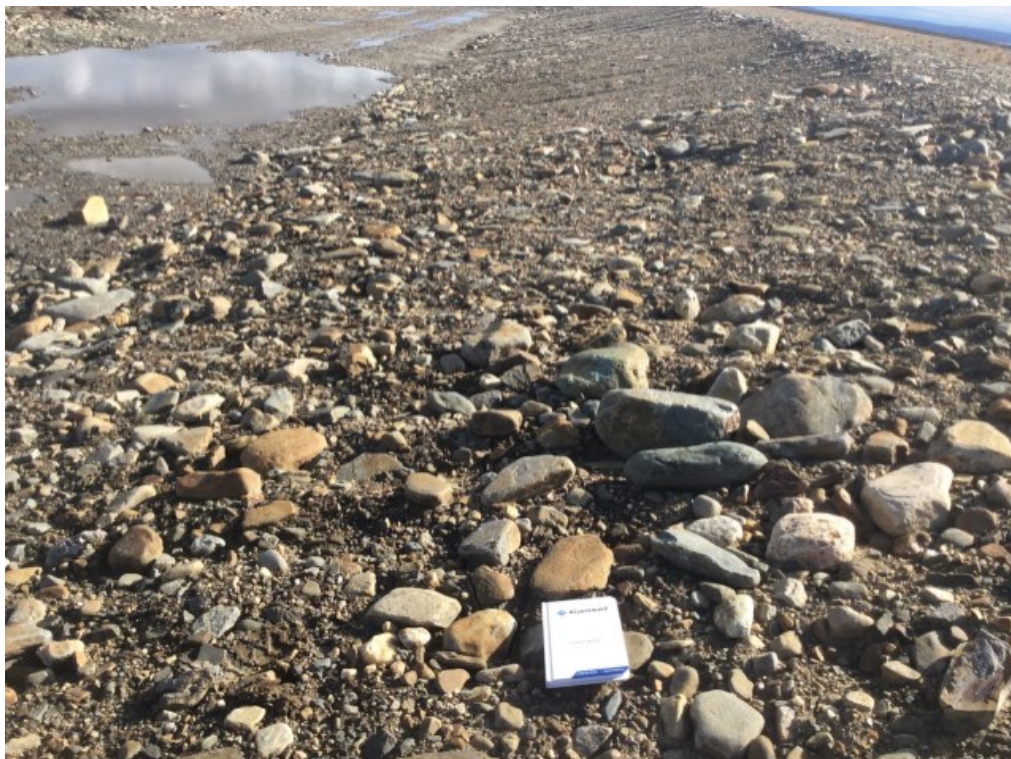
Photo 25: FOX-3 – Non Hazardous Waste Landfill – North slope – Feature N – Tension crack extended along the north slope below which the area is wet but no signs of seepage, facing east (ATT36_Photo36.jpg)
