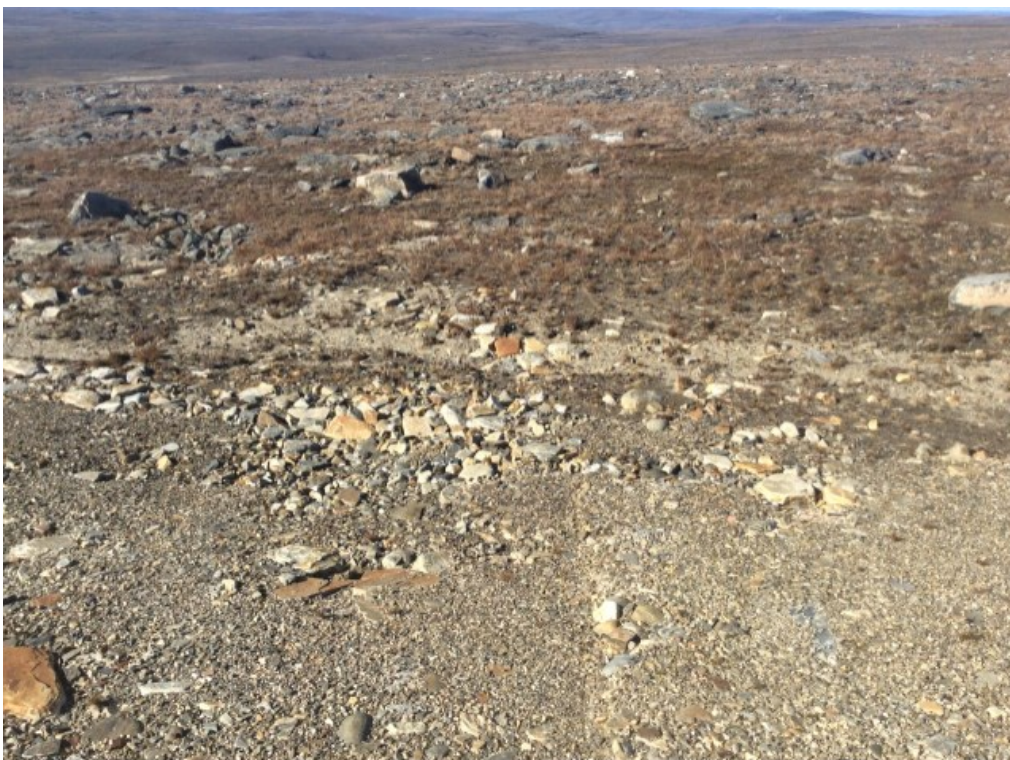
Photo 78: FOX-3 – Station West Landfill – Lobe E2, north toe – No ponded water along toe (previous Feature AA) [Acceptable], facing east (ATT21_Photo21.jpg)
