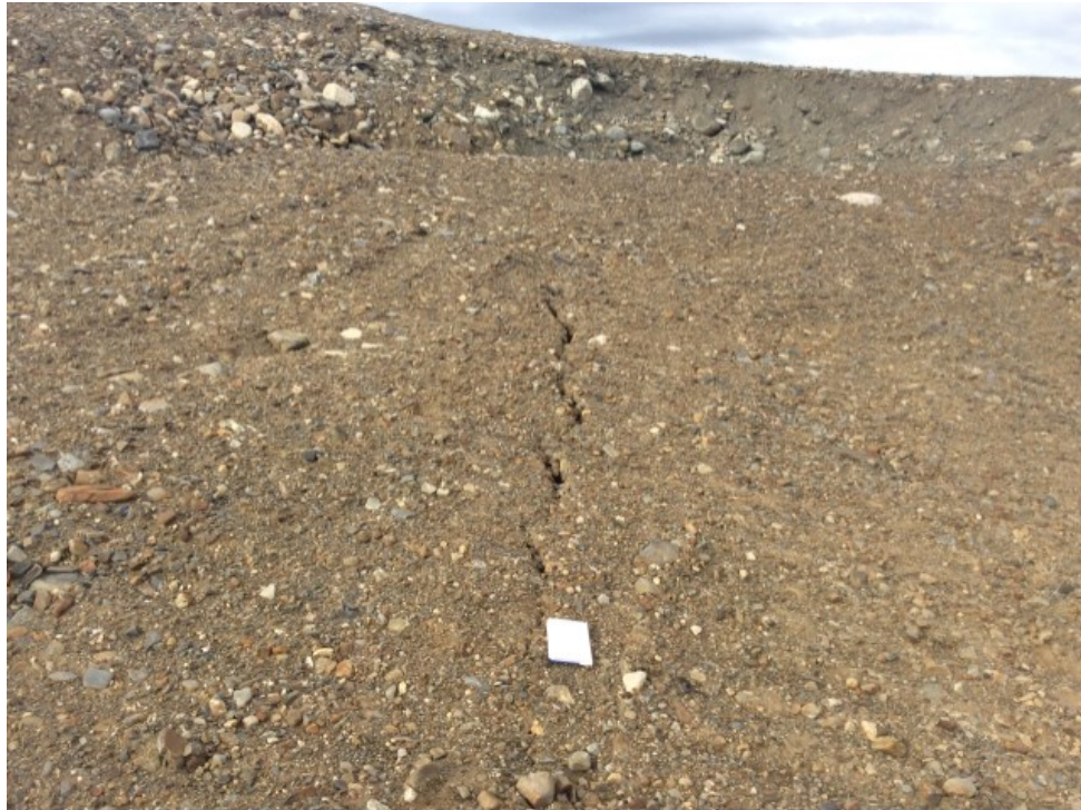
Photo E9: FOX-3 – Thermokarst Area – Feature E – Cracking extended along the edge of settlement, facing north (ATT67_Photo67.jpg)
