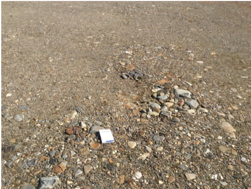
Photo 19: FOX-3 – Non Hazardous Waste Landfill – Central crest surface – Feature M – Small depression [Acceptable], facing south (ATT44_Photo44.jpg)
