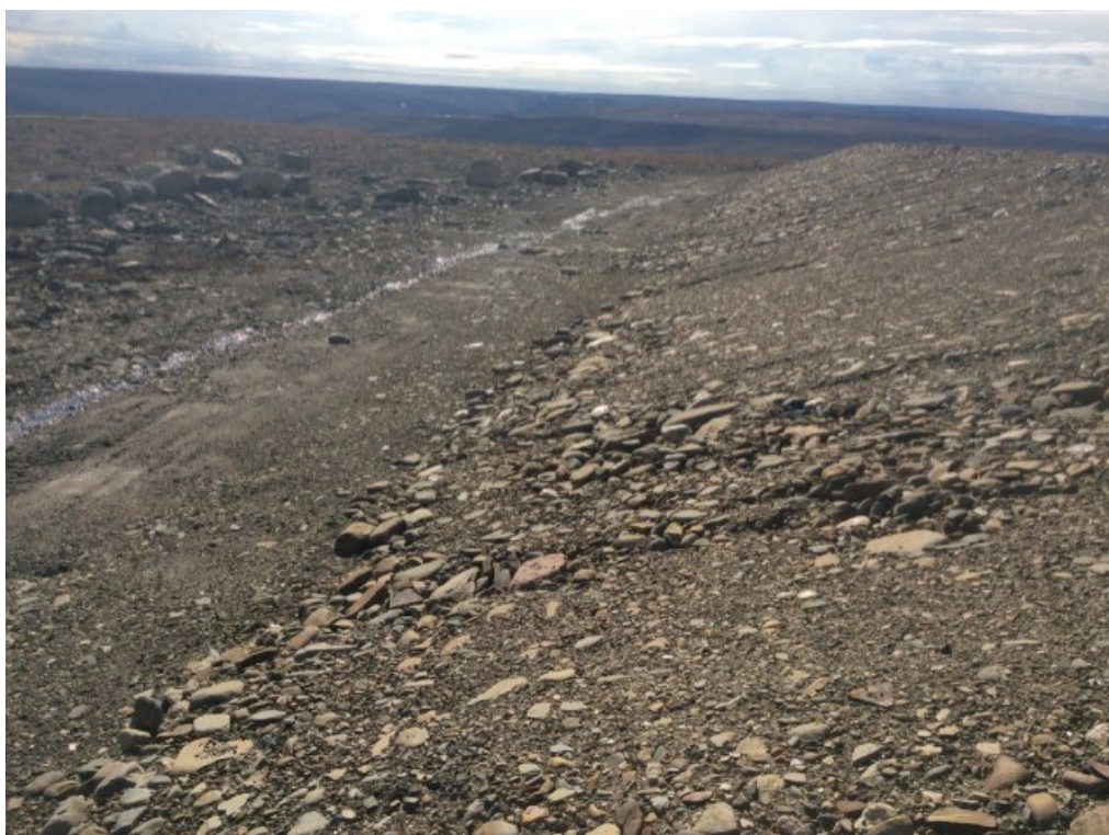
Photo 24: FOX-3 – Non Hazardous Waste Landfill – East toe – Feature K – Ponded water running along toe [Acceptable], facing south (ATT38_Photo38.jpg)
