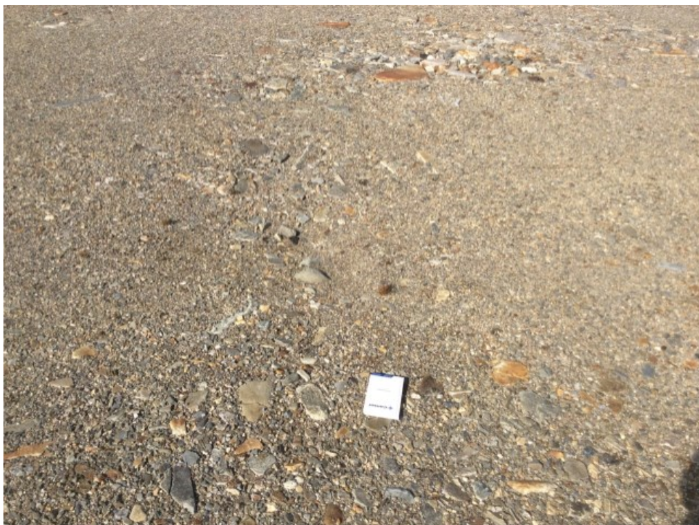
Photo 190: FOX-3 – West Landfill – Cover surface – Feature B – Minor settlement with no ponded water. [Acceptable], facing northeast (ATT53_Photo53.jpg)
