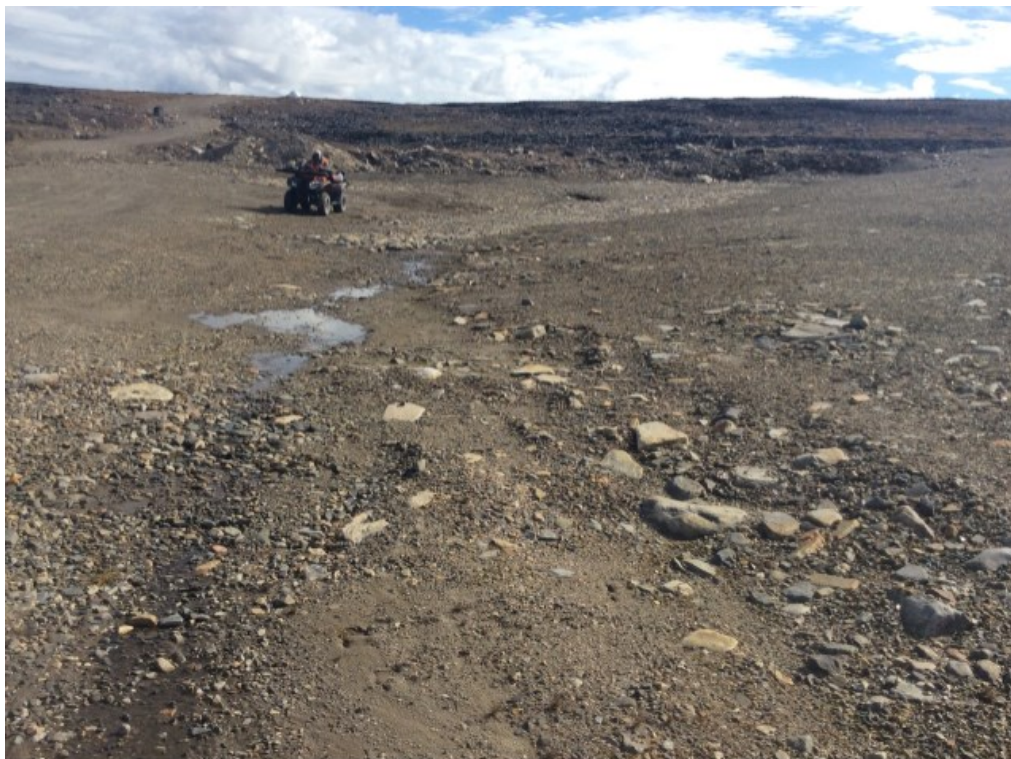
Photo 169: FOX-3 – West Landfill – Feature D – ponded water at the north toe, facing east (ATT86_Photo86.jpg)
