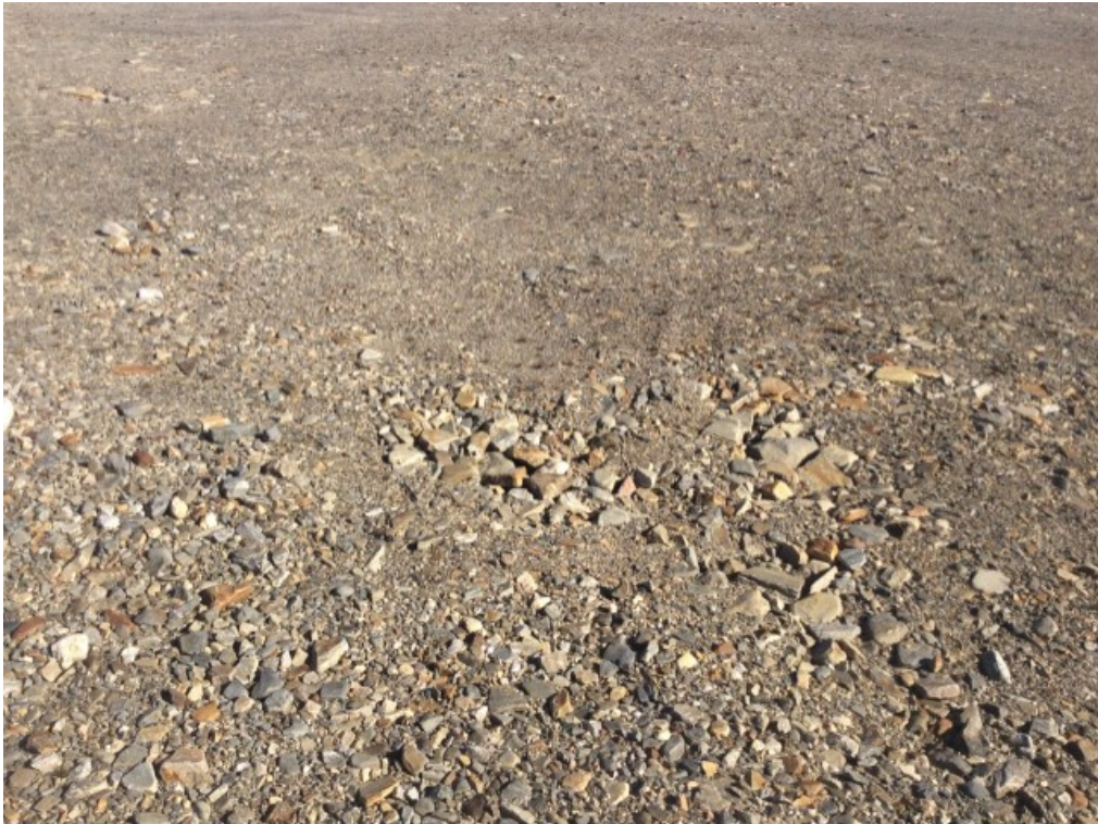
Photo 89: FOX-3 – Station West Landfill – Lobe A, central crest surface – Feature W – Shallow depressions [Acceptable], facing southeast (ATT11_Photo11.jpg)
