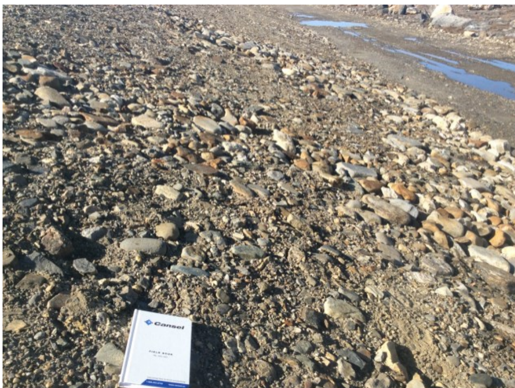
Photo 26: FOX-3 – Non Hazardous Waste Landfill – North slope – Feature N – Tension crack extended along the north slope below which the area is wet but no signs of seepage, facing west (ATT37_Photo37.jpg)
