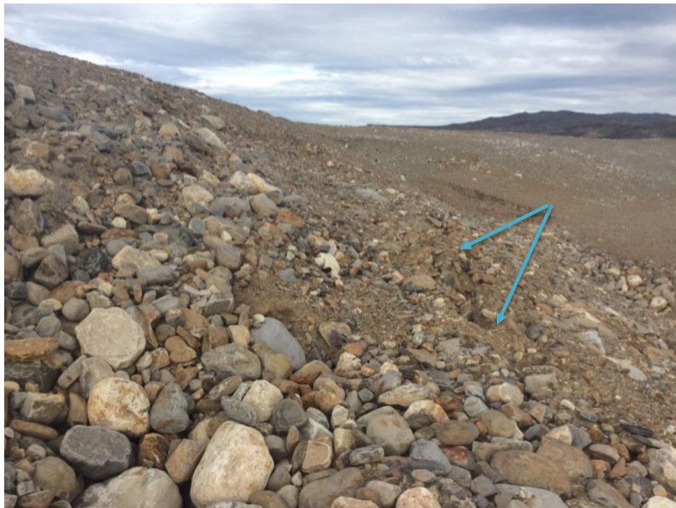
Photo E23: FOX-3 – Thermokarst Area – Extended tension crack (Feature B), facing northeast (ATT111_Photo111.jpg)
