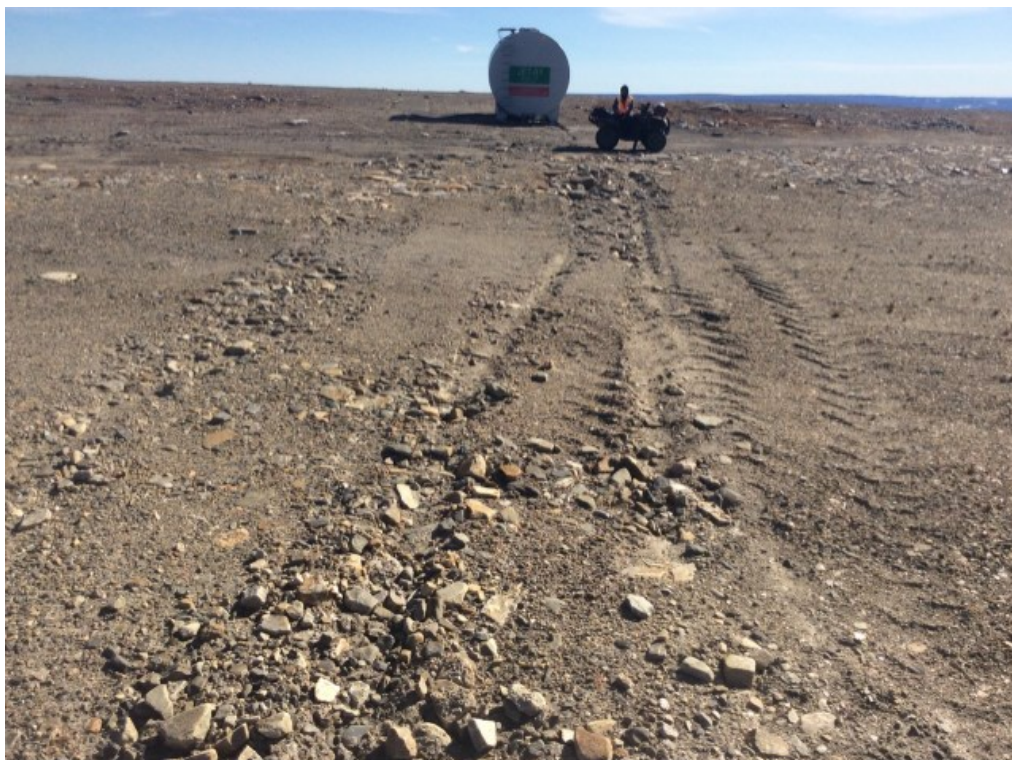
Photo 98: FOX-3 – Station West Landfill – Lobe A, cover surface – Feature AD – Tire track on the cover surface and east slope – Feature Y is also shown, facing southeast (ATT17_Photo17.jpg)
