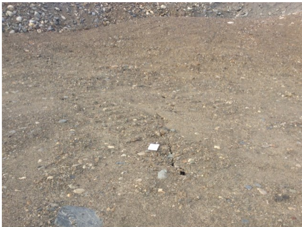
Photo E6: FOX-3 – Thermokarst Area – Feature E – Cracking extended towards the settlement area, facing northwest (ATT64_Photo64.jpg)
