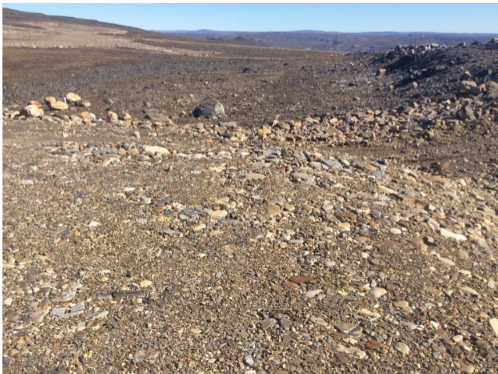
Photo 149: FOX-3 – Tier II Disposal Facility – Crest surface in southeast corner – (Previous Feature I- no ponded water-minor Depression), facing southeast (ATT4_Photo4.jpg)
