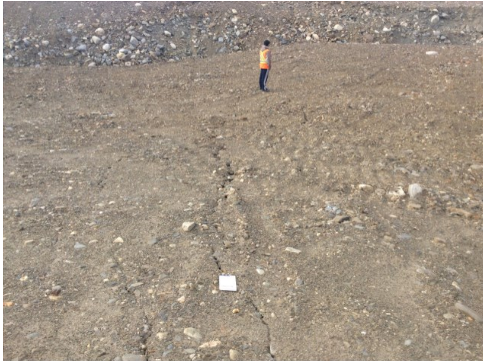
Photo E7: FOX-3 – Thermokarst Area – Feature E – Cracking extended towards the settlement area, facing northwest (ATT65_Photo65.jpg)
