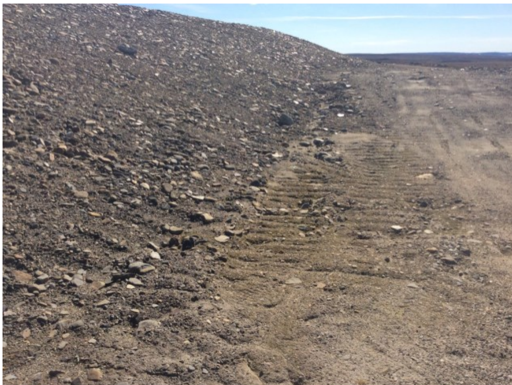
Photo 146: FOX-3 – Tier II Disposal Facility – west toe – No ponded water along toe (previous Feature K), facing south (ATT2_Photo2.jpg)
