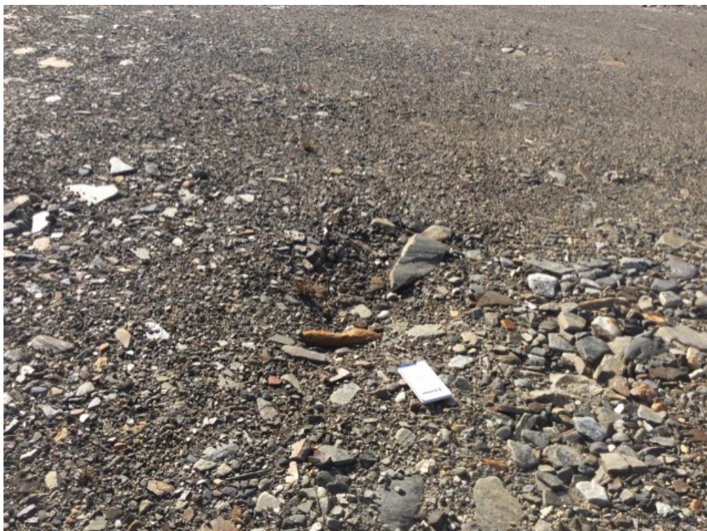
Photo 188: FOX-3 – West Landfill – Cover surface – Feature A – Minor settlement and rough area [Acceptable], facing northeast (ATT52_Photo52.jpg)
