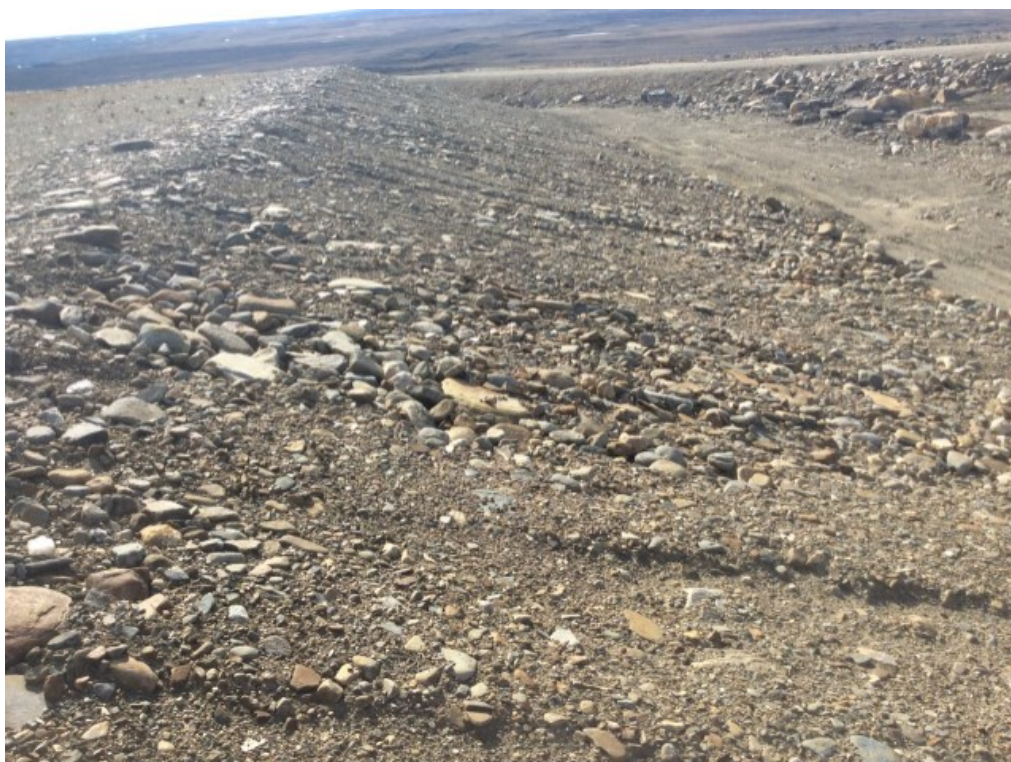
Photo 16: FOX-3 – Non Hazardous Waste Landfill – West slope – Feature I – Self-armoured erosion [Acceptable], facing south (ATT42_Photo42.jpg)
