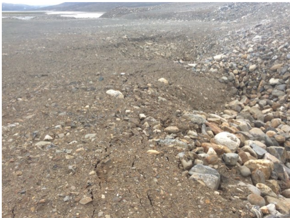
Photo E4: FOX-3 – Thermokarst Area – Feature D – Cracking, facing southwest (ATT62_Photo62.jpg)
