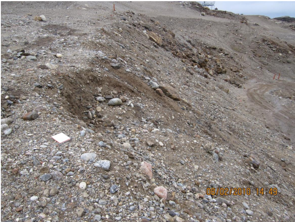
Photograph 16. Slump Block in Barrell Dump Landfill
