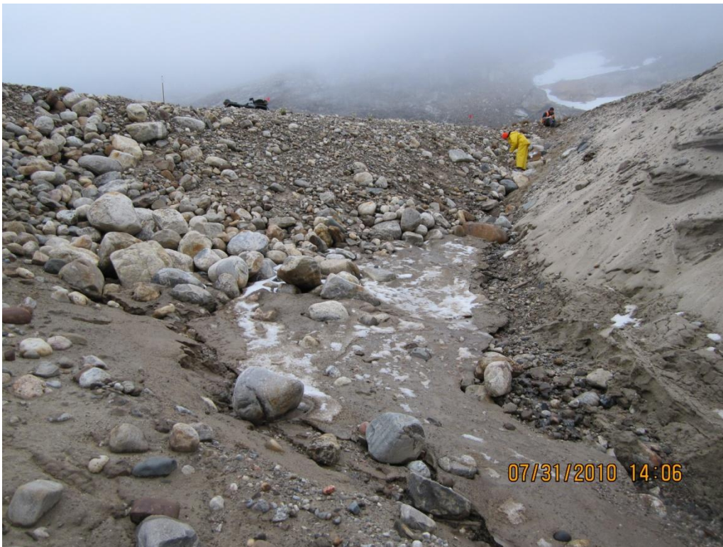
Photograph 12. Erosion Channel and Debris in Airstrip Landfill
