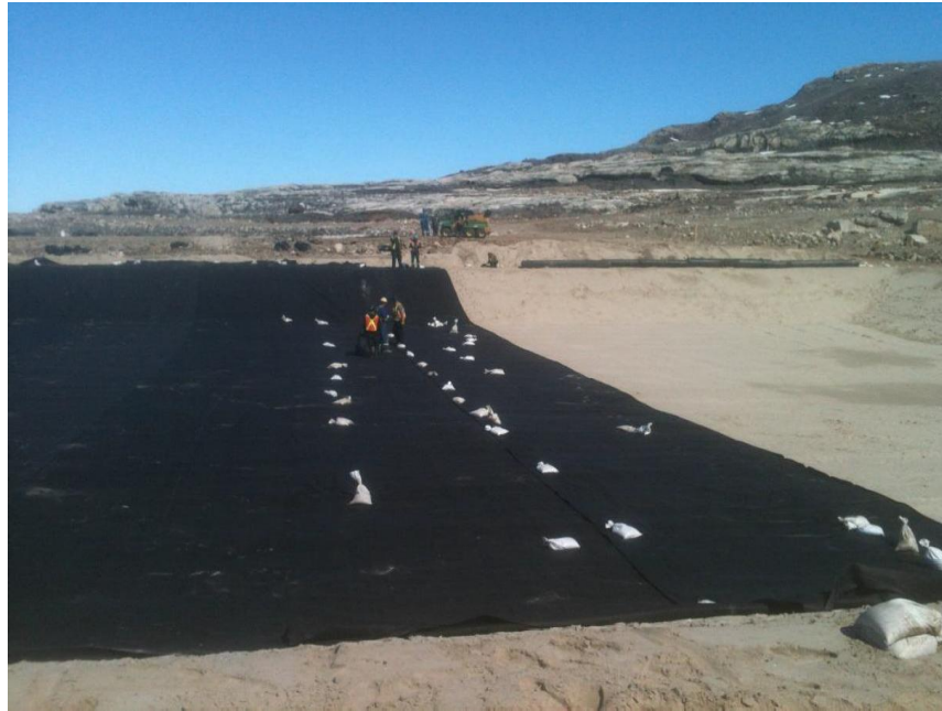
Photograph 1. First Layer of Geotextile at the Tier II Facility
