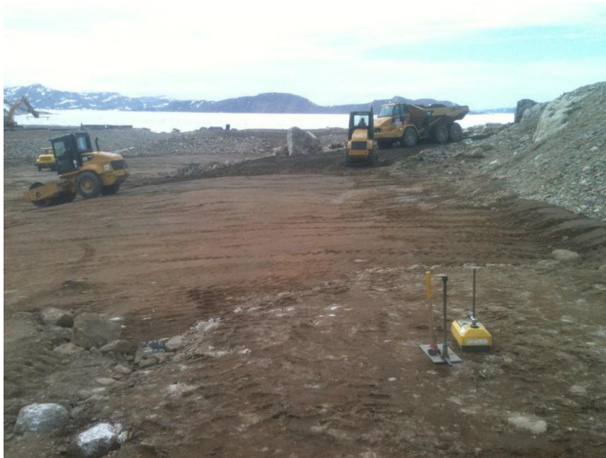
Photograph 8. Type 2 Granular Fill Compaction at Pallet Line Landfill Regrade
