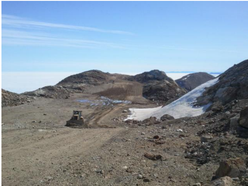
Photograph 15. Station Area Ridge Regrade - Completed
