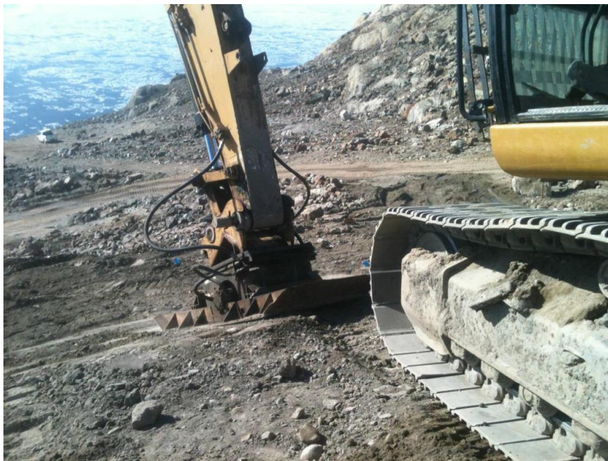
Photograph 25. Compaction Attachment for Excavator at Helipad-West Regrade
