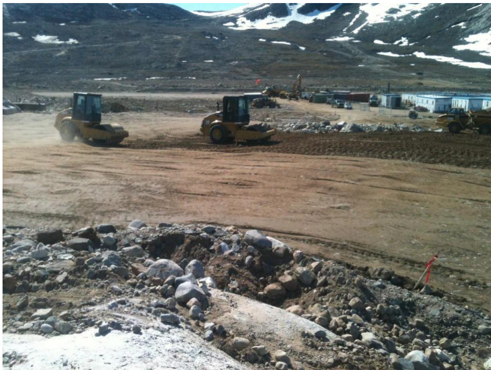
Photograph 6. HVS Buried Debris Area Regrade Type 2 Granular Fill Compaction
