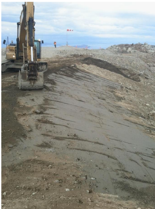
Photograph 38. Helipad East – East Lobe – Backfilling Complete
