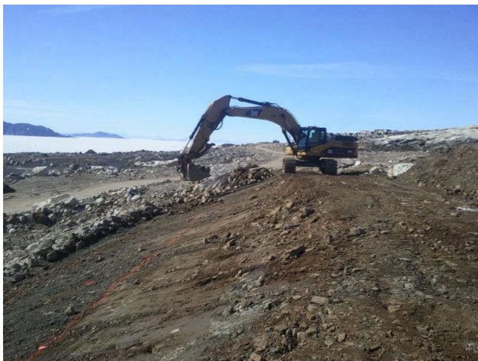
Photograph 13. Pallet Line Landfill Regrade – Placing Type 1 Fill material
