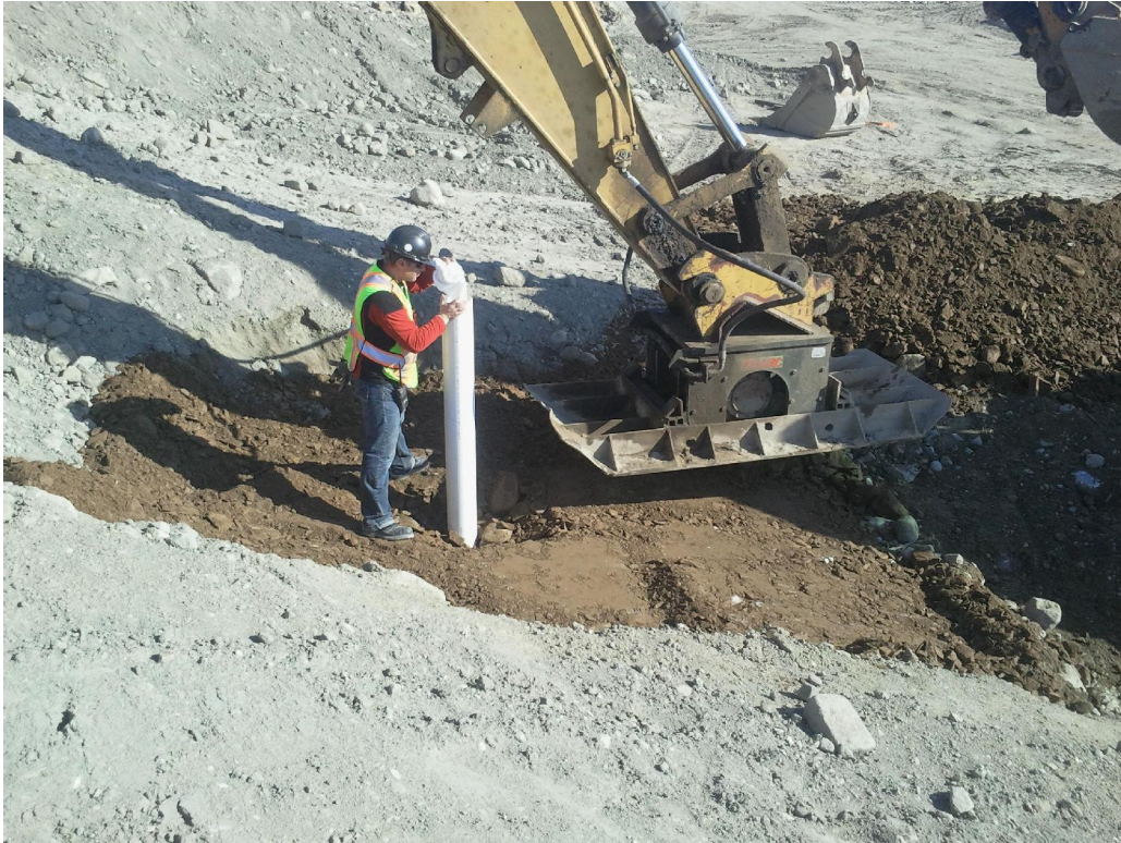
Photograph 30. Helipad West Regrade – Compacting Type 2 Granular Fill around MW-01
