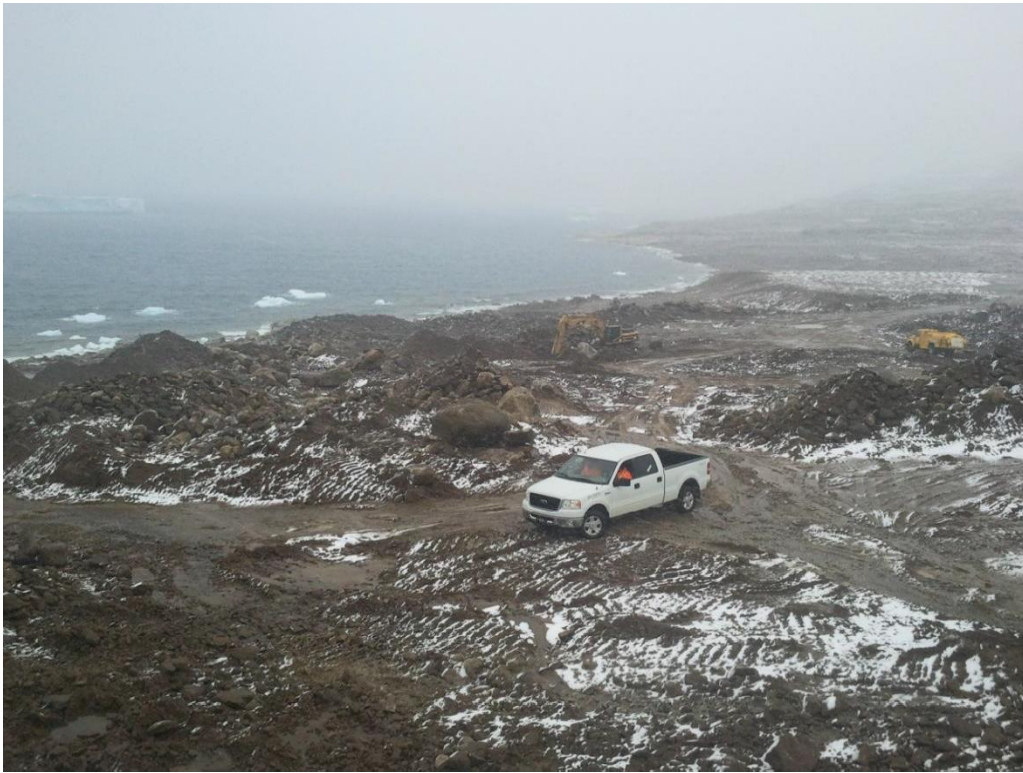
Photograph 52. Borrow Area 3 – Type 2 Granular Fill Mining Activities
