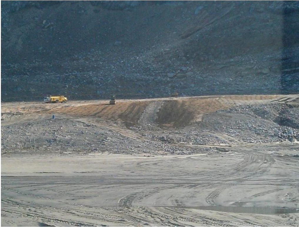
Photograph 45. Airstrip Landfill – Completed Swale and Type 2 Granular Fill Cap
