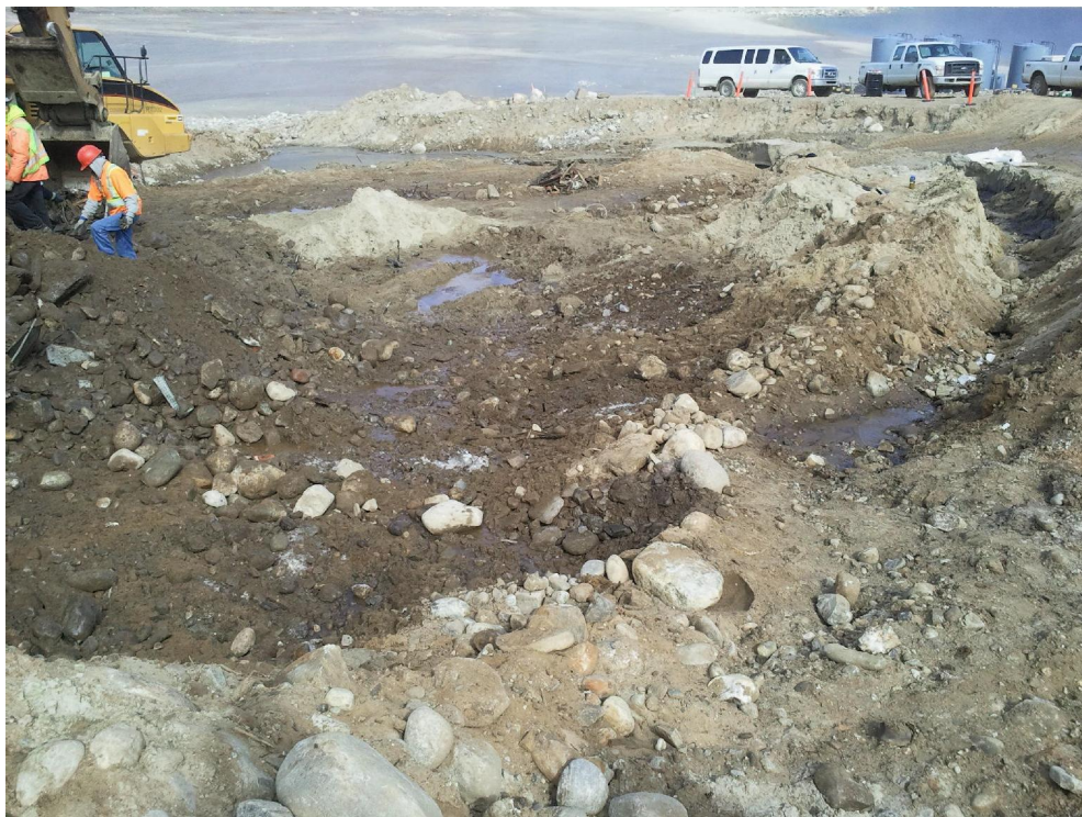
Photograph 28. Airstrip Landfill West – Groundwater Seepage
