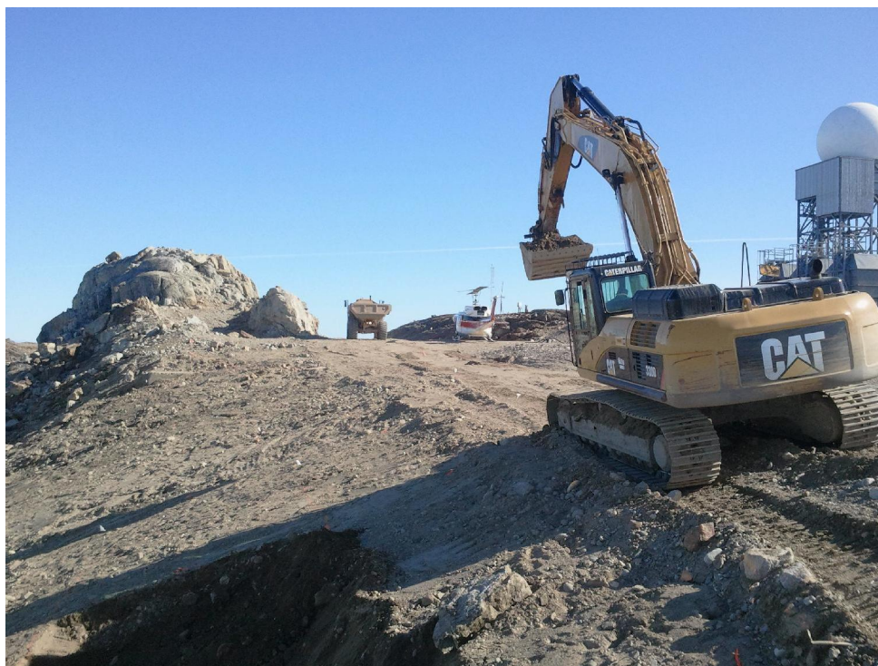
Photograph 29. Helipad Landfill East - Excavation
