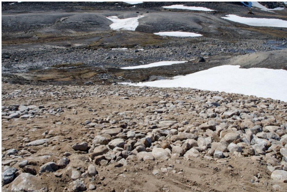
Photograph 4. Type1 Granular Fill at on Tanner Bay Regrade Slopes
