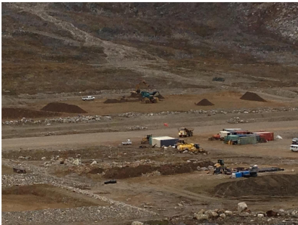
Photograph 32. Landfarm – Before spreading the three separate areas of material: 2,500 – 5,000 ppm (not screened), +10,000 ppm (screened), and 5,000 – 7,500 ppm (screened) from right to left.
