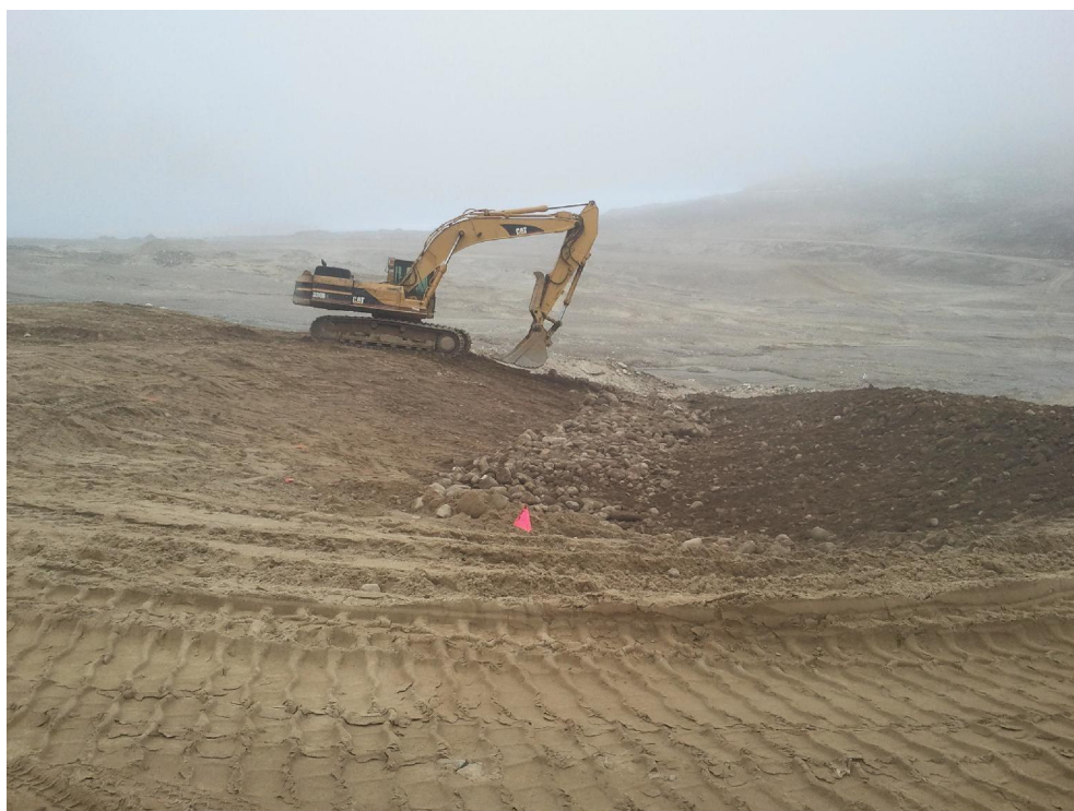
Photograph 34. Airstrip Landfill East – Drainage Swale
