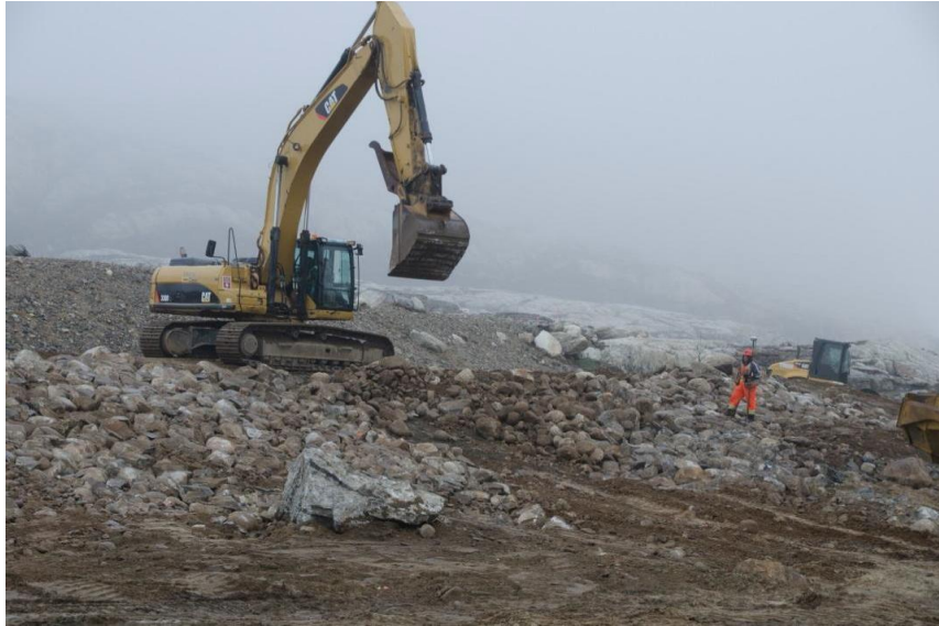
Photograph 7. Type 1 Granular Fill Placement at Pallet Line Landfill Regrade
