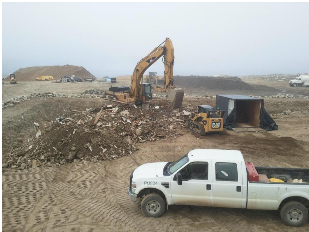
Photograph 37. Non-Hazardous Waste Facility – Using a Modified Barge Container QM is Preparing Wood PCB Paint for Transport Off Site
