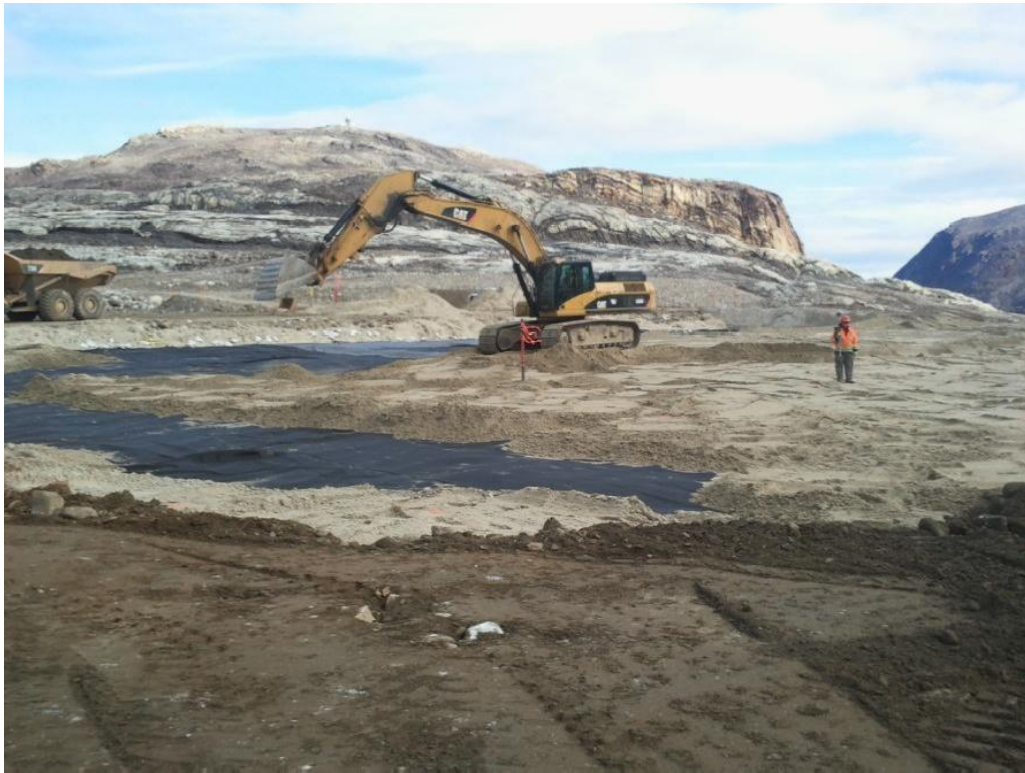
Photograph 47. Tier II Facility – Placing Type 5 Granular Fill over Synthetic Liner
