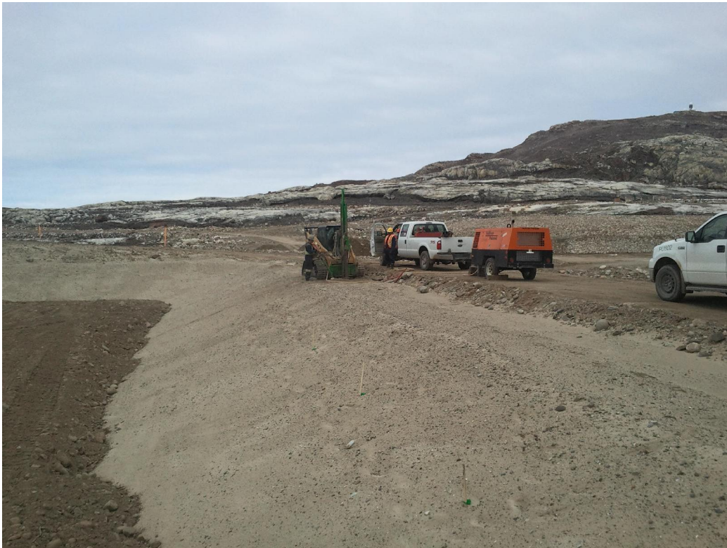
Photograph 27. Tier II Facility – Drilling VT-10 on Western Berm
