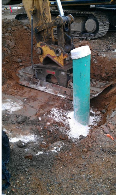
Photograph 40. Existing Tier II Facility - Backfilling Ground Temperature Monitoring Excavation
