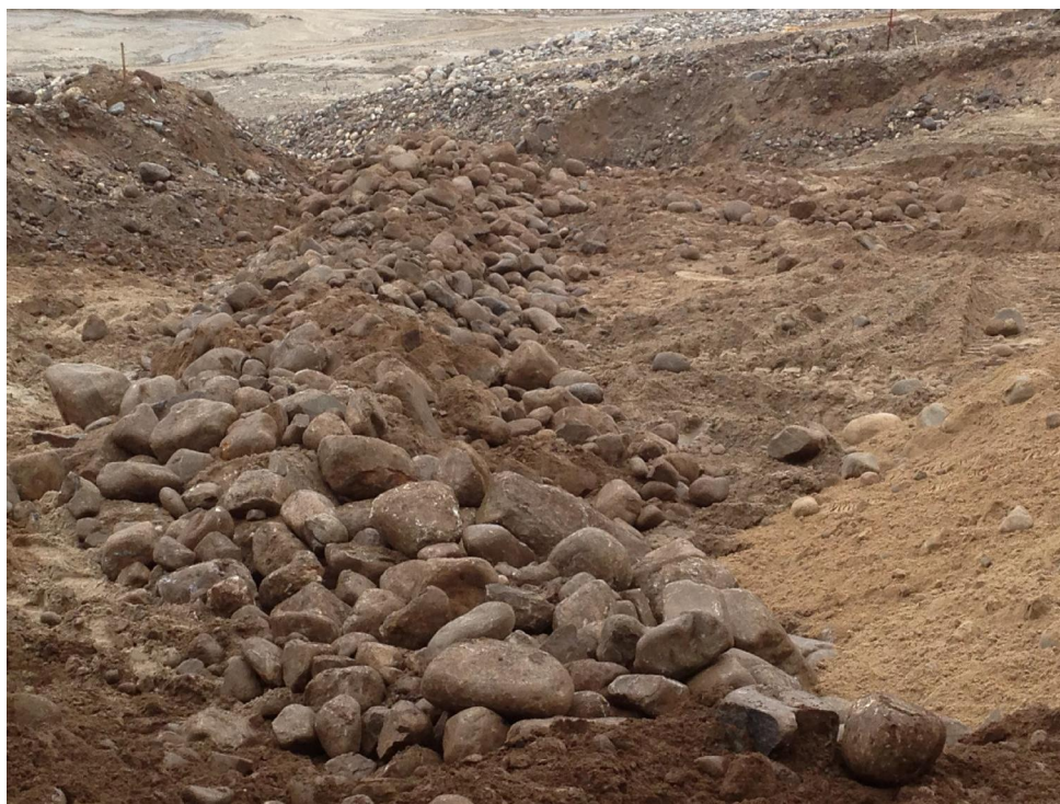
Photograph 33. Airstrip Landfill East – French Drain System
