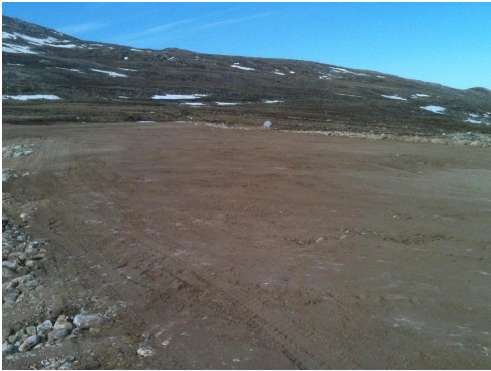
Photograph 5. Final Type 2 Granular Fill Surface at Tanner Bay Regrade
