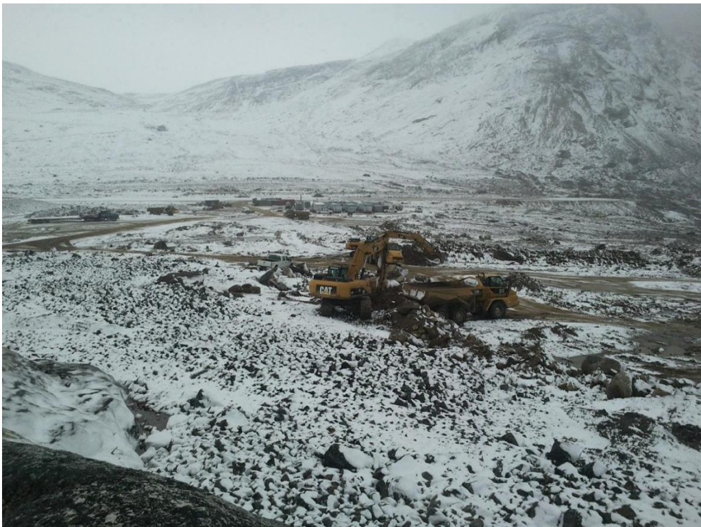
Photograph 55. Borrow Area 6 – Mining Material to be Screened for Airstrip Improvement Project
