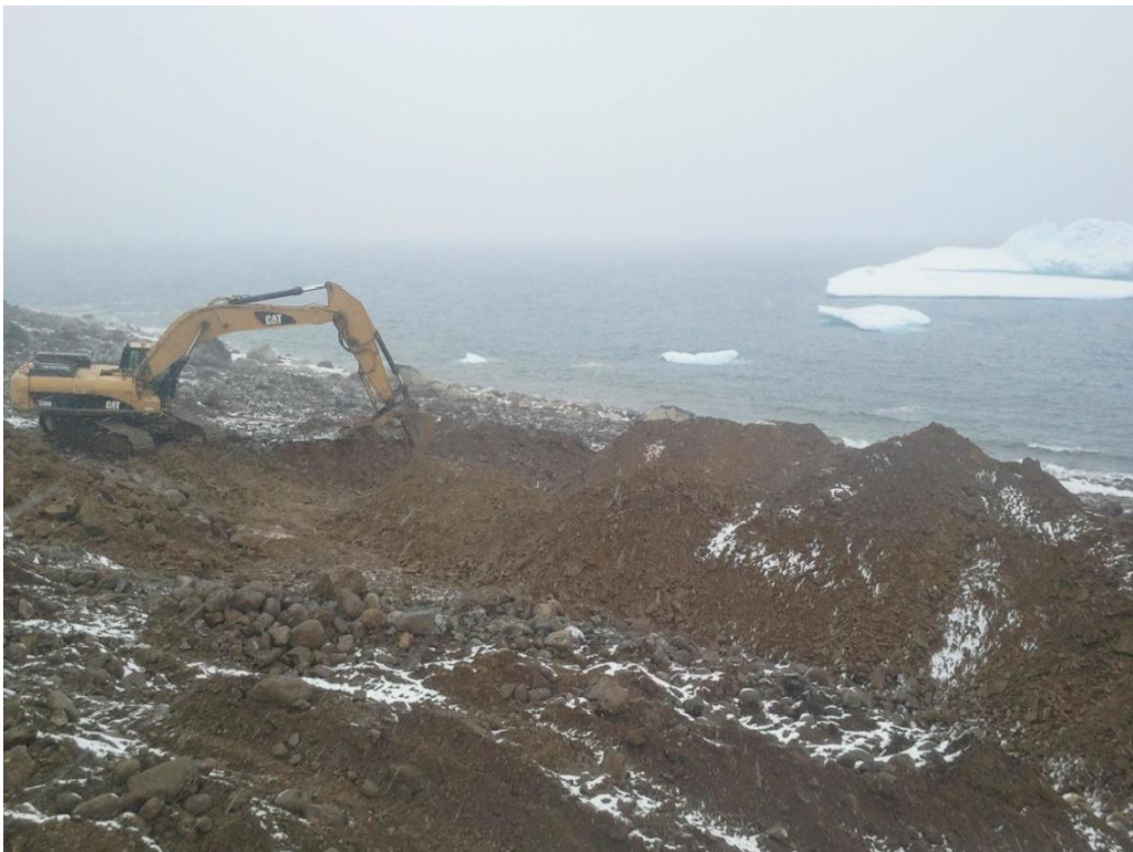
Photograph 53. Borrow Area 3 – Type 2 Granular Fill Mining Activities
