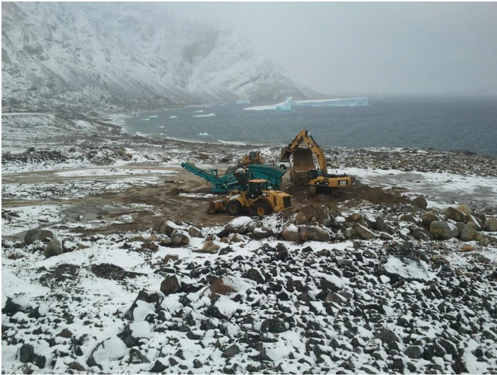
Photograph 54. Borrow Area 6 – Screening Material for Airstrip Improvement Project
