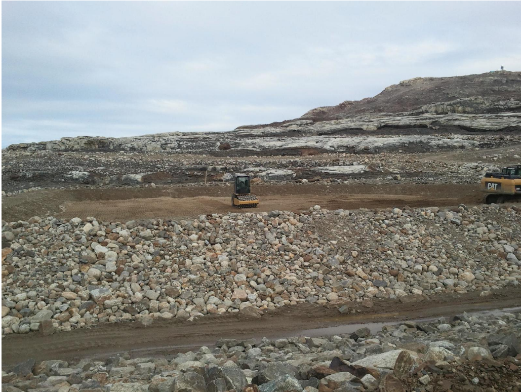
Photograph 26. Non-Hazardous Waste Landfill – Compacting Type 6 Granular Fill over Debris
