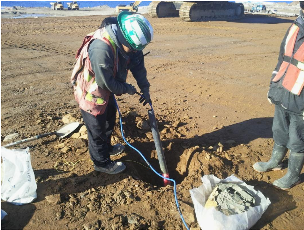
Photograph 60. Tier II Facility – Installing Thermistors
