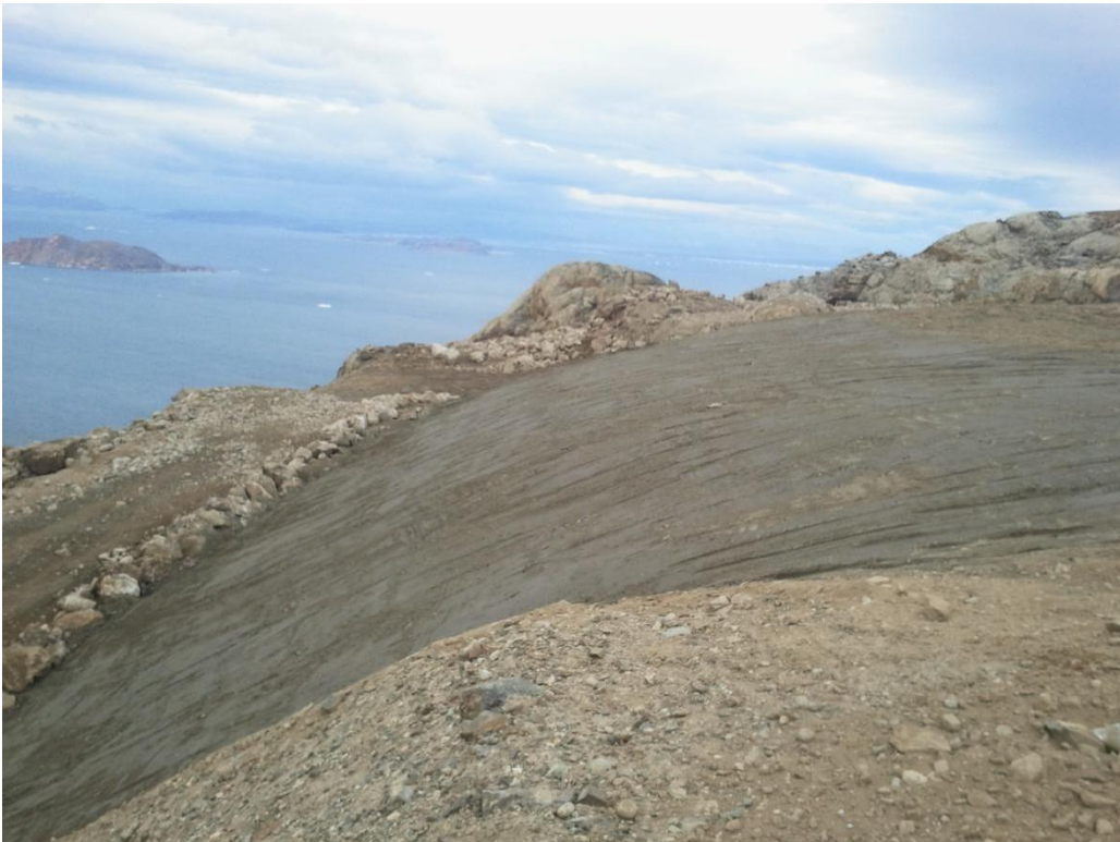
Photograph 36. Barrel Dump Landfill – Type 2 Granular Fill Material Cap Complete
