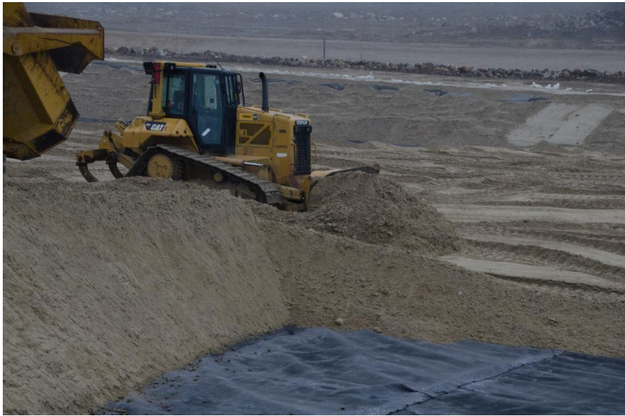
Photograph 3. Placement of Type 5 Granular Fill Above Liner
