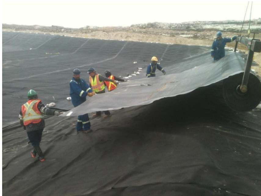
Photograph 2. Placement of HDPE Liner (Geomembrane) at the Tier II Facility
