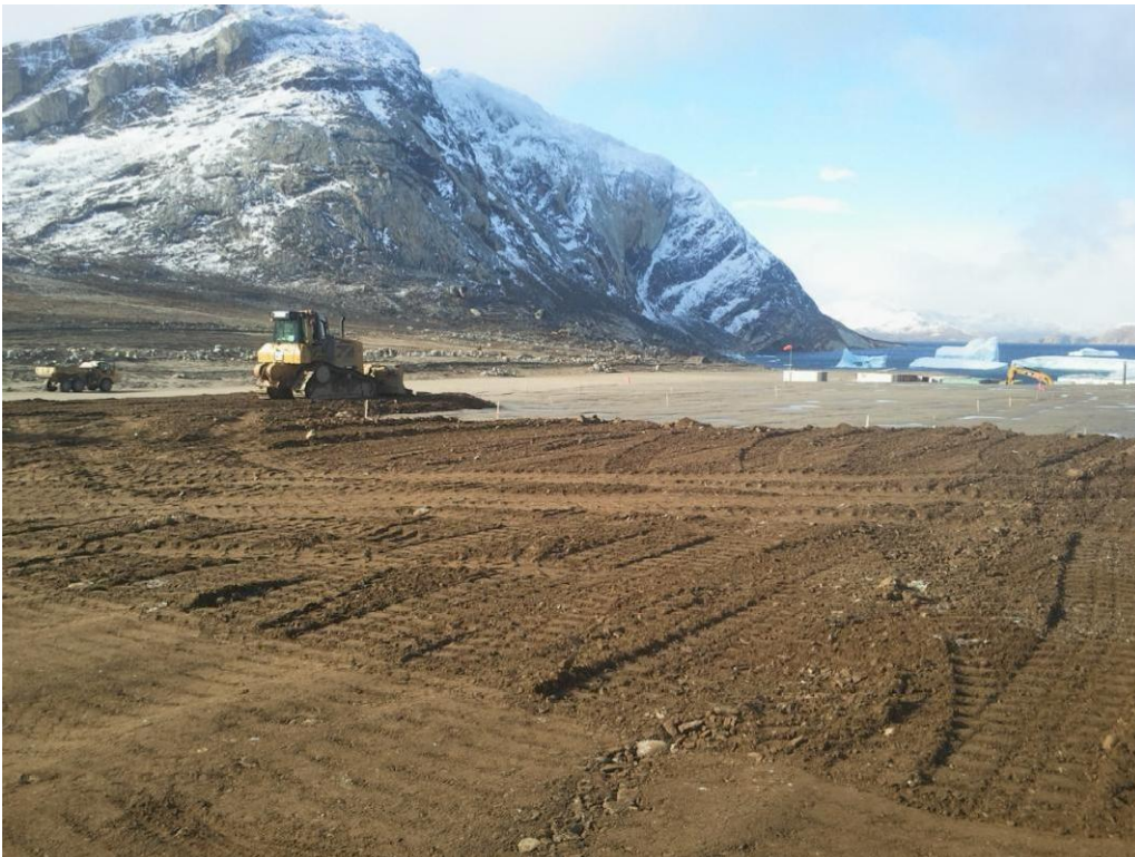
Photograph 57. Tier II Facility – Spreading Final Lift
