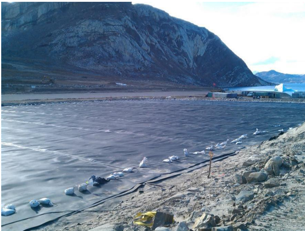
Photograph 46. Tier II Facility – Geomembrane Laid Out
