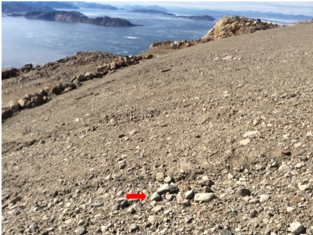
Photo 103: FOX-4 – Helipad West Landfill – Slope northwest of landfill facing northwest – Feature M – Self-armouring erosion (Acceptable) (ATT140_Photo140.jpg)
