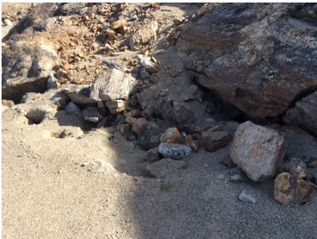
Photo 132: FOX-4 – Station Area Landfill – Feature E – Sink holes along south edge of landfill, facing southeast (Acceptable) (ATT132_Photo132.jpg)
