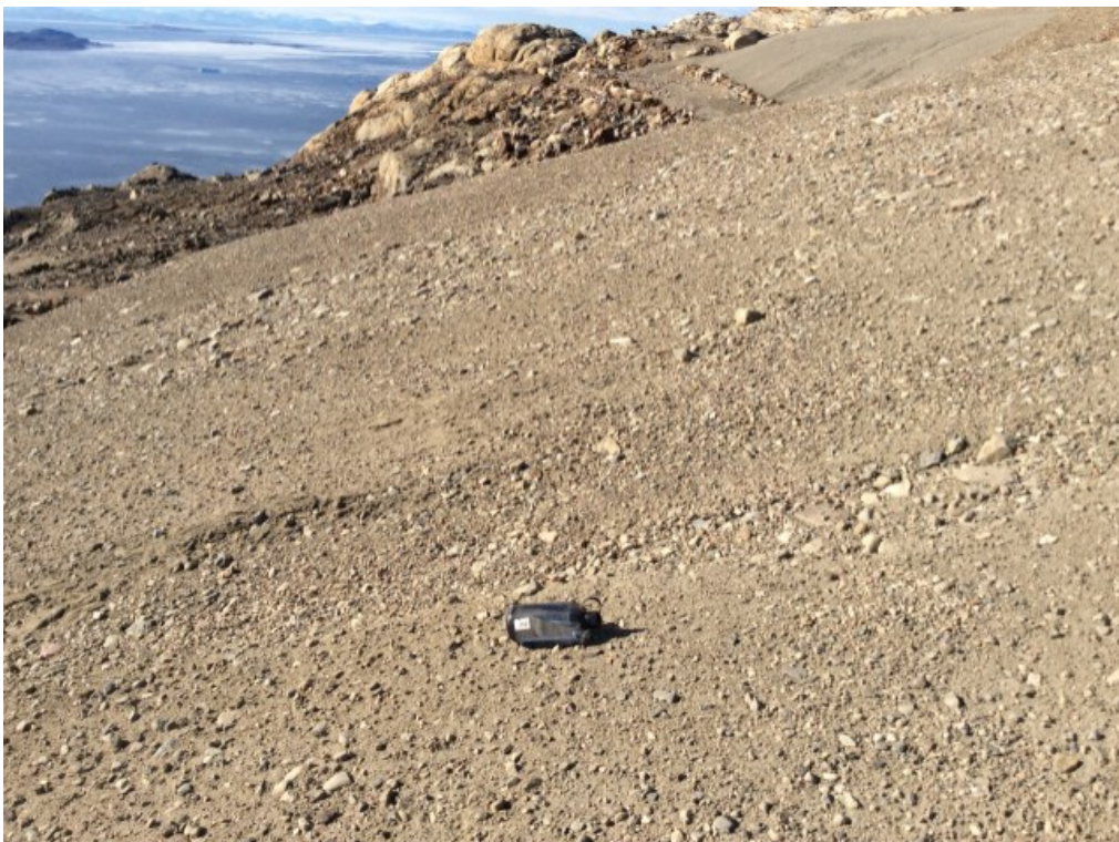
Photo 106: FOX-4 – Helipad West Landfill – West slope west – Feature C – Self-armouring erosion (Acceptable) (ATT152_Photo152.jpg)
