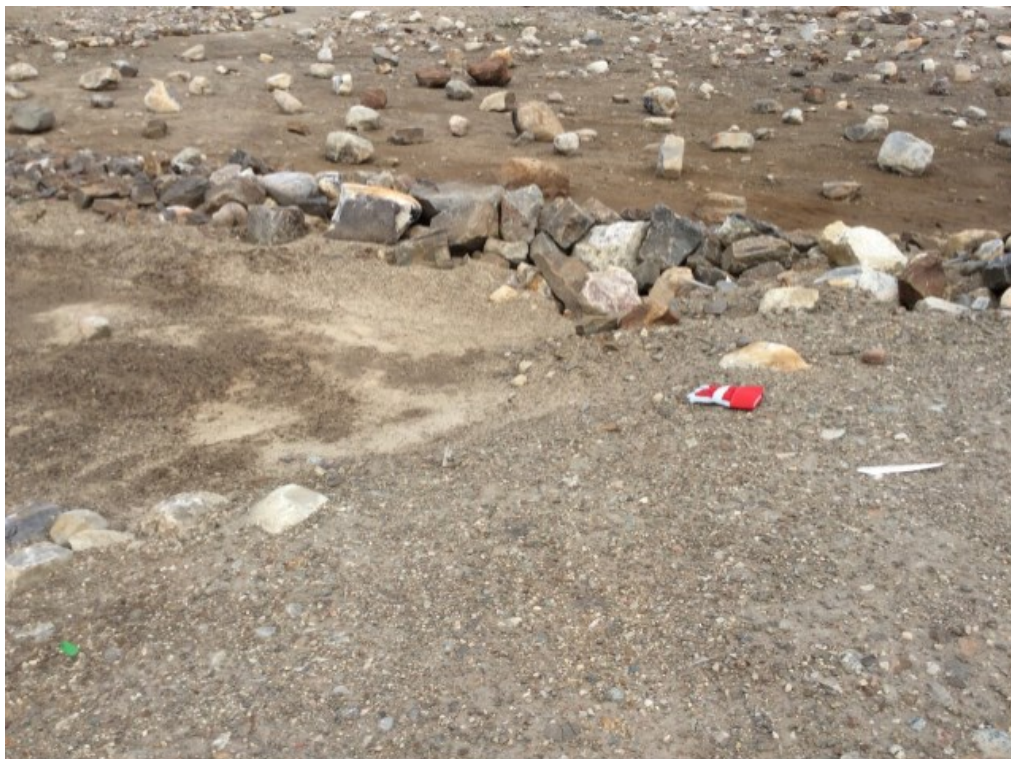
Photo 19: FOX-4 – NHWL/Tier II DF – Feature C – Minor erosion of internal sloped crest at edge (Acceptable), facing south (ATT116_Photo116.jpg)
