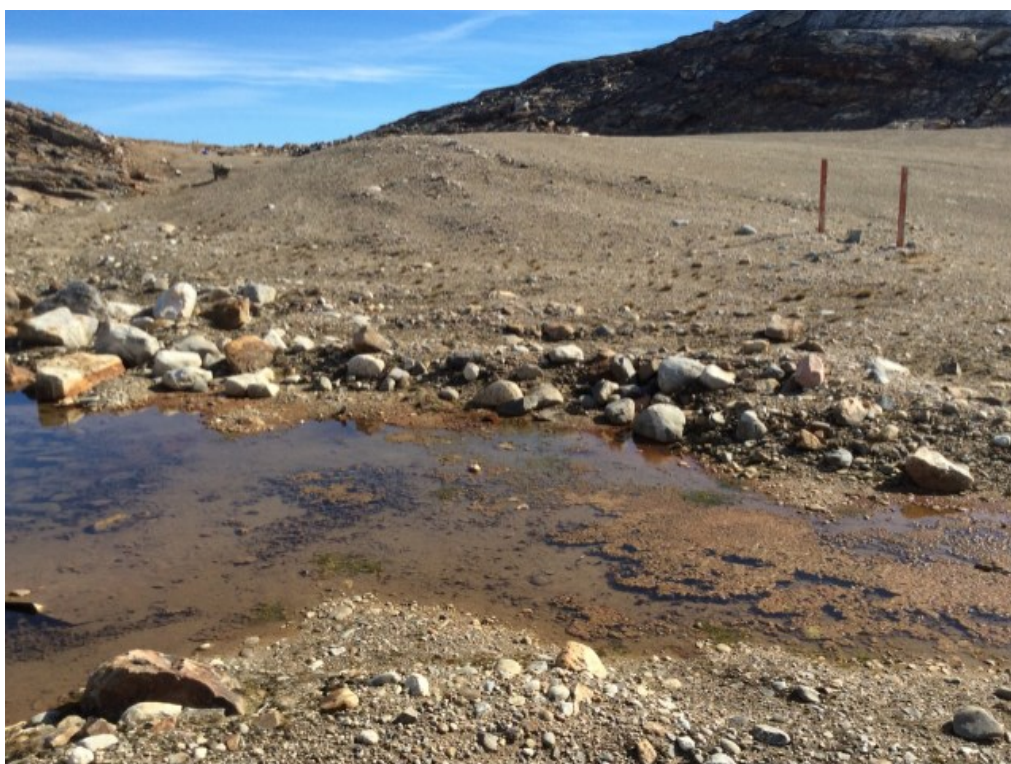
Photo 136: FOX-4 – Station Area Landfill – Northwest toe facing southeast towards landfill – Feature B – Ponded water with orange staining (Acceptable) (ATT135_Photo135.jpg)
