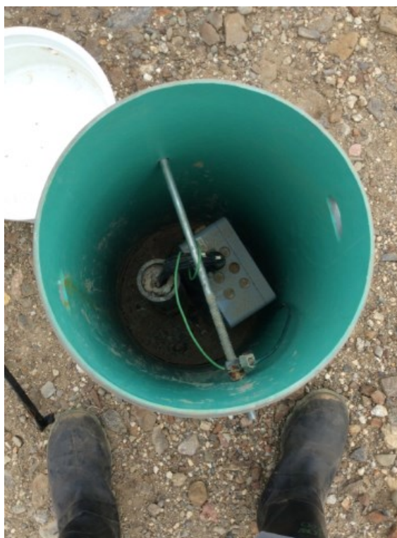
Photo 47: FOX-4 – NHWL/Tier II DF – Thermistor VT-2 (short datalogger cable) (ATT125_Photo125.jpg)
