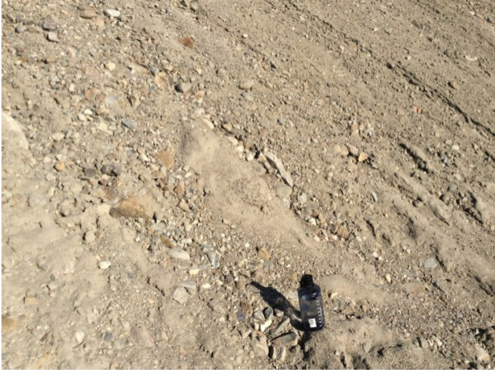
Photo 91: FOX-4 – Helipad West Landfill – Toe of slope facing east – Feature C – Minor self armouring erosion channels (Acceptable) (ATT153_Photo153.jpg)
