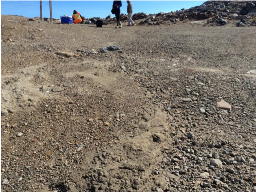
Photo 129: FOX-4 – Station Area Landfill – East end facing east – Feature C – Minor self-armouring erosion with fines washed down slope, soft ground at bottom of slope (Acceptable) (ATT130_Photo130.jpg)
