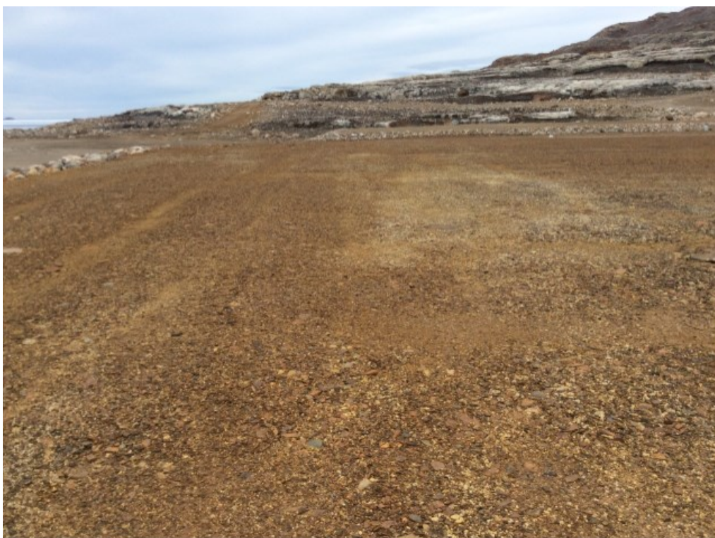
Photo 15: FOX-4 – NHWL/Tier II DF – Crest surface facing west – Feature A – Tire tracks (Acceptable) (ATT98_Photo98.jpg)
