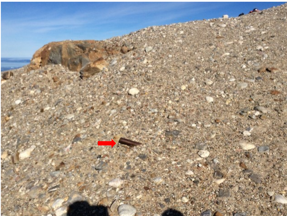
Photo 102: FOX-4 – Helipad West Landfill – Slope east of MW98-06 facing south – Feature L – Exposed steel pipe (Acceptable) (ATT142_Photo142.jpg)
