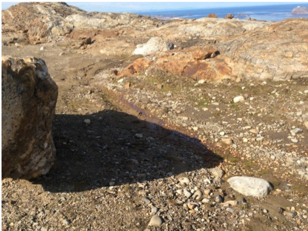
Photo 127: FOX-4 – Station Area Landfill – East end toe facing northwest – Previously observed Feature A - Seepage with orange staining (Acceptable) (ATT134_Photo134.jpg)
