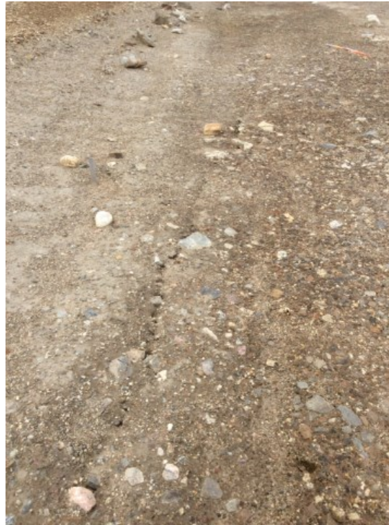
Photo 33: FOX-4 – NHWL/Tier II DF – Feature O – East end of cracking at toe of crest surface grade change (Acceptable), facing south (ATT129_Photo129.jpg)
