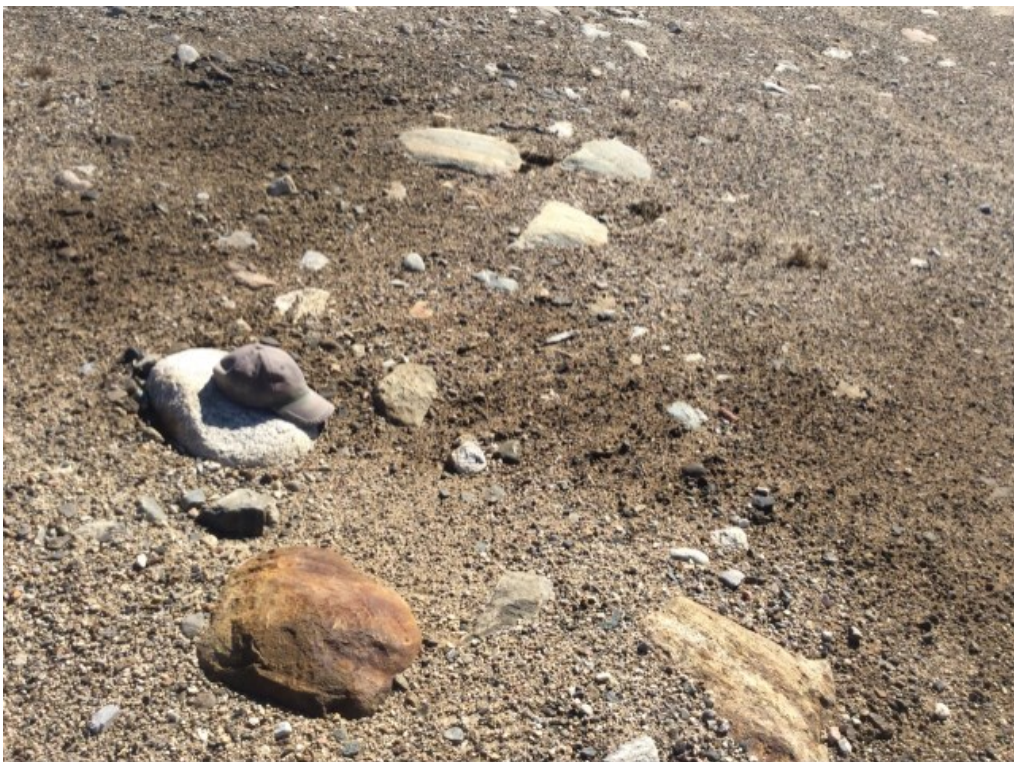
Photo 162: FOX-4 – Pallet Line Landfill – Crest surface of landfill facing north – Feature B – Minor dark (potential hydrocarbon) staining not related to landfill performance (Acceptable) (ATT94_Photo94.jpg)
