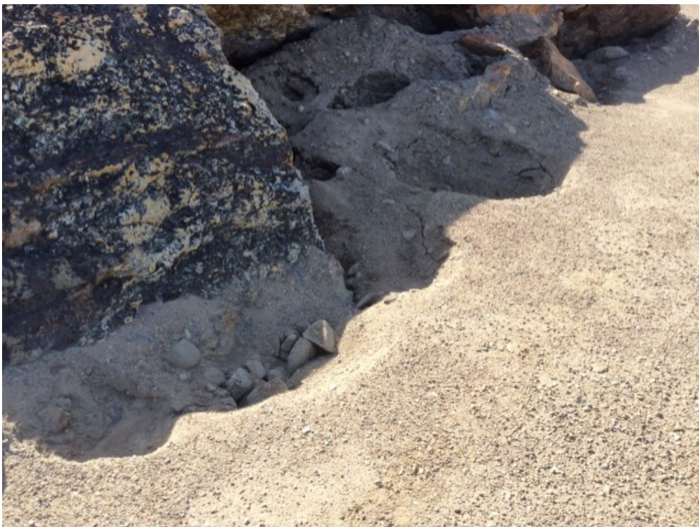
Photo 130: FOX-4 – Station Area Landfill – Feature D – Sink holes along south edge of landfill facing southwest (Acceptable) (ATT131_Photo131.jpg)
