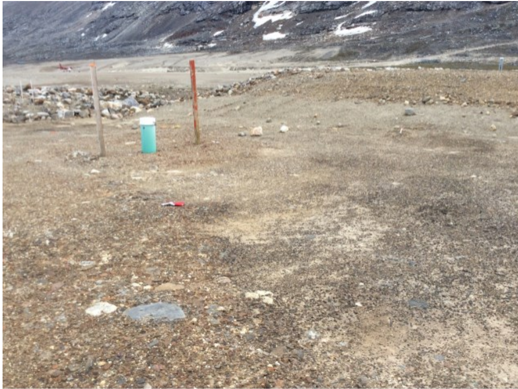
Photo 31: FOX-4 – NHWL/Tier II DF – Crest surface facing southeast – Feature N – Minor settlement (Acceptable) (ATT114_Photo114.jpg)
