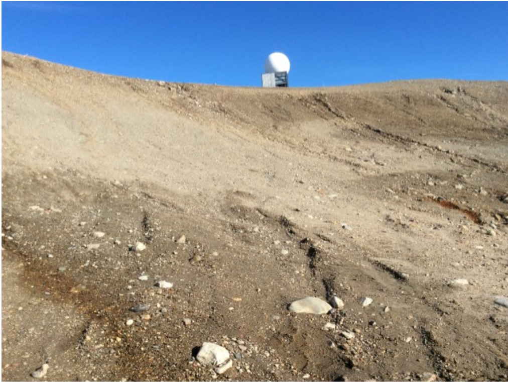
Photo 87: FOX-4 – Helipad West Landfill – NW toe facing southeast upslope – Previously observed settlement (Feature G) is uneven ground at centre and previously observed staining (Feature J) at right (ATT30_Photo30.jpg)
