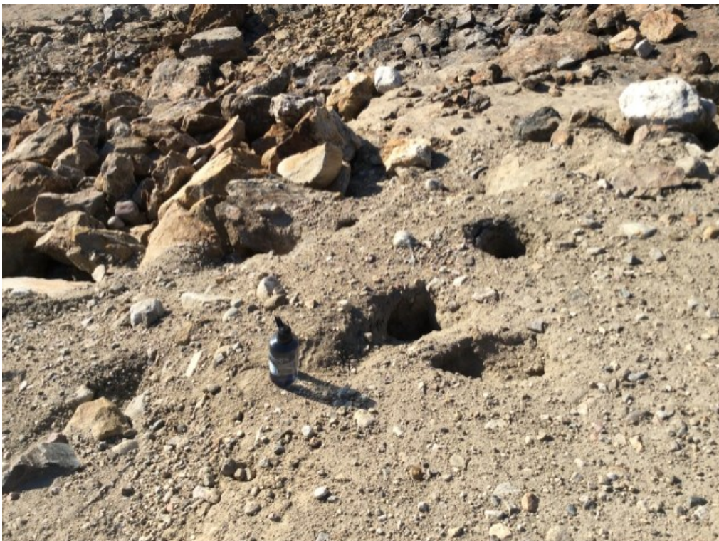
Photo 98: FOX-4 – Helipad West Landfill – West toe facing north – Feature I – Minor sink holes at edge of coarse rock fill (Acceptable) (ATT154_Photo154.jpg)
