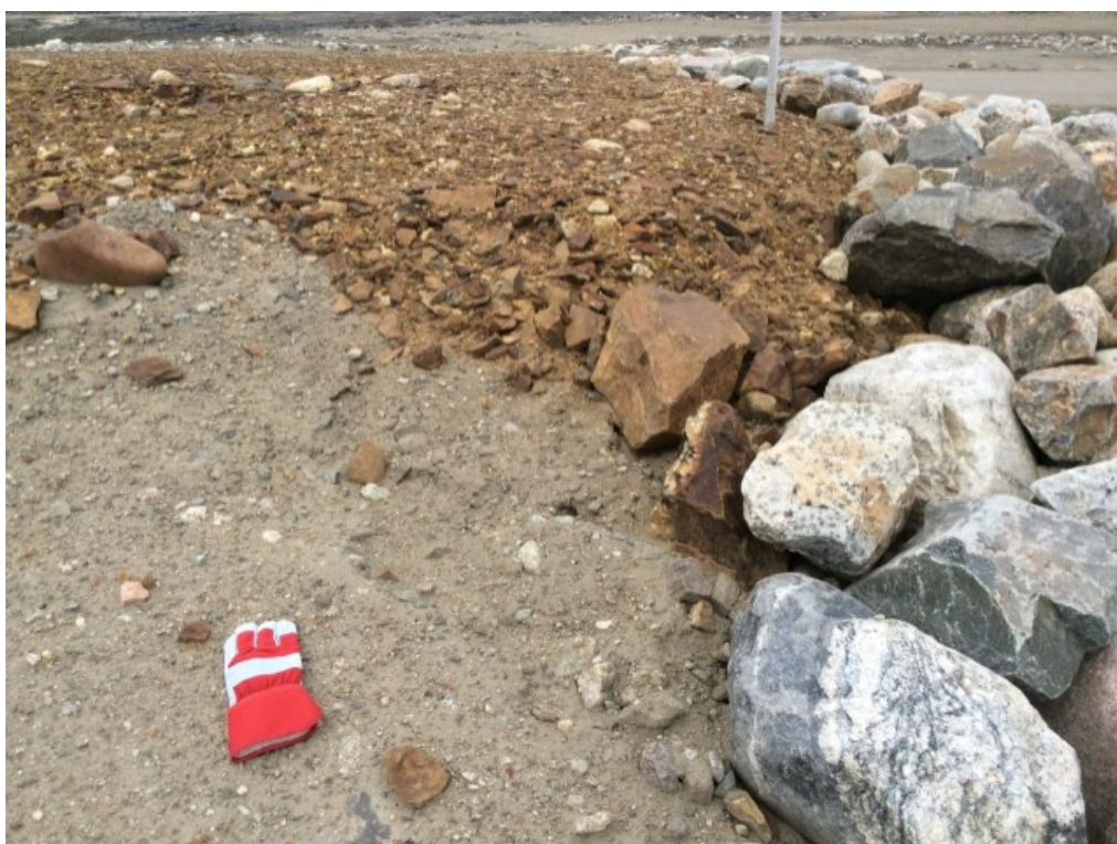
Photo 20: FOX-4 – NHWL/Tier II DF – Slope between crest surfaces facing east – Feature D – Minor erosion (Acceptable) (ATT99_Photo99.jpg)
