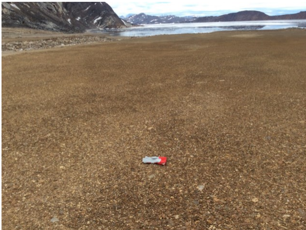
Photo 25: FOX-4 – NHWL/Tier II DF – Crest surface facing west – Previously observed minor settlement (Feature I) considered as-built undulations (Acceptable) (ATT102_Photo102.jpg)
