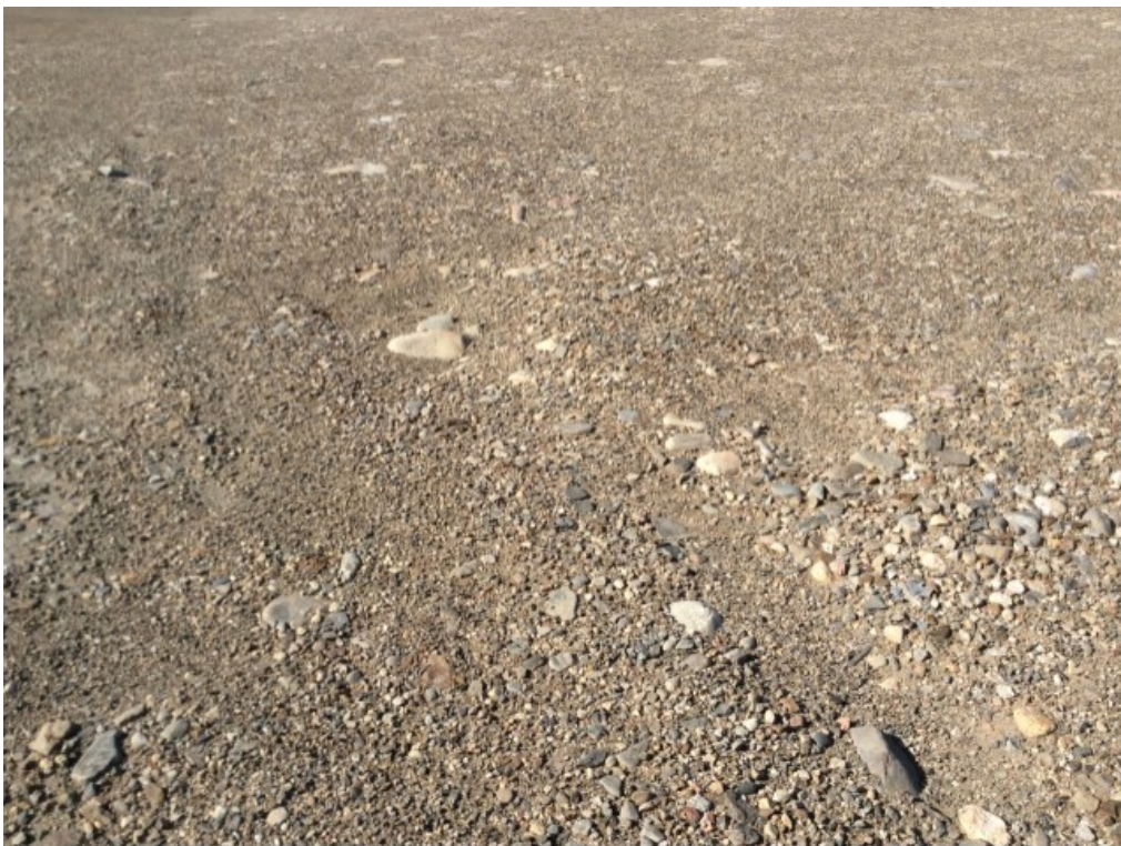
Photo 134: FOX-4 – Station Area Landfill – Central crest surface facing southwest – Feature G – Previously observed minor settlement (<0.1 m deep) may just be rough grading (Acceptable) (ATT133_Photo133.jpg)
