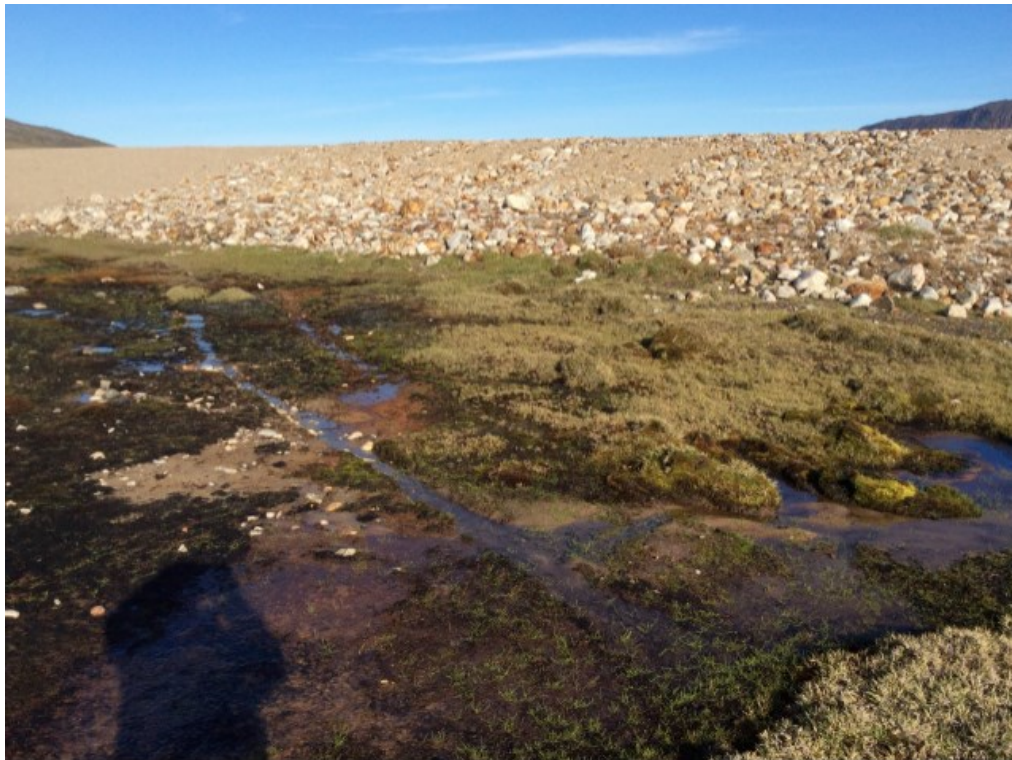
Photo 187: FOX-4 – Tanner Bay Landfill – Feature C – Ponded water at west toe, facing east (Acceptable) (ATT158_Photo158.jpg)
