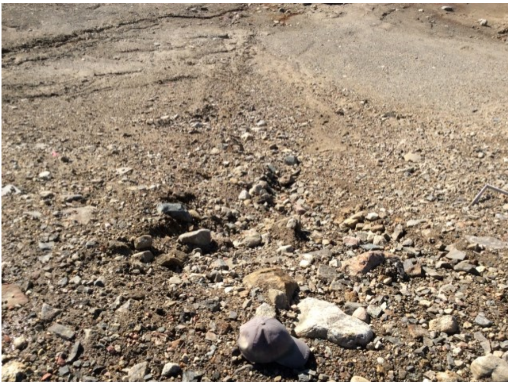
Photo 92: FOX-4 – Helipad West Landfill – Crest of slope facing northwest – Feature D – Minor self armouring erosion at top of slope (Acceptable) (ATT143_Photo143.jpg)
