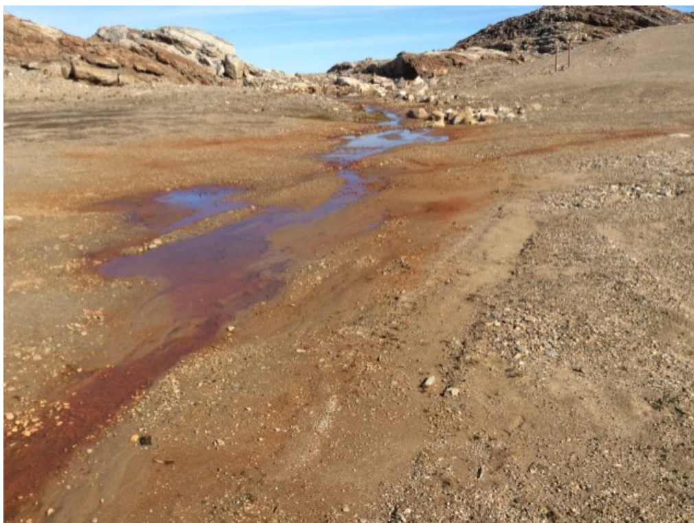
Photo 128: FOX-4 – Station Area Landfill – Northwest toe facing east – Feature B – Ponded water with orange staining (Acceptable) (ATT137_Photo137.jpg)
