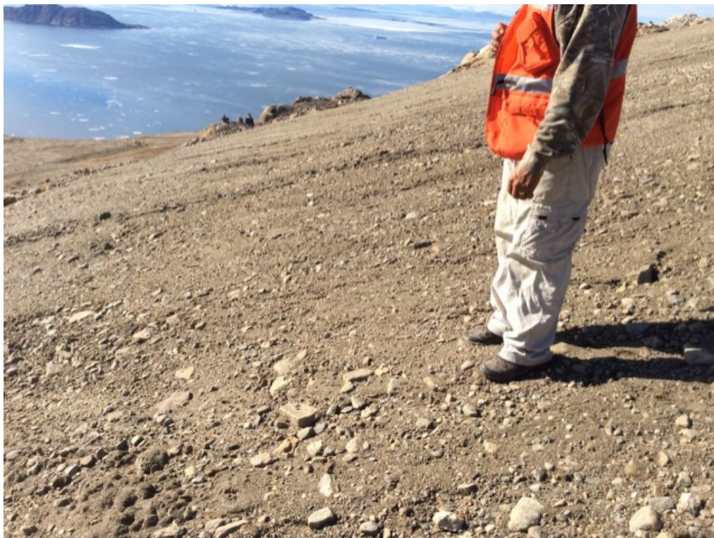
Photo 89: FOX-4 – Helipad West Landfill – SW slope facing northwest – Feature B – Minor self armouring erosion channels (Acceptable) (ATT149_Photo149.jpg)
