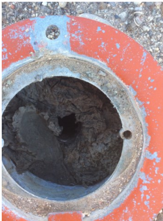
Photo 119: FOX-4 – Helipad West Landfill – MW98-06 monitoring well casing full of bentonite (ATT75_Photo75.jpg)
