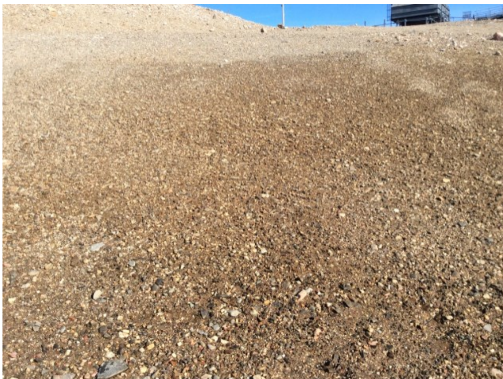
Photo 104: FOX-4 – Helipad West Landfill – Feature N – Saturated wet slope with seepage at toe – West slope facing southeast (ATT144_Photo144.jpg)
