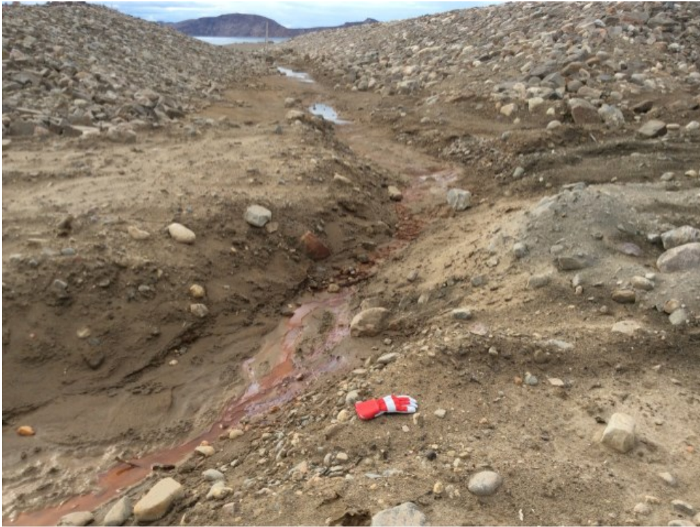
Photo 21: FOX-4 – NHWL/Tier II DF – Ditch between landfills facing west – Feature E – Orange staining and seepage (Acceptable) (ATT117_Photo117.jpg)
