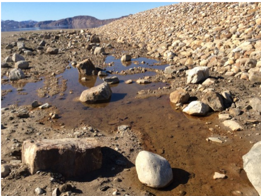
Photo 16: FOX-4 – NHWL/Tier II DF – South toe facing west – Feature B – Ponded water (Acceptable) (ATT164_Photo164.jpg)
