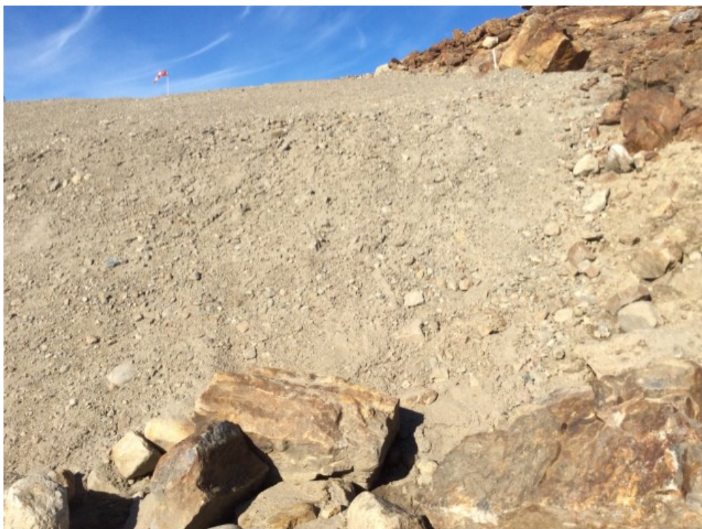
Photo 90: FOX-4 – Helipad West Landfill – South end of west slope facing north – Feature B – Minor self armouring erosion (Acceptable) (ATT150_Photo150.jpg)
