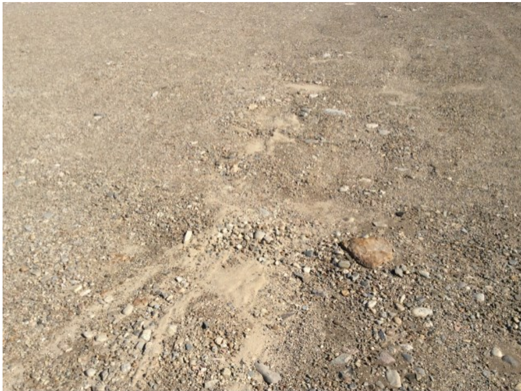
Photo 131: FOX-4 – Station Area Landfill – Crest surface facing east – Feature C – Minor self-armouring erosion (Acceptable) (ATT139_Photo139.jpg)
