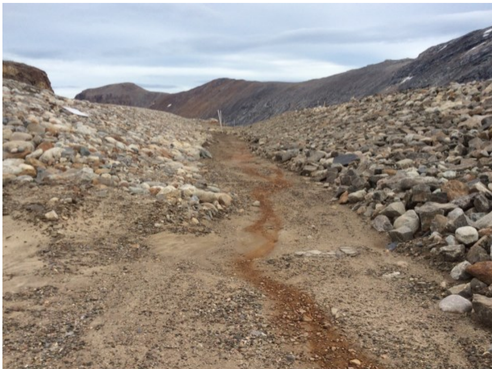
Photo 7: FOX-4 – NHWL/Tier II DF – Ditch between landfills facing east – Feature L – Orange staining (Acceptable) (ATT16_Photo16.jpg)
