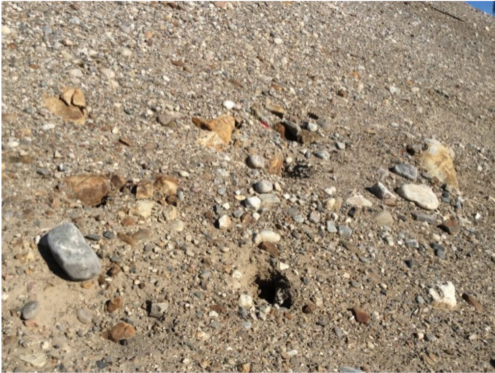
Photo 97: FOX-4 – Helipad West Landfill – Slope above landfill facing south – Feature H – Previously observed settlement area with small sinkholes (Acceptable) (ATT141_Photo141.jpg)
