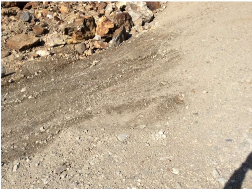
Photo 96: FOX-4 – Helipad West Landfill – NW toe facing northwest – Previously observed settlement (Feature G) appears to be area of uneven ground and not considered noteworthy in 2016 (ATT157_Photo157.jpg)
