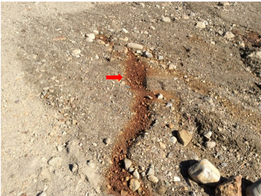
Photo 100: FOX-4 – Helipad West Landfill – Feature J – Orange staining with no seepage at time of 2016 inspection – West toe facing southeast (ATT156_Photo156.jpg)
