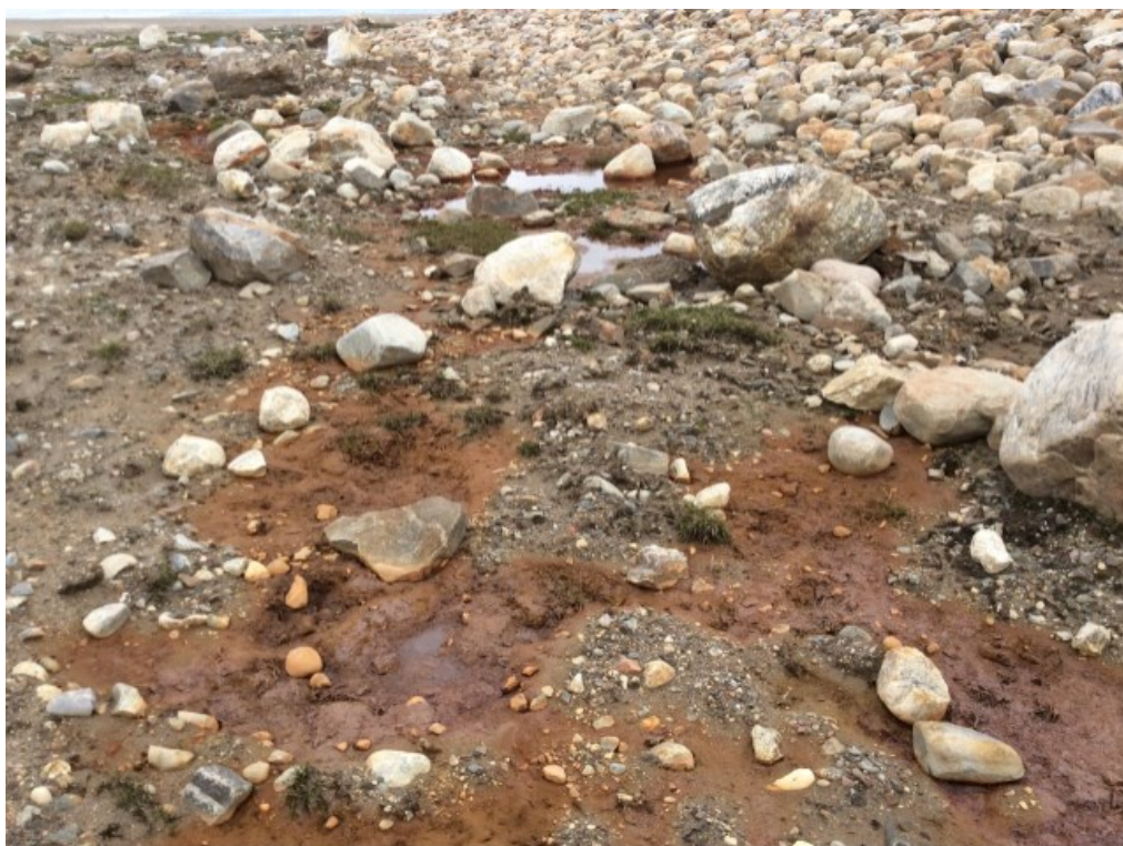
Photo 18: FOX-4 – NHWL/Tier II DF – South toe facing west – Feature B – Ponded water with some orange staining (Acceptable) (ATT97_Photo97.jpg)
