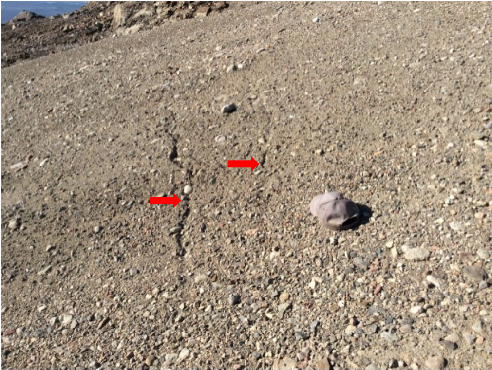
Photo 105: FOX-4 – Helipad West Landfill – West slope facing northwest – Feature O – Minor cracking at top of slope (Marginal), weathered, small parallel crack above (ATT151_Photo151.jpg)
