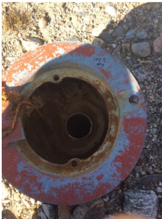
Photo 144: FOX-4 – Station Area Landfill – MW98-08 monitoring well casing filled with bentonite (ATT73_Photo73.jpg)
