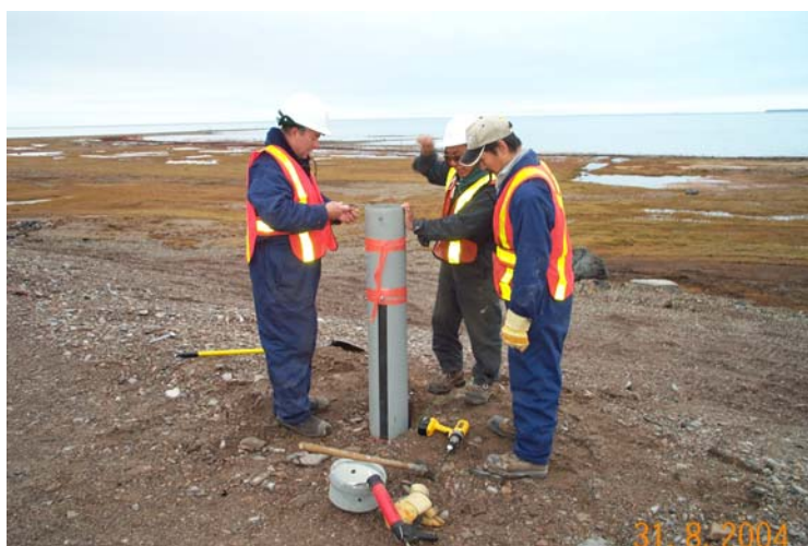
Installation of a thermistor at the Main Landfill.
