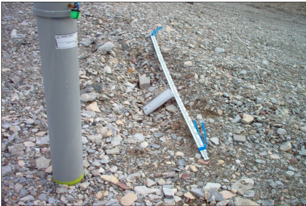
Photo B-1 Tier II Landfill. View of settlement feature A near VT-7.
