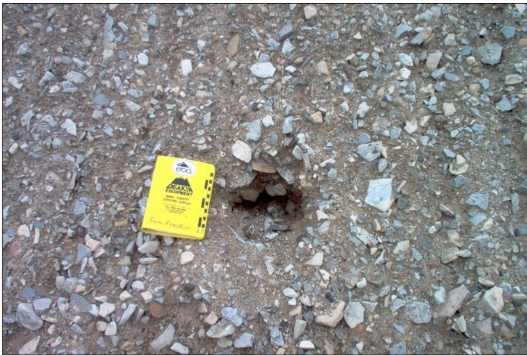
Photo A-1 Main Landfill. Close-up view of erosion feature.
