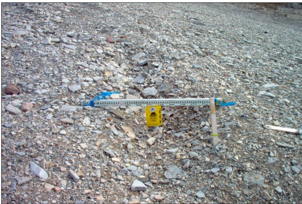
Photo B-2 Tier II Landfill. View of settlement feature B near southwest corner crest.
