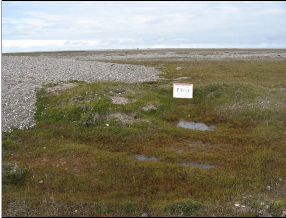
Photograph 25. South Landfill West Cell: Ponded water and staining along eastern edge of the West Cell. Pin 12958 and sample hole are located next to ponded water. Whiteboard for scale (61cm by 46cm).↑
