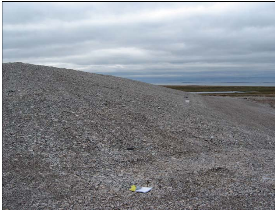
Photograph 7. Tier II Landfill: Looking S along the western toe of the landfill from about 3m N of NW corner. Broad zones of depression are visible which are consistent with poor construction finish.↑
