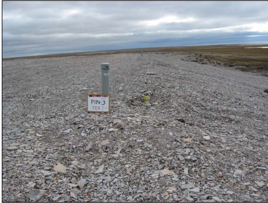
Photograph 15. Tier II Landfill: Deep rut immediately south of VT-7. The depression appears unchanged since the time of the 2006 inspection but should continue to be monitored.↑
