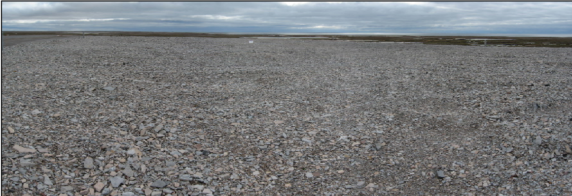
Photograph 23. Tier II Landfill: Panoramic view of top of Tier II landfill looking SE from near the NW corner. Note general undulation and inconsitent construction finish.↑
