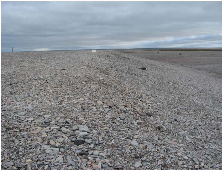
Photograph 20. Tier II Landfill: Looking N along crest from the SE corner of the landfill. Slope appears stable with no signs of slope movement. Numerous vehicle tracks and ruts are present.↑
