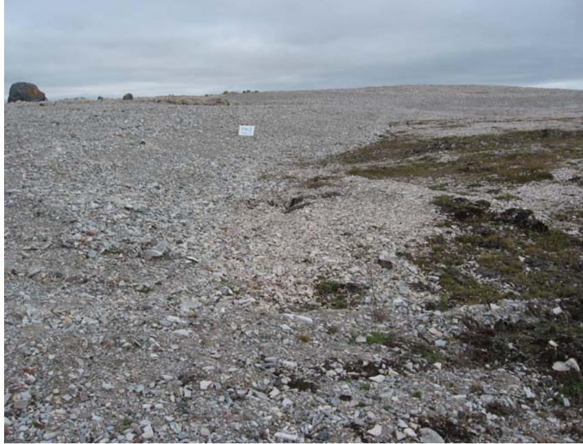
Photograph 17. NWS Landfill (West Cell): Looking east along the south edge of the landfill from the SW corner to SE corner. The landfill cover abuts organics. No indications of movement or seepage.↑
