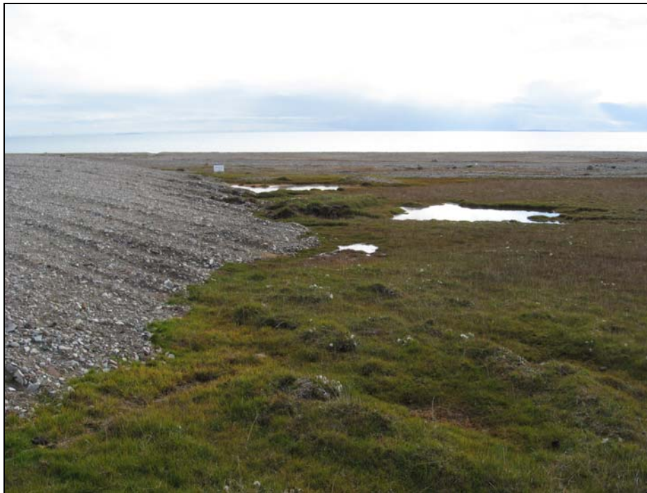
Photograph 12. South Landfill East Cell: Looking towards ponded water along the SW corner of landfill cell. Ponded water accumulates in depressions adjacent to the landfill.↑
