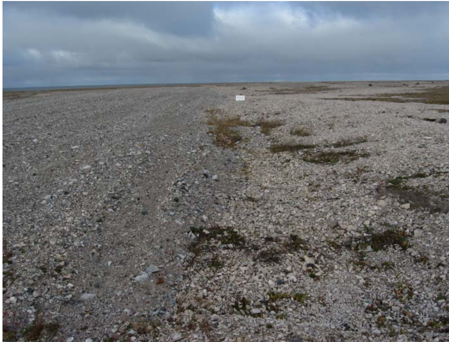
Photograph 10. North Landfill (West Cell): Looking NE along the south side of the landfill cover from the SW corner. Whiteboard located about half way to the SE corner. Toe is indistinct. Cover material is more uniform and darker grey coloured rock.↑
