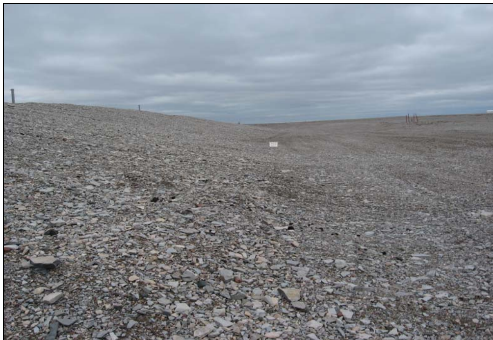
Photograph 2. Tier II Landfill: Looking west from NE corner along downslope north toe. Slope appears stable with no signs of cracking; however, inconsistent finished grade (undulations and vehicle ruts) makes it difficult to differentiate differential settlement from poor finish at the time of construction.↑
