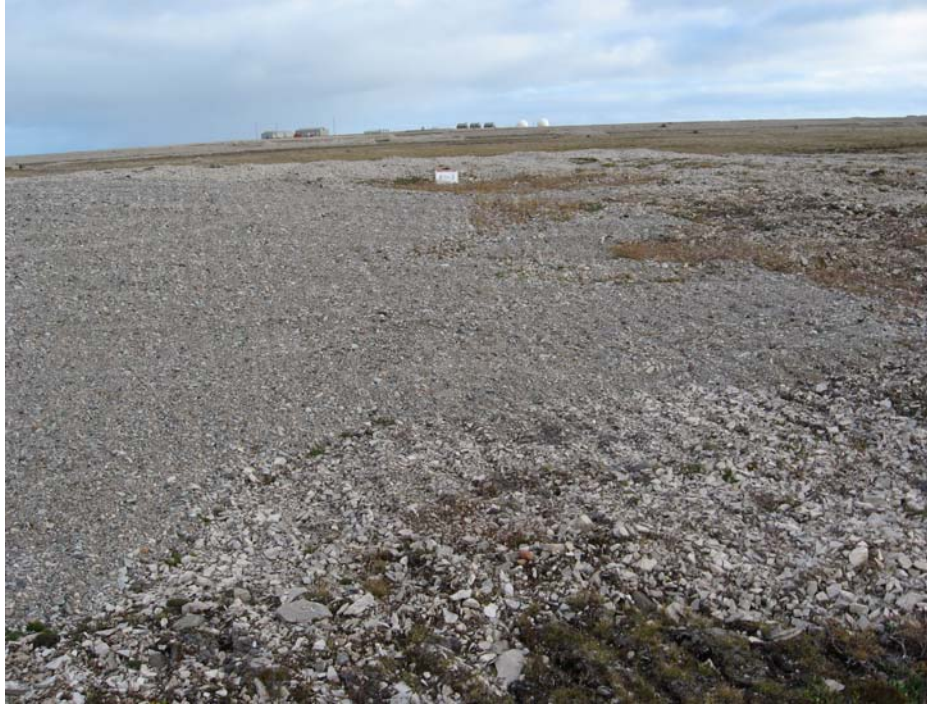
Photograph 9. North Landfill (West Cell): Looking S along the western toe of the landfill cover from the NW corner. Toe is unclear however the cover appears stable.↑
