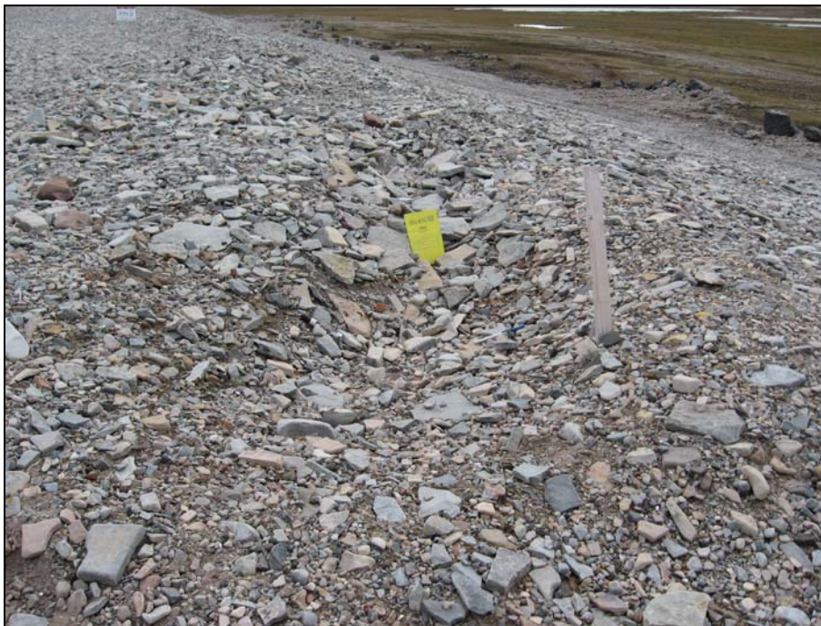
Photograph 14. Tier II Landfill: Close-up of deep rut along the crest in the SW corner of the landfill. The feature is consistent with rutting due to vehicle traffic (i.e., not settlement) but show continue to be monitored.↑
