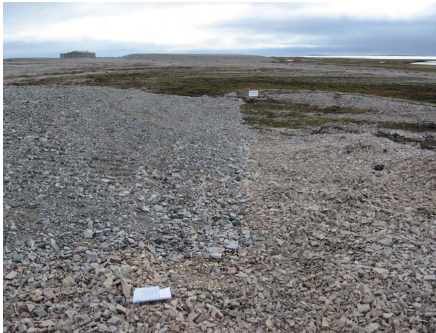
Photograph 16. NWS Landfill (West Cell): Looking SSE to SW corner NWS West. Minor organics along portion of toe. No indications of slope movement or seepage. Note Main Landfill in background.↑
