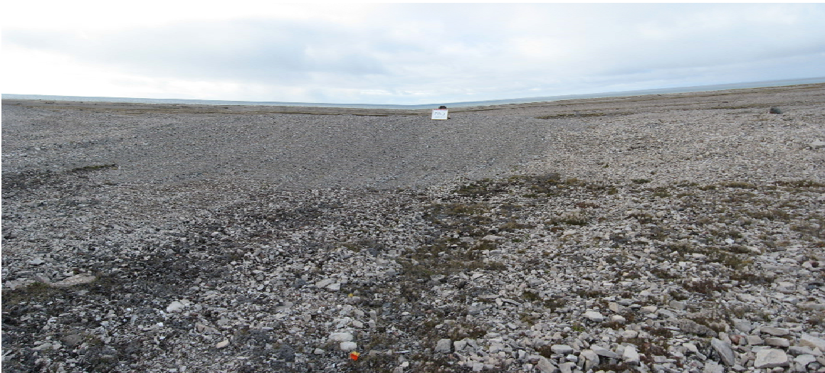
Photograph 4. North Landfill (Central Cell): Looking NW to the SW corner of the central landfill cell. Landfill cover is identifiable by the darker, uniformly coloured grey rock. Lighter coloured, less evenly graded rock to the east & west.↑
