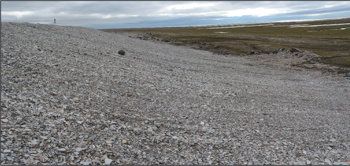
Photograph 17. Tier II Landfill: Looking east from mid-slope of the southern slope of the landfill. Thermistor VT-8 visible along crest. Slope appears stable.↑
