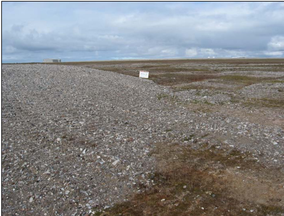
Photograph 4. South Landfill East Cell: Looking NW to NE corner of landfill. Whiteboard situated in area of previous seepage/staining (tags 12991 and 12990 indicate previous sampling).↑
