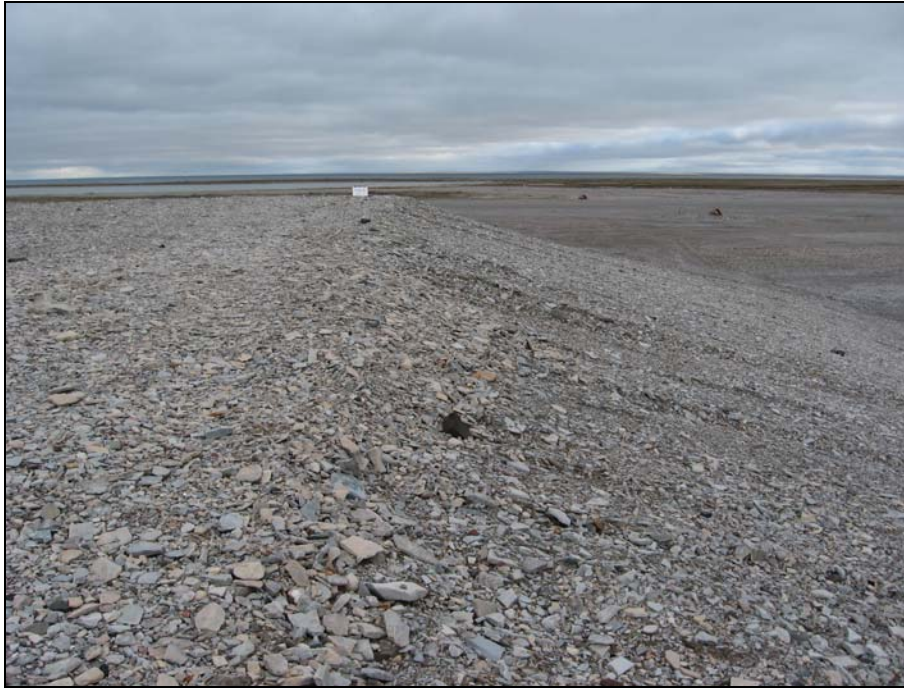
Photograph 21. Tier II Landfill: Looking N along the eastern crest of the landfill. Significant vehicle ruts and inconsistent construction finish in this area. Slope appears stable with no signs of movement.↑
