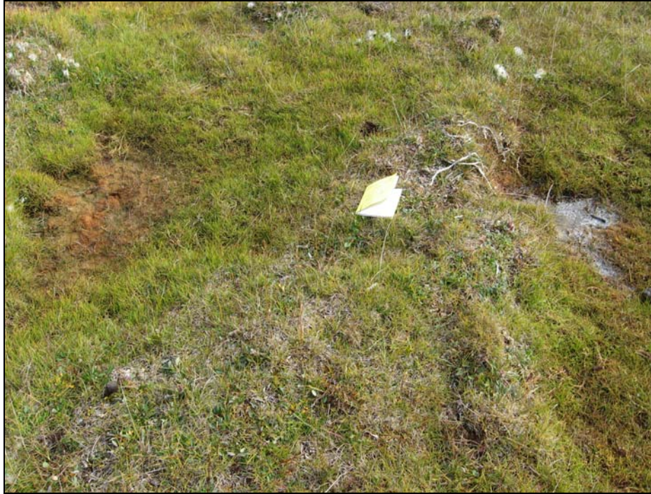
Photograph 11. South Landfill East Cell: Close up of typical staining and ponding along western perimeter of the landfill cell.↑
