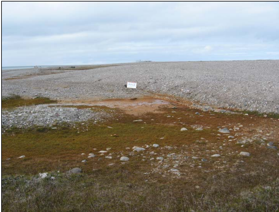
Photograph 18. South Landfill East Cell: Looking NW towards seepage area and staining along the SE corner of the landfill cell. Whiteboard for scale (61cm by 46cm).↑
