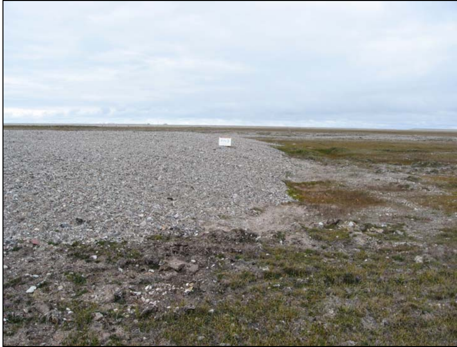
Photograph 23. South Landfill West Cell: Looking N along east side of the larger (northern) lobe of the West Cell. Displaced organics and some minor ponding, Staining along eastern toe.↑
