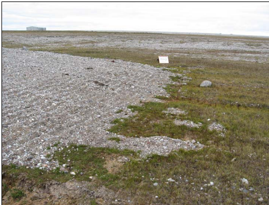
Photograph 26. South Landfill West Cell: Looking N to NE corner of larger northern lobe. Minor displacement of organics in vehicle ruts.↑
