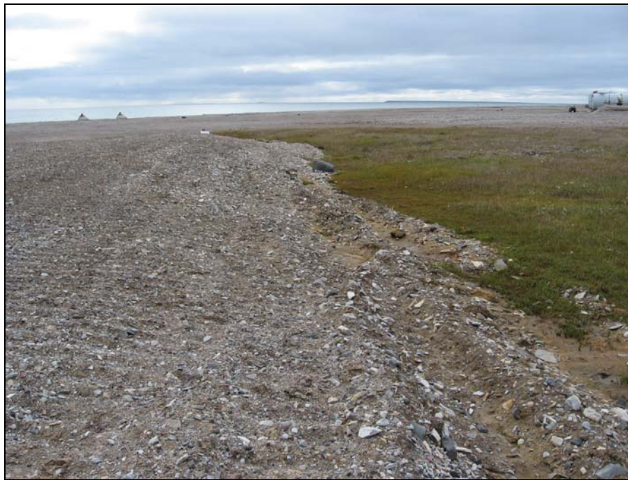
Photograph 28. South Landfill West Cell: Looking WSW along north edge of landfill cell. Heavy rutting, minor staining, indicative of periodic ponding. ↑
