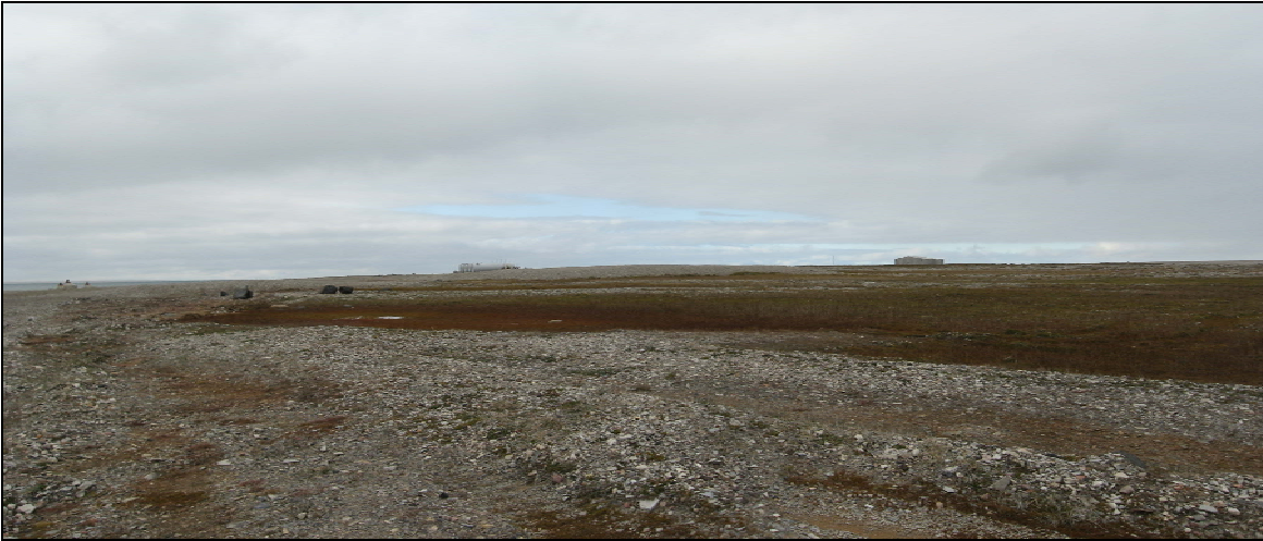
Photograph 19. South Landfill East Cell: Panoramic looking NNE over the upper surface of the landfill cover. Granular cover appears stable.↑
