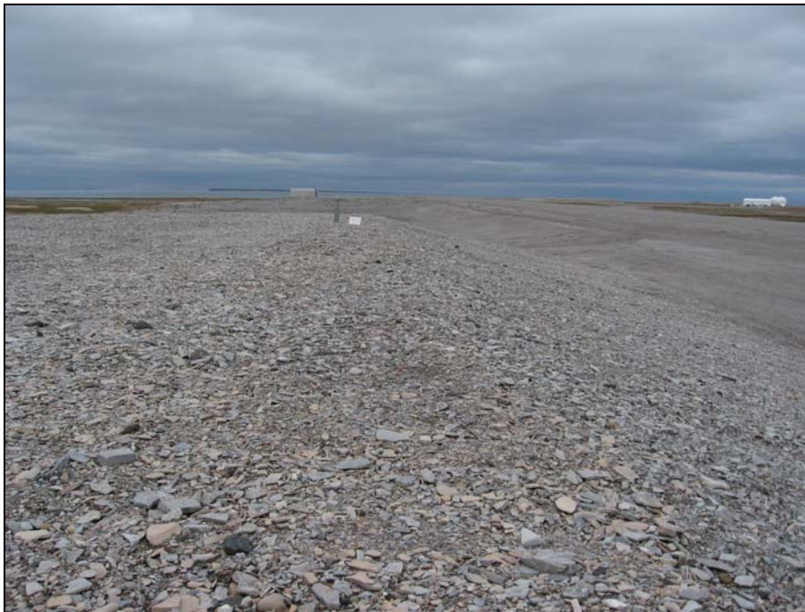
Photograph 4. Tier II Landfill: Looking west along crest from VT-6 to VT-5. Large depression just NW of VT-5 approx. 0.7m deep. Feature appears consistent with poor construction finish. Should be monitored).↑
