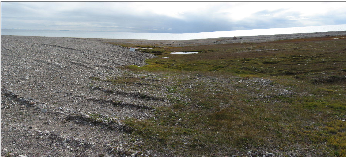
Photograph 10. South Landfill East Cell: Looking S along west side the landfill cell to standing water in displaced peat/muskeg. Pond appears smaller than last year. Orange staining around most ponded water.↑
