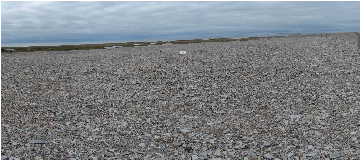
Photograph 22. Tier II Landfill: Panoramic of the top of the landfill viewed from the NE corner. There are no obvious indications of problematic conditions (e.g., significant differential settlement or slope movement). The seemingly irregular construction finish makes it difficult to observe minor changes.↑
