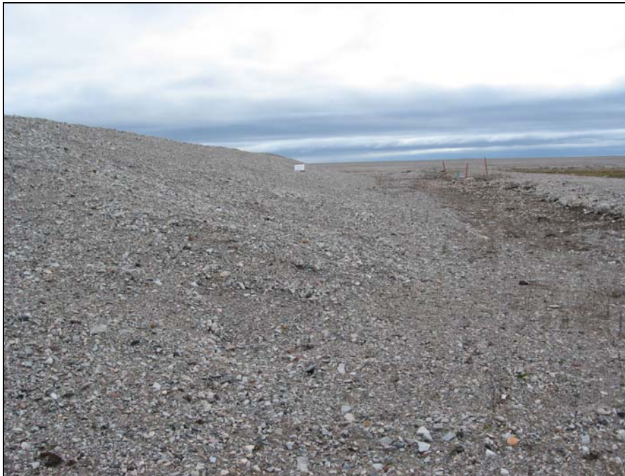
Photograph 6. Non-Hazardous Waste Landfill: Looking S along downslope toe of NW corner. Stable slope, minor irregularities in finish. The granular fill appears to be self armouring.↑
