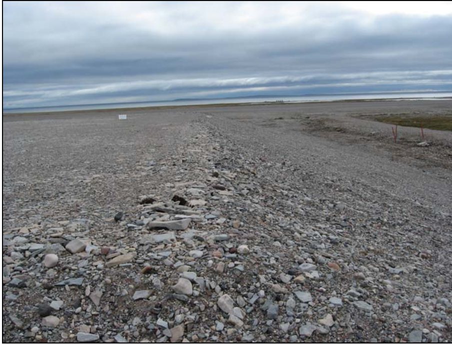
Photograph 5. Non-Hazardous Waste Landfill: Looking south along crest from the NW corner of the landfill. MW-15 visible along toe of slope. Whiteboard (61cm by 46cm) for scale.↑
