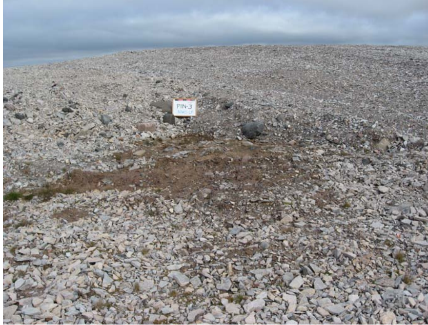
Photograph 9. NWS Landfill (Central Cell): Looking N to ponded water along west side of east cell of NWS. Water is clear. Darker ground is saturated with significant fines (mud) at surface. Ponded water is approximately 8m east of SE corner of central cell.↑
