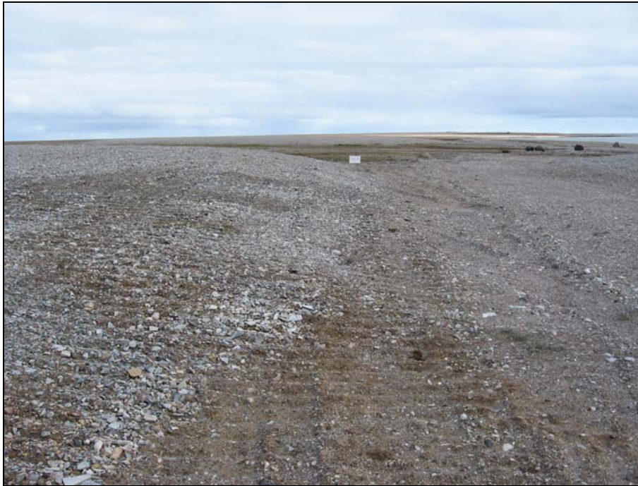
Photograph 30. South Landfill West Cell: Looking E along south side of the larger (northern) West Cell. Granular cover appears stable. South Landfill East Cell is visible in the background.
