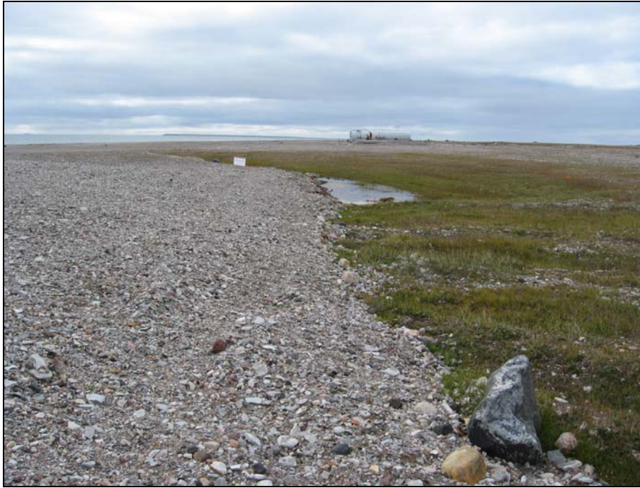
Photograph 27. South Landfill West Cell: Looking W along northern toe of north lobe. Pounded water is approximately 15m x 3m. Depression surrounded by extensive construction equipment rutting.↑
