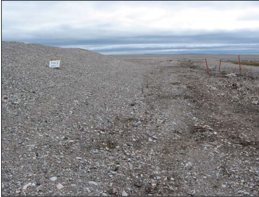
Photograph 7. Non-Hazardous Waste Landfill: Looking S along downslope toe mid-way along west side. MW-15 in the distance. Toe area is damp (organics present) but there is no clear evidence of seepage.↑
