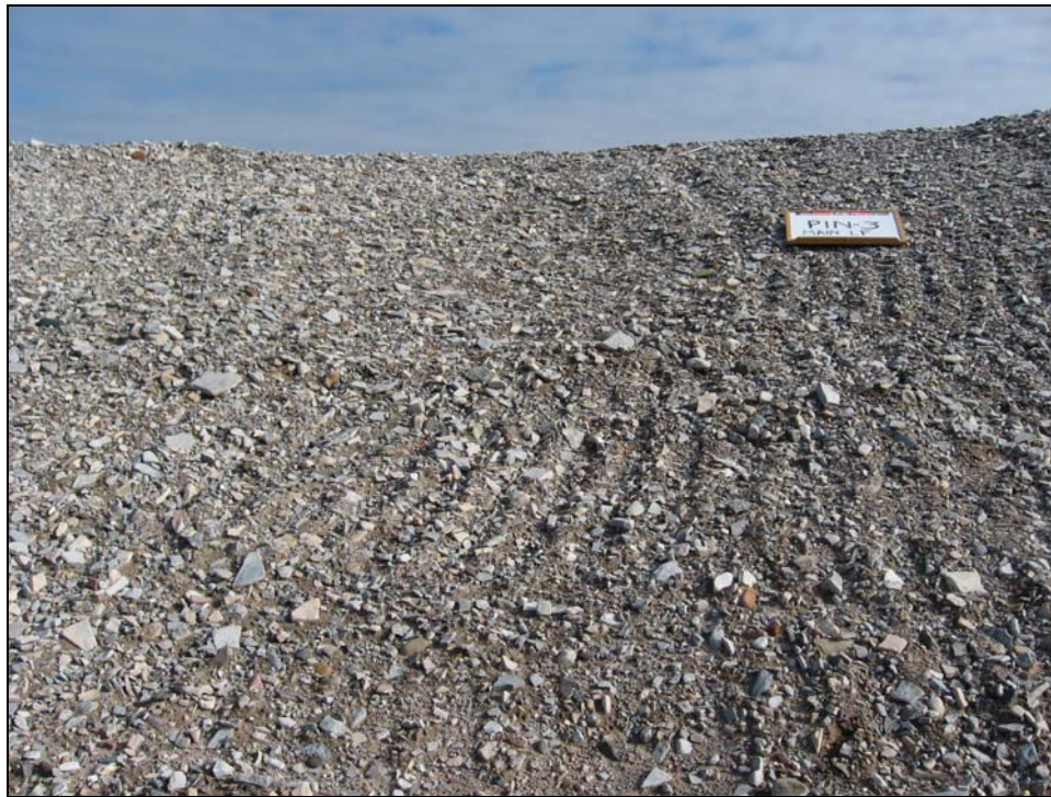
Photograph 18. Close up of area previously identified as surficial erosion to monitor. It has completely self armoured - not a problem. ↑
