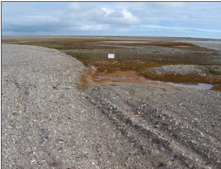
Photograph 16. South Landfill East Cell: Looking east to the SE corner of landfill. Extensive staining and indications of ongoing seepage.↑
