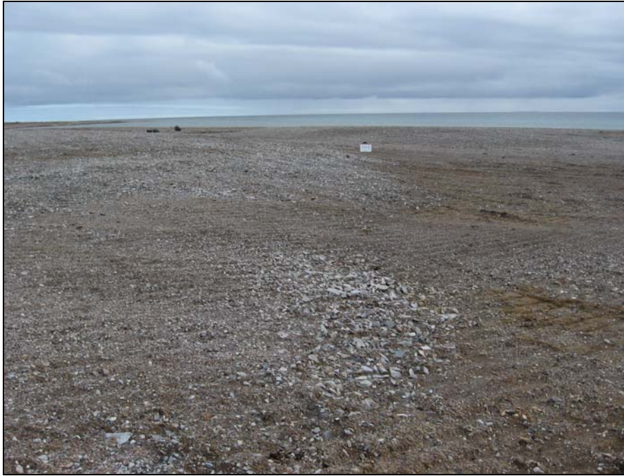
Photograph 29. South Landfill West Cell: Looking S along west sided of landfill cell. The granular cover appears stable. South lobe of the West Cell is visible in the in distance.↑
