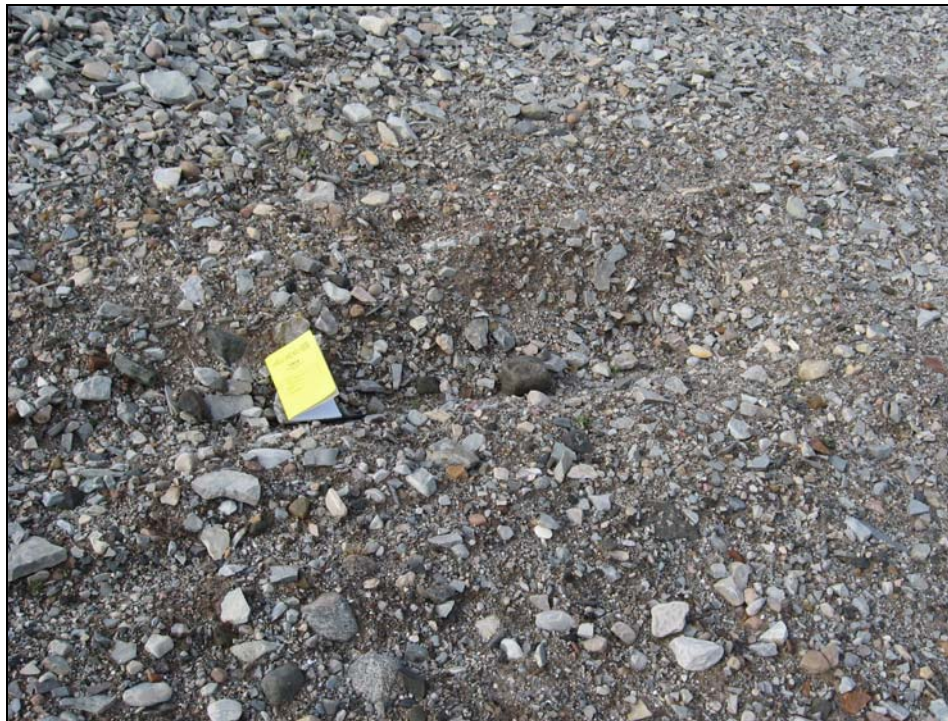
Photograph 10. Close up of rut (self armoured). ↑
