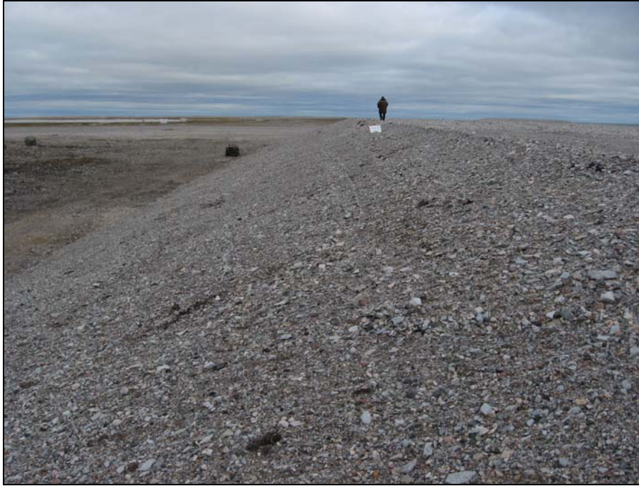
Photograph 3. Non-Hazardous Waste Landfill: Looking east from midslope NW corner. Slope appears stable with no indications of degraded performance.↑
