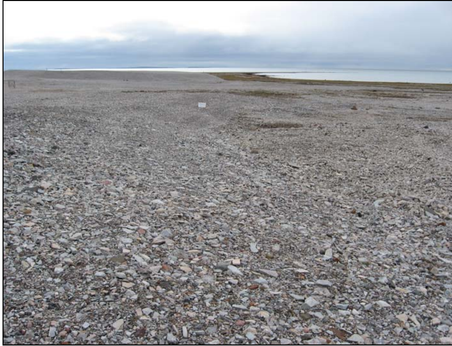
Photograph 5. NWS Landfill (East Cell): Looking south along west side of the east cell to the SW corner. Landfill cover rock can be differentiated from adjacent ground cover rock by the more uniform grey colour.↑
