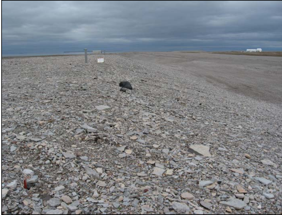
Photograph 3. Tier II Landfill: Looking west along crest from NE corner to VT-6. There is a 0.5m deep depression about 4m x 6m wide centred 4m NE of VT-6. Appears consistent with poor construction finish (i.e., not post construction settlement) but will need to be monitored.↑
