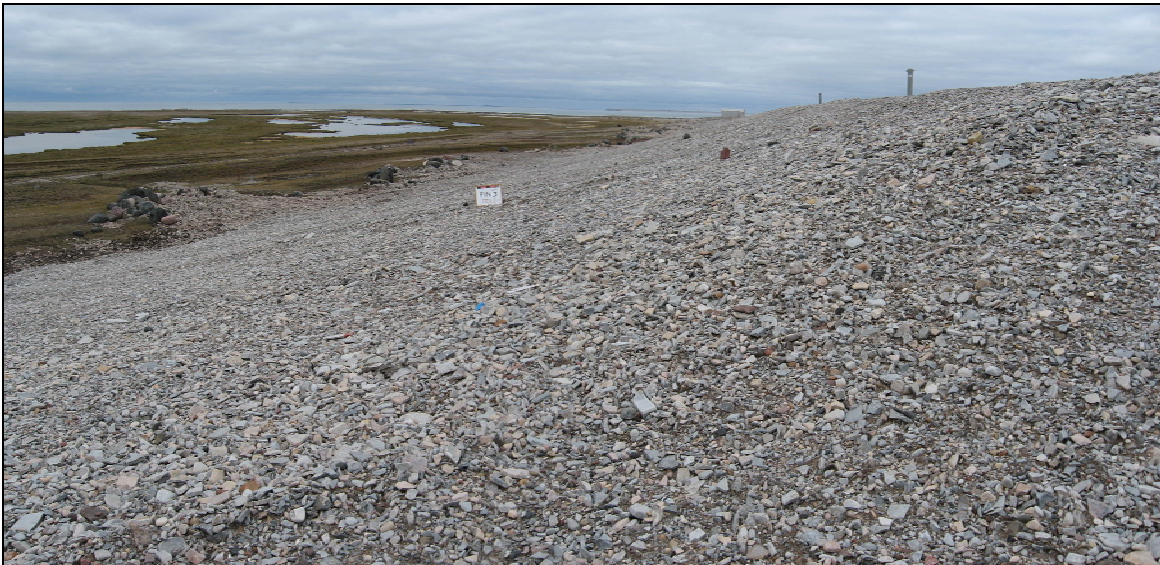
Photograph 18. Tier II Landfill: Panoramic looking WSW along south slope of the landfill from mid-slope of the SE corner. Whiteboard is located slightly west of a shallow zone of depression. Slope appears stable with no indication of slope movement. The area(s) of depression are consistent with construction finish but should continue to be monitored for change.↑
