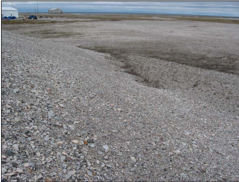
Photograph 12. Non-Hazardous Waste Landfill: Looking NE to toe of slope/access road interface from centre crest east slope. Slope abuts onto organic layer (darker area). No indications of instability.↑
