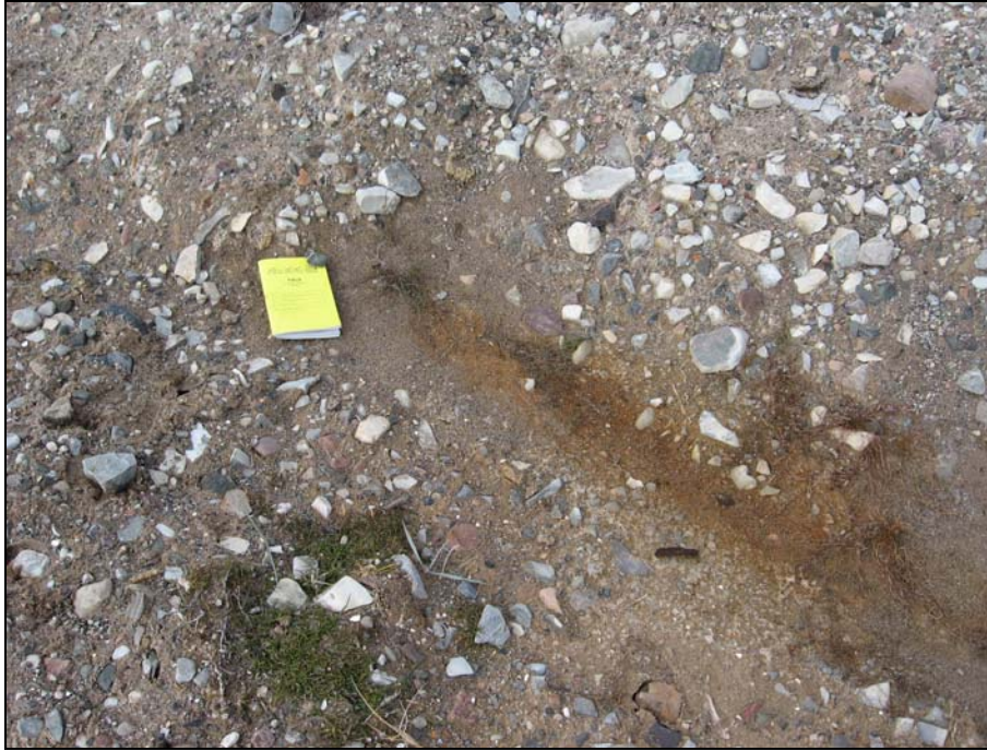
Photograph 17. South Landfill East Cell: Staining/seepage along the SE portion of the landfill cell. Seepage appears to come to surface adjacent to the field book.↑
