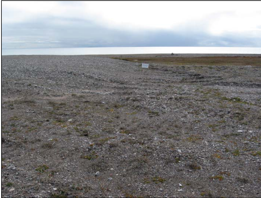
Photograph 9. South Landfill East Cell: Looking south along the West side of the landfill cell from 10 m NW of the NW corner. Gravel slope pushed into peat. Geometry is problematic for surface drainage.↑
