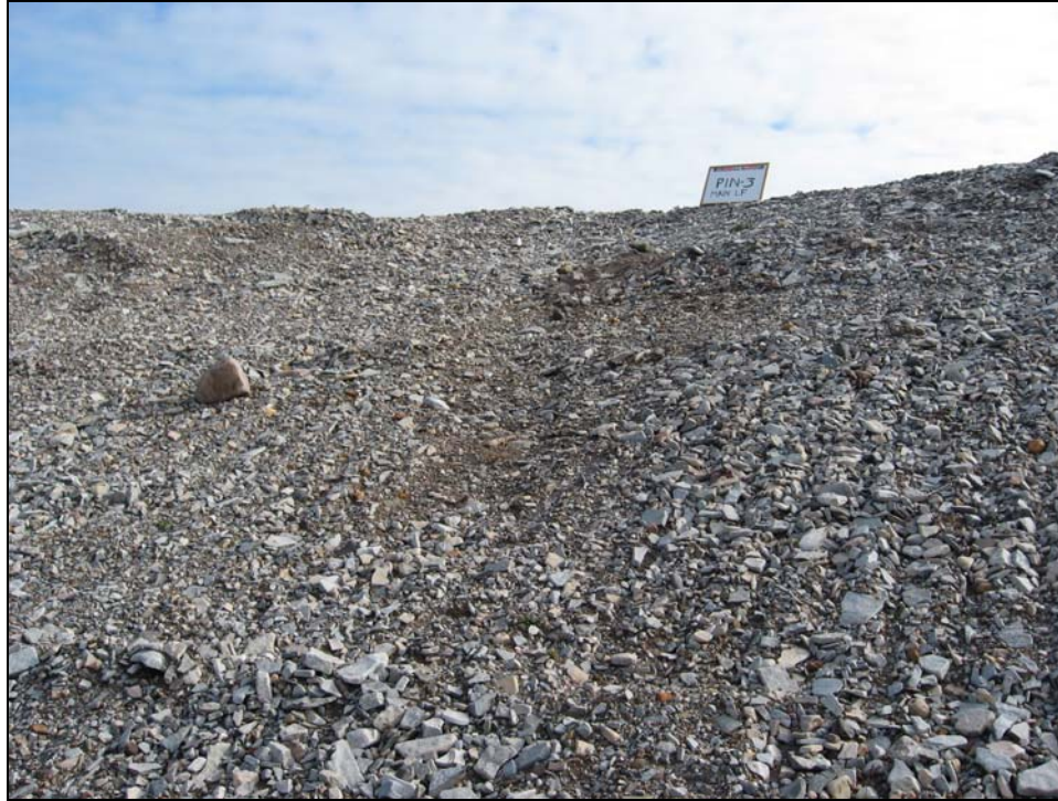
Photograph 19. Close up of another area previously identified as erosional and to monitor. Self armoured, not problematic. Looking upslope ENE.↑
