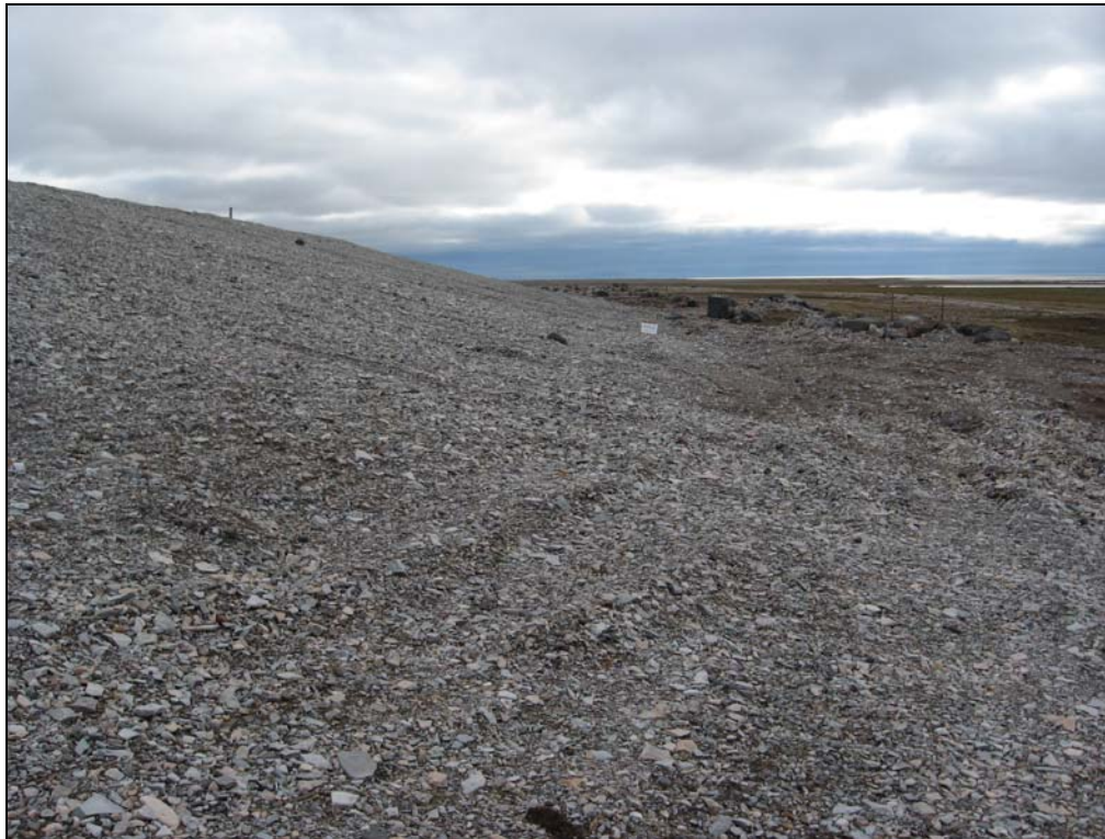
Photograph 12. Tier II Landfill: Looking east along the downstream toe of the landfill from the SW corner. Slope abuts into organic layer. Slope has relatively gentle grade and appears stable.↑
