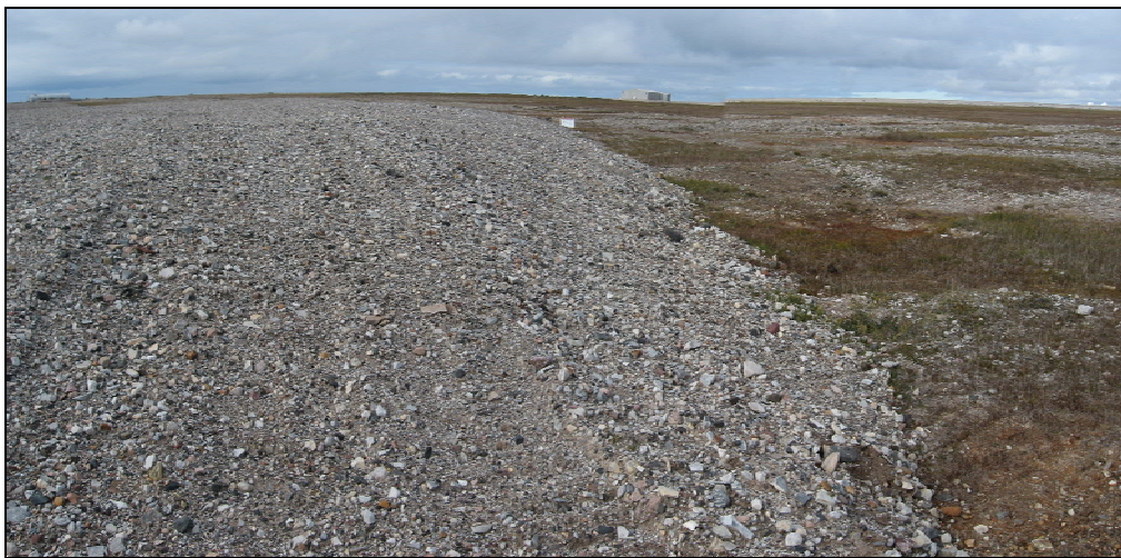
Photograph 6. South Landfill East Cell: Looking NW along NE edge of landfill. Entire downslope toe is dry. No signs of instability.↑
