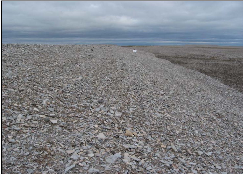
Photograph 10. Non-Hazardous Waste Landfill: South slope looking East to the SE corner from mid-slope, mid-way to corner. The slope has a slightly irregular finish and steepens (still gentle) downslope of whiteboard towards the toe of slope. Slope appears stable with no indications of degraded performance.↑
