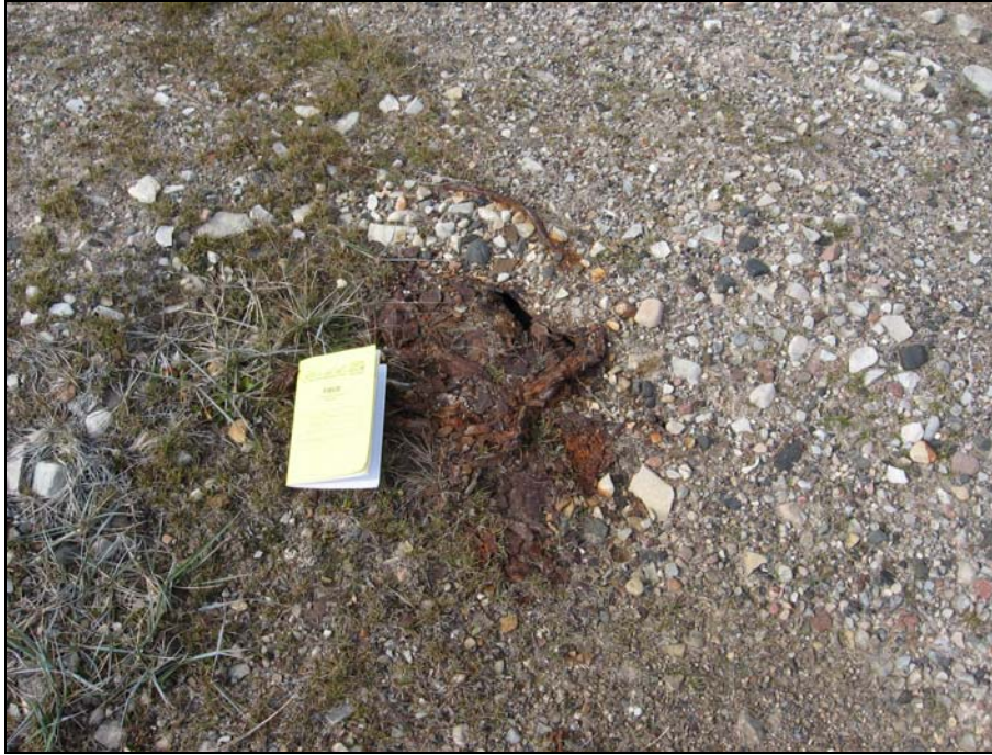
Photograph 7. South Landfill East Cell: Close up of rusty barrel exposed at surface.↑
