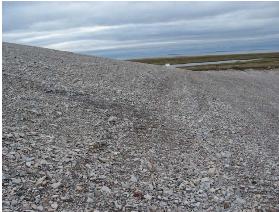
Photograph 10. Tier II Landfill: Looking S along the western toe of slope to the SW corner of the landfill. No features of note. Slope appears stable with no indications of instability or slope movement.↑
