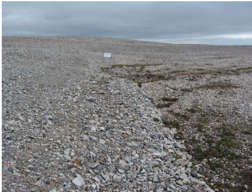
Photograph 18. NWS Landfill (West Cell): Looking to SE corner from midpoint of south side of the western cell. No staining or ponding. Note organics along perimeter. White board for scale (61cm by 46cm).↑
