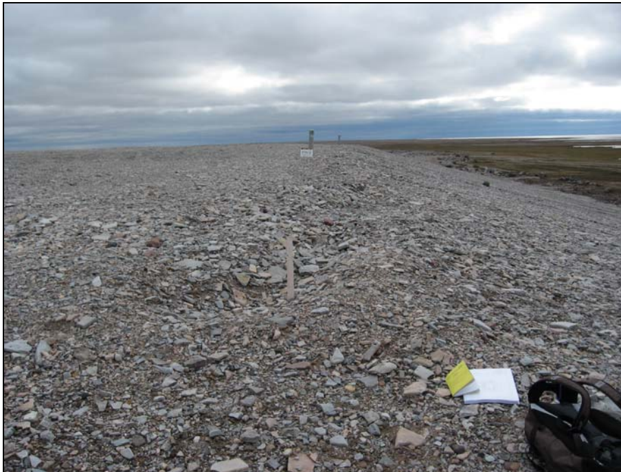
Photograph 13. Tier II Landfill: Looking east along the top of slope to VT-7 from SW corner of the landfill. Note the deep rutting in foreground and irregular rutting and fill placement along crest. The granular fill is self armouring and not susceptible to erosion by surface runoff. ↑
