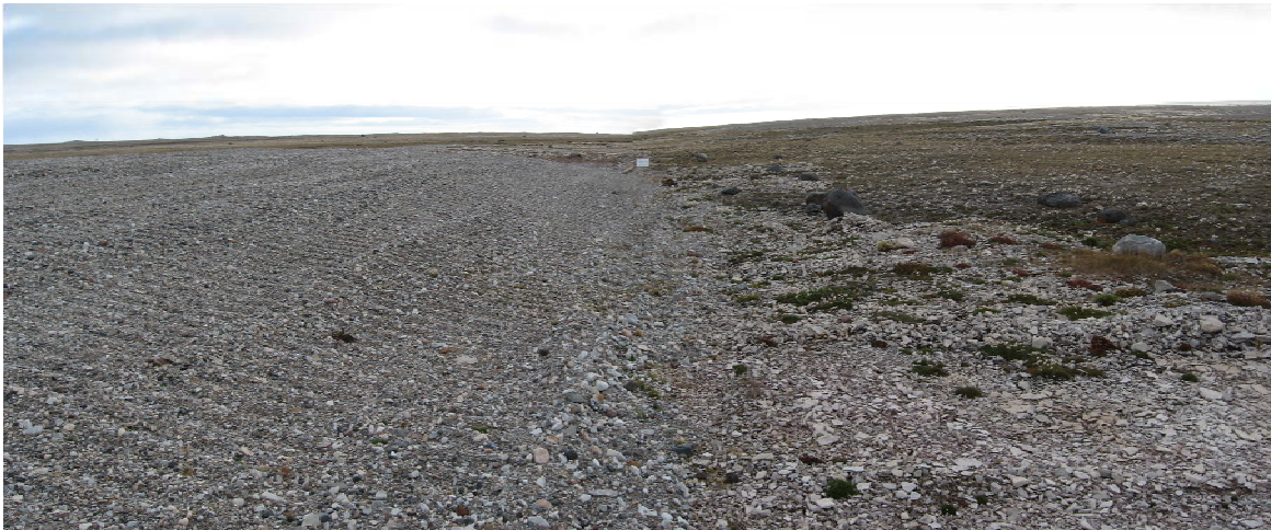
Photograph 8. North Landfill (West Cell): Looking SW along the north toe of the landfill cover. Whiteboard located at the NW corner of the cell. Cover is stable. No features of note.↑
