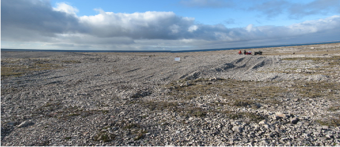
Photograph 1. North Landfill (East Cell): Looking NW from about 15m S of SE corner. Granular cover is rutted due to heavy equipment traffic (likely associated with construction) but appears stable and is self armouring against erosion.↑
