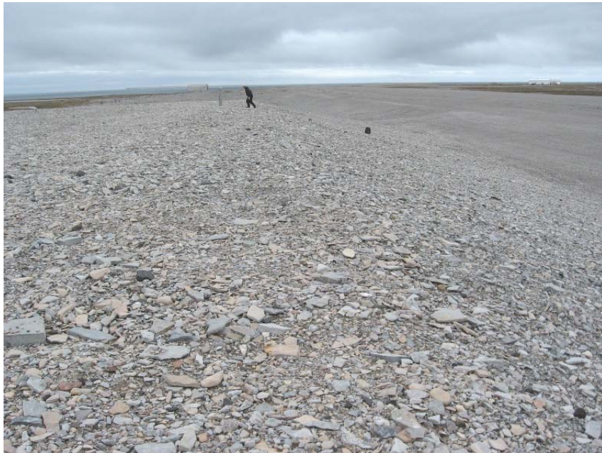
Photograph T2-4. Looking W along crest of N face from adjacent to VT-6. Looking to VT-5. A large zone of depression (approx. 10m x 10m and up to 0.5m deep) centred about 12m north of VT-5 appears unchanged from previous inspection. No indications of slope movement. ↑
