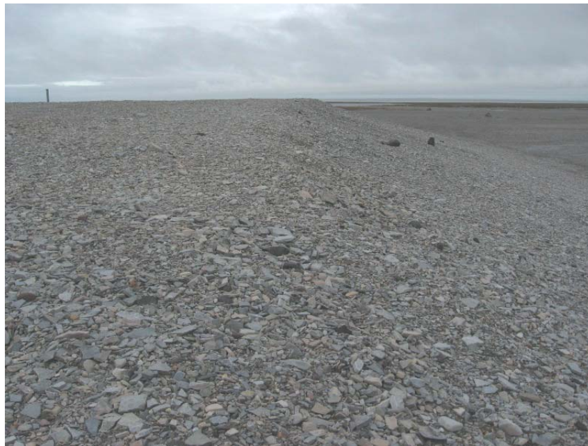
Photograph T2-20. Looking N along E crest from about SE corner. Significant vehicle ruts and inconsistent construction finish in the area. Slope appears stable and the surface irregularities are self armouring and not susceptible to further erosion. ↑
