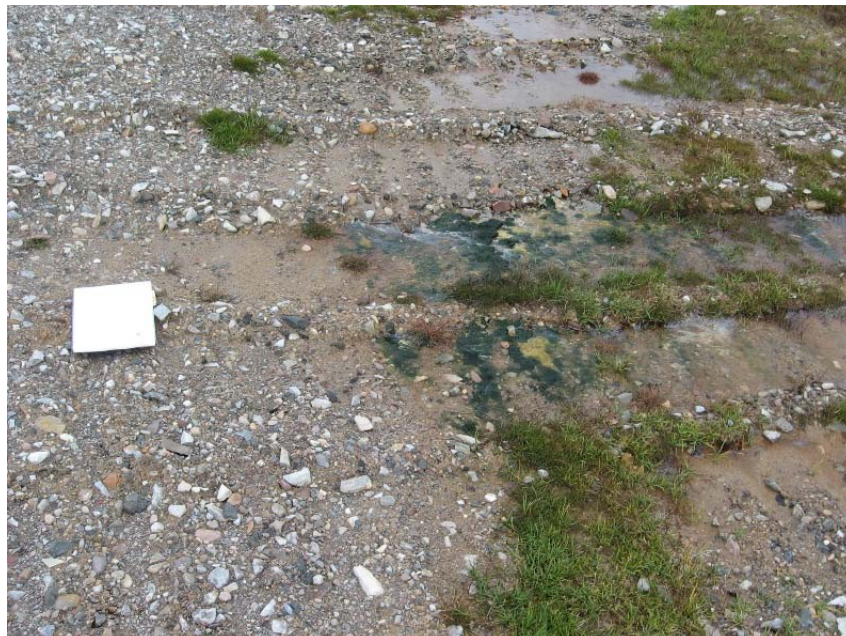
Photograph SLF-4. Close-up of green algae growing along toe in area of staining. ↑
