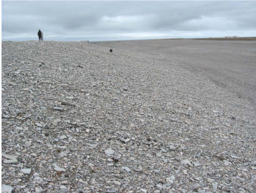
Photograph T2-5. Looking W from mid-slope along N face. Backpack is located near eastern limit of the above noted zone of depression. Zone of depression appears unchanged since previous inspection; however, no as-built survey is available for comparison. ↑
