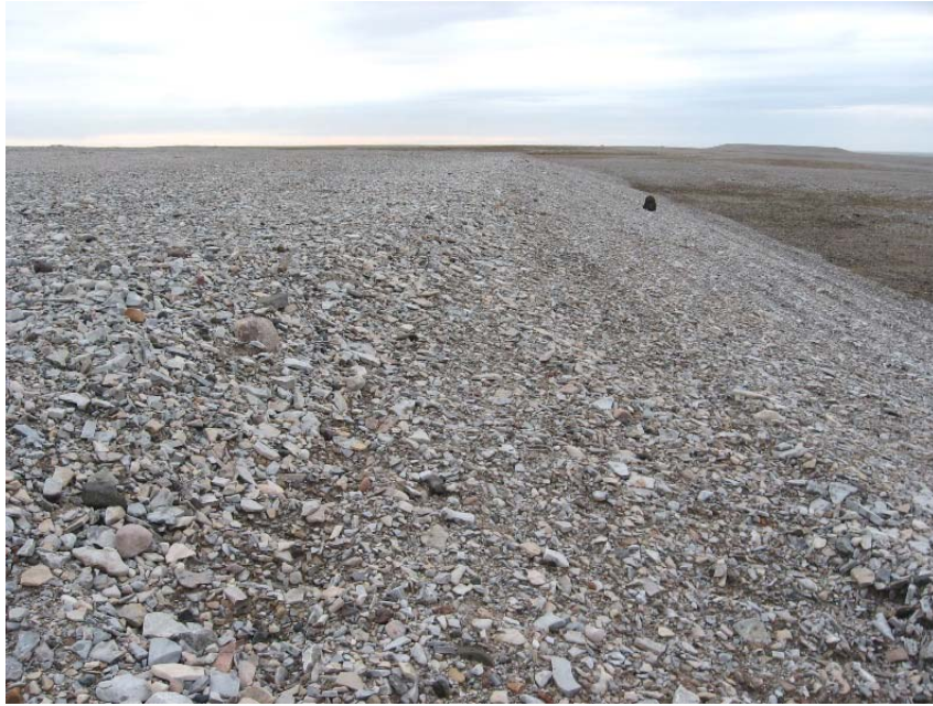
Photograph NonHaz-9. Looking E along crest from SW corner. Note final granular capping layer does not extend all the way to original granular side slope (i.e. ends abruptly, does not grade uniformly). ↑
