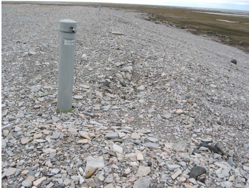
Photograph T2-15. Close-up of deep rut adjacent to VT-7. Unchanged from previous two inspections. The rut is self armoured and not susceptible to further erosion. No indications of slope instability. ↑
