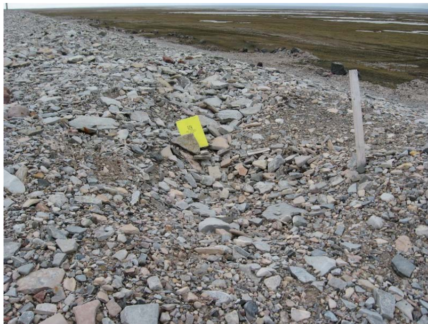
Photograph T2-14. Close-up of deep rut along crest of SW corner. Unchanged from previous two inspections. ↑
