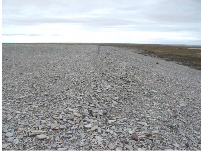
Photograph T2-13. Looking E from SW crest of the LF. VT-7 in foreground, VT-8 further away. Deep rutting (up to 0.5m deep x 1m wide x 5 m long) appears to be a construction remnant. The rut is self armoured and not susceptible to further erosion. ↑
