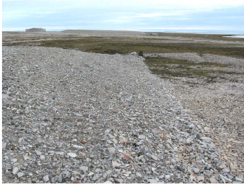
Photograph NWS-17. Looking S to SW corner of West cell from NW corner. Stable interface with organics. Main LF and hangar visible in the background. ↑
