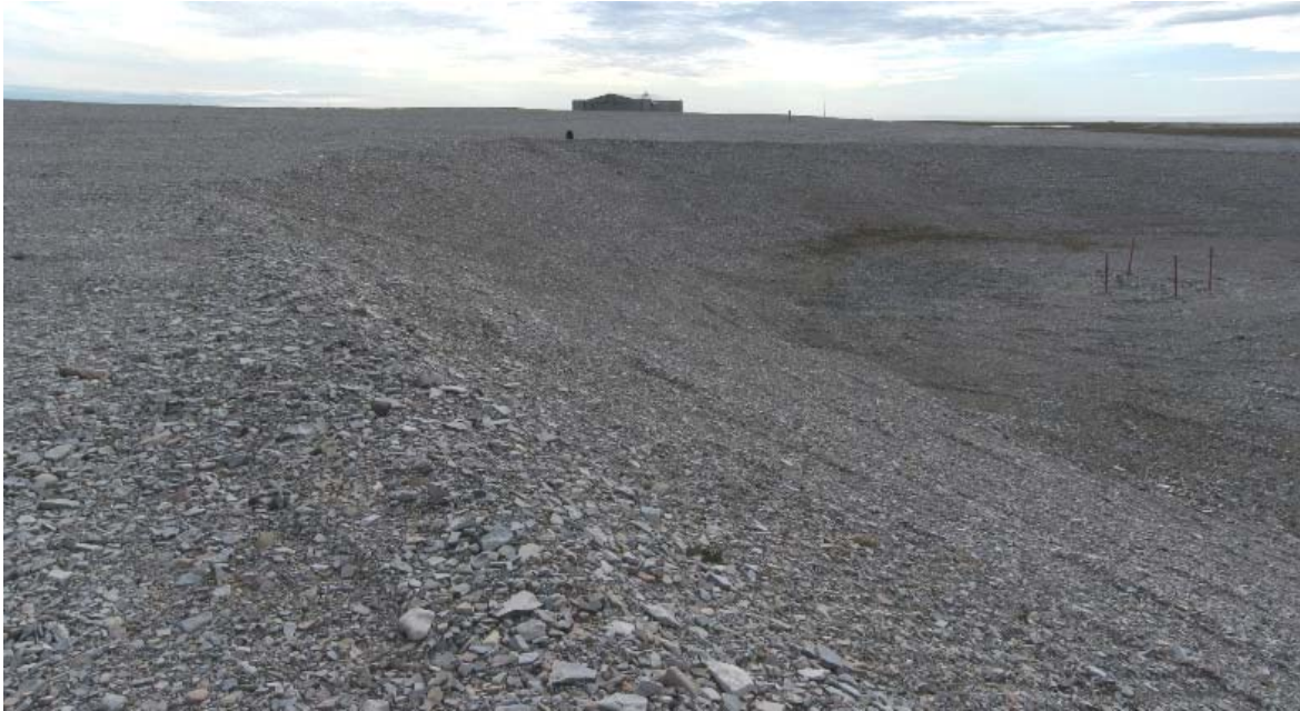
Photograph MLF-15. Panoramic looking ESE to SE from crest to curved slope. Hangar and VT-3 visible in the background. Slope and crest appear stable and well armoured. ↑
