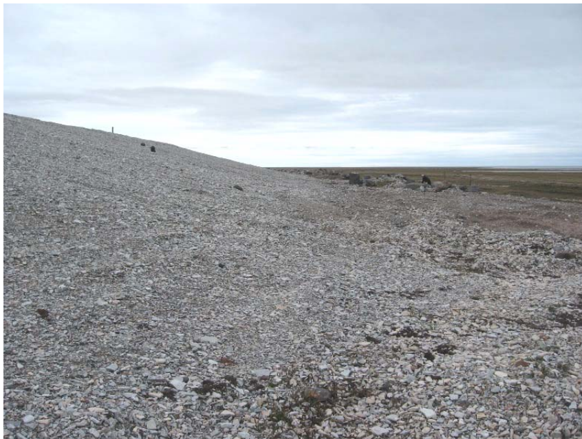
Photograph T2-12. Looking E along S slope from partway up slope near SW corner. MW-11 visible in distance to the south of the toe of slope. Slope has relatively gentle grade and abuts into organic layer. No indications of slope instability. ↑
