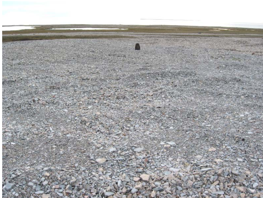
Photograph NWS-15. Looking W from NE limit of cover to what appears to be NE crest. Landfill limits are poorly defined due to the continuous gravel cover in the area around the landfill cells. ↑
