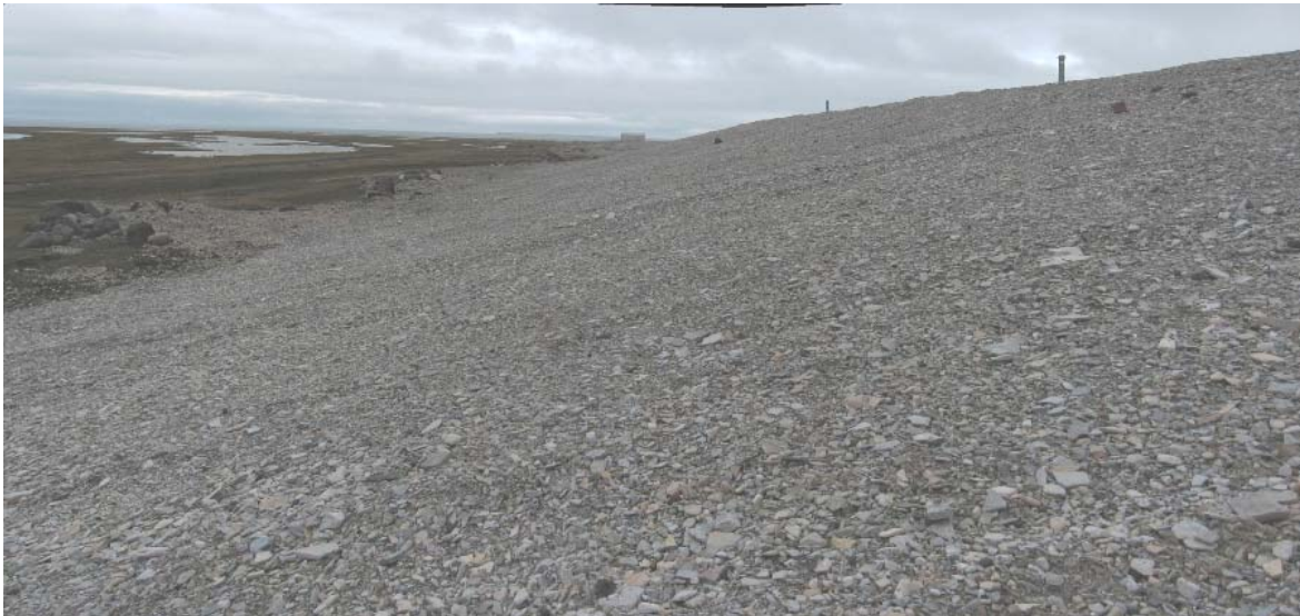
Photograph T2-18. Looking W along S slope from about mid-slope near SE corner. VT-8 (near) and VT-7 (distant) visible along crest. Minor surface irregularities and undulations are visible (consistent with irregular construction finish); however, the slope appears stable. ↑
