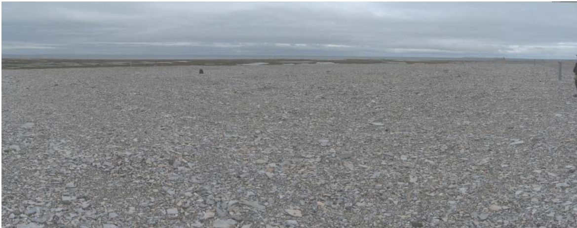
Photograph T2-22. Panoramic, L to R, looking SW from NE corner. VT-6 visible along right side of photo. No clear indications of problematic conditions (i.e., slope movement or significant differential settlement). The irregular surface (poor construction finish) masks minor changes. Condition of the landfill cover should continue to be monitored. ↑
