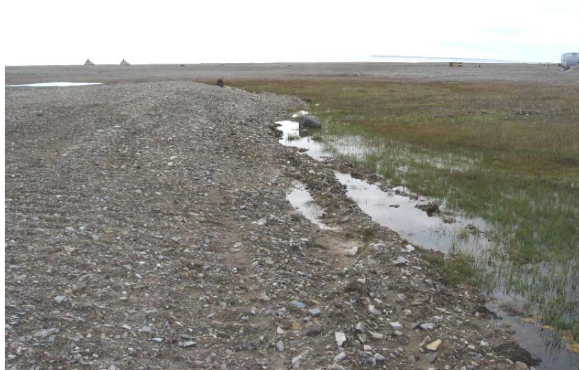
Photograph SLF-25. Looking W to the NW corner of North cell. Ponded water along most of toe.
