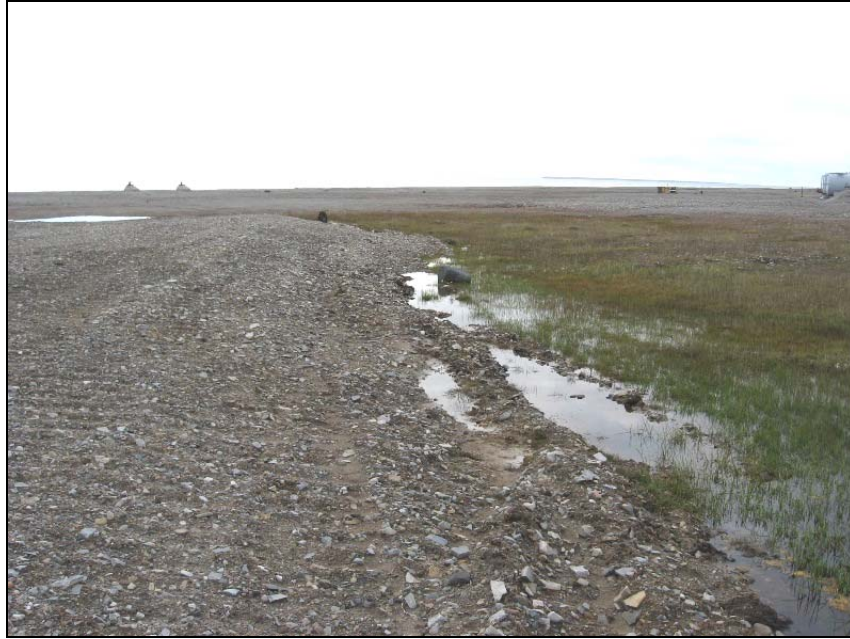
Photograph SLF-25. Looking W to the NW corner of North cell. Ponded water along most of toe. ↑
