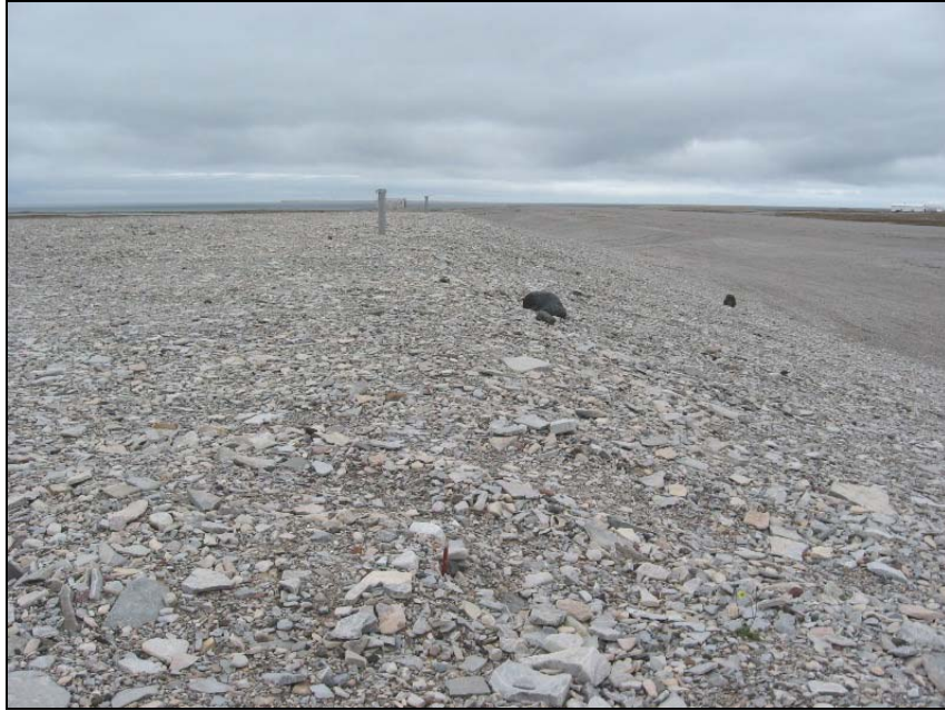
Photograph T2-3. Looking W along crest from NE corner of landfill. VT-6 visible in frame. A depression (0.5mx 4mx6m) centred about 4m NE of VT-6 appears unchanged from previous inspection. ↑
