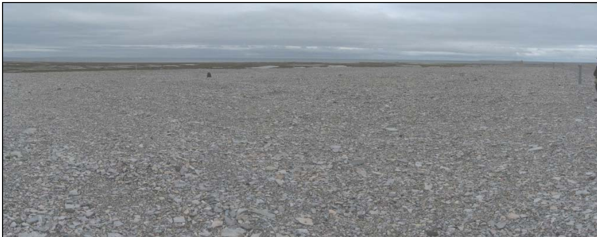
Photograph T2-22. Panoramic, L to R, looking SW from NE corner. VT-6 visible along right side of photo. No clear indications of problematic conditions (i.e., slope movement or significant differential settlement). The irregular surface (poor construction finish) masks minor changes. Condition of the landfill cover should continue to be monitored. ↑
