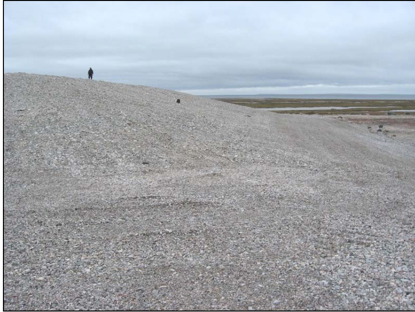
Photograph T2-7 Looking S along downstream toe of W slope from about 20m N of NW toe. Broad zones of depression are visible which is consistent with poor construction finish. There is no evidence of slope instability. ↑
