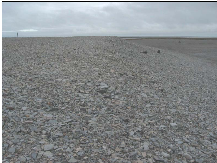
Photograph T2-20. Looking N along E crest from about SE corner. Significant vehicle ruts and inconsistent construction finish in the area. Slope appears stable and the surface irregularities are self armoured and not susceptible to further erosion. ↑
