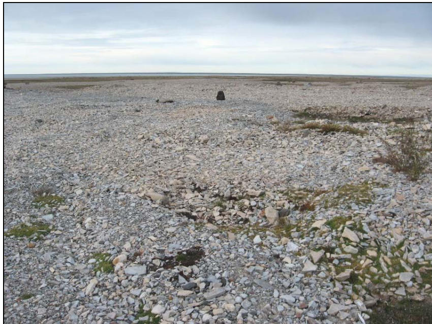
Photograph NWS-14. Looking NE from central east side of the West cell. Gravelly toe getting away from poorly defined crest. Very minimal relief. ↑
