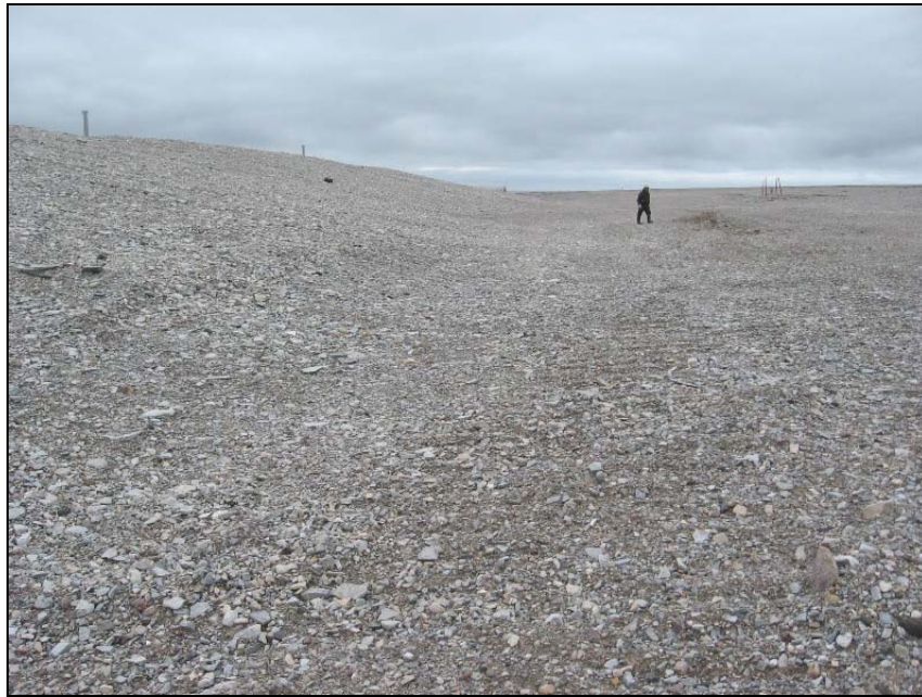
Photograph T2-2. Looking W from NE corner along toe of N slope. Condition of slope appears unchanged from previous two inspections (2006 and 2007); however, inconsistent finished grade (undulations and vehicle ruts) makes it difficult to discern differential settlement. ↑
