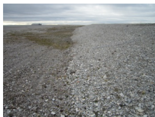
Photo D5 West view of South slope and toe
