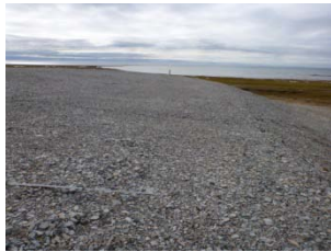
Photo A7 Southwest view of top from north corner
