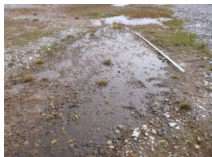
Photo G19 West view of stained area
