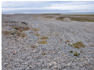
Photo C7 South view of west regraded area
