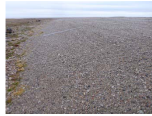
Photo E3 Northeast view of west regraded area from northwest corner
