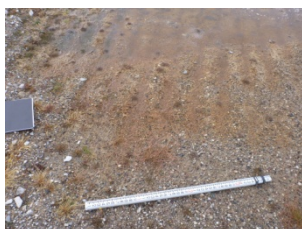
Photo F11 South view of Iron Oxide staining
