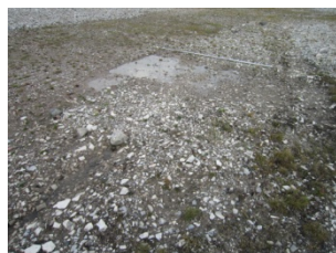
Photo D6 Ponded water looking northeast
