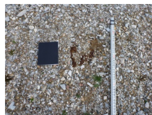
Photo F12 North view of exposed debris on south slope
