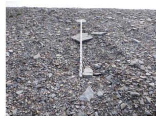
Photo B4 View of erosion feature D near northwest corner
