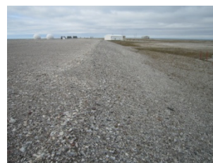
Photo D3 North view of east slope
