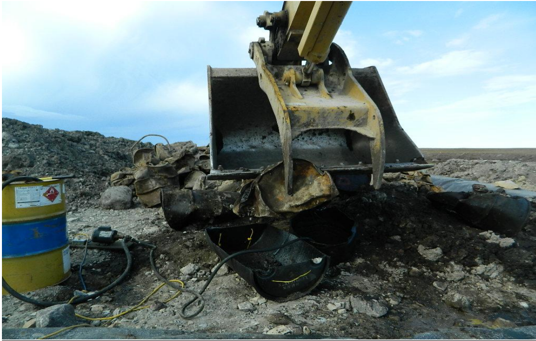
Photo #47: Removing free product from excavated barrels. Free product was captured and placed into new barrels for off-site removal.
