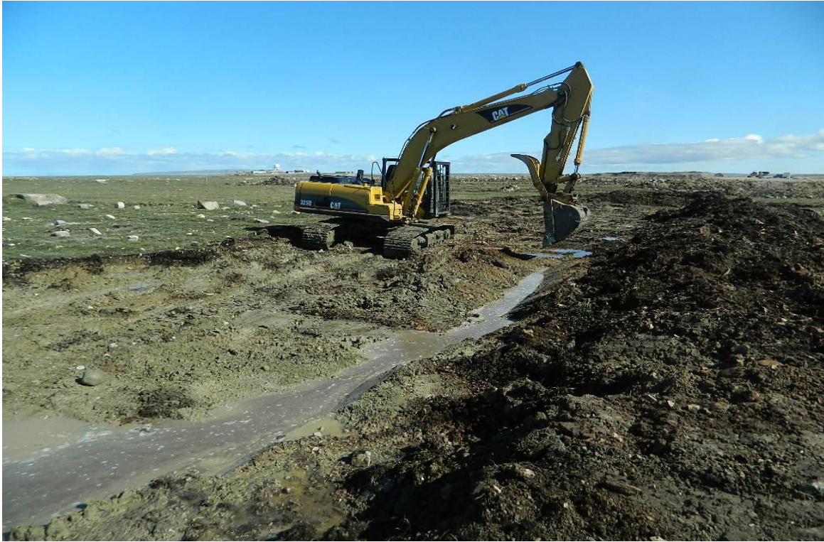
Photo #5: View looking northeast of excavator digging trench for water drainage of FTA LTU.
