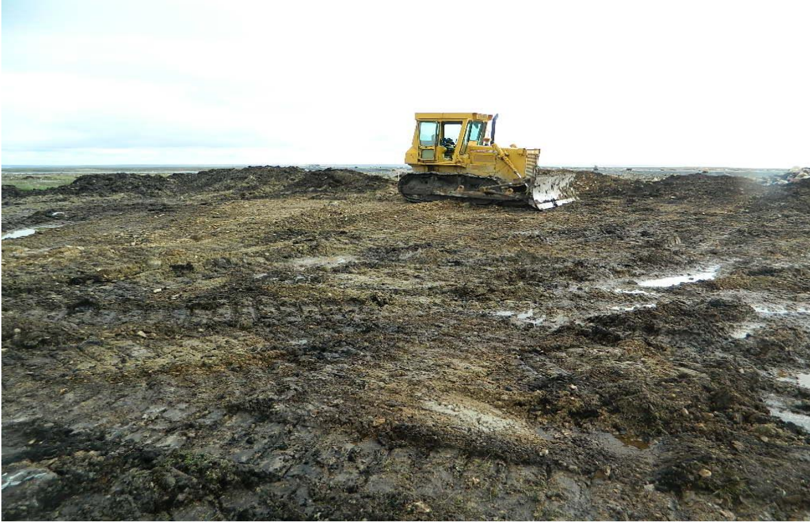
Photo #9: View looking southwest at FTA LTU after some success with bulldozer in grubbing soils. A small portion of the total LTU area was found to contain less clays and more silty gravels.
