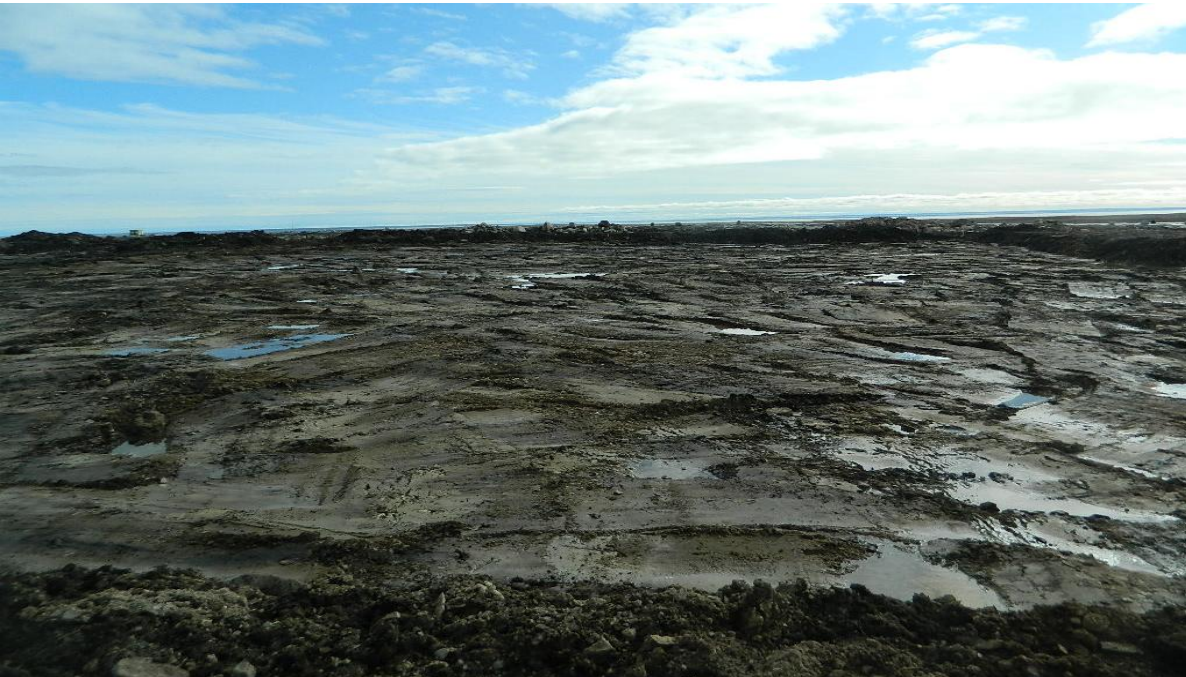
Photo #14: View looking south after flattening LTU base with wide track bulldozer.
