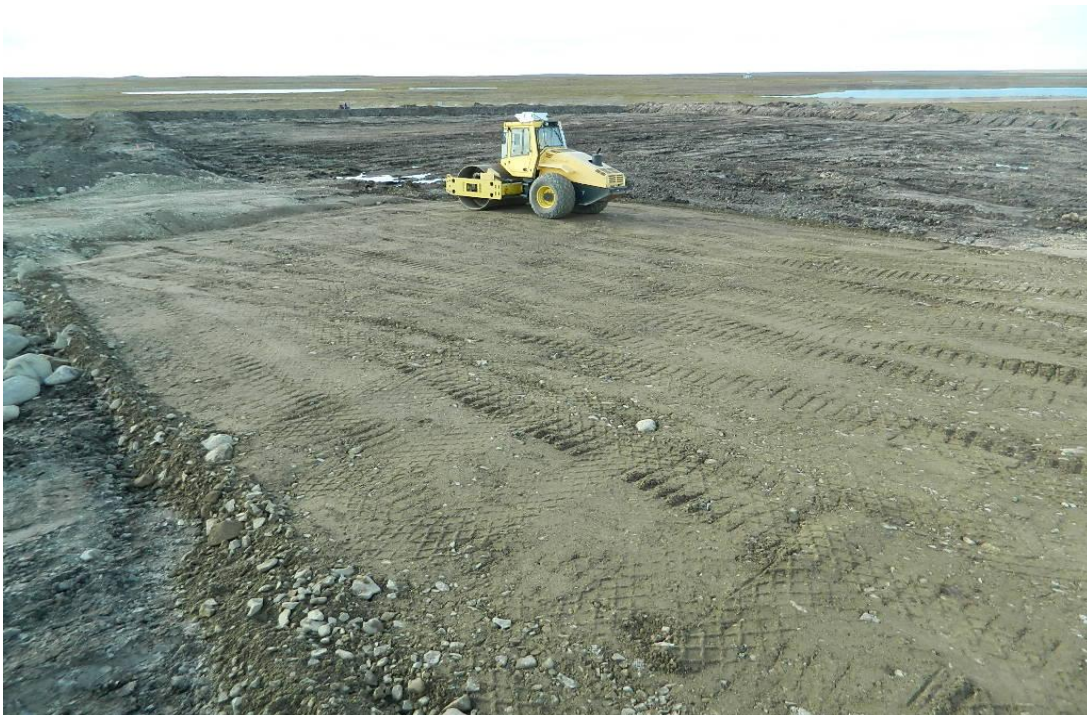
Photo #43: View looking north at the backfilling and compacting of barrel cache excavation.
