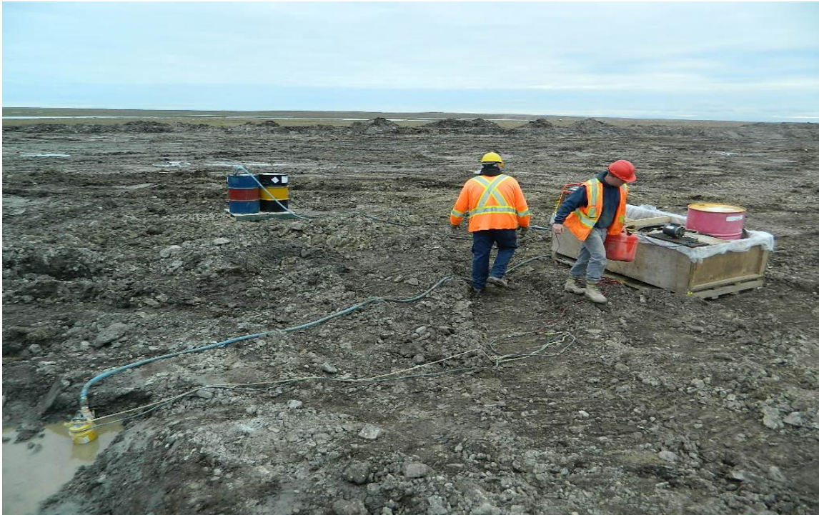
Photo #33: View looking north as impacted water is pumped out of barrel cache pits and stored in barrels.
