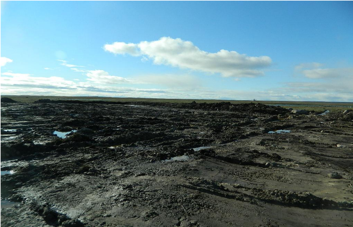
Photo #15: View looking north, material bailed out of LTU footprint and placed for outer berm construction.
