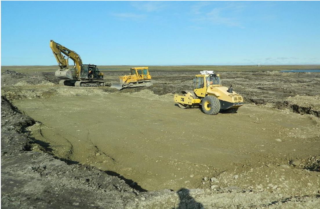
Photo #43: View looking north at the backfilling and compacting of barrel cache excavation.
