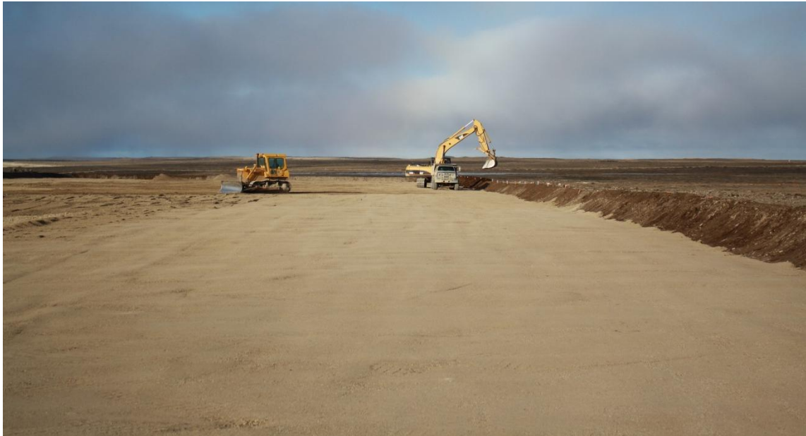
Photo #67: View looking west, preparing demarcation layer.
