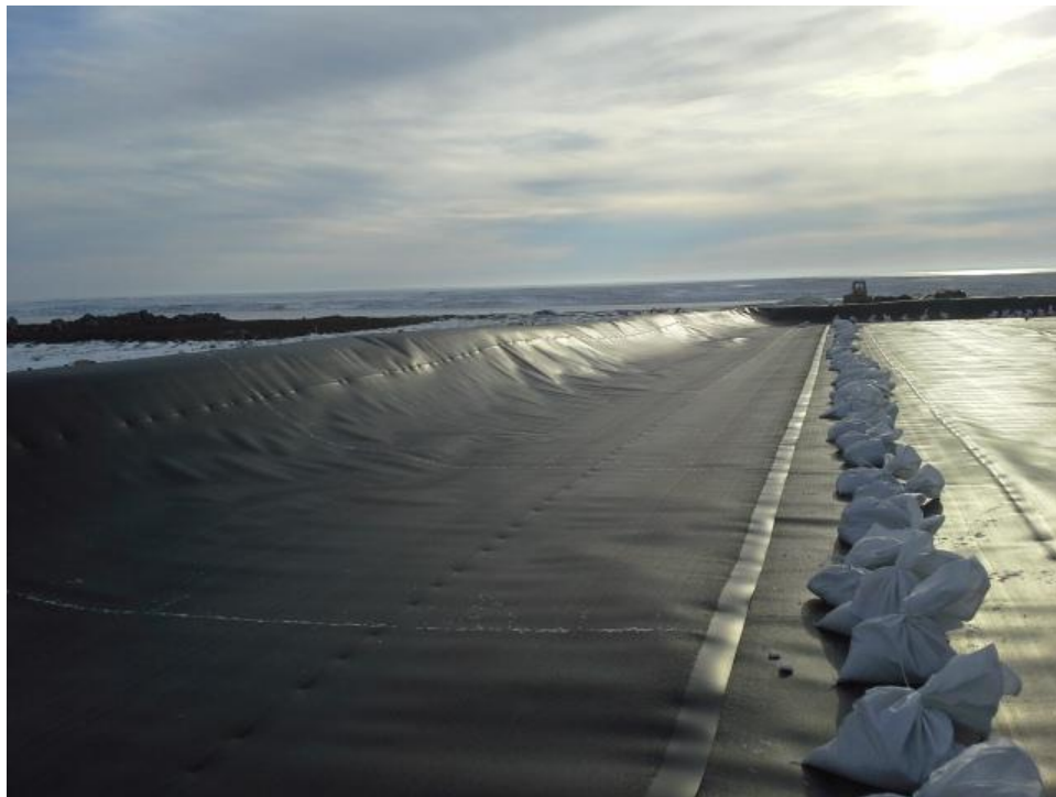
Photo #76: Looking east along northern berm, liner installation.
