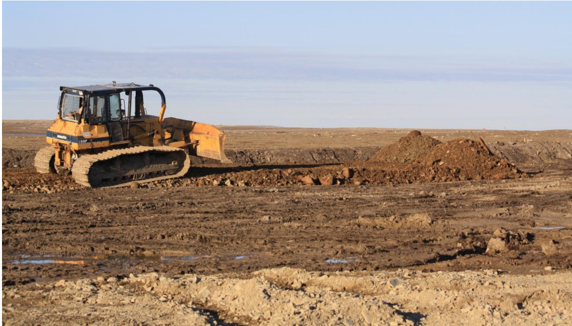
Photo #51: View looking east FTA LTU construction, ballast layer.
