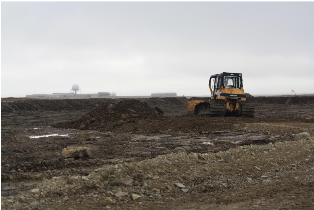
Photo #50: Looking northwest FTA constuction, ballast layer.
