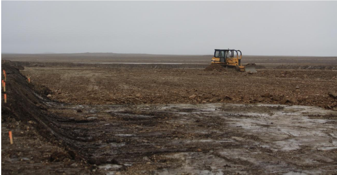
Photo #53: View looking east FTA LTU construction, ballast layer.
