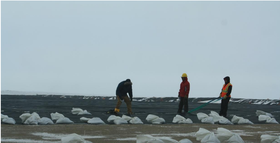
Photo #75: Looking northwest, liner installation.
