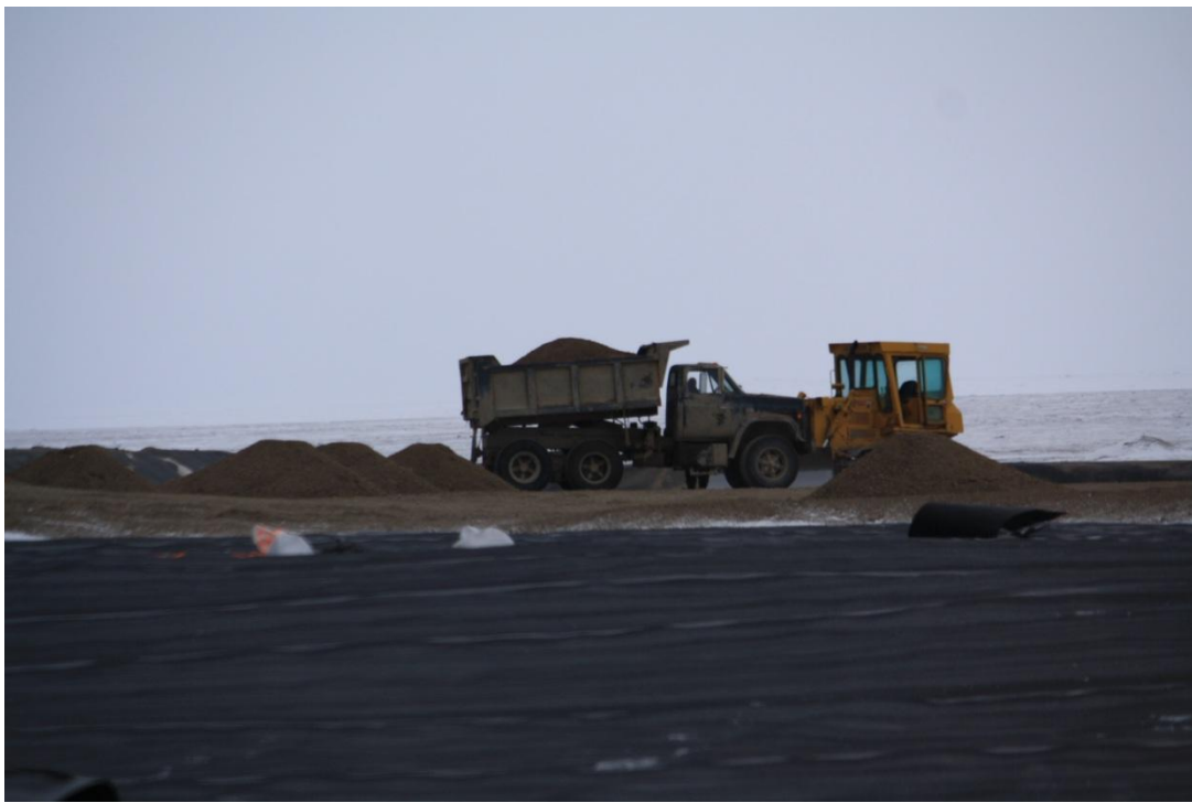
Photo #74: Looking east, spreading demarcation material.
