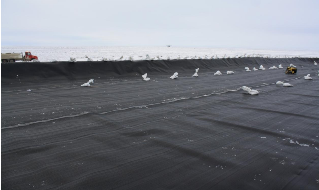
Photo #69: View looking northwest liner installation.
