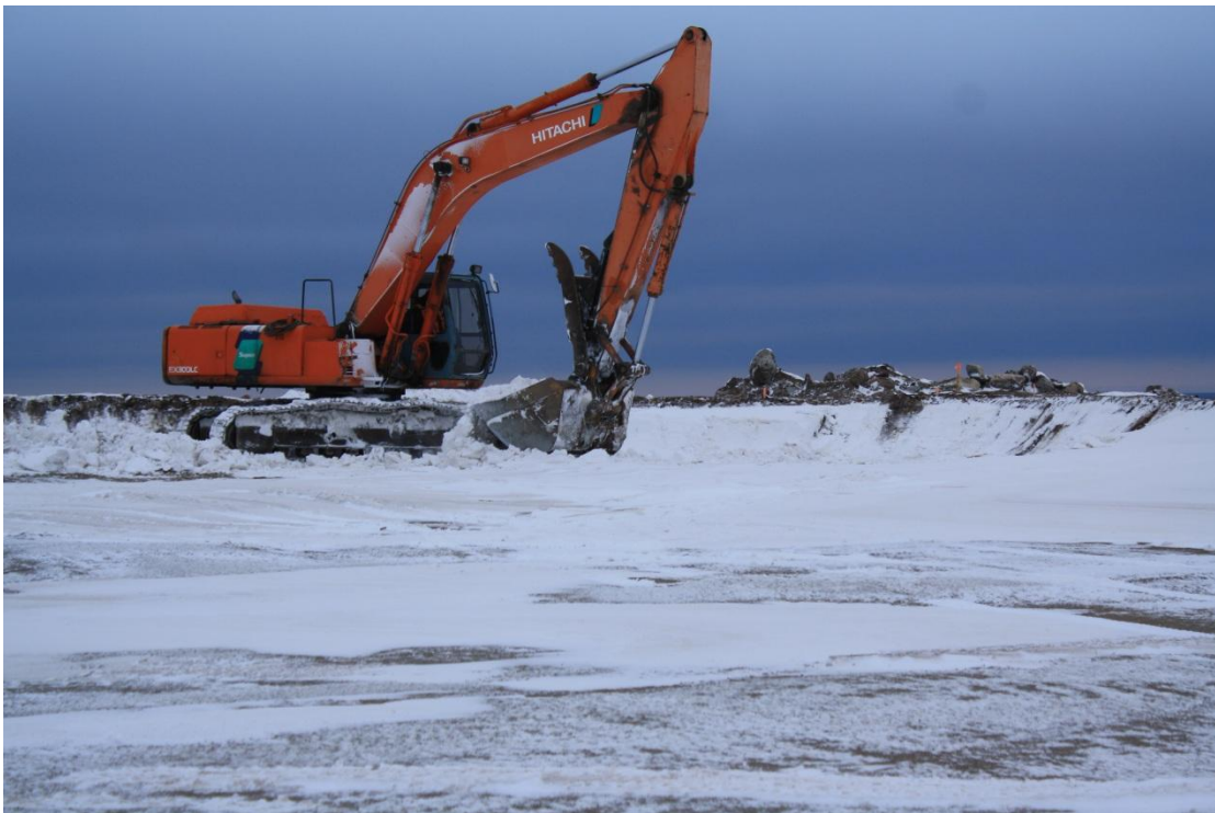
Photo #68: Looking northwest, removing snow in preparation for liner installation.
