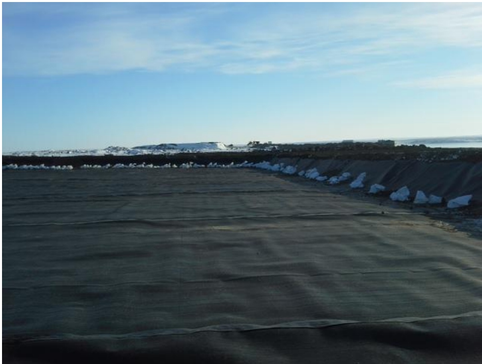
Photo #78: Looking east, uncovered liner to be address in 2015.
