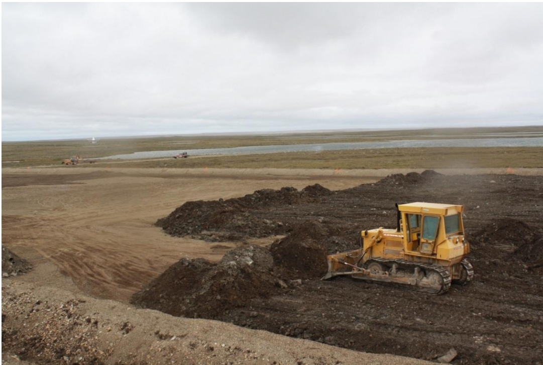
Photo #26: View looking north east, spreading impacted soil in the FTA LTU.
