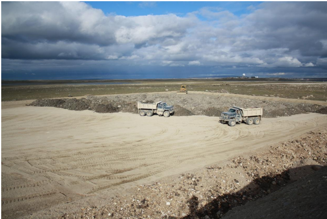
Photo #22: View looking north east, spreading impacted soil in the FTA LTU.
