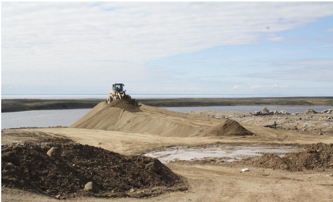
Photo #8: View looking south, importing demarcation material/crush.
