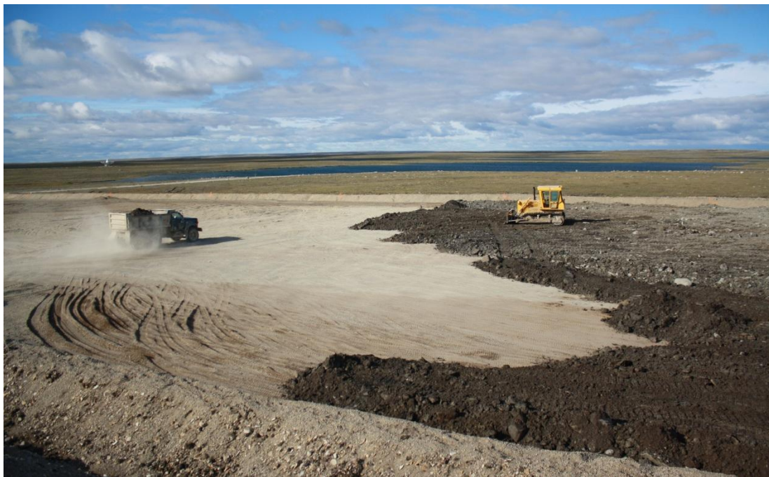
Photo #24: View looking north east, spreading impacted soil in the FTA LTU.
