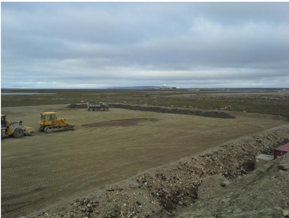
Photo #20: View looking north east, spreading impacted soil in the FTA LTU.
