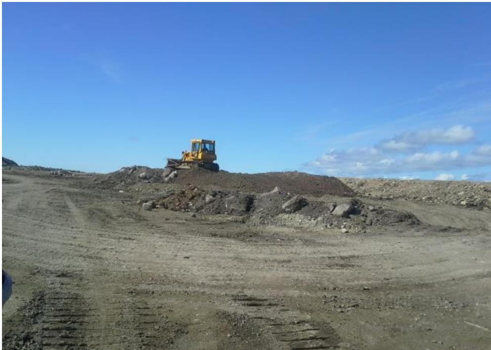
Photo #2: View looking north, importing backfill for FTA excavation.
