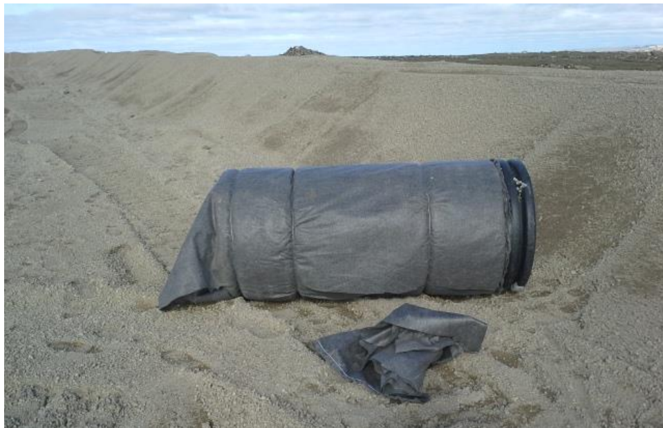
Photo #14: Looking at the south eastern sump prior to installation.
