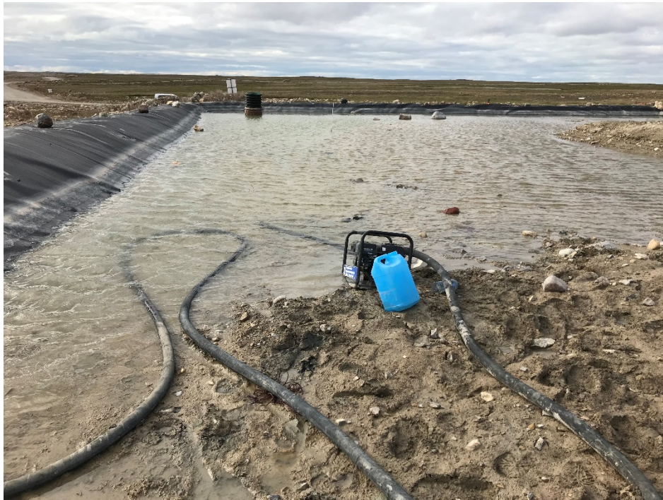
Photograph 3: West view of Apron LTU sump during initiation of de-watering, August 15, 2018.
