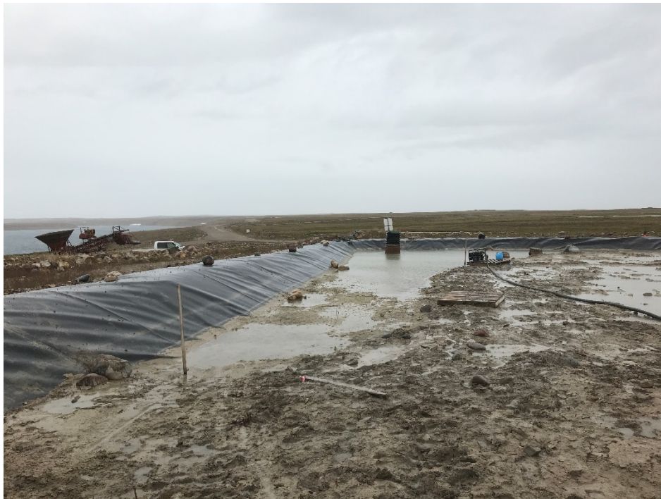
Photograph 4: West view of Apron LTU sump during de-watering, August 16, 2018
