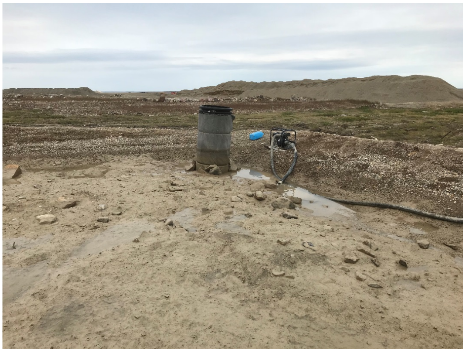
Photograph 8: Southeast view of FTA southeast sump after dewatering, August 18, 2018.
