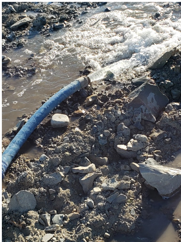
Photo 1 – Hose discharging water from Apron LTU sump onto LTU
