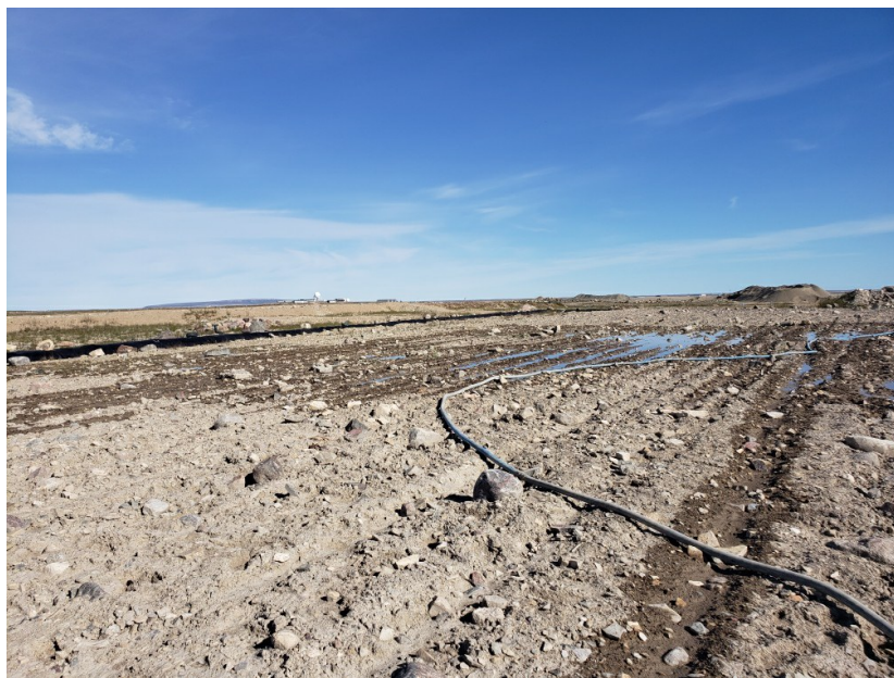
Photo 3 -Apron LTU sump facing NE during dewatering showing good absorption and dispersion of discharged sump water
