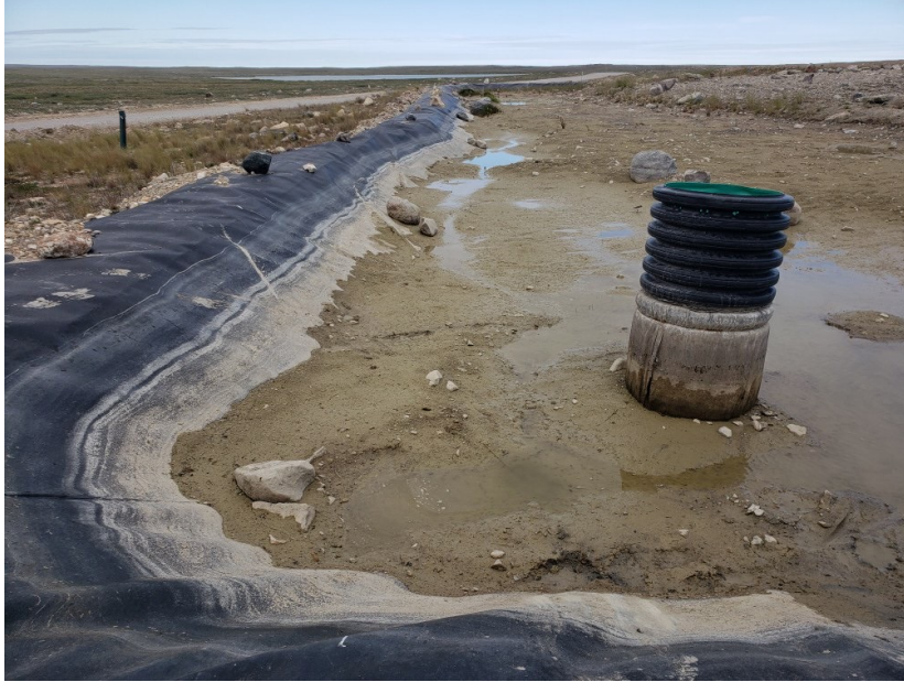
Photo 2 – Apron LTU sump facing north after second dewatering event completed
