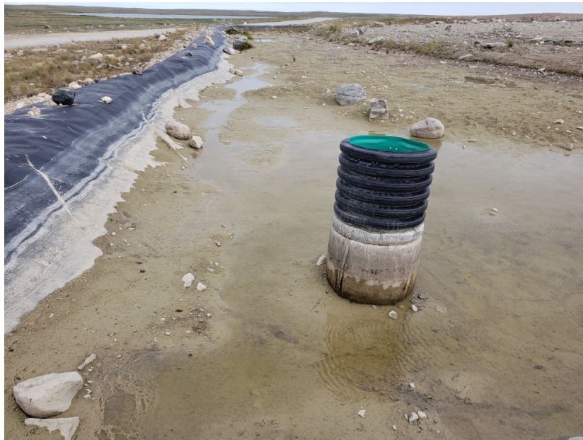
Photo 1 – Apron LTU sump facing north one day after dewatering
