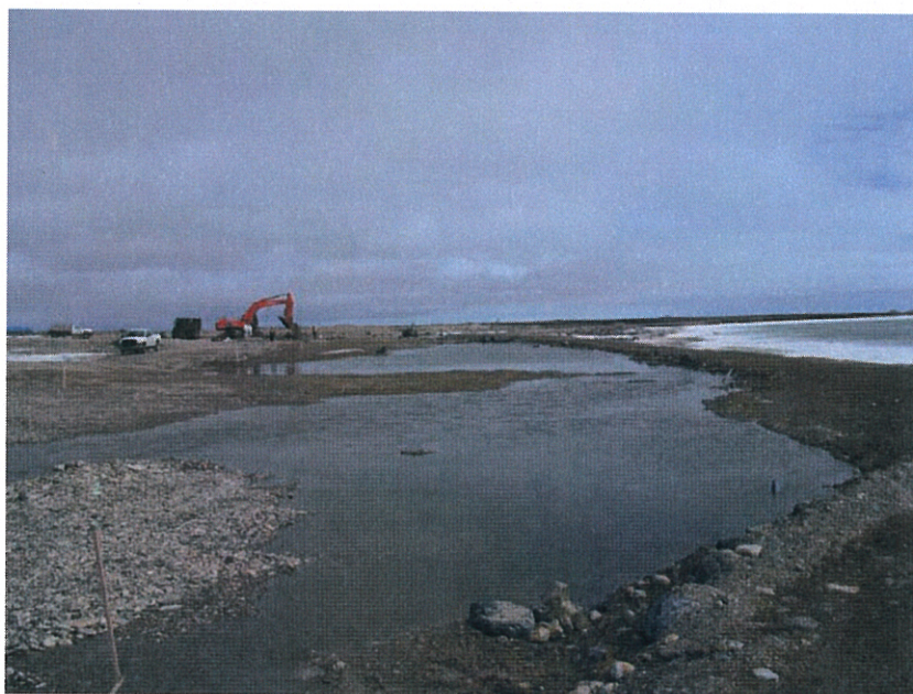
Photograph 1: Excavation work at the Airstrip Landfill. Note the water ponded in the excavation behind the berm and the proximity of the excavation to the ocean. Photograph taken June 27, facing east.
