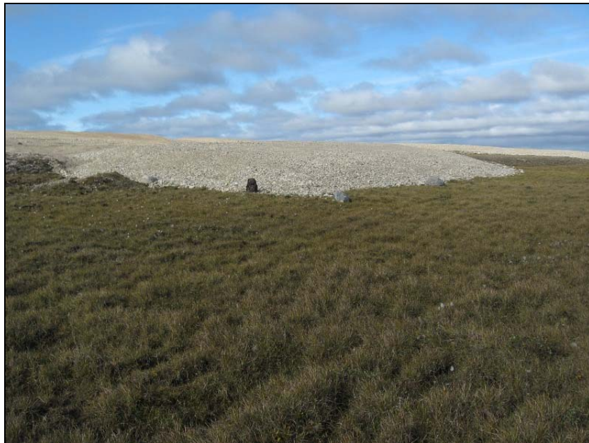
Photograph WLFN-14. Looking WNW to SE corner of small E cell. Granular cover appears stable. No features of note. ↑
