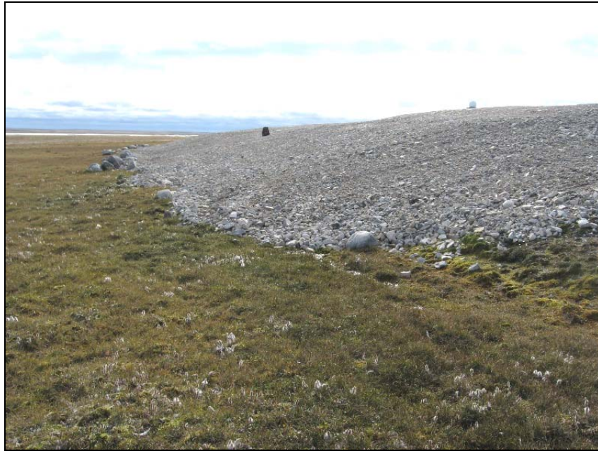
Photograph WLFN-7. Looking SE along N toe of the large central cell from NW corner. Granular cover and toe area appear stable. No problematic conditions observed. ↑
