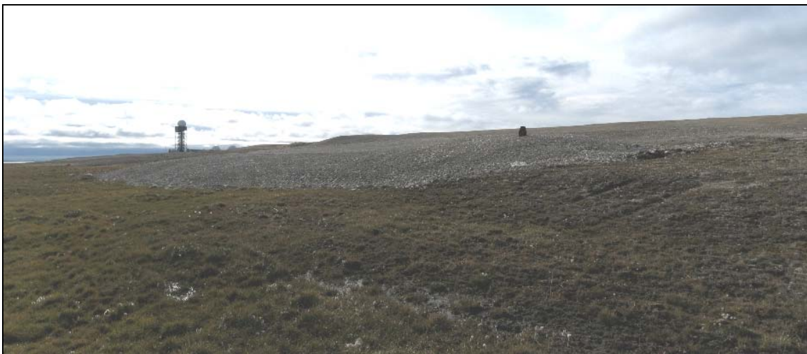
Photograph WLFN-12. Looking S to small eastern cell. Granular cover appears stable. Smallest SE cell visible in background. ↑
