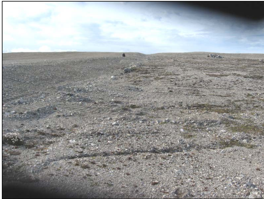
Photograph WLFN-6. Looking SSW along the W side of the large central landfill cell. Granular cover appears stable. 3rd cell is visible at the right side of the frame. ↑
