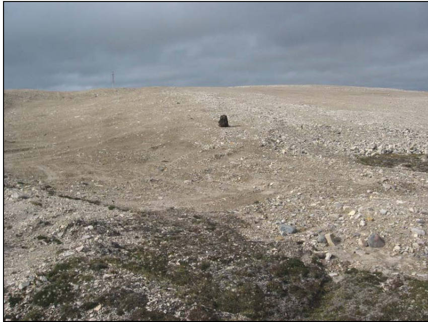
Photograph WLFS-13. Looking W to SE corner of large southern landfill cell. Drainage swale is visible, however it does not appear to be protected by erosion protection. ↑
