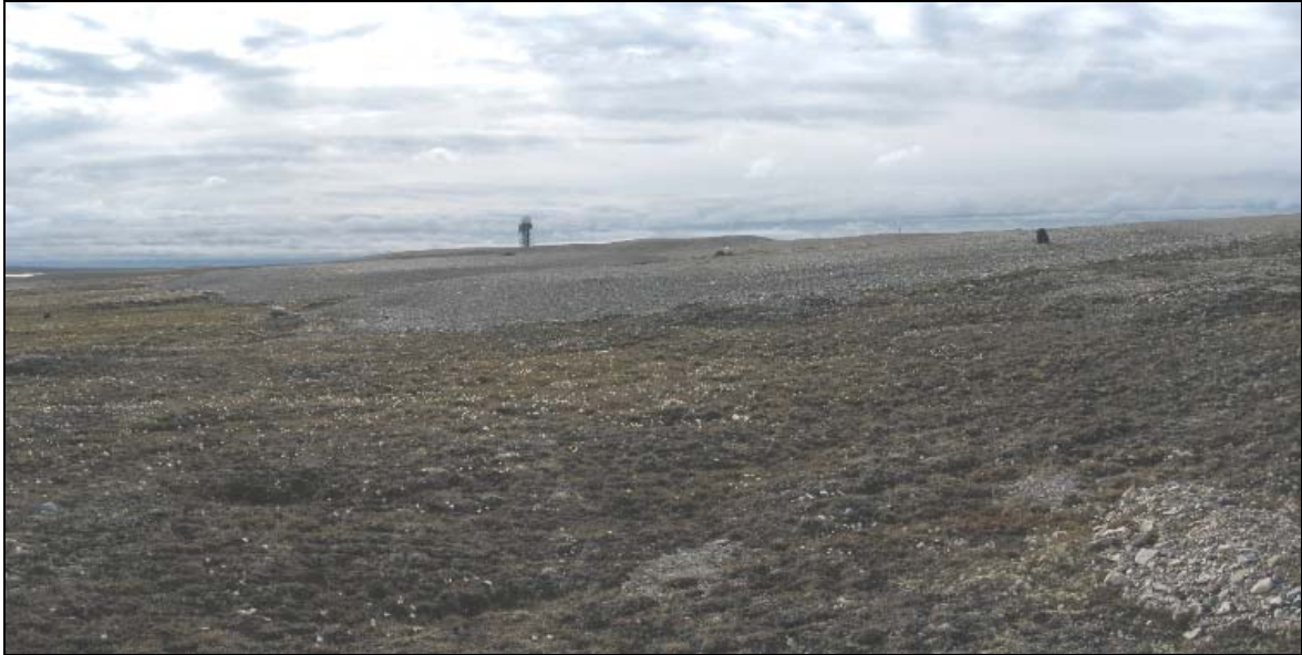
Photograph WLFN-1. Looking SW to NE corner of northern most landfill cell. Granular cover appears stable. No features of note. ↑
