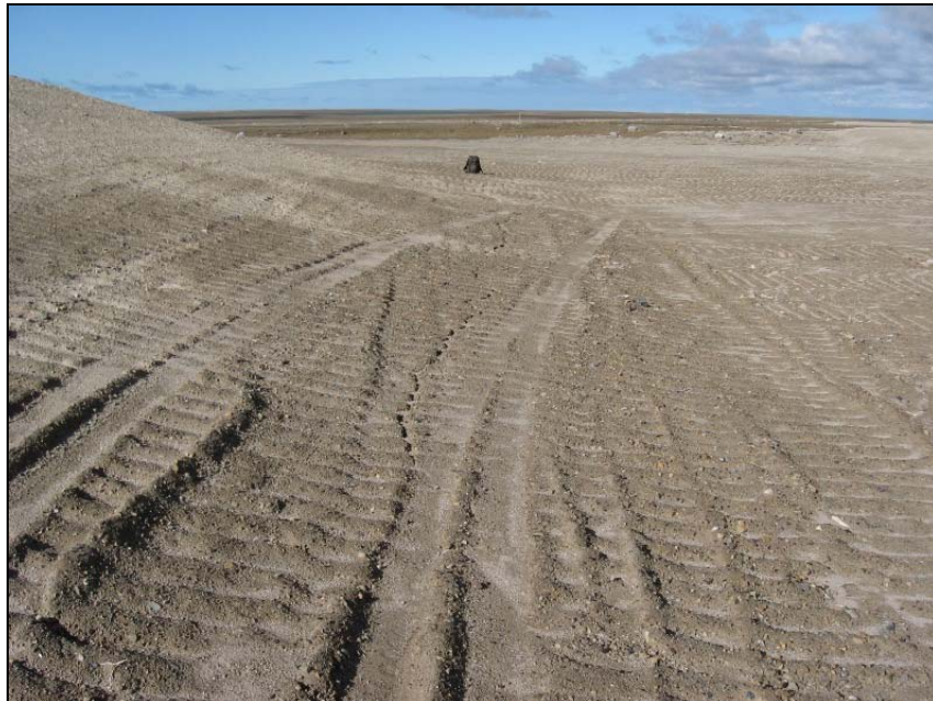
Photograph T2-24. Looking W to NW corner along toe and old eroded tension crack. Heavy rains and wind has essentially in-filled the other cracks that were observed last year. ↑
