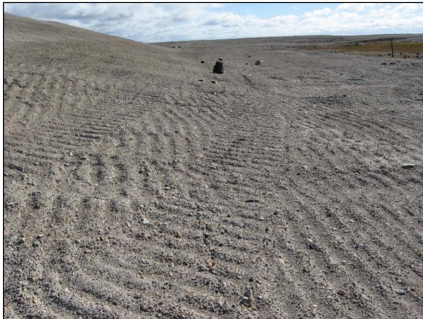
Photograph T2-30. Looking E along toe from SW corner. Old crack runs between gloves and ends at backpack. All other cracks in this area that were observed in 2007 were either completely in-filled or not observed. ↑
