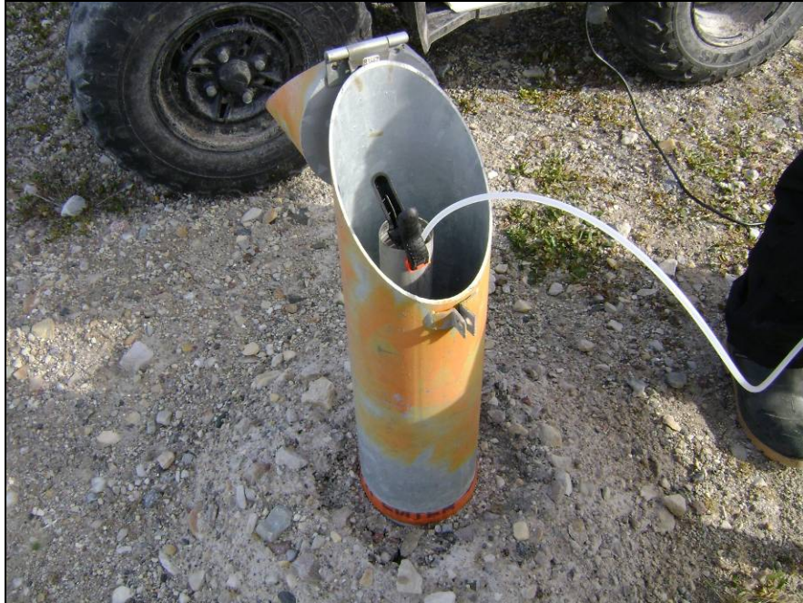
Photograph 1. Monitoring well MW-1. Sample C2-MW-1 collected. ↑
