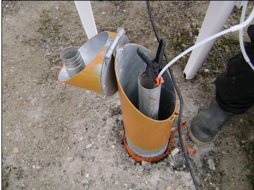
Photograph 5. Monitoring well MW-3. Sample C2-MW-3 collected. ↑
