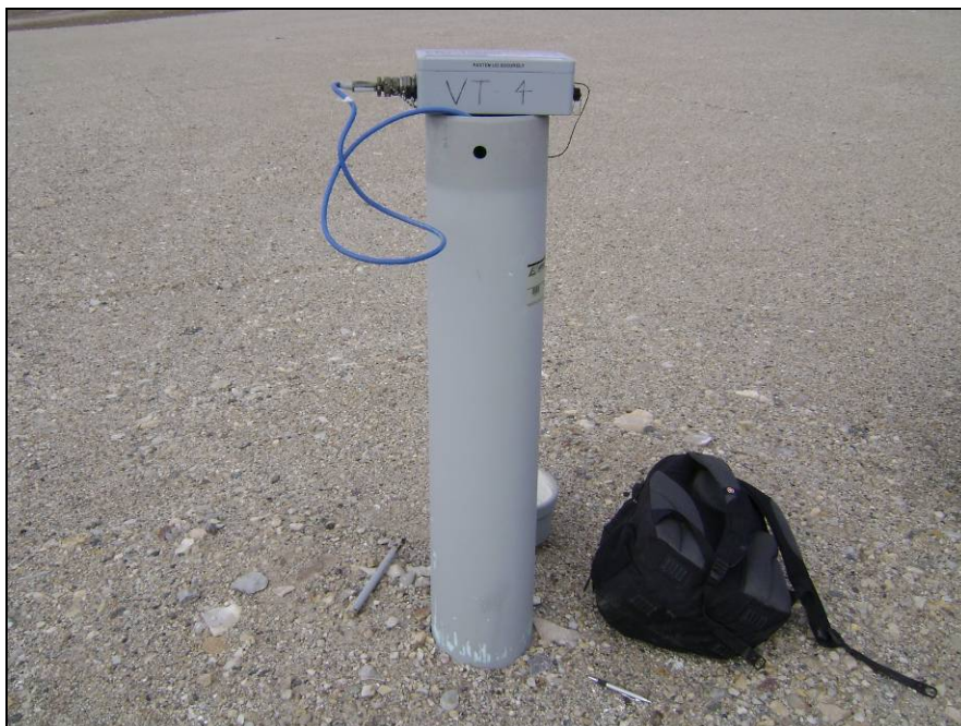
Photograph 12. Vertical thermistor VT-4. ↑
