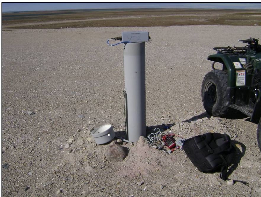
Photograph 10. Vertical thermistor VT-2. ↑
