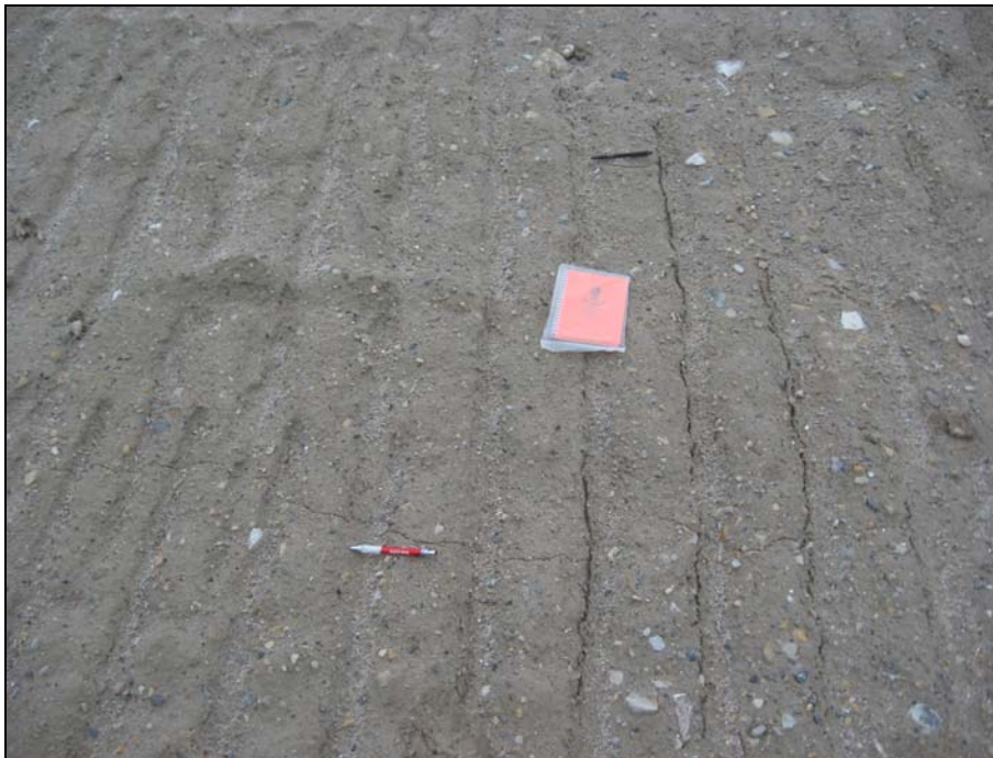
Photograph 24. Area where two parallel cracks (5m and 6m upslope from toe) merge into one. Note additional cracks perpendicular to slope. The cracks that are perpendicular to slope appear to be related to erosion/weathering of fine cover material in dozer tracks. Looking upslope. ↑
