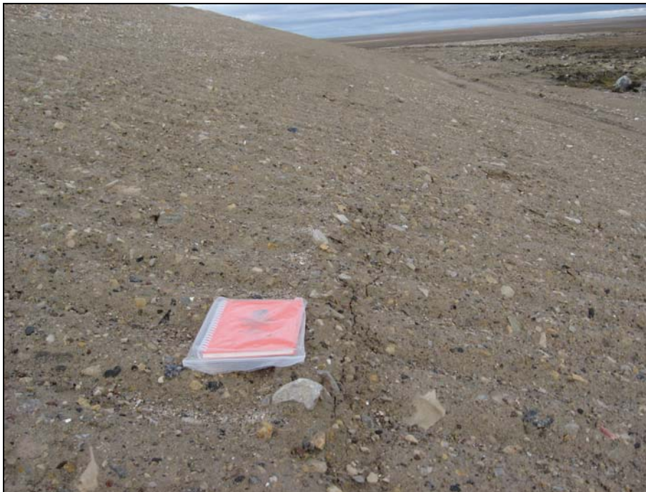
Photograph 22. Tension crack observed mid-slope of the south side of the landfill. Looking E from about 10m east for the SW corner. ↑
