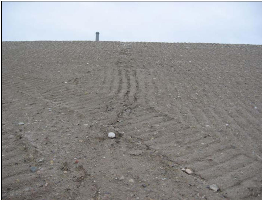
Photograph 32. Minor surface erosion and gulying adjacent to VT-4 downslope to within 4m of toe of slope. Surface runoff appears to have been concentrated in equipment tracks. Granular cover appears to be self-armouring. ↑
