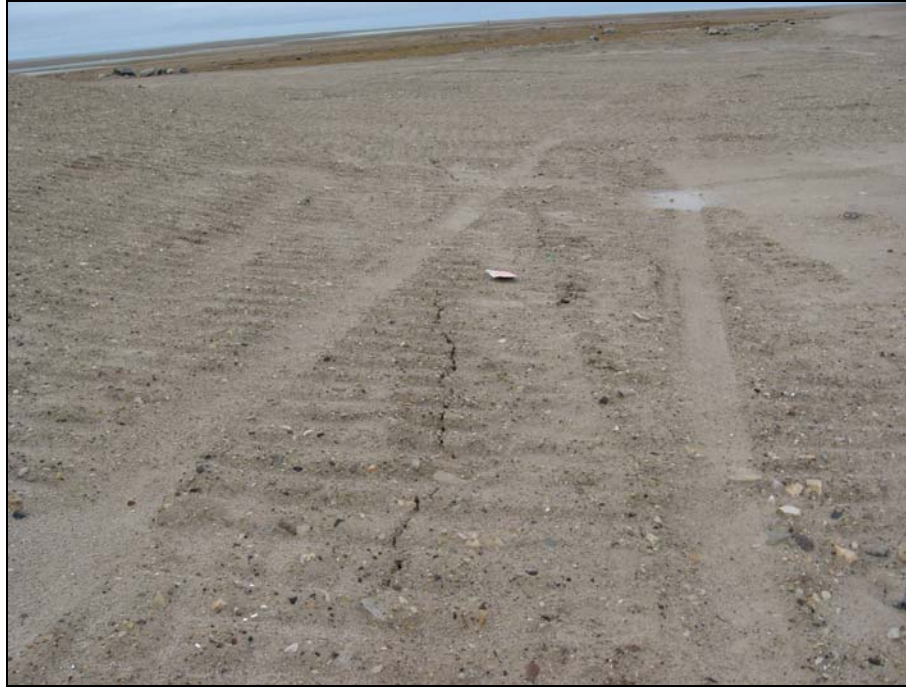
Photograph 13. Looking WNW along toe of slope to larger (up to 2cm wide) tension crack near the NW corner. Additional fine cracks continue 3m upslope. Large crack continues until it is obscured by sediment infilling. ↑
