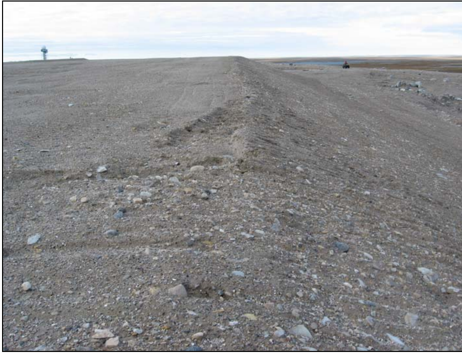
Photograph 29. Looking N along east crest from SE corner. Tension crack along entire crest. ↑
