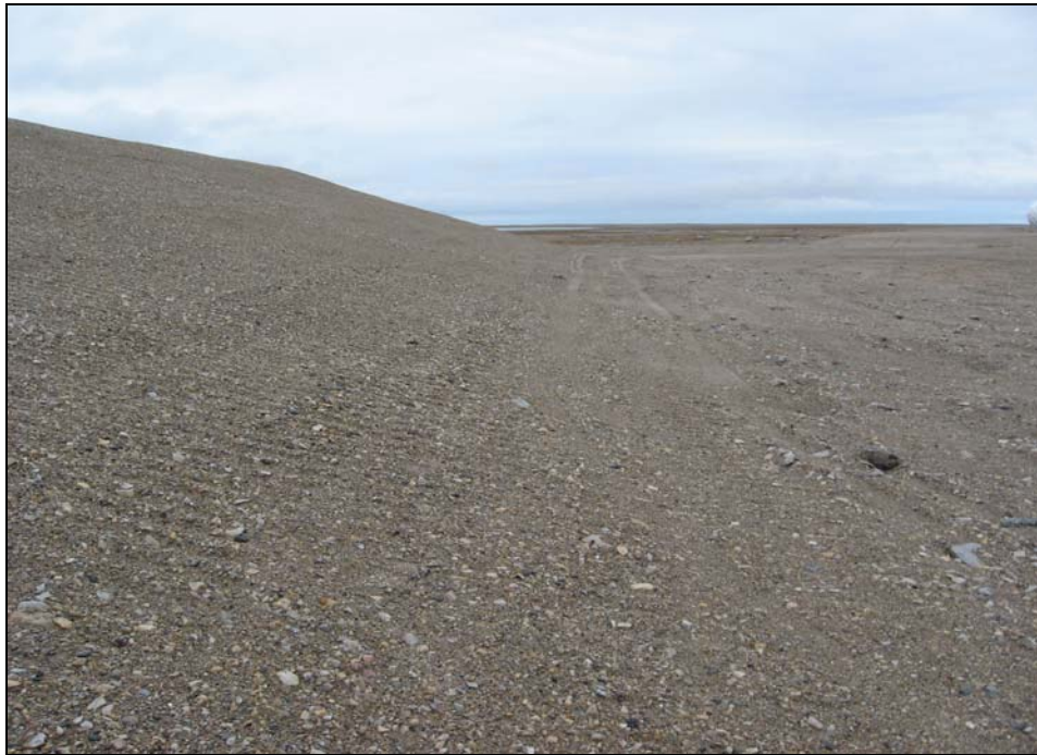
Photograph 2. Looking WNW along northern toe of the landfill from the NE corner . Granular cover has even slope and level construction finish. ↑
