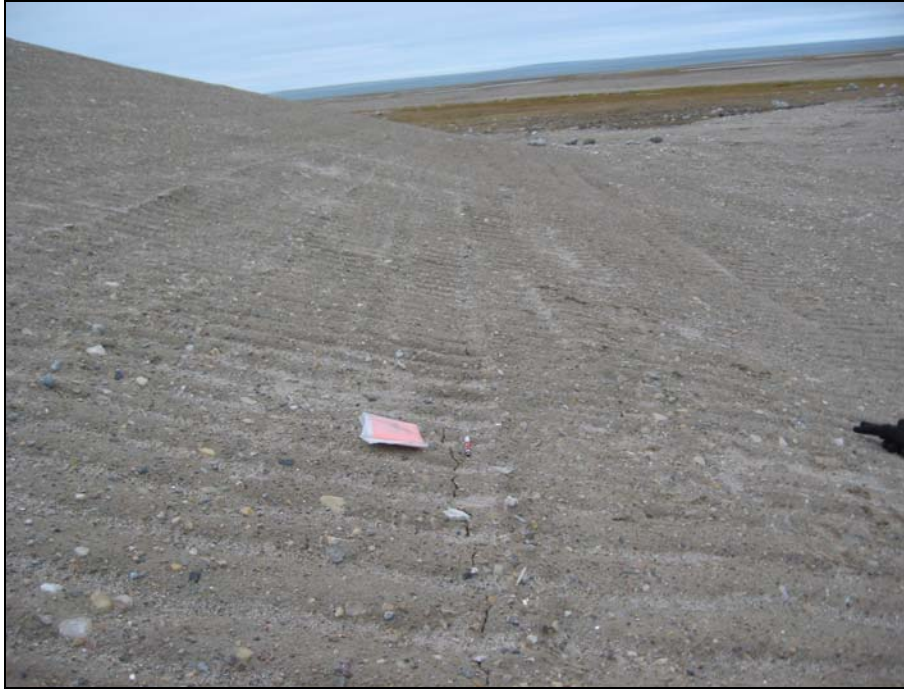
Photograph 25. Typical tension crack looking south along west slope. Fine tension cracks (up to 3 sets) often appear adjacent to and parallel to the larger (e.g. 1 to 2 cm width) cracks . ↑
