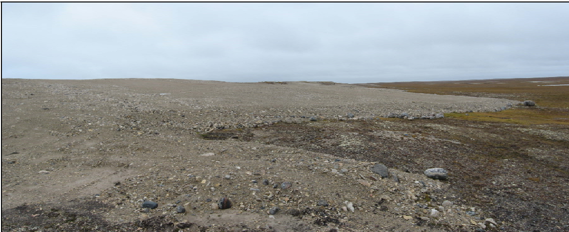
Photograph 8. Looking N to NW towards the south end of the most southerly cell. Granular cover is stable and low profile. ↑
