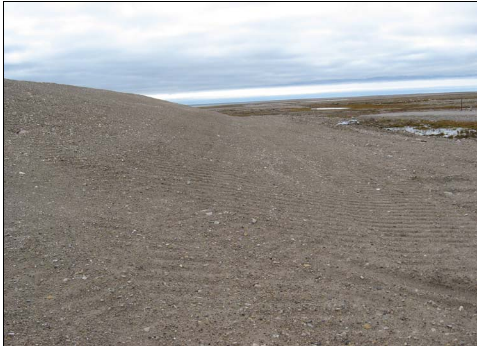
Photograph 2. Looking west along the toe of the north side of the landfill from the NE corner Granular slope is graded uniformly and appears stable. ↑
