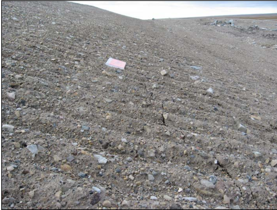
Photograph 35. Tension crack on east slope starting at SE corner and 1/3 up slope (continues from south side). ↑
