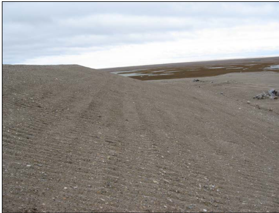
Photograph 34. Looking N from mid-slope east side Tier II . Note minor depression in upslope foreground. There are no indications of recent movement or problematic conditions. ↑
