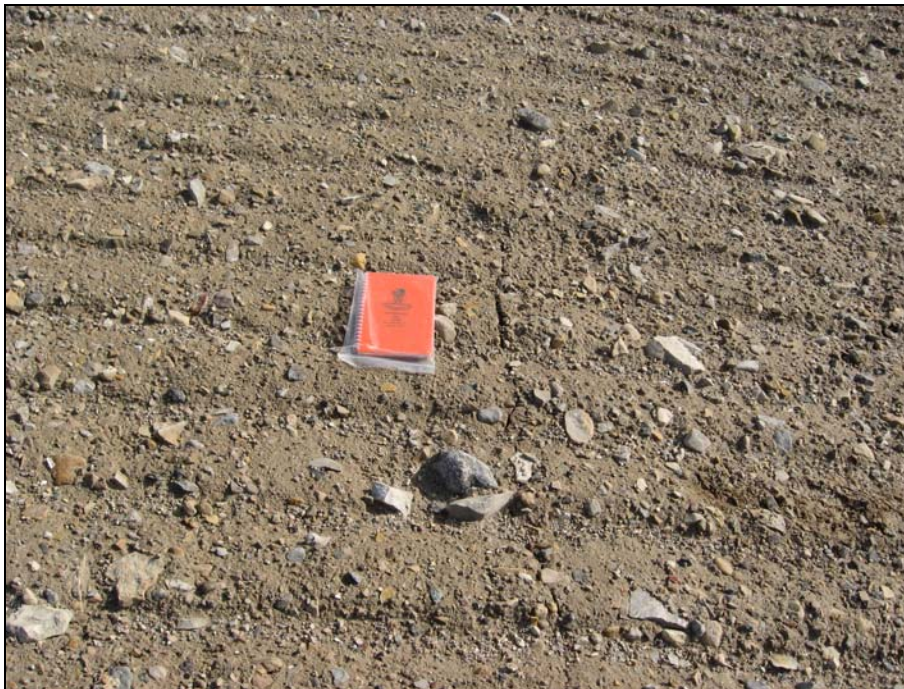
Photograph 16. Tension crack along the upper slope west side looking south (5m from crest). Crack runs parallel to the crest. ↑
