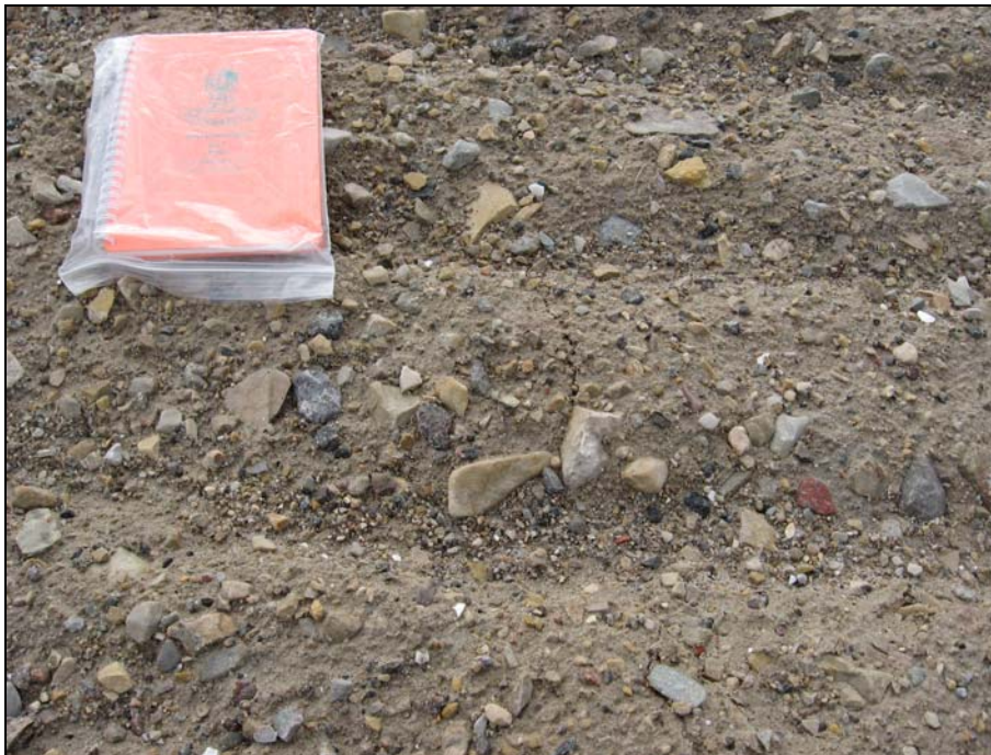
Photograph 8. Tension crack observed midslope on north face about 5m upslope from toe. Field book for scale. ↑
