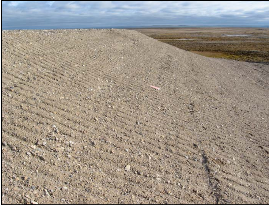
Photograph 17. Following the tension crack noted in Photo 16 to the south. Field book at the end of the visible crack (see Photo 18 for close-up). ↑
