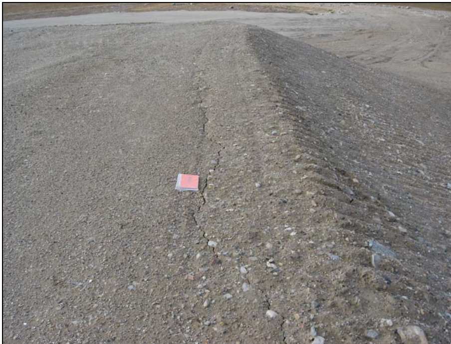
Photograph 32. Single tension crack continues to NE corner along the east crest of the landfill. ↑
