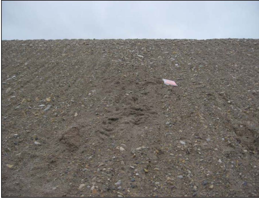
Photograph 27. Minor surface erosion (3m long, 0.7m wide) near crest of west slope about 10m N of the SW corner. Granular cover appears to be self armouring. Excess sand shifted exposing gravel. ↑
