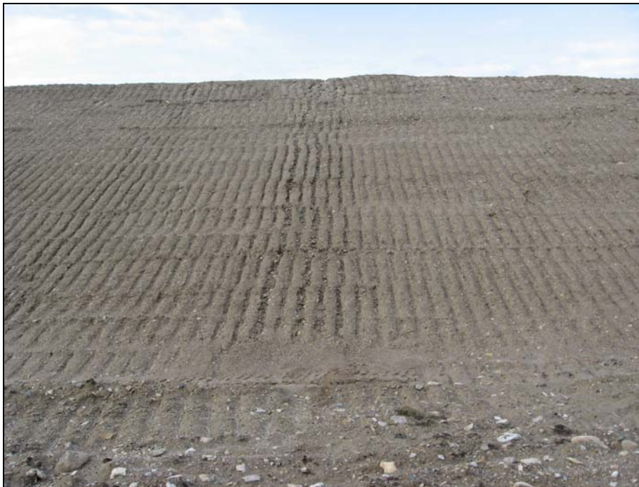
Photograph 28. Minor surficial erosion, self armouring, along east side of south slope looking north from downslope of toe. ↑
