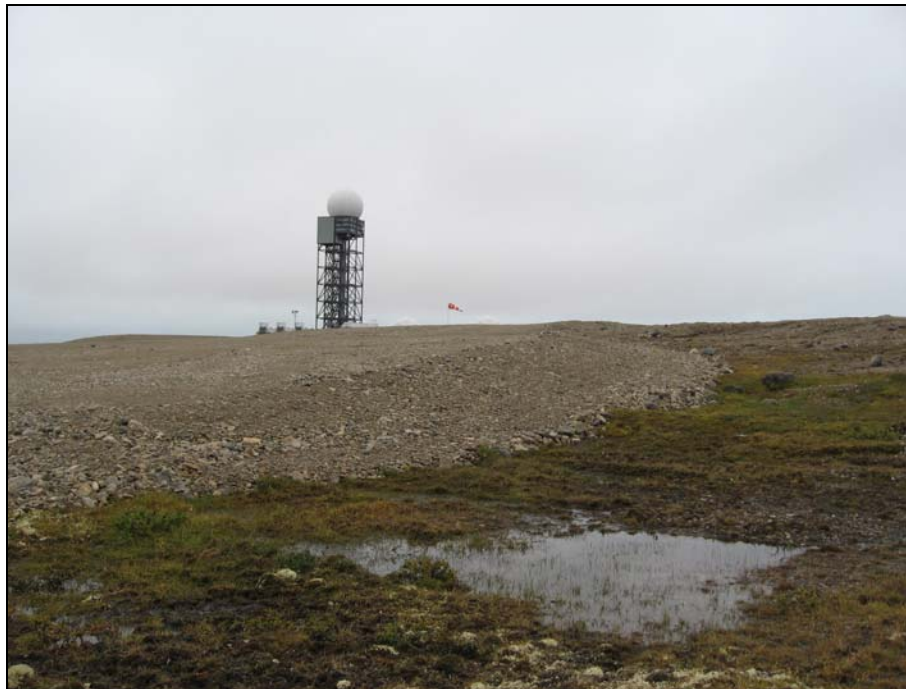
Photograph 6. Looking SSW to the north end of the southern (largest) granular covered cell. Note ponded water. Slope appears stable. ↑
