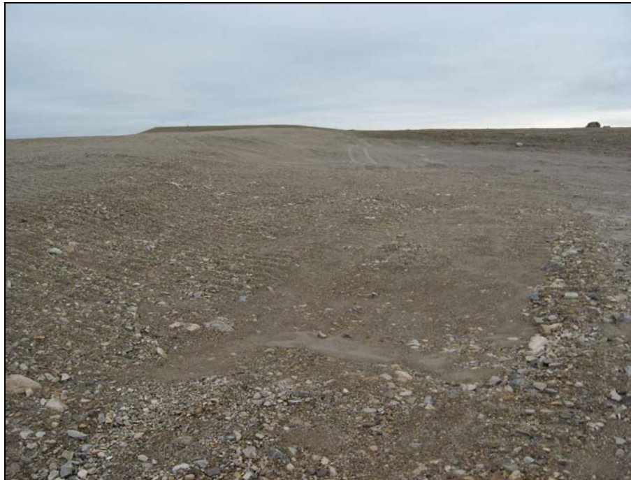
Photograph 8. Station Landfill: Looking S along west side of Station Landfill from the north end of the landfill. The granular cover has minimal slope and appears to be very stable. Tier II LF visible in the background.↑
