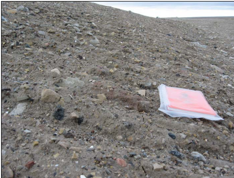
Photograph 38. Tension crack ends mid-slope about 13m south of NE corner. ↑
