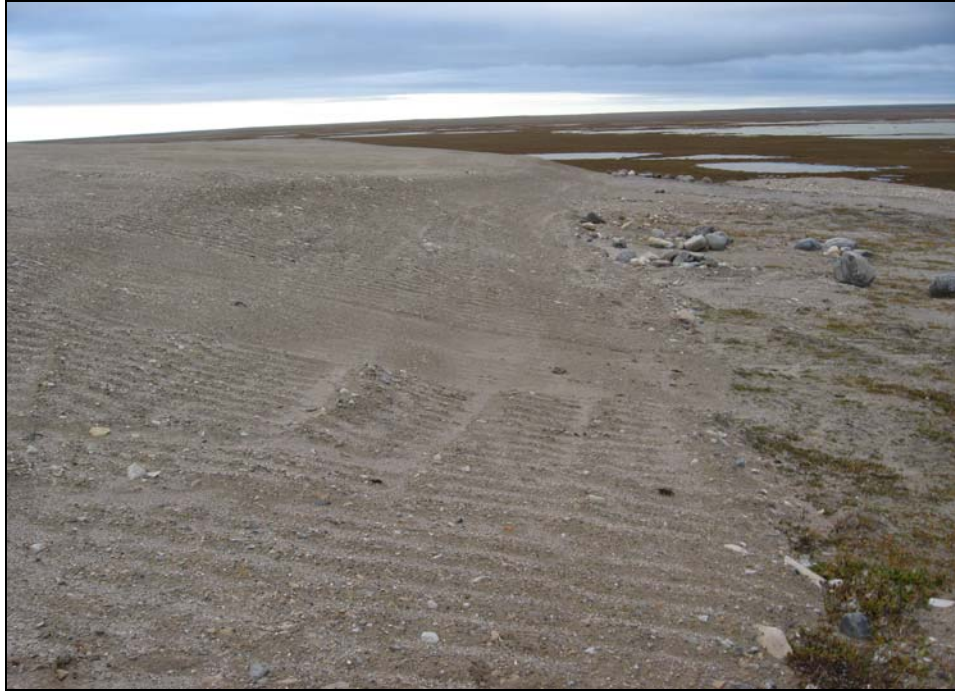
Photograph 1. Station Landfill: Looking north along the east side of the landfill from the SE corner. Slope appears shallow and stable. No features of note. ↑
