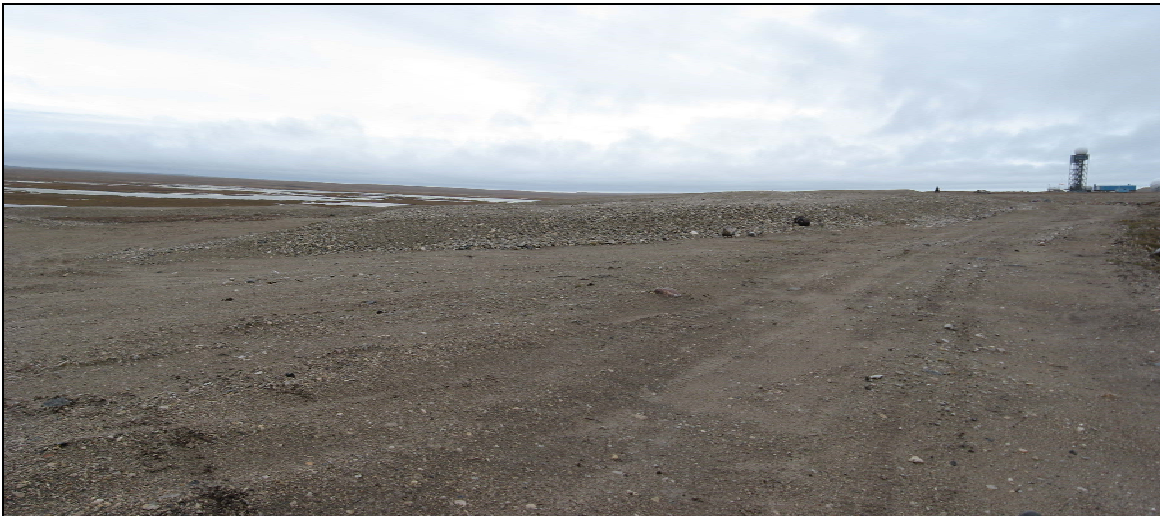
Photograph 2. Looking SE to NW corner of 3rd cell from the north along the west side of the landfill. No features of note. Granular cover appears stable. ↑
