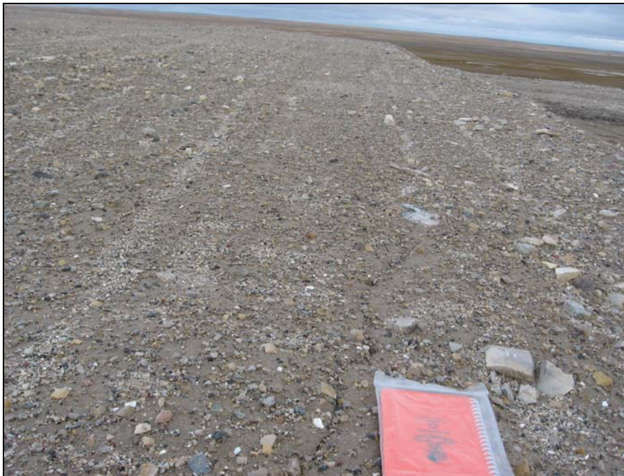
Photograph 26. Tension crack along the crest of the south slope. Looking east to SE corner. The crack is largely infilled with sediments and migrates from 0.5m to 2m in. ↑
