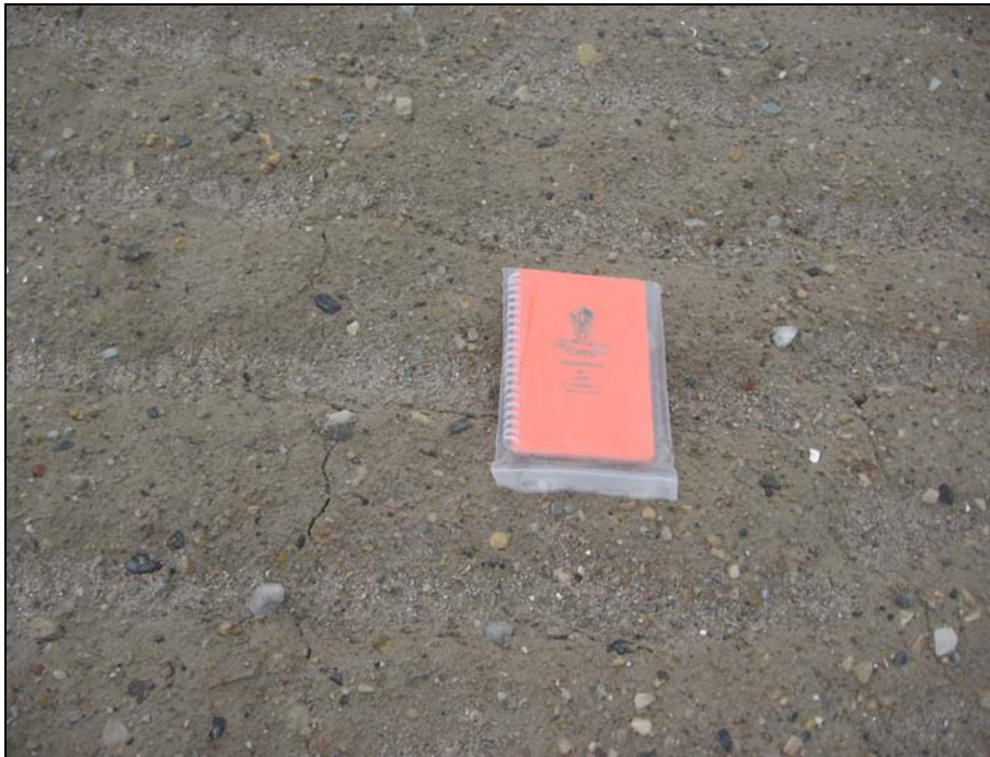
Photograph 26. Following the tension crack along the toe of slope. Moving S, the cracking appears to shift upslope to approx. 7m from toe. Portions obscured by sediment infilling. ↑
