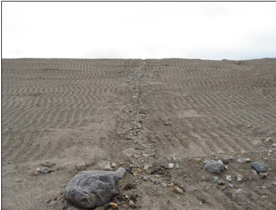
Photograph 4. Station Landfill: Looking upslope (west) to minor surficial slope erosion. The granular cover material appears to be self armoured. ↑
