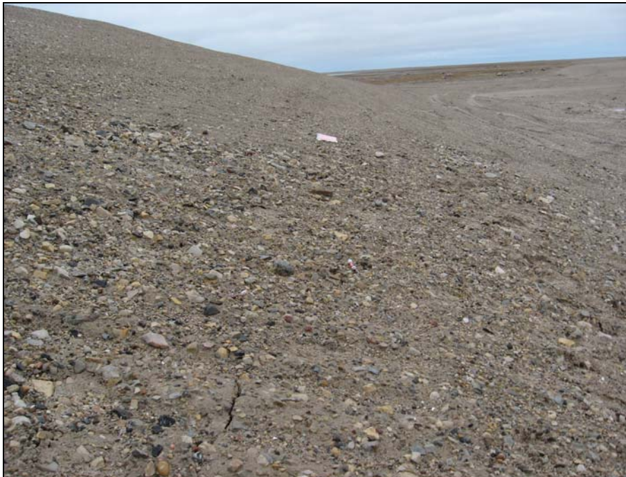
Photograph 10. Continuing to track the lower (most consistent) tension crack along the north toe of the landfill. Looking west along toe of north slope. Field book for scale. ↑
