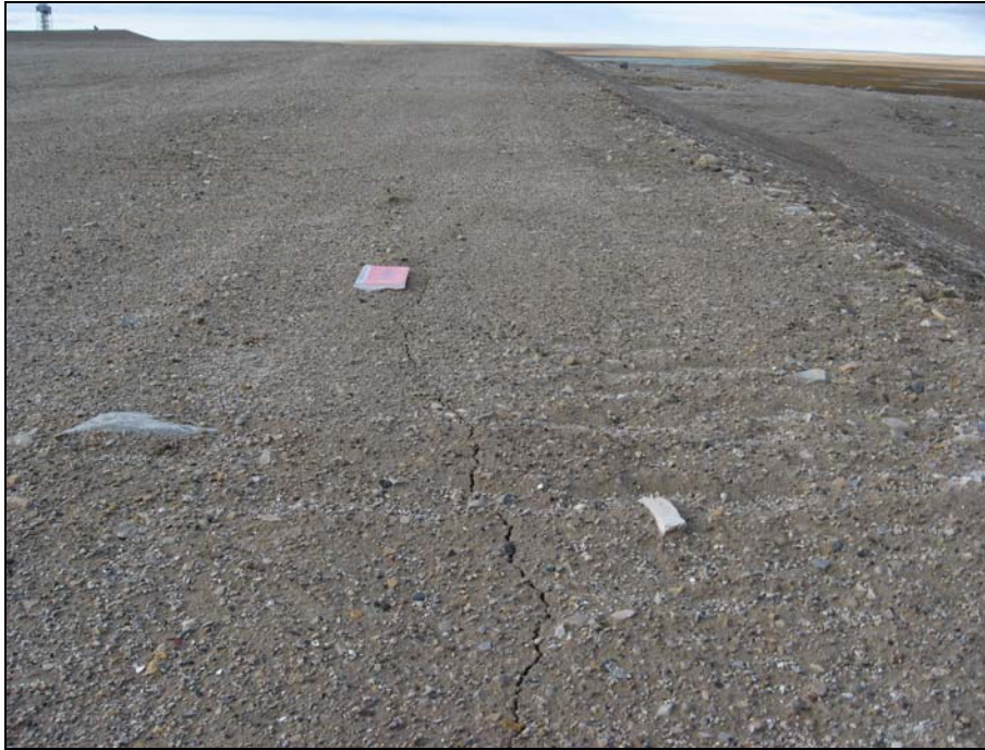
Photograph 31. Following the tension crack north. Crack is essentially continuous from the SE corner and splays and migrates up to 6 m from the crest. ↑
