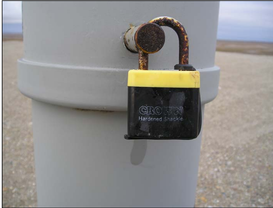
Photograph 5. Example of a typical lock at CAM-2, PIN-3, and CAM-M. Locks are very rusted, and most are difficult to insert key into and turn. ↑
