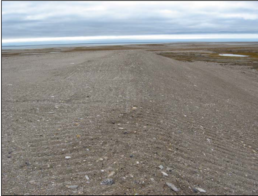
Photograph 3. Looking west along crest from NE corner. Faint tension crack visible along the top of slope. ↑
