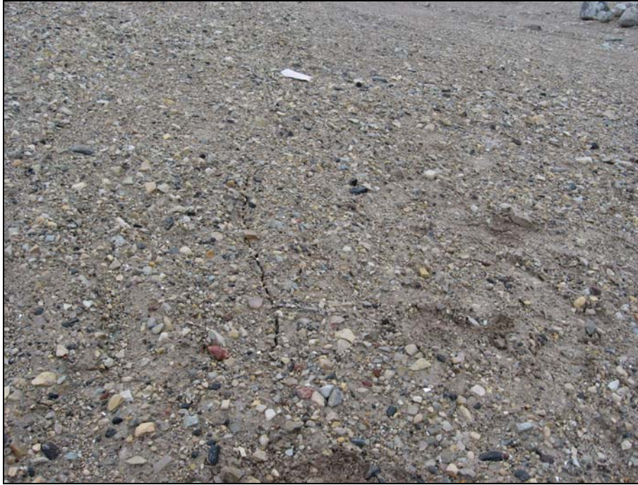
Photograph 7. Tracking the lower (most consistent) tension crack that originated near Photo 4. Looking WNW along the northern toe of the landfill from near the NE corner. ↑
