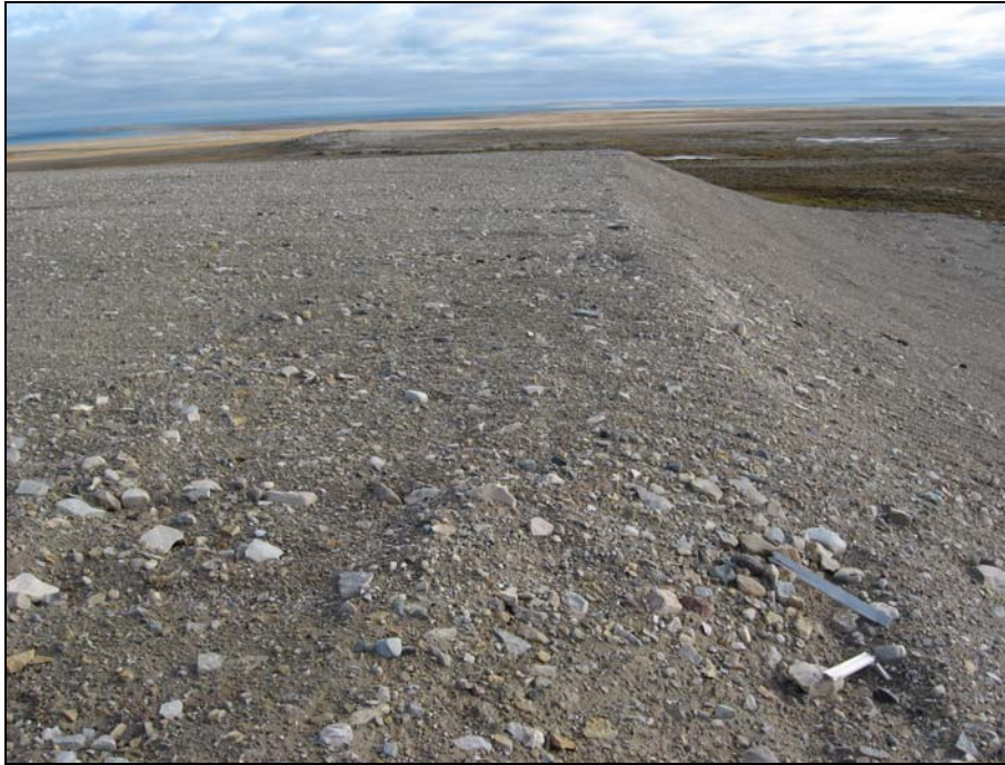
Photograph 19. Looking S from crest at NW corner. No tension cracks observed along top of crest. ↑
