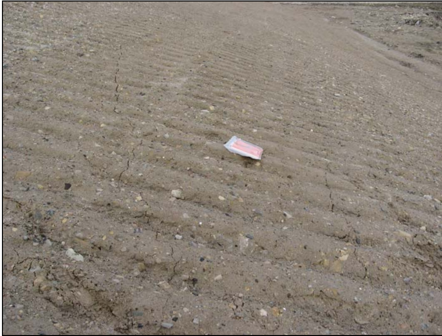
Photograph 23. Tension crack mid-slope on the south slope splays into two cracks with 0.6m to 1.5m roughly parallel spacing. ↑
