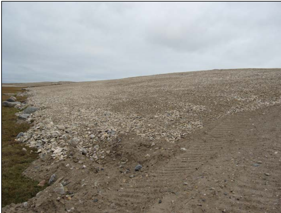
Photograph 6. Station Landfill: Looking SSE along east side of Station LF from near NE corner. Coarse granular cover appears stable and has been contoured to a shallow slope.
