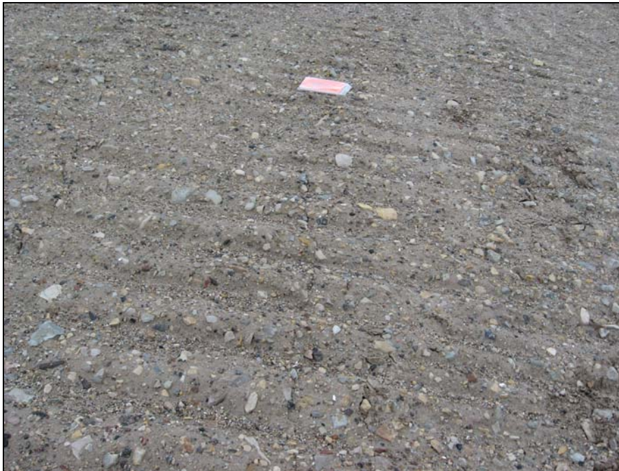
Photograph 4. Close-up of two fine parallel tension cracks that start on NE side of the landfill, about 5m up-slope from toe, and extend essentially all the way to the NW corner. Orange field book for scale. ↑
