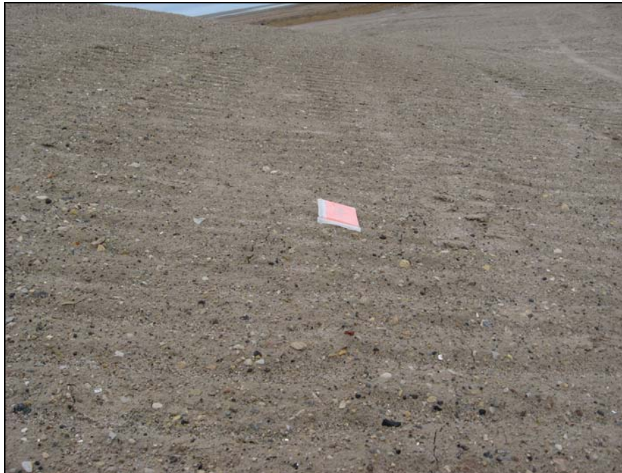
Photograph 12. Tension crack in parallel. Cracks remain fine, but geometry is becoming consistent with slow retrogression. Looking west to NW corner. Hints of tension cracks upslope but sediment infilling prevents clear diagnosis. ↑
