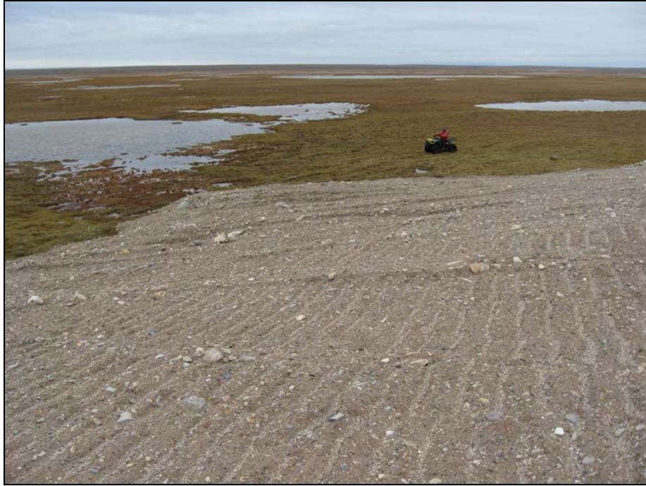
Photograph 7. Station Landfill: Looking ESE from near the northern limit of the landfill. The granular cover has been contoured to a shallow slope. Fine tension cracks and indications of minor movement are visible adjacent to where roughly graded granular fill abuts the organics (beyond the limit of the landfill). ↑
