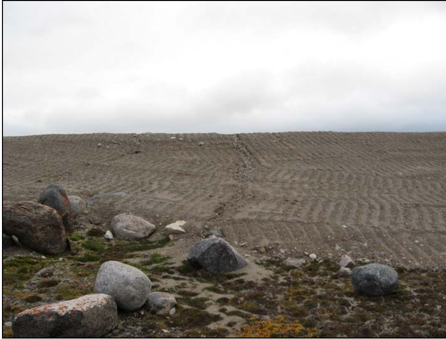
Photograph 3. Station Landfill: Looking upslope to an area of minor surficial erosion along the eastern slope of the landfill. Granular cover material appears to be self armoured and stable. ↑
