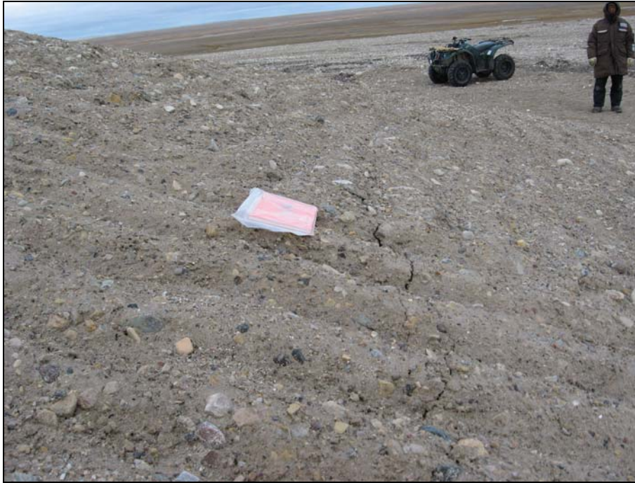
Photograph 25. Tension crack approaching the SE corner. Midslope tension crack continues around SE corner from where it turns north shifting to 1/3 up the slope. ↑
