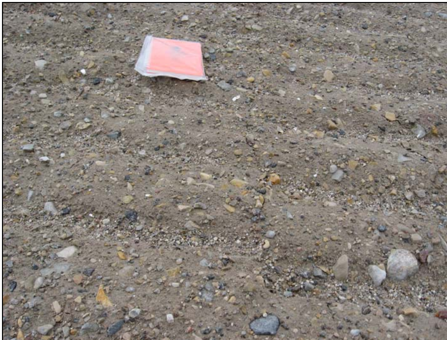
Photograph 20. Following a thin tension crack along west side of landfill from the NW corner. Crack runs parallel to slope about 4m upslope from downslope toe. Appears to continue from the north side of the landfill. ↑
