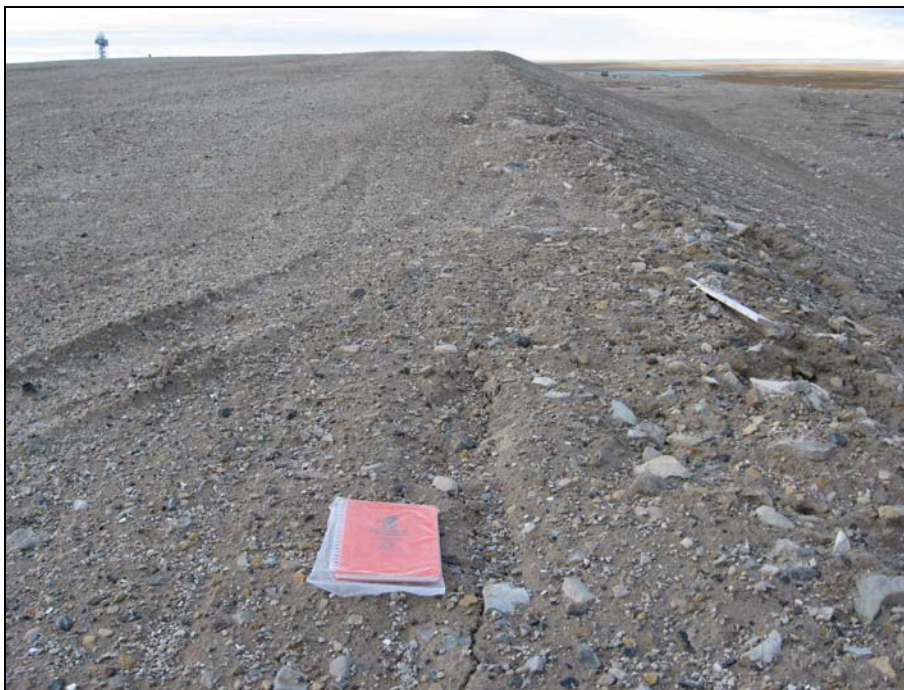
Photograph 30. Following tension crack N along east crest from Photo 29. ↑
