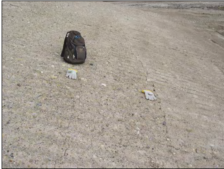
Photograph NH-13. Looking ENE at parallel cracks (old) approaching SE corner. Area of minor (self armoured) surficial erosion visible in background. Zone of erosion appears unchanged from the time of the 2007 inspection. ↑
