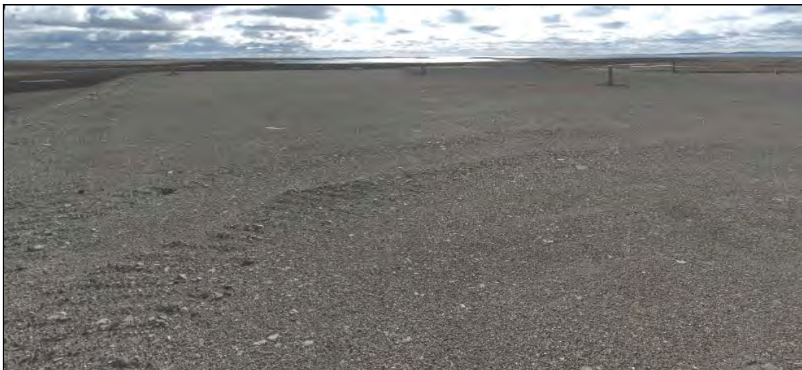
Photograph T2-15. Looking ESE from NW corner. Panoramic showing upper surface of landfill. Granular cover appears stable with no indications of problematic conditions. ↑
