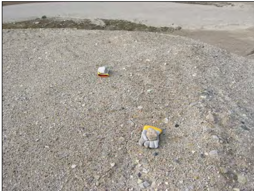
Photograph NH-20. Following crest crack to NE corner. Crack largely in-filled as it rounds corner. Faintly visible from about 30m W along N crest. ↑
