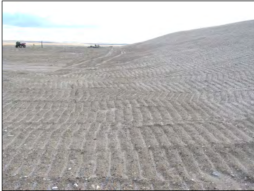
Photograph T2-5. Looking ESE along toe from NW corner of LF towards area where minor cracking was observed in 2007. The previously observed cracks (in foreground) are largely in-filled with sediments and show no indication of recent movement. ↑
