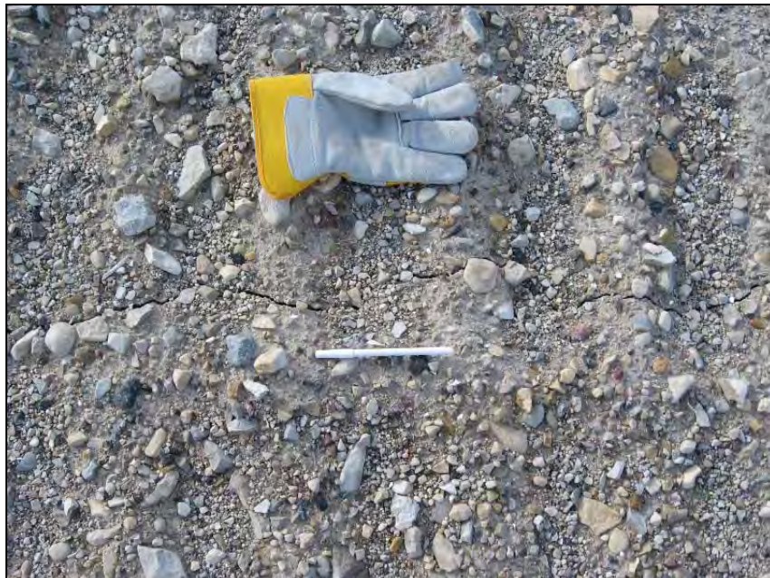
Photograph T2-20. Close-up of crack on N slope near NE toe. About 10m W of the NE corner of the landfill. Edges of the crack appear rounded (weathered) and portions of the crack are infilled with sediments. ↑
