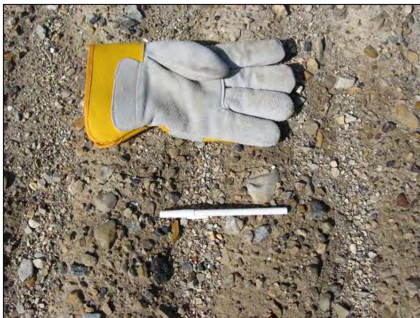
Photograph T2-16. Start of fine crack that runs from 20m S of NE corner to about 20m W of NE corner. 1 to 4mm wide, parallel to toe, 5 m upslope from toe, portions in-filled. Crack was observed in 2007 and appears to have stabilized. No indications of recent movement or degraded condition. ↑
