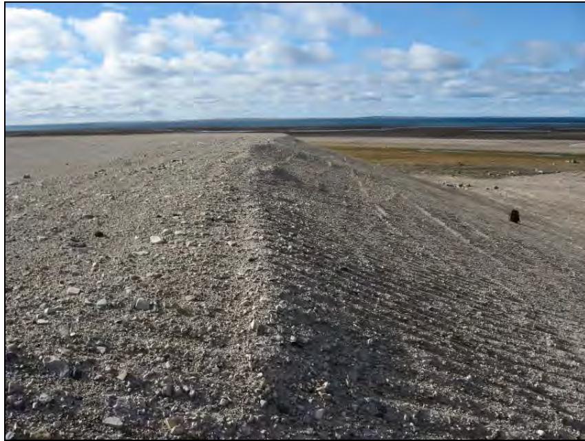
Photograph T2-7. Looking S along crest from NW corner. Minor cracks that were noted last year are barely visible and partially infilled. No sign of recent movement. ↑
