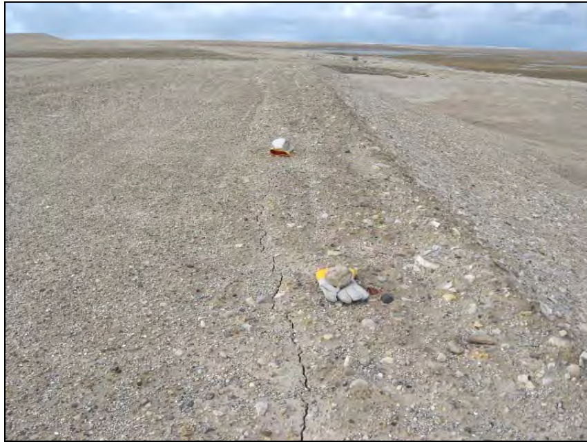
Photograph NH-19. Following crack on crest. Looking N approaching NE corner. ↑
