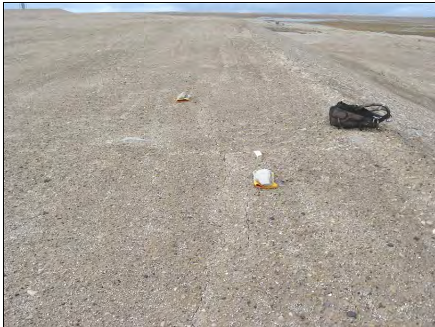
Photograph NH-18. Crack along E crest looking N. Similar to last year. Gloves on either side of crack. ↑
