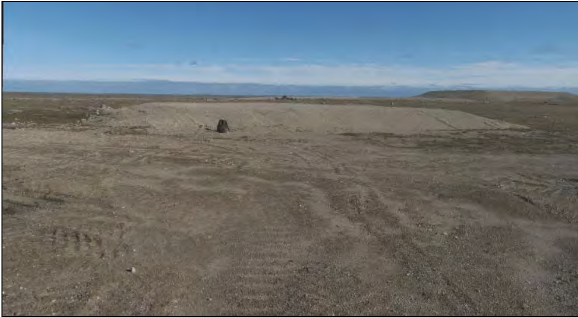
Photograph STA-13. Looking SE to the NW corner of the SE most of the two small landfill cells. Granular cover appears stable. No features of note. ↑
