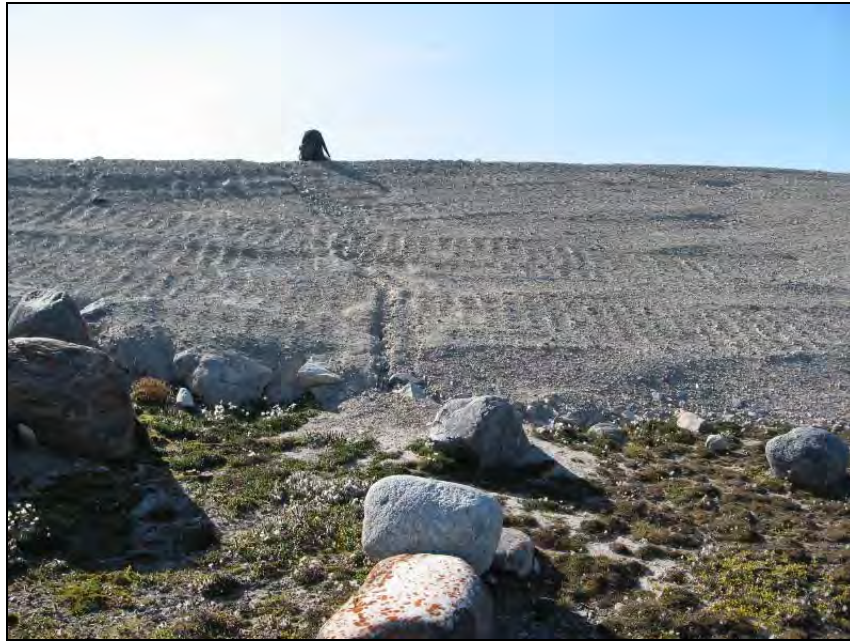
Photograph STA-3. Looking upslope to area of minor surficial erosion. Condition is essentially unchanged from last year. Granular cover is self-armouring. ↑
