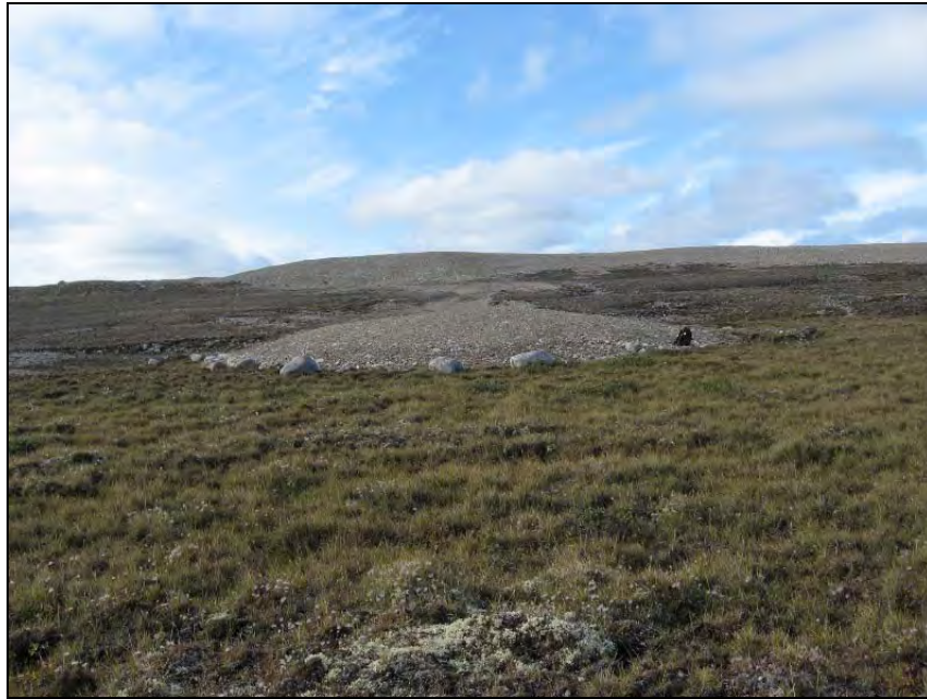
Photograph WLFN-15. Looking W to smallest SE cell. Granular cover appears stable. Long SW landfill cell visible in background. ↑
