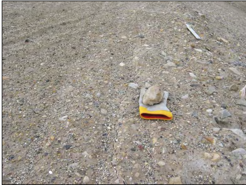
Photograph NH-17. Minor crack along crest (old) looking N. ↑
