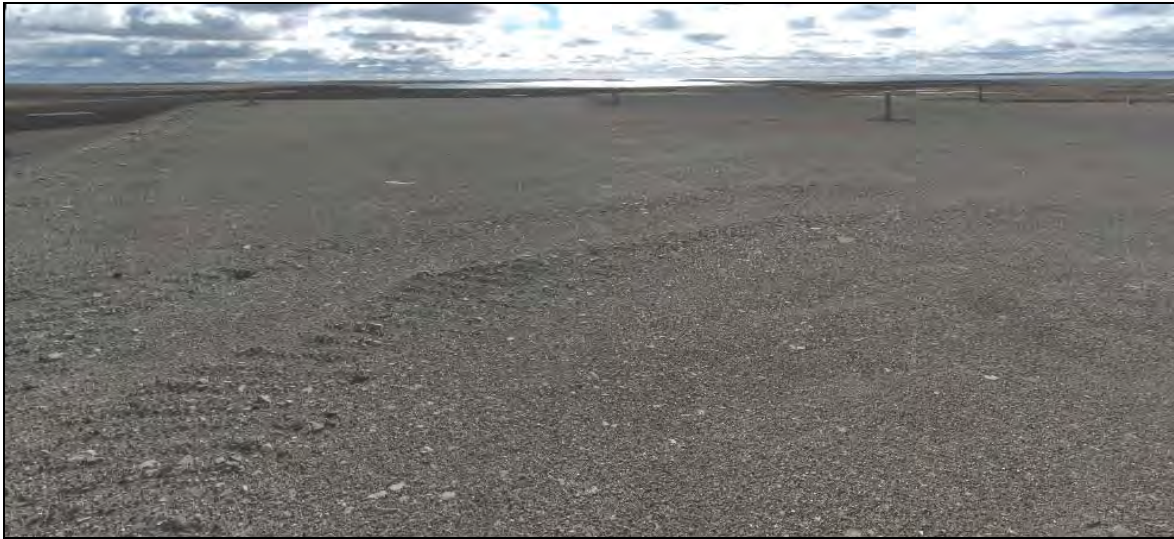
Photograph T2-15. Looking ESE from NW corner. Panoramic showing upper surface of landfill. Granular cover appears stable with no indications of problematic conditions. ↑
