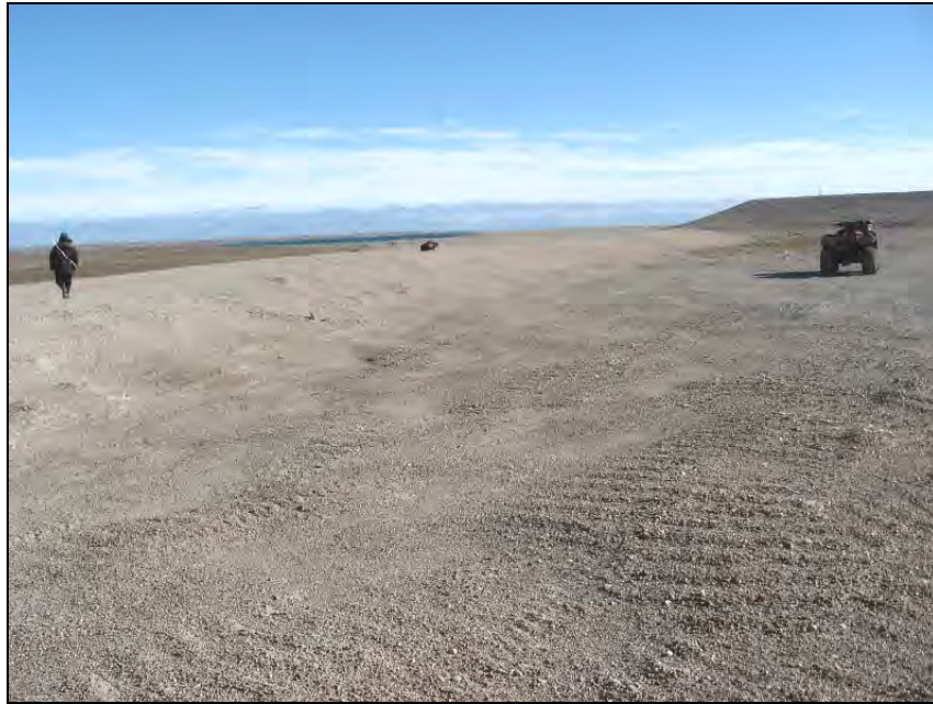
Photograph STA-9. Looking SSE along W side of the main cell of the Station landfill to the SW corner. Minor relief. Granular cover appears stable. ↑
