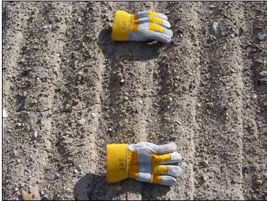
Photograph T2-27. Close-up of representative crack. This crack continues, splaying into two parallel cracks, 1m to 2m apart, and back again along entire toe of slope. Crack was observed in 2007 and shows no indication of recent movement. ↑
