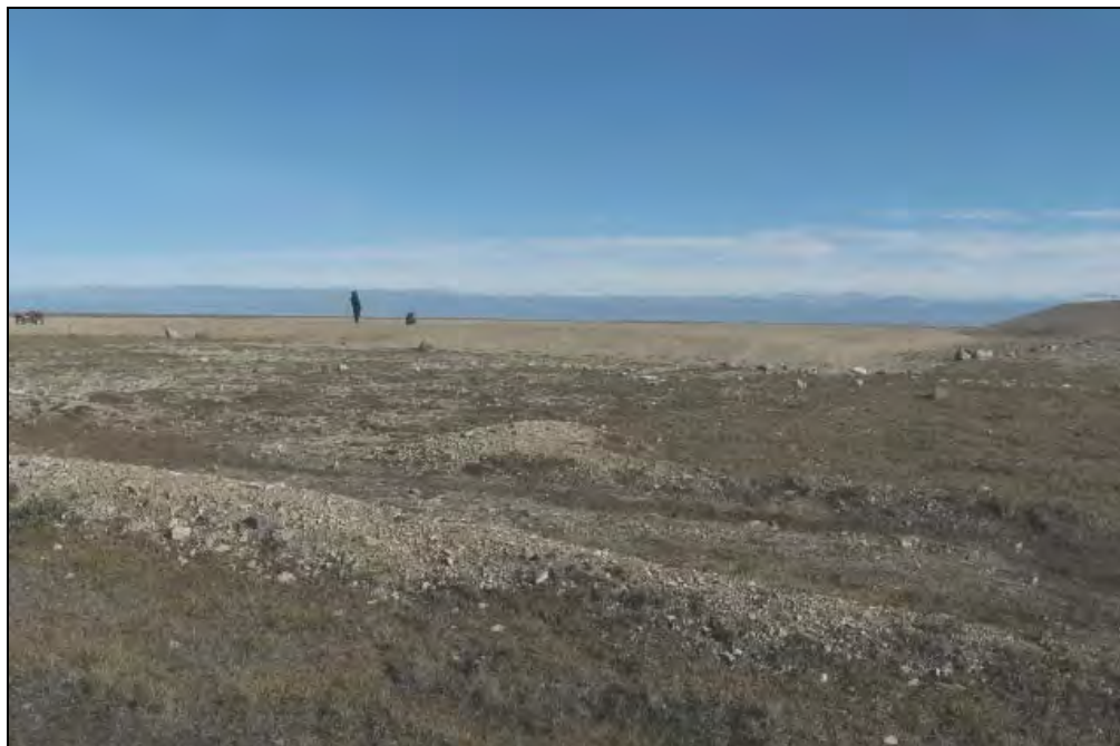
Photograph STA-10. Looking E to NW corner of the small SW cell of the Station Landfill. Granular cover appears stable. Honda parked adjacent to main cell on the extreme left of the photo. Tier II landfill (NE corner) visible in the background. ↑
