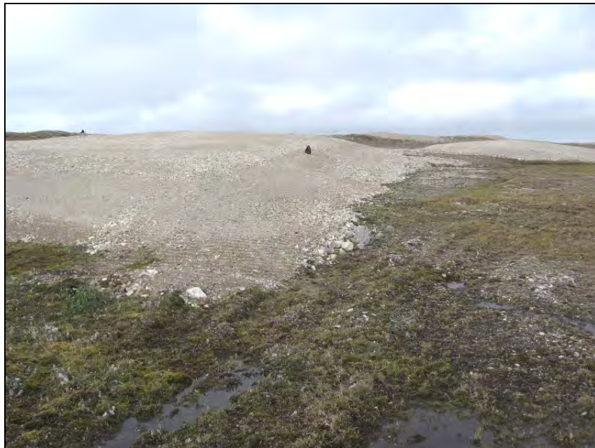
Photograph WLFS-8. Looking NW along east side of 3rd cell from NE corner of large S cell. Granular cover appears stable. ↑
