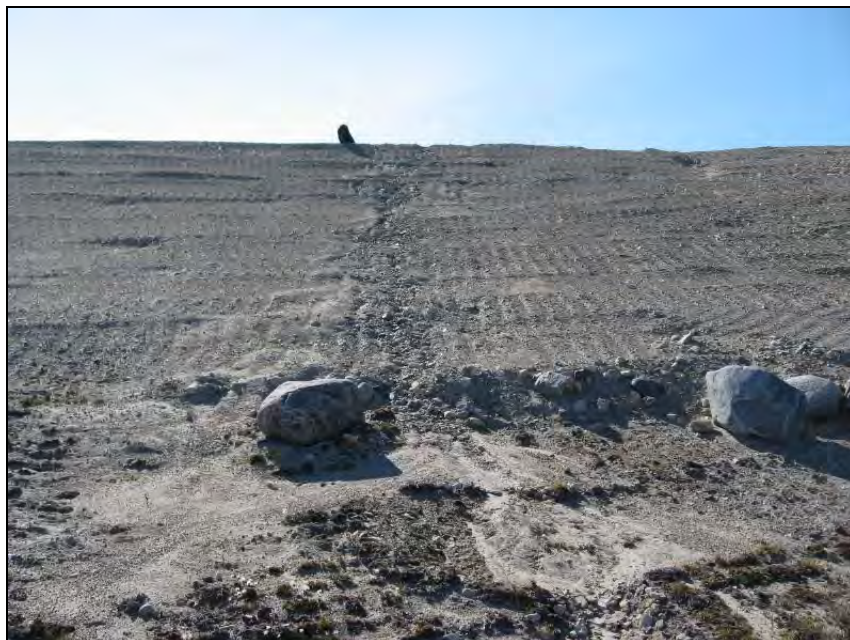
Photograph STA-4. Looking upslope to area of minor surficial erosion. Condition is essentially unchanged from last year. Granular cover is self-armouring. ↑
