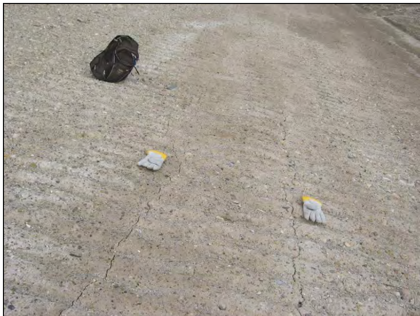
Photograph NH-12. Looking ENE at parallel cracks (old). ↑
