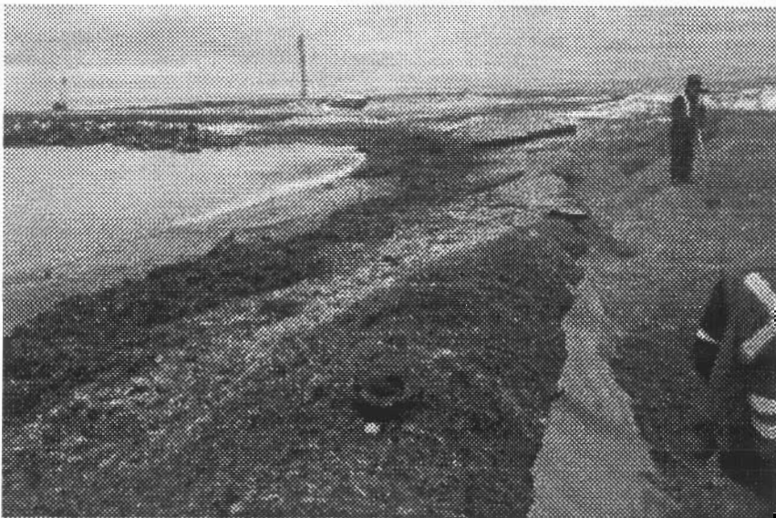
Photograph 10: Installation of geomembrane, east side of excavation
