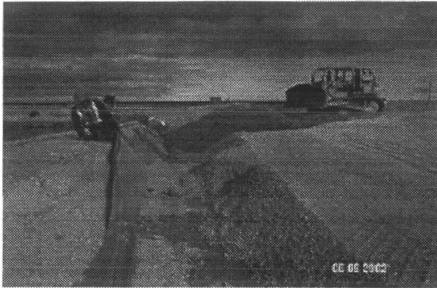
Photograph 9: Installation of Geomembrane around refuel lines
