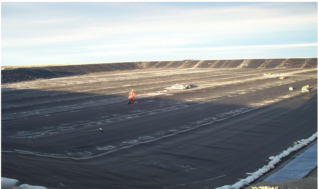
Photo 2: Cell 2 of the Tier II Soil Disposal Facility
