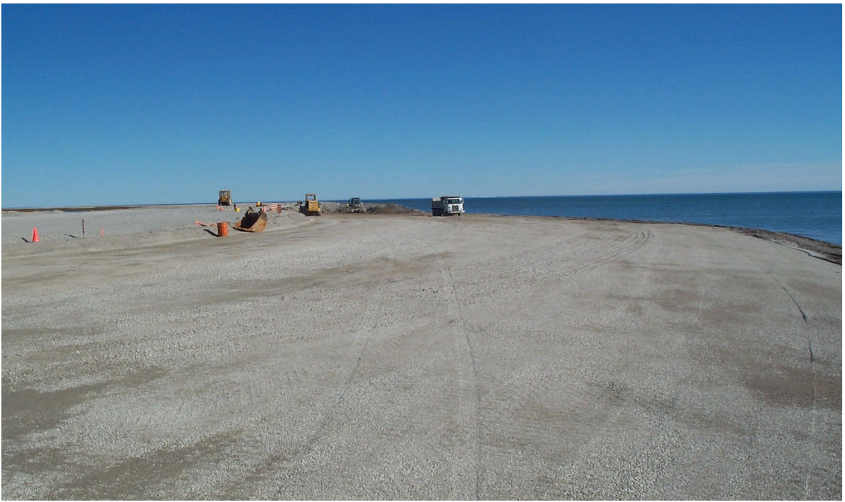
Photo 4: East Beach Landfill (Area 8) – backfill completion
