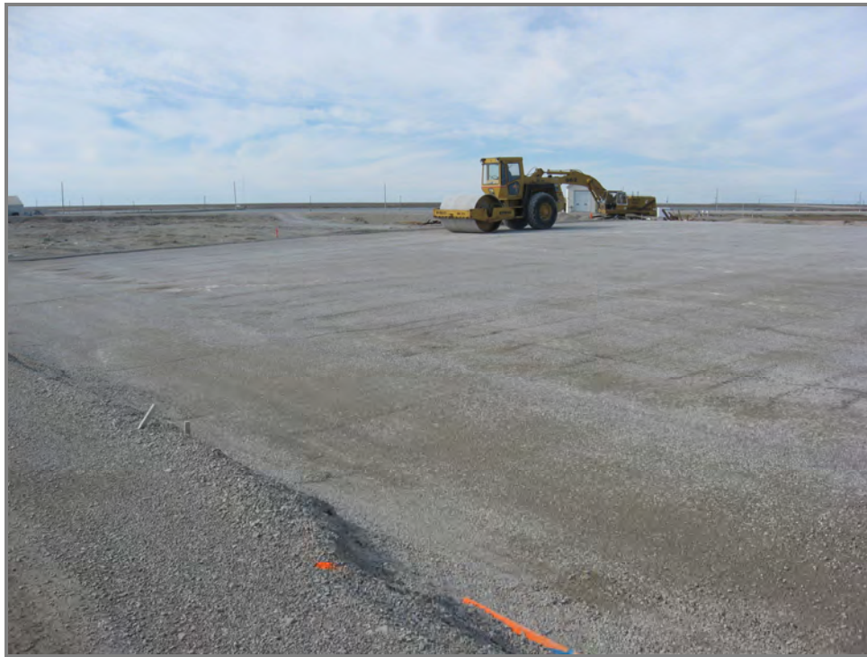
Picture #15 - Construction of Final Cover Layer of NHW Landfill, Viewing North West – August 8, 2007
