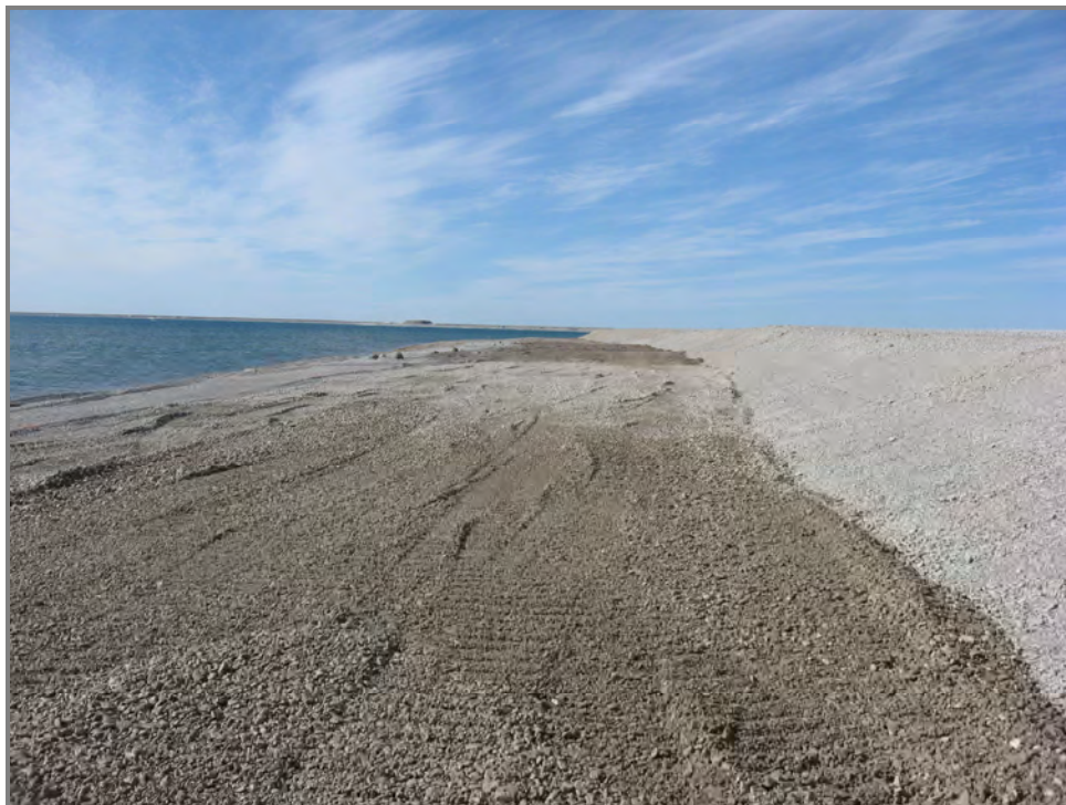
Picture #6 - Placement of Granular Fill to Promote Positive Drainage at the East Beach Landfill, Viewing West – July 12, 2007
