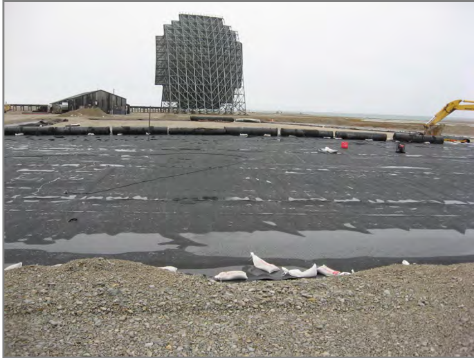
Picture #5 - Installation of Cover Liner of Tier II Disposal Facility, Viewing North – August 25, 2007
