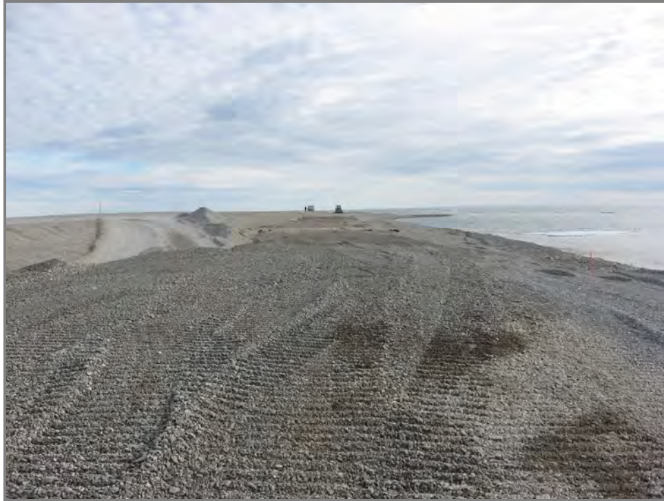
Picture #7 - Placement of Type 3 Granular Fill to Promote Positive Drainage at the East Beach Landfill, Viewing East – July 13, 2007
