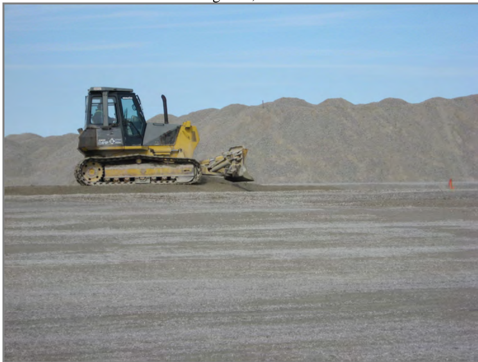
Picture # 16 - Construction of Final Cover Layer of NHW Landfill, Viewing North East – August 8, 2007
