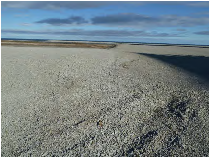
Photograph 18. Communications North Landfill: Settlement on south side slope (Photo 418)↑
