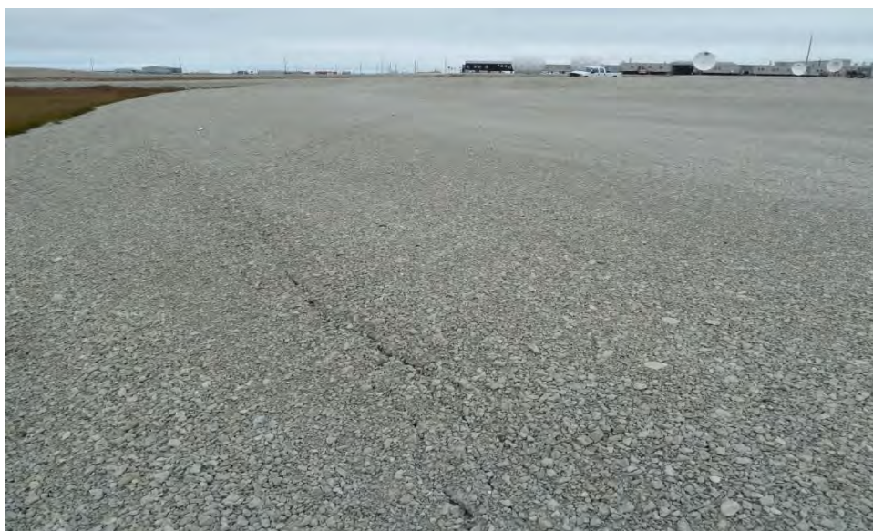
Photograph 8. G217 West Landfill: Looking N at Cracking Along the W Side Slope of Landfill (Photo 475)↑
