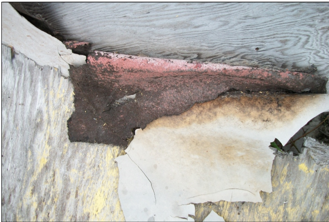
Photo 160 Hope Lake WK027: APEC 3C, linoleum sampled and does not contain asbestos
