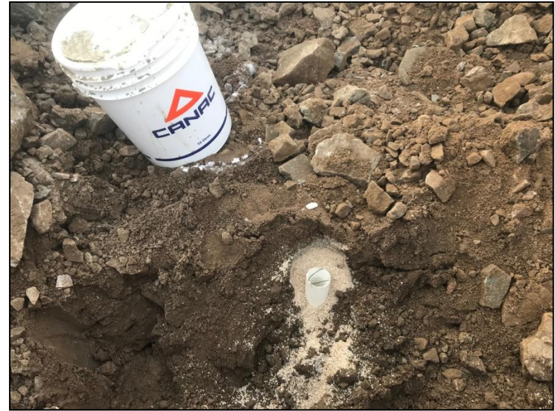
Photo 2: PVC cut below ground surface
