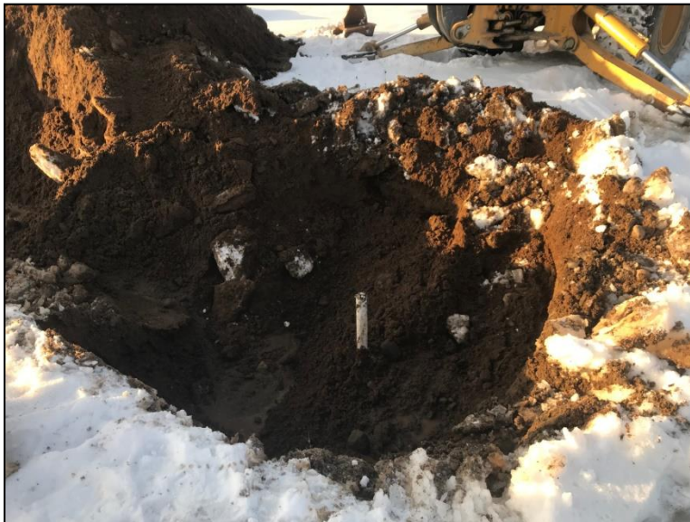
Photo 7: MW19-03 casing excavation
