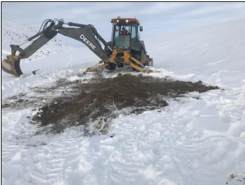
Photo 3: Excavation to grade following MW19-01 decommissioning
