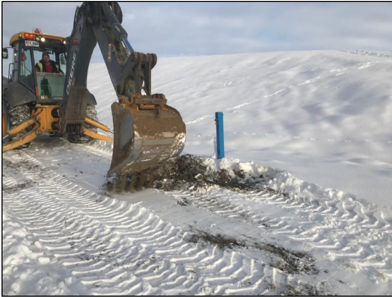
Photo 1: Metal Casing Excavation MW19-01
