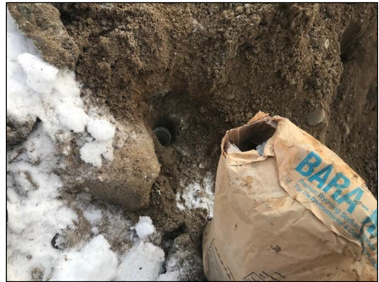
Photo 6: Filling MW19-02 with bentonite chips
