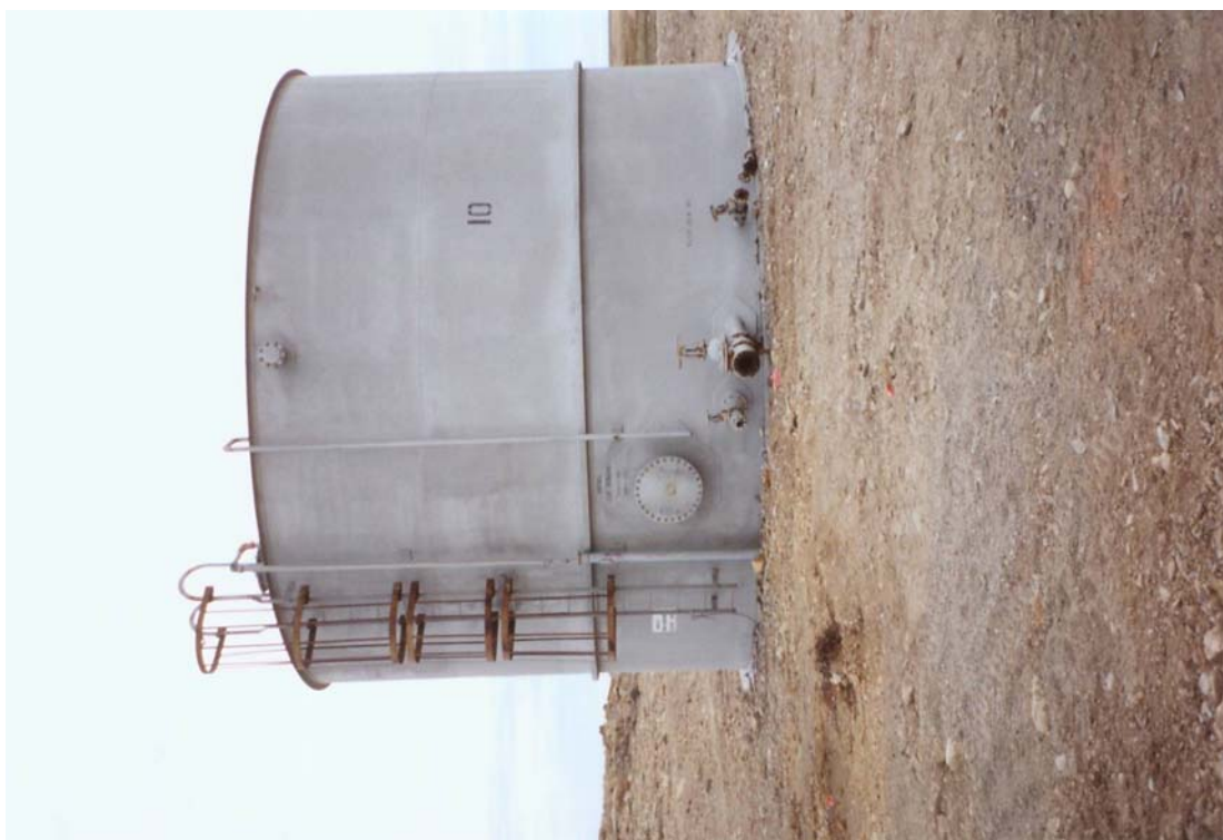
Photo 52: 65,000 gallon diesel tank (typical).
