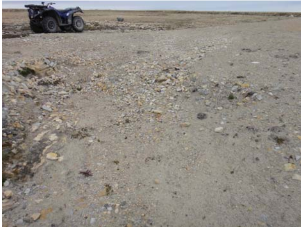
MLF-7: (left) View north at minor erosion on northwest corner (Feature D).
