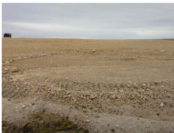
SWLF-6: (left) View looking northeast at minor depressions on side slope (Feature A).
