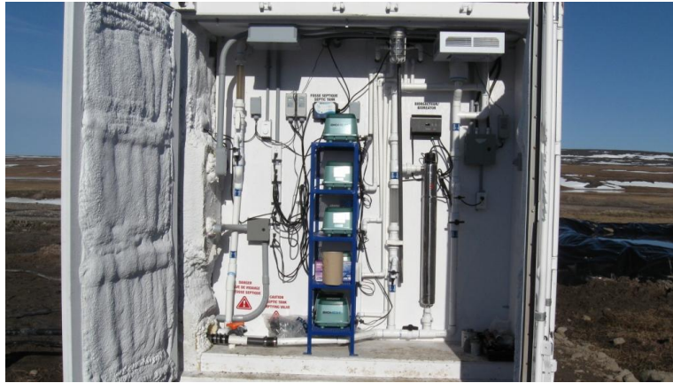
Insulated Bionest used at the CAM-D project, Simpson Lake
