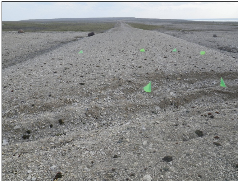
Photo 1: Washout of main access roadway between Area 1 and Area 2; south aspect.
