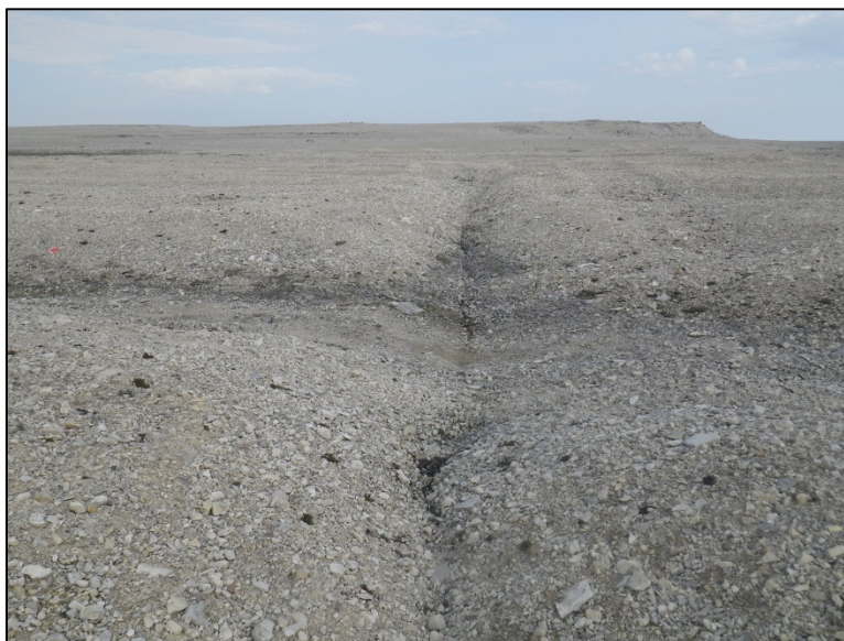
Photo 3: Washout of main access roadway between Area 1 and Area 2; east (upstream) aspect.
