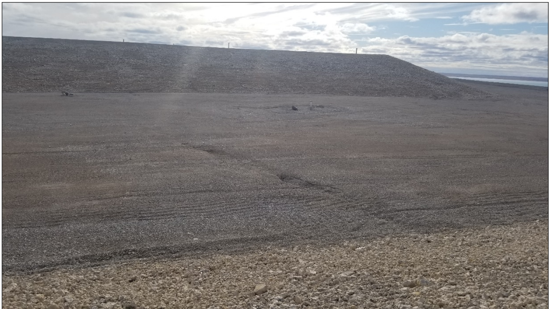
Photo 6: Crack adjacent to Non-Hazardous Waste Landfill.
