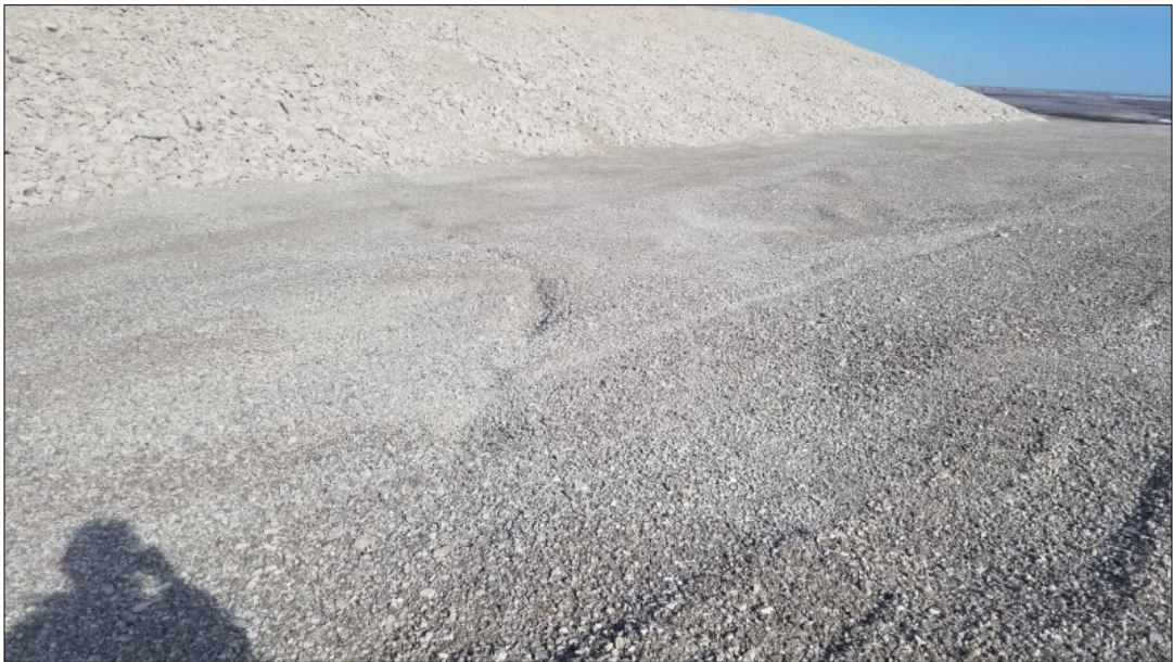
Photo 2: Crack adjacent to Tier II Landfill.
