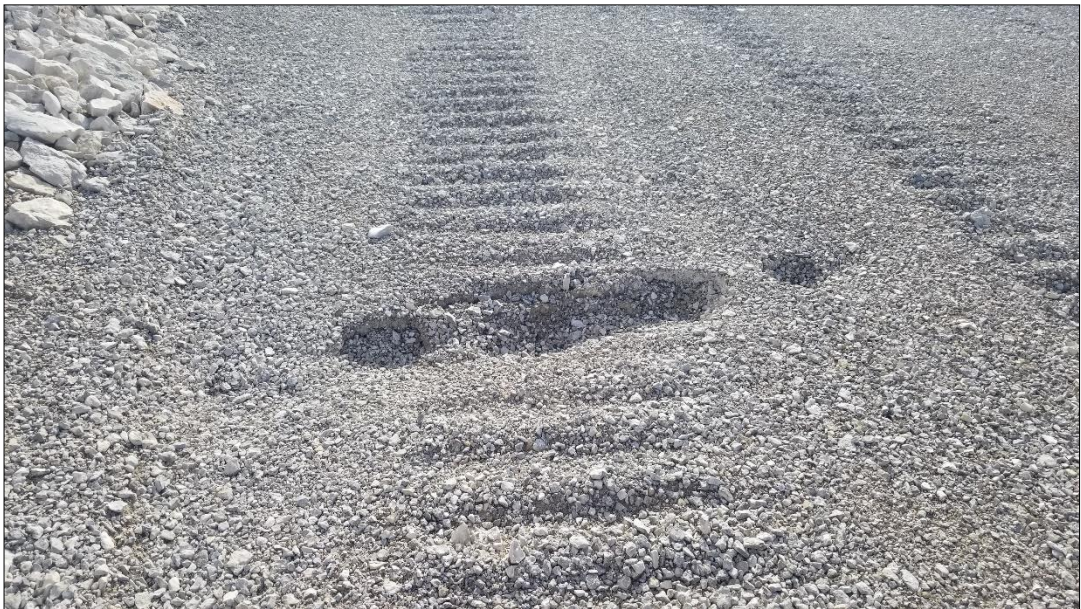
Photo 3: Crack Northwest of Tier II Landfill.
