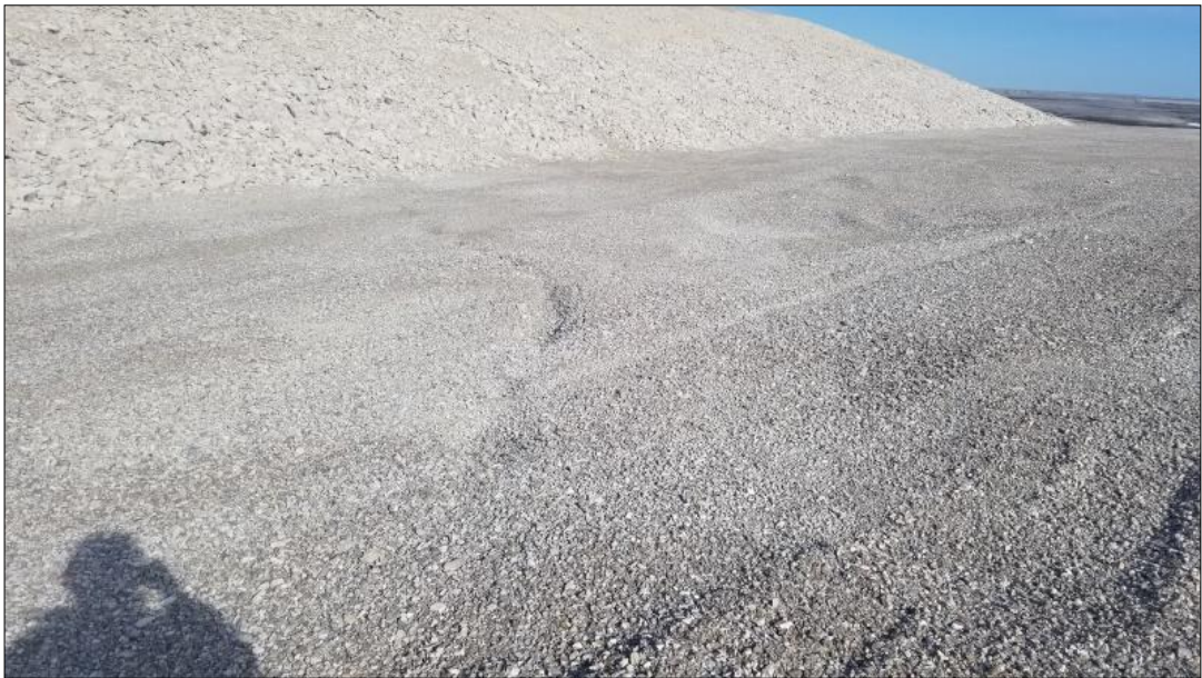
Photo 2: Crack adjacent to Tier II Landfill.
