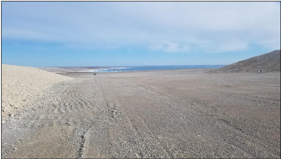
Photo 9: Washboard South of Non-Hazardous Waste Landfill.
