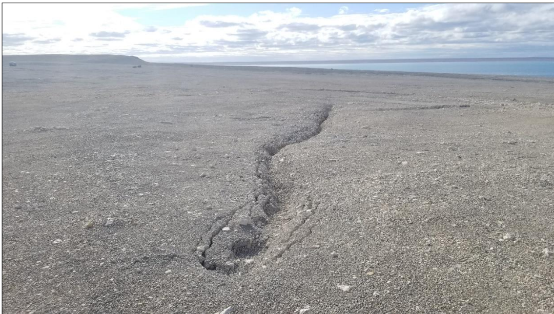
Photo 8: Large Crack West of Non-Hazardous Waste Landfill.
