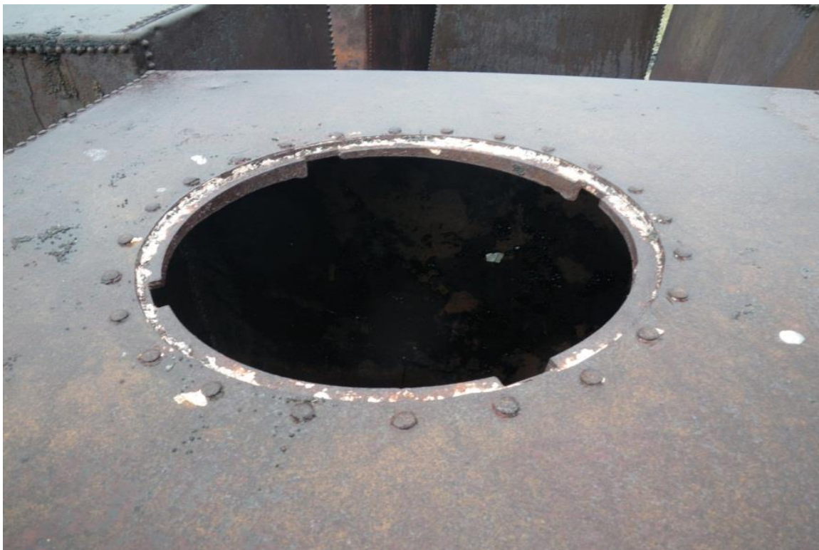
Plate 22: Detail of the closure on the boilers.
