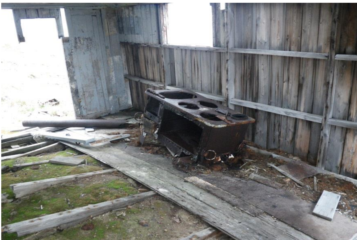
Plate 25: Photo of the interior of the cabin showing dimensional lumber framing and cast iron stove.
