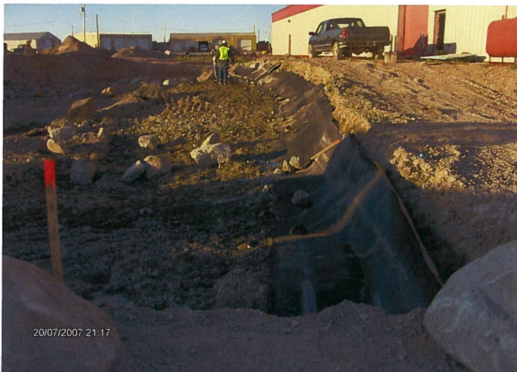
Photo 3: View of the southern portion of the Recreation Complex excavation. Note geomembrane liner along the south wall.
