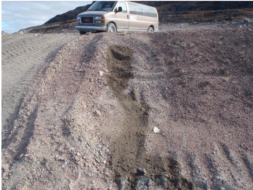
Photo 4: View of the stains on the inside of the treatment cell berm – September 2011.
