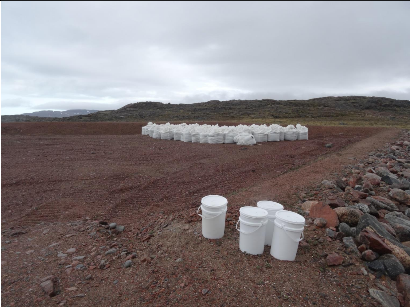
Description: Top half of Upper Cell containing Mega Bags of Contaminated Soil
